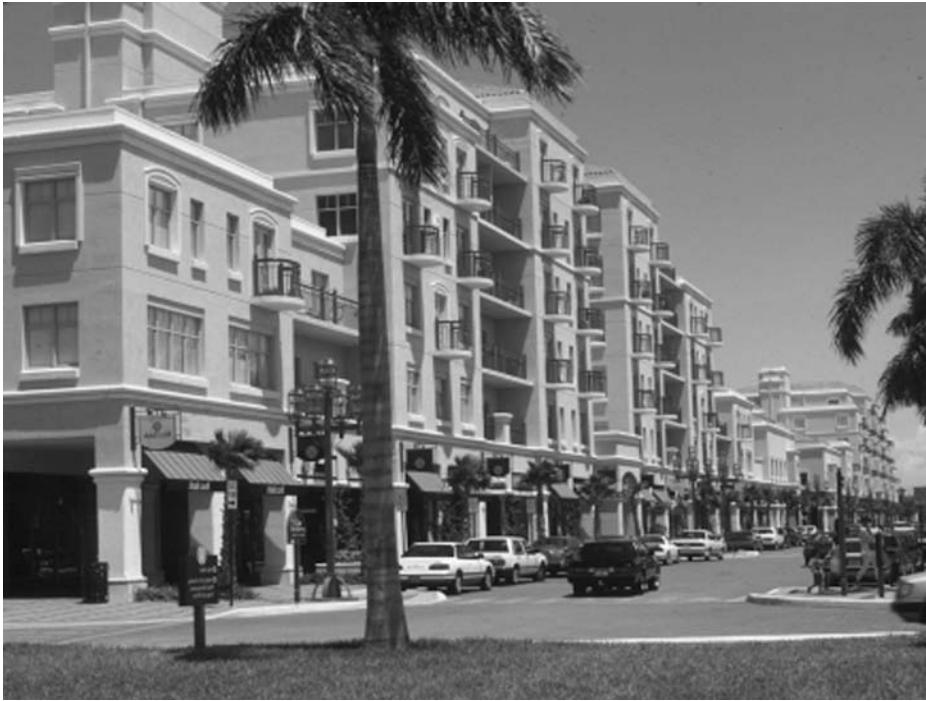
Figure 10-9 Rectilinear framework organizes the massing and articulation of the mixed-use Mizner Court building in Boca Raton, Florida.
