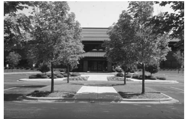
Figure 10-26 Walkway within a parking lot separates pedestrians from vehicle traffic.
