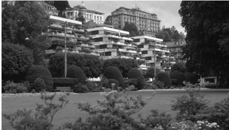
Figure 9-7 Building “steps back” from the street, reducing its scale at the street level, while improving solar access and creating useable outdoor terrace space for each residential unit in Zurich, Switzerland.
