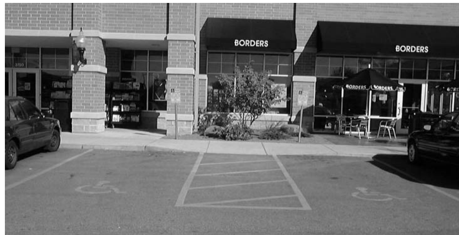
Figure 10-19 Direct access provided from a disabled parking space to an adjacent walkway.
