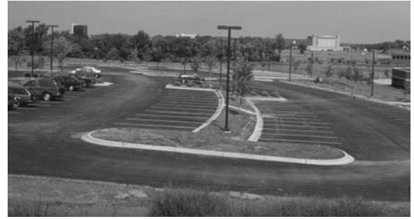
Figure 10-29 Parking lot on a sloping site. The planted island reduces the cross-slope or gradient of the adjacent parking bays.
