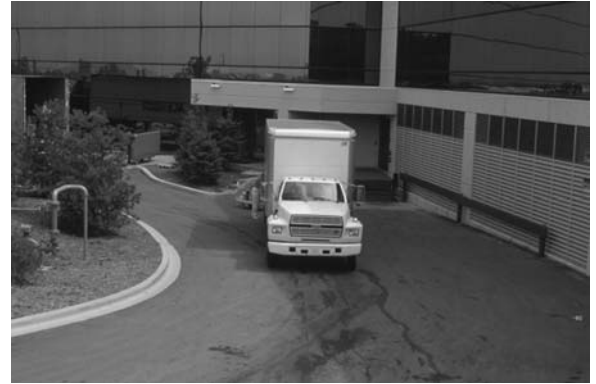
Figure 10-32 Recessed loading dock for a suburban office building.
