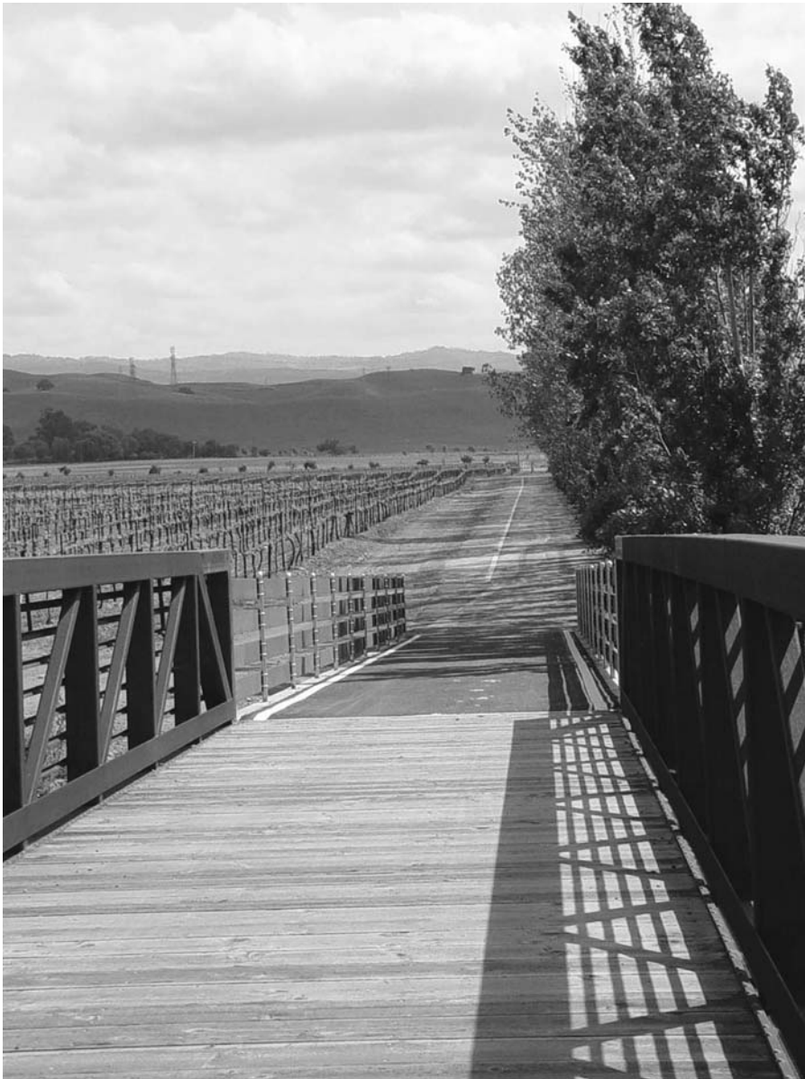
Figure 8-23 The plan contributed 6.5 miles of new multiuse trails that extend the length of the valley, connecting the new neighborhoods and creating an important recreational resource for the broader community. Source: Wallace Roberts & Todd, LLC.
