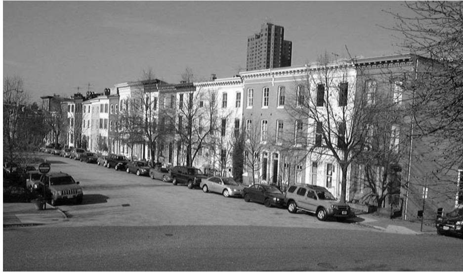
Figure 10-4 Unity at the street block scale: historic townhouses in Baltimore, Maryland. Note: repetition of vertical lines and rectilinear forms and openings (windows and doors) with nearly equal sizes and proportions.
