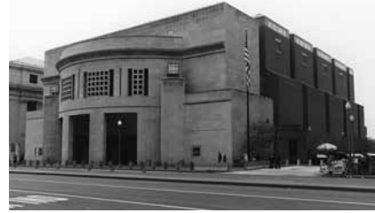
3.16 14th Street entrance in the existing building
