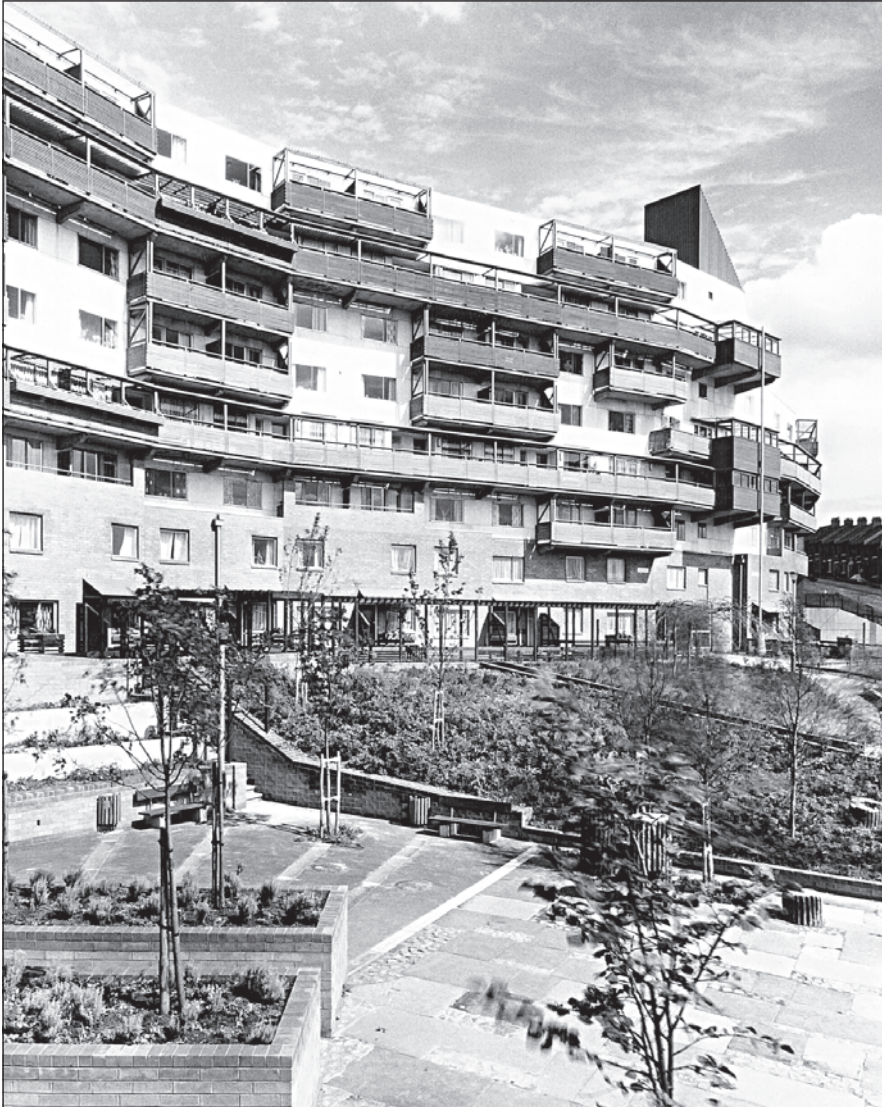
Figure 4.2: The Byker 'wall' redevelopment, Newcastle upon Tyne – the multi-storey element of a predominantly low-rise development. The 'wall' was the key to ensuring the existing community could be kept together
