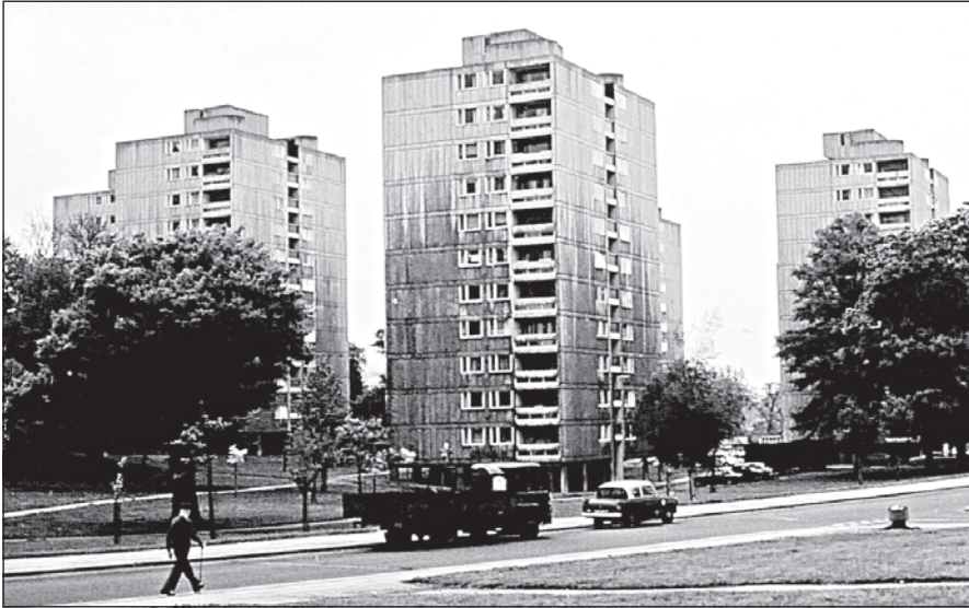
Figure 2.10: Alton West Estate, Roehampton (1952-60). Alongside slab blocks inspired by Le Corbusier are point blocks, such as these, influenced by Swedish punkthus
