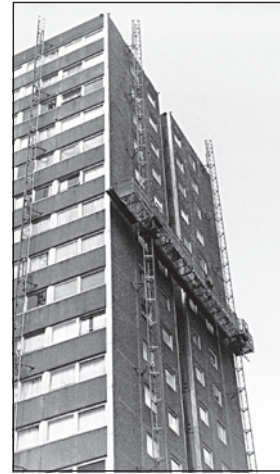
Figure 6.1: Harvist Estate, Islington. (above) Panels fixed by a 'mast climber' create a new, lightweight external skin (left)
