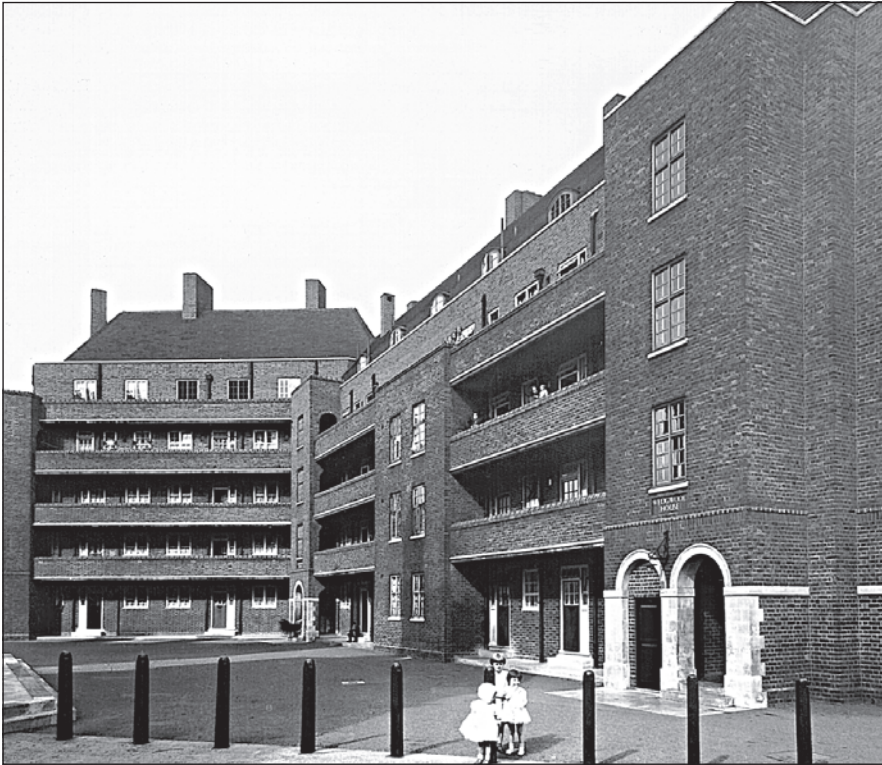
Figure 2.6: China Walk, Lambeth, slum clearance scheme (1934). Typical of the balcony access tenement blocks built in the inter-war period
