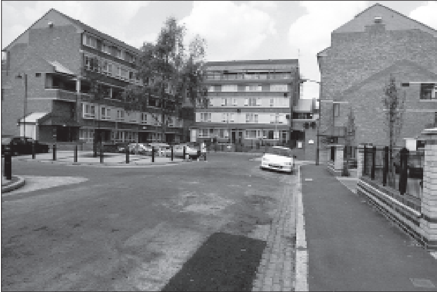
Figure 8.4: North Peckham Estate, Southwark. Improved courtyard on Phase 2
