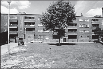
Figure 5.2: Bentham Court, Islington. (left) Unimproved block and (below) similar block after modernisation
