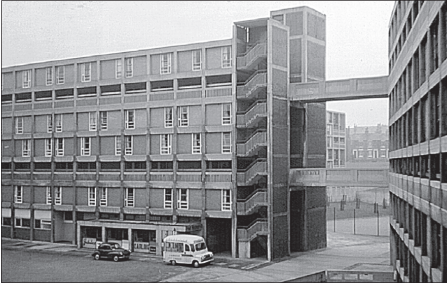
Figure 2.12: Park Hill, Sheffield completed early 1960s. The first large scheme to realise the ‘streets in the sky’ concept. Pedestrian decks link all the blocks together, bridging across at several levels
