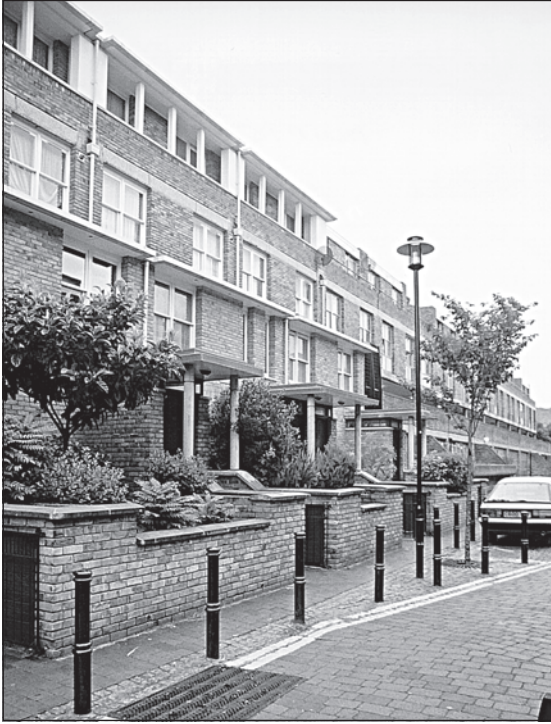
Figure 6.3: Angell Town Estate, Lambeth. Foreground, the modernised housing with ground level access. Beyond, the unimproved flats reached by a walkway with garages at ground level
