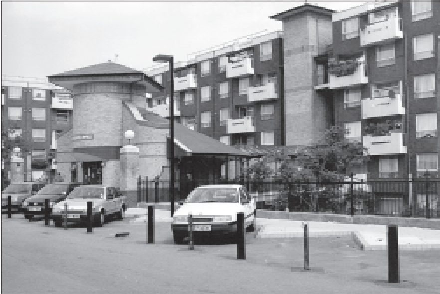
Figure 8.2: Packington Estate, Islington. New estate office, entrance and lift shaft
