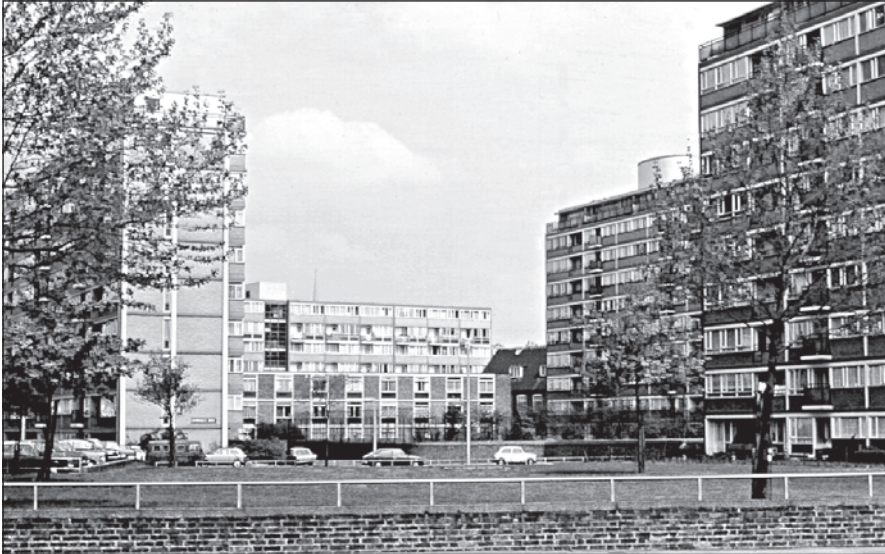
Figure 2.9: Churchill Gardens, Westminster (1946). The scheme was the first in Britain to follow the Zeilenbau principle. All the large blocks are orientated strictly on a north–south axis, disregarding and destroying the building’s relationship with the street
