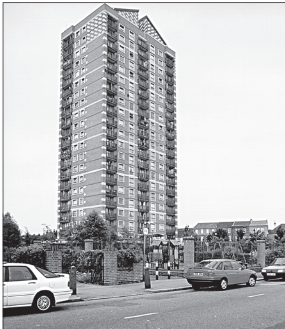
Figure 6.2: Northwood Tower, Waltham Forest. Heavy overcladding with a new skin of traditional brickwork and replacement windows
