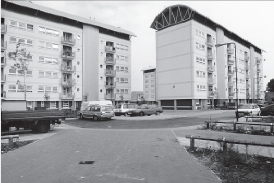
Figure 8.5: Priory Court Estate, Waltham Forest. Blocks improved with new roofs, windows and cladding
