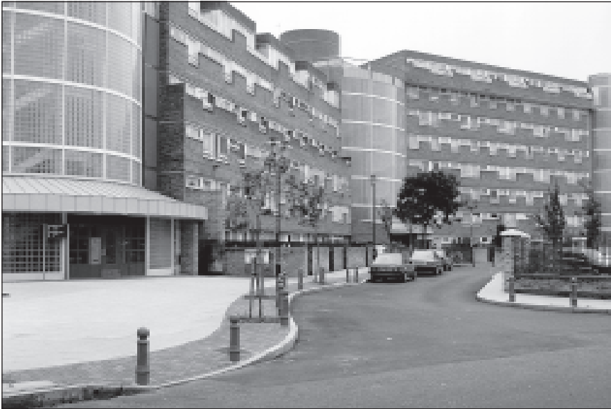
Figure 8.3: Gloucester Grove Estate, Southwark. North façade showing new entrance enclosures
