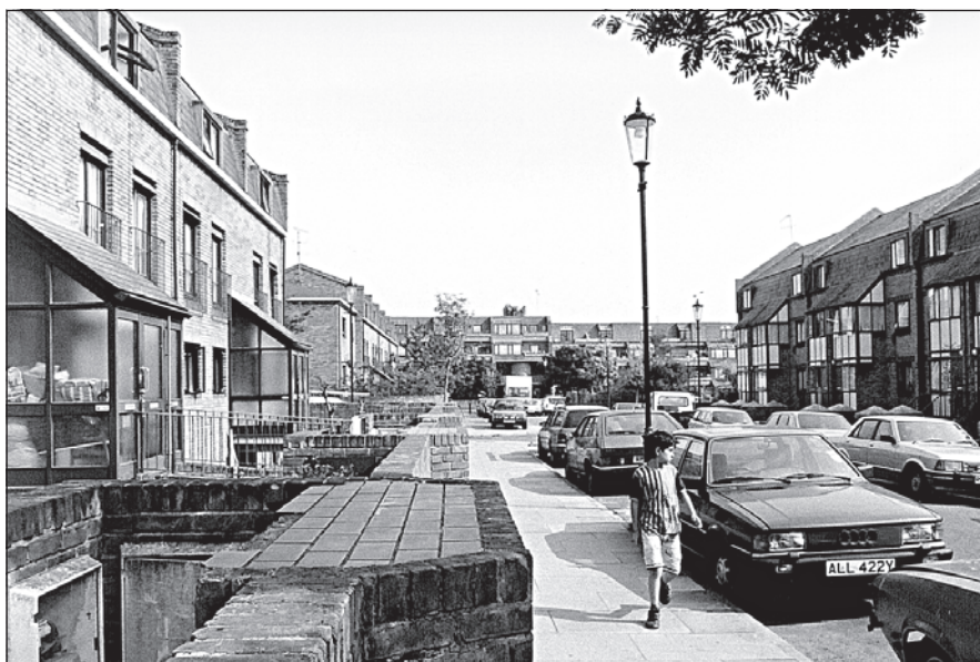
Figure 4.3: Swinbrook, North Kensington. As a result of a prolonged resident campaign the area was redeveloped as four-storey flats and maisonettes on the existing street pattern
