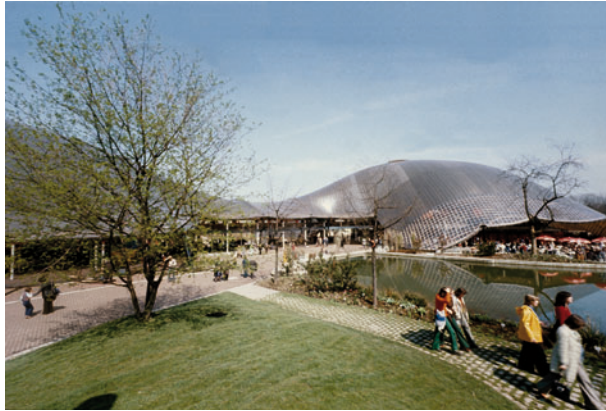
Figure 19.1 The gridshells for the Mannheim Multihalle
