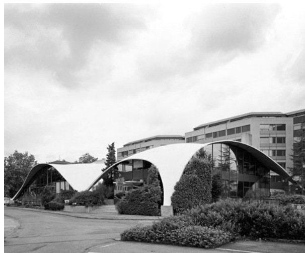
Figure 20.16 Sicli Company Building, Geneva, 1969
