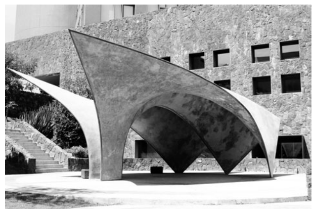
Figure 9.11 (top) Mexico City shell with bent pipe edge curves and timber waffle formwork and (bottom) resulting concrete shell canopy
