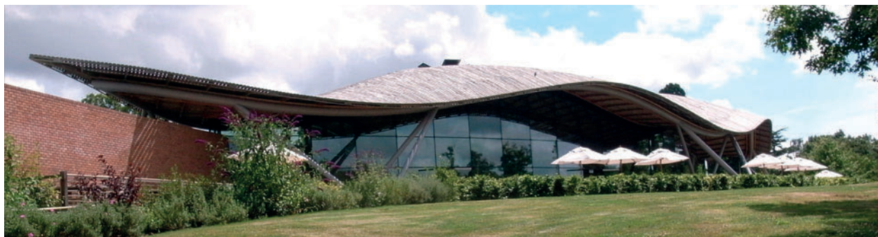
Figure 8.1 The gridshell roof of the Savill Building at the Windsor Great Park, UK, 2006
