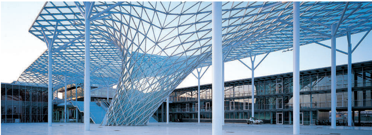
Figure 15.1 Roof of the New Trade Fair, Rho-Pero, Milan, Italy, 2002–2005, by Massimiliano and Doriana Fuksas architects, with a grid mapping onto a complex surface
