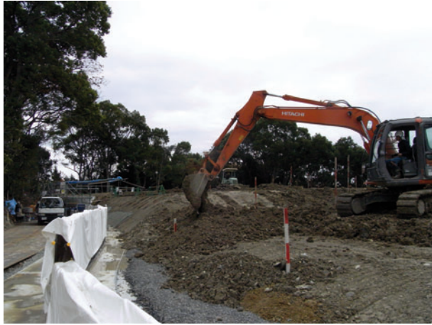
Figure 21.14 Formation of the earth-filled formwork
