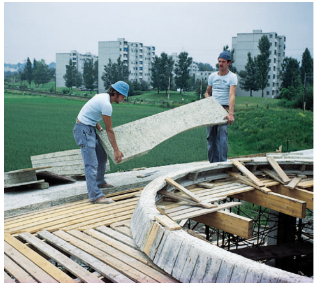
Figure 20.18 Leuzlinger Sons Building, 1979. Isler standing beside glued laminated timber arches, and formwork of fibreboard insulation placed on wooden boards
