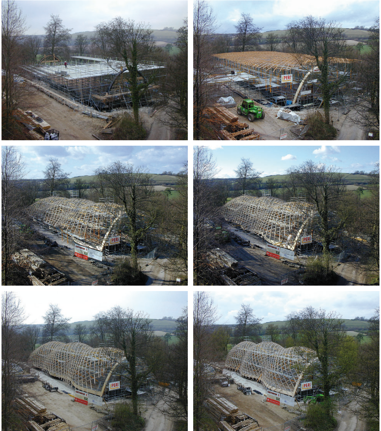
Figure 8.13 The lowering process for the Downland gridshell
