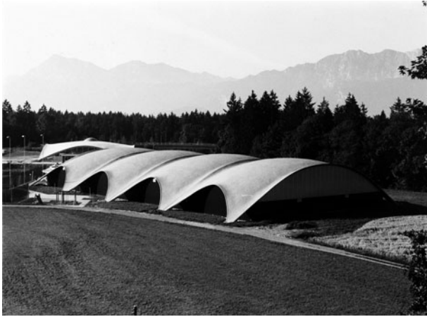
Figure 20.17 Heimberg tennis court shells, 1979
