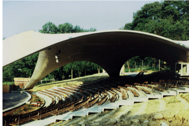
Figure 3.14 Aichtal Outdoor Theatre with a ‘lip’ at the free edges, Germany, 1977
