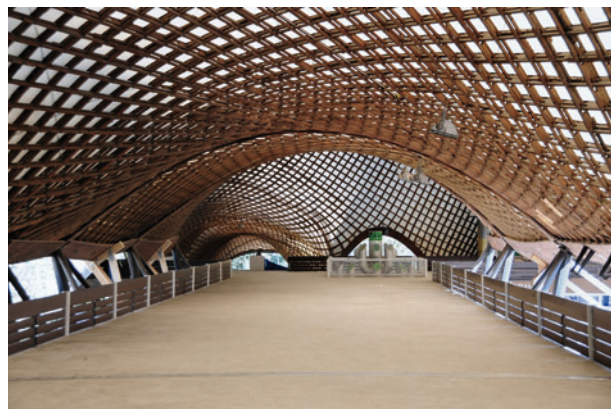
Figure 12.1 The Multihalle in Mannheim, 1976, an application of nonlinear FDM
