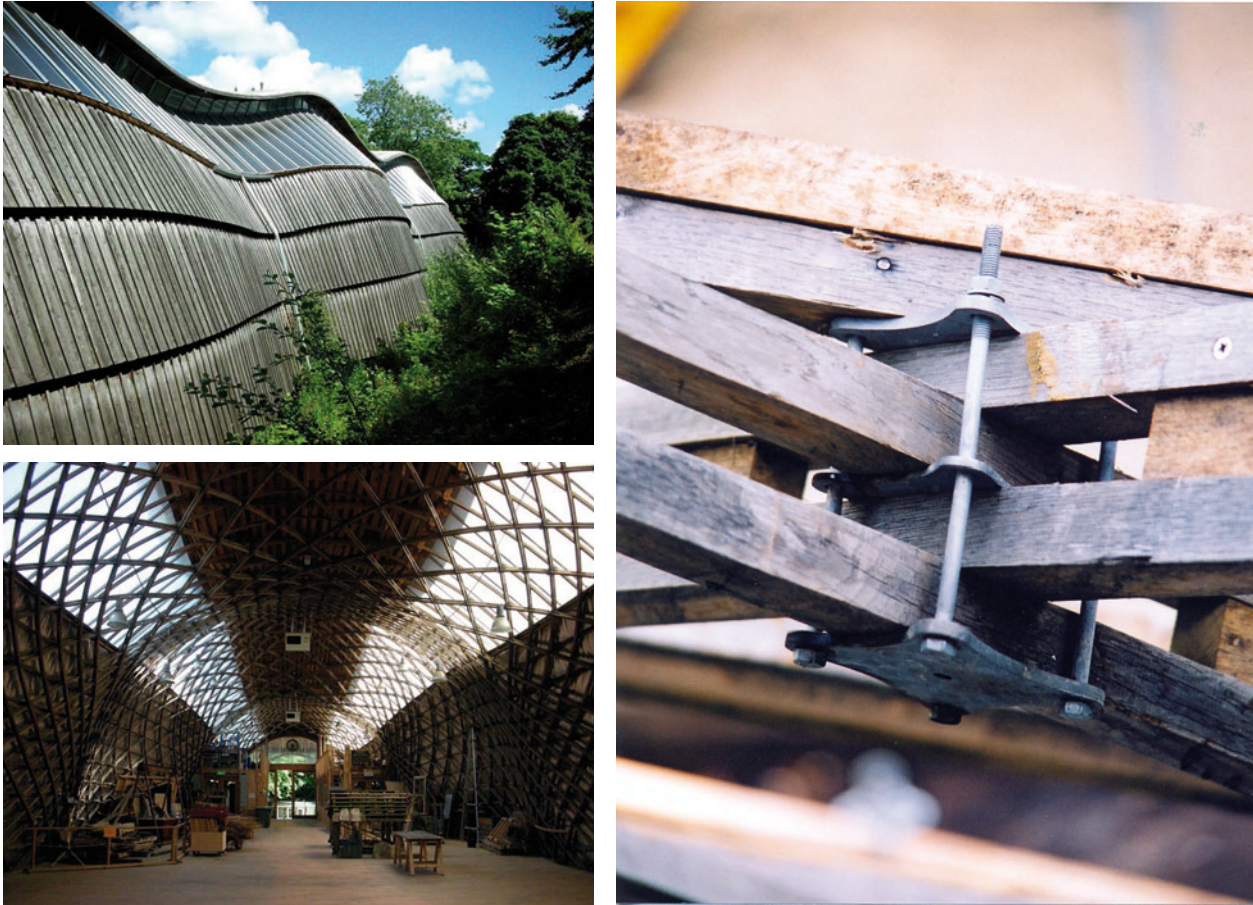
Figure 8.12: Downland gridshell, Chichester, UK, 2002, with (top left) western red cedar cladding, (bottom left) housing a workshop and (right) detail of connectors
