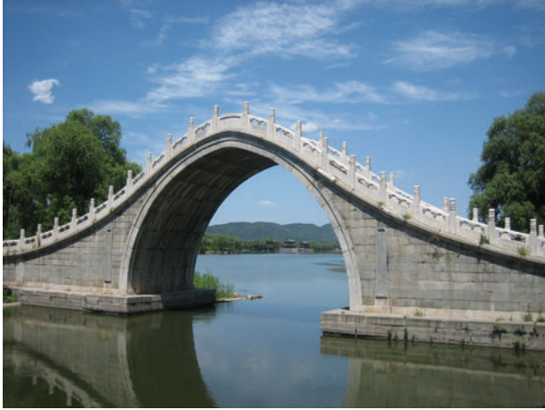
Figure 3.10 (left) The Gaoliang Bridge of the Summer Palace, Beijing, 1751–1764, resembles (right) a funicular circular arch of increasing thickness
