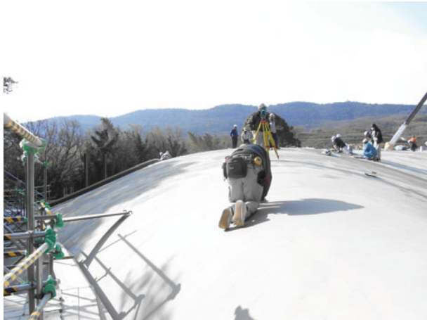
Figure 21.15 Shape measurement of the formwork
