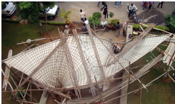
Figure 9.10 On-site fabric guidework with rebar in place
