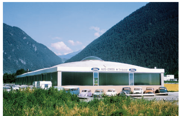
Figure 20.9 Pneumatic form roof. (top) Interior of the Eschmann Company, 1958, and (bottom) exterior of one of Isler's designs with prestressed tension ties concealing the shell's thickness
