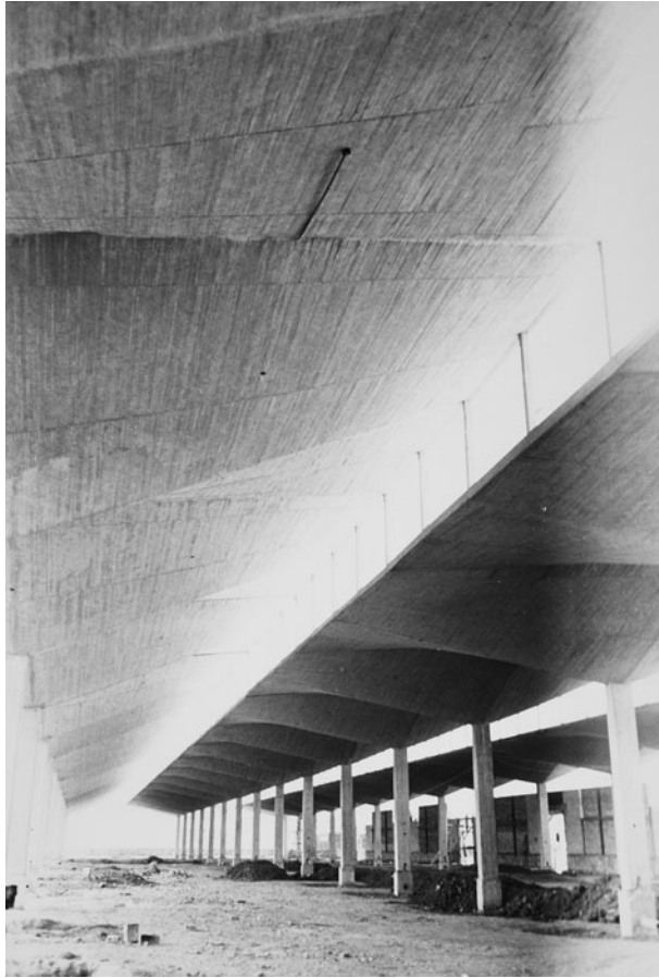
Figure 20.7 A series of umbrellas comprising Rio's Warehouse, Mexico City, 1954
