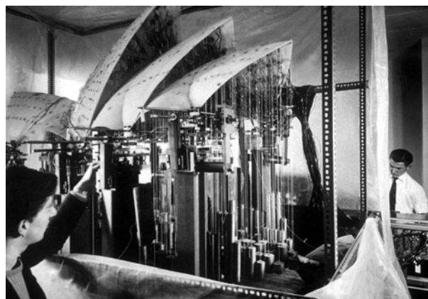
Figure 4.10 A 1:60 scale model of a thin-shell version of the Sydney Opera House roof being tested at the University of Southampton
