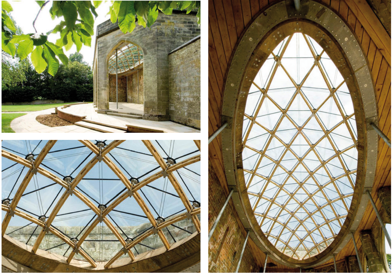
Figure 8.4 The double-layer gridshell with external bracing of the Chiddingstone Orangery in Kent, UK, 2007
