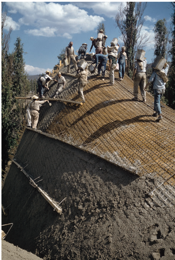
Figure 20.15 Laborers placing buckets of concrete on the shell for Los Manantiales Restaurant (see Fig. 20.10)
