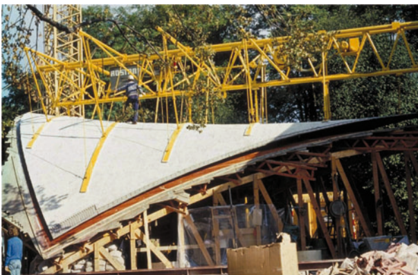
Figure 0.1 Bundesgartenschau Pavilion, with a 12mm fibre reinforced concrete shell, Stuttgart, 1977
