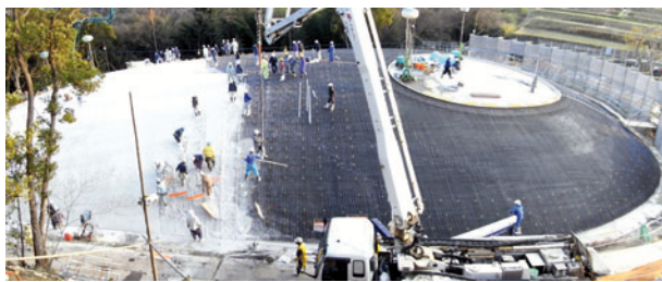
Figure 21.16 Concrete placement
