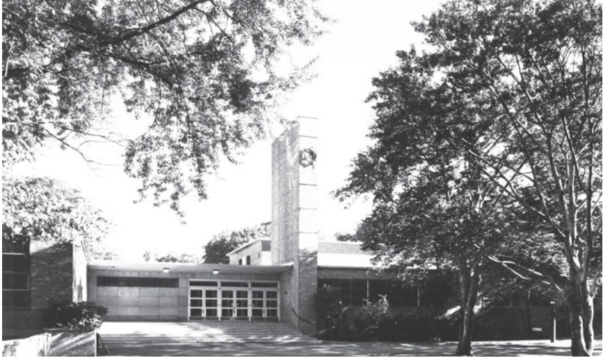
Figure 4. Crow Island School building entrance emphasized by a large vertical clock tower. (By Steven R. Turckes, AIA, LEED AP, REFP - Principal, Perkins + Will.)
