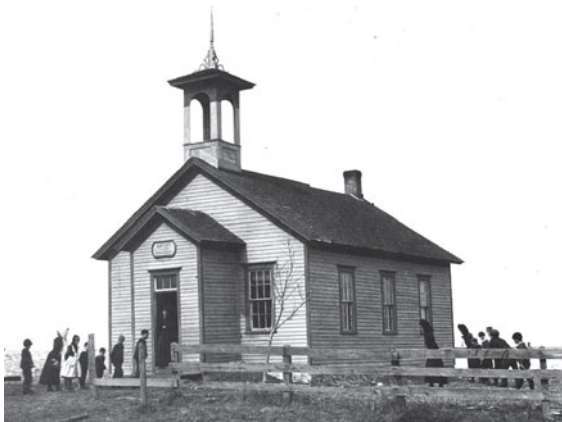
Figure 1. Bear Creek School (c. 1870), Iowa. (Iowa State Historical Society; Courtesy and permission of author Andrew Guildford (1984). America's Country Schools . National Trust for Historic Preservation.)
