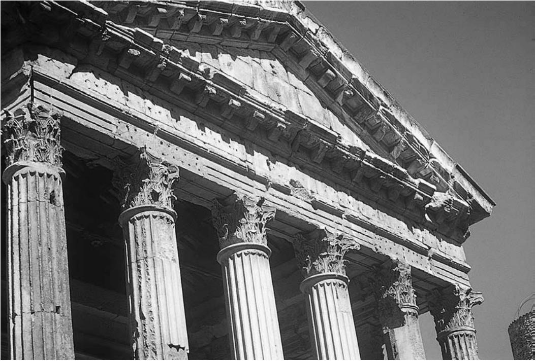
59 Detail of entablature showing clamp holes, temple at Vienne (photo by the author).
