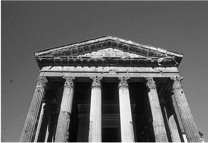
58 Façade of the temple at Vienne (photo by the author).
