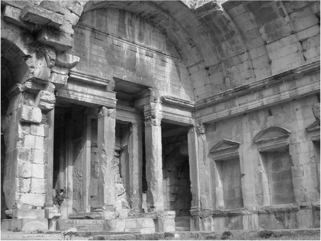
110 Rear wall of bibliotheca , with niches, staircase, and barrel-vaulted roof, Nîmes (photo by the author).
