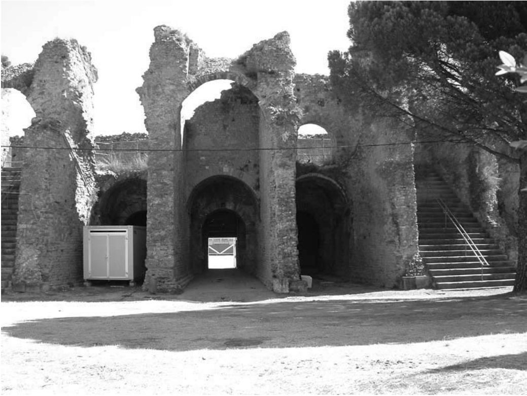
105 View of vaults beneath cavea , amphitheater at Fréjus (photo by the author).
