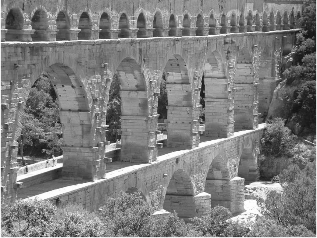
128 Superimposed vaults of the Pont du Gard (photo by the author).
