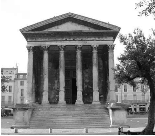
52 Façade and Corinthian order of the Maison Carrée (photo by the author).
