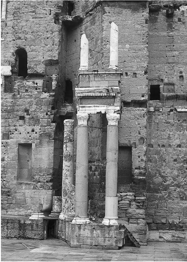
87 Columnatio as restored on scenae frons of the theater at Orange (photo by the author).
