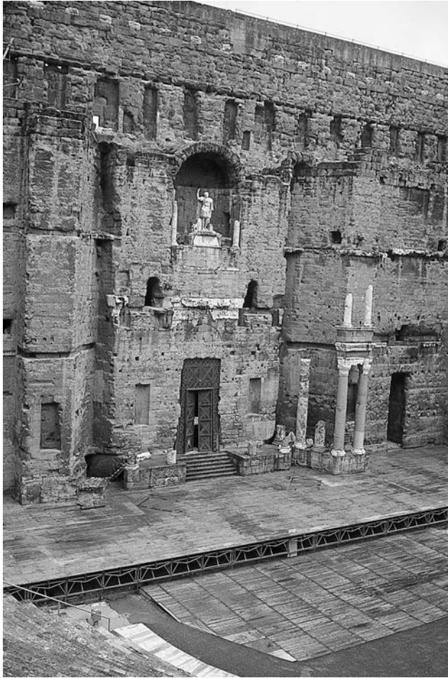
86 View of scenae frons as restored, theater at Orange (photo by the author).
