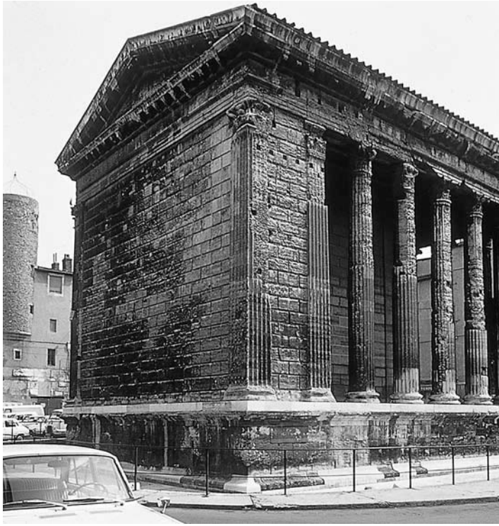
57 Flank and rear of the temple at Vienne, a peripteros sine postico (photo by the author).
