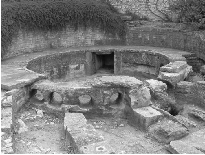
125 Castellum divisorium (distribution tank) of aqueduct at Nîmes (photo by the author).
