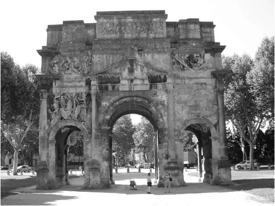
39 Orange arch, view of north face showing double attic (photo by the author).
