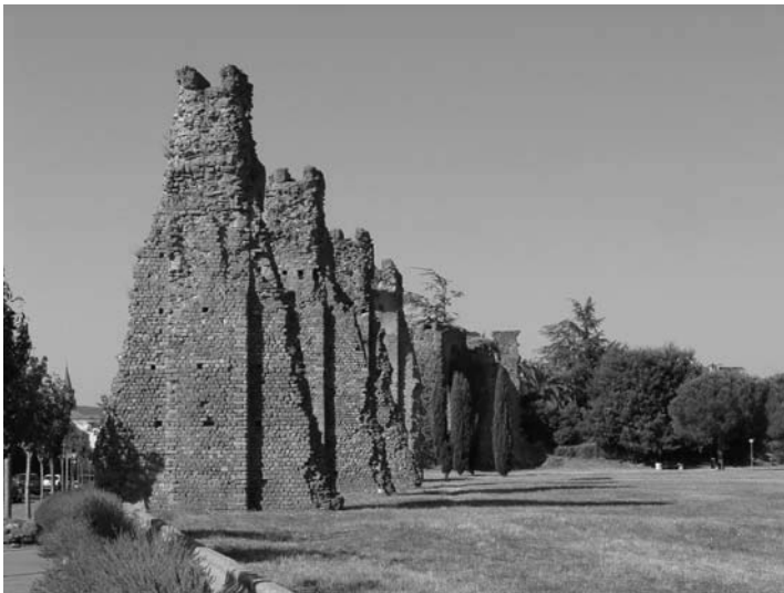
124 Aqueduct piers near the Roman walls of Fréjus (photo by the author).
