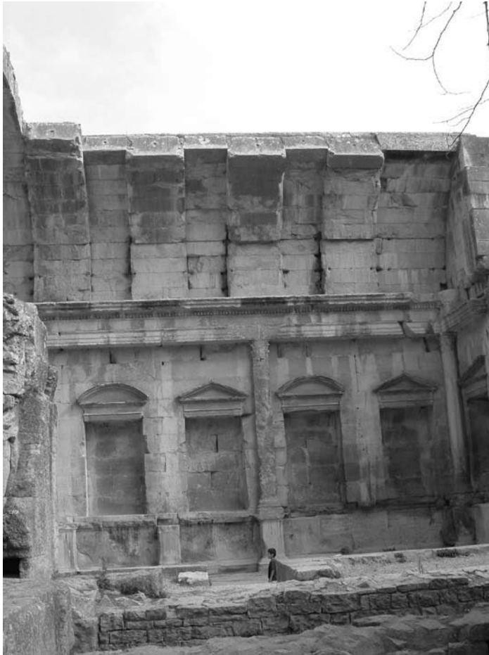
111 Niches lining flank walls of bibliotheca at Nîmes (photo by the author).
