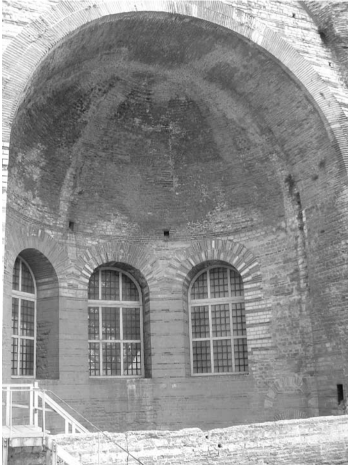
115 Interior cupola of caldarium , Constantinian baths at Arles (photo by the author).
