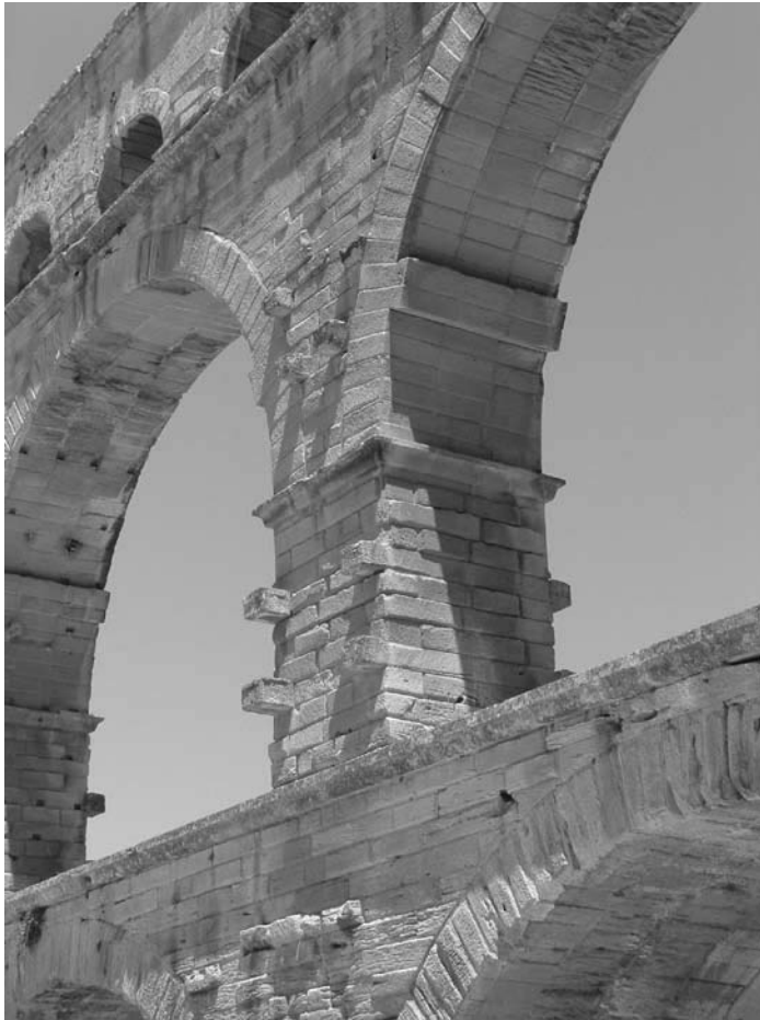
127 Detail of Pont du Gard, showing protruding stone bosses (photo by the author).
