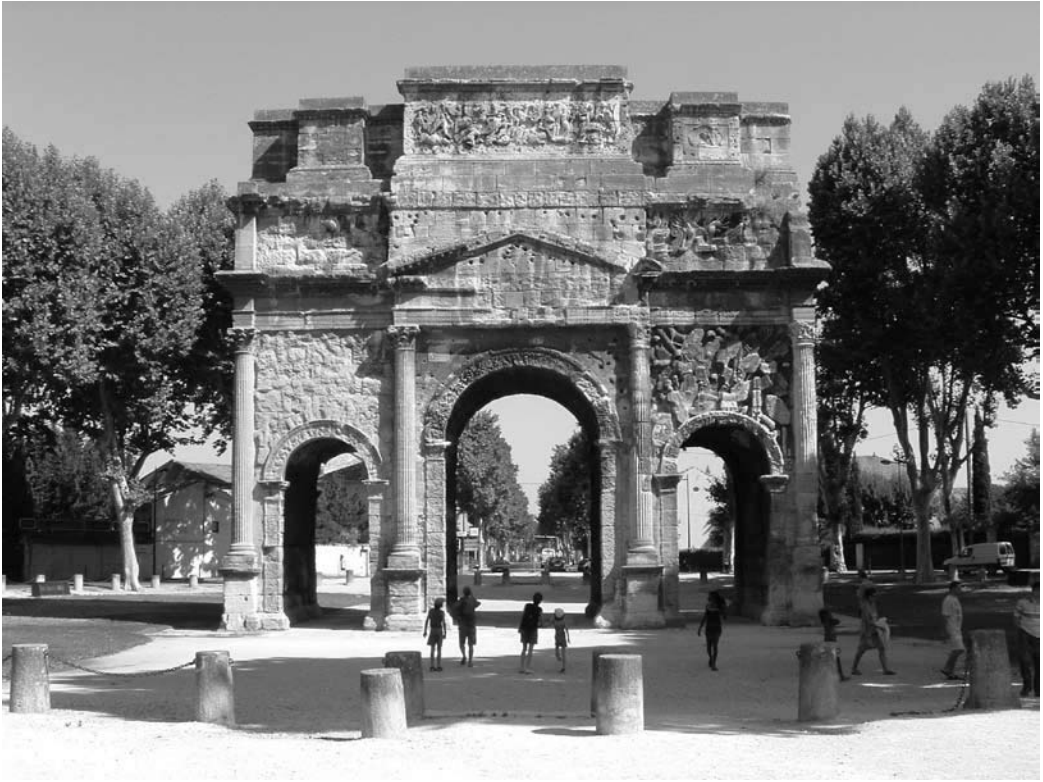
33 The Arch at Orange (Arausio), south face (photo by the author).
