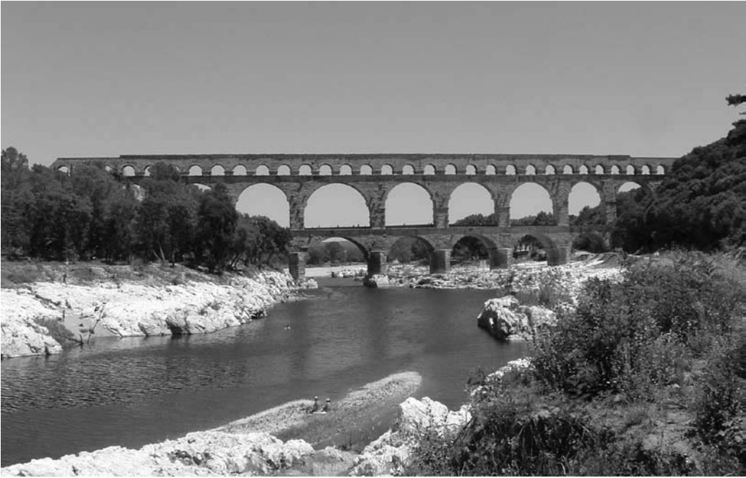
129 Central section of Pont du Gard, showing variant-sized vault spans (photo by the author).
