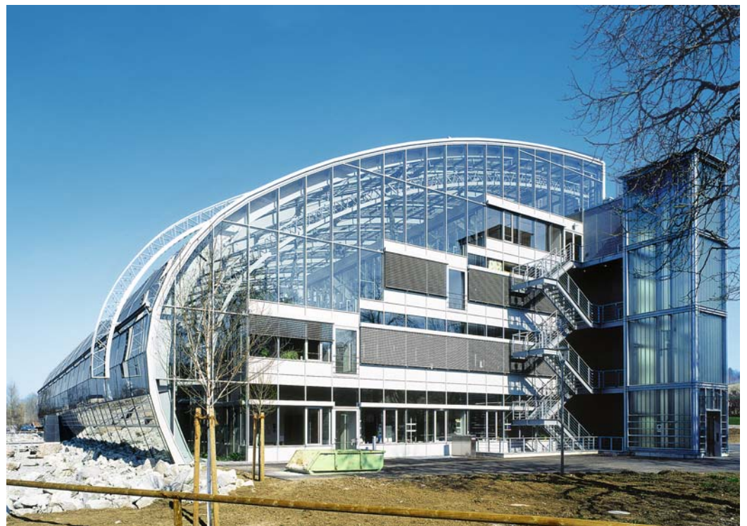
from left to right Stepped floors and transparency | Glazed west façade | Conventional offices are positioned behind the east façade
