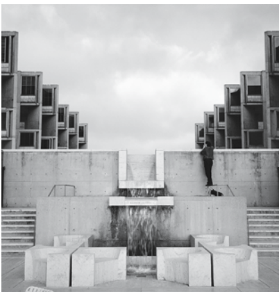
Salk Institute for Biological Studies, La Jolla/San Diego, California, USA; architect: Louis I. Kahn, 1959-1967 Fountain, closing off the central court space
