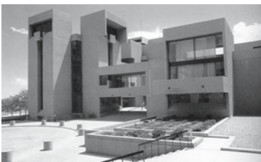
National Center for Atmospheric Research, Boulder, Colorado, USA; architect: I. M. Pei, 1961-67
