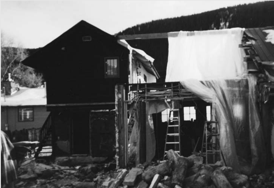
Figure 4.1 Taking the house down to the studs
