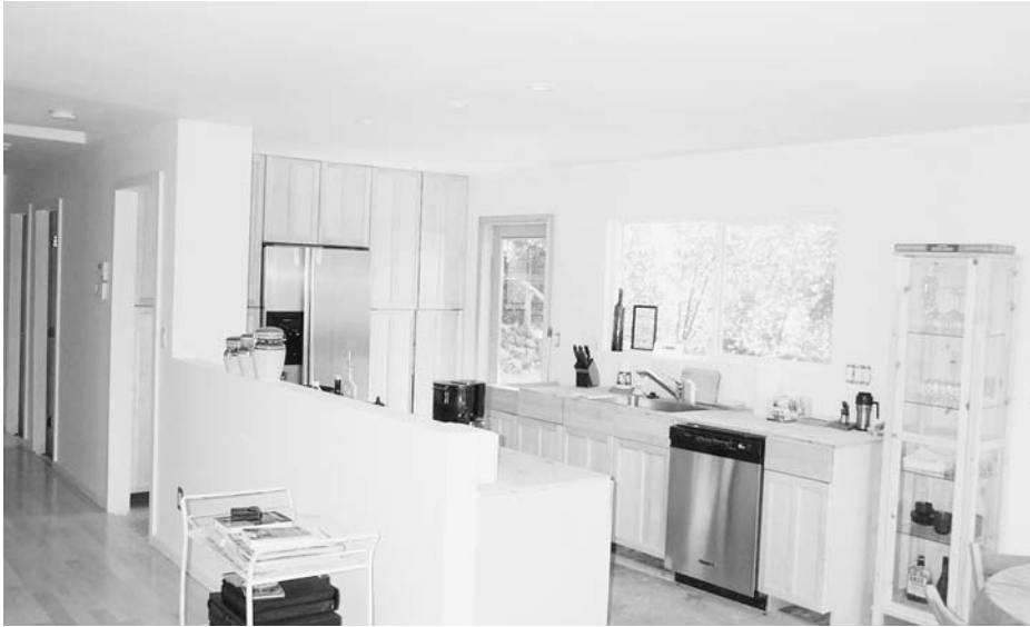
Figure 3.9 Sonoma kitchen renovation in progress
