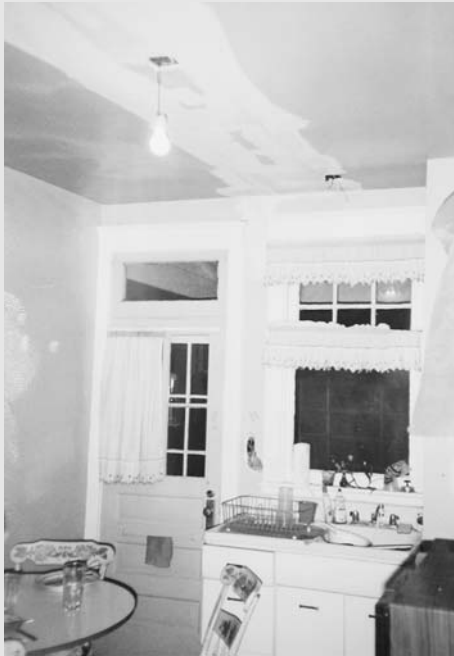
Figure 8.1 Kitchen under construction (but still in use!)
