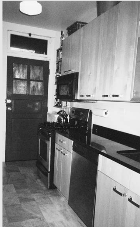
Figure 1.4 Kitchen after renovation
