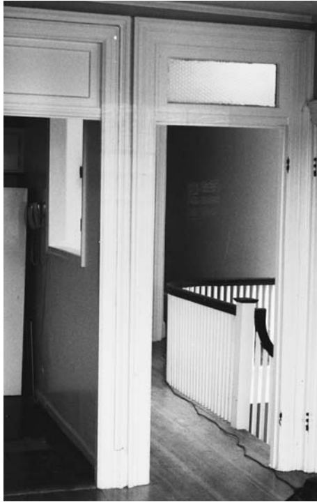
Figure 3.2 Interior entryway before renovation
