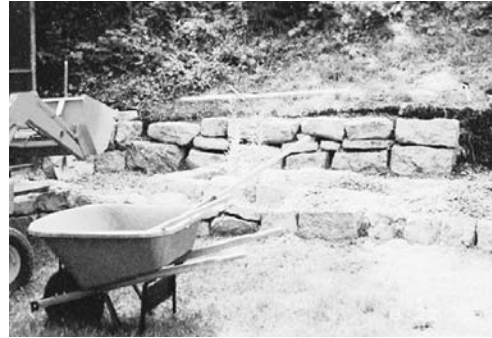
Figure 3.6 Patio area under construction
