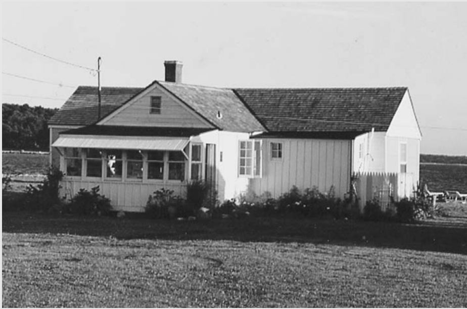
Figure 8.4 Cottage exterior after renovation
