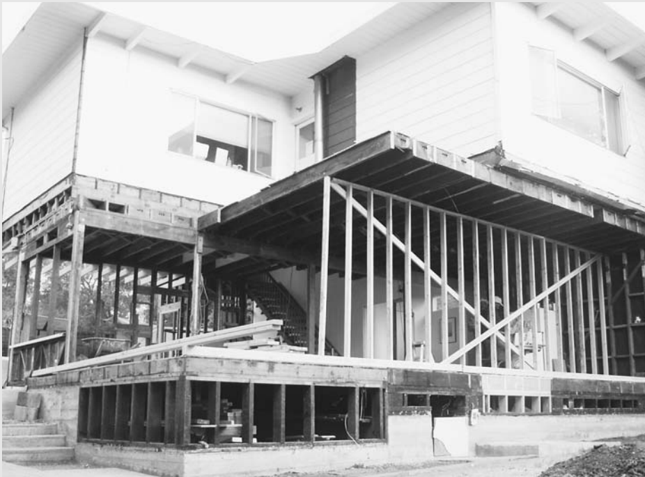
Figure 10.1 First floor totally gutted
