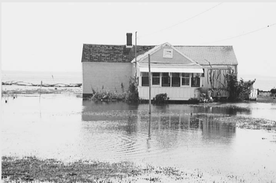
Figure 8.3 Exterior of cottage before renovation
