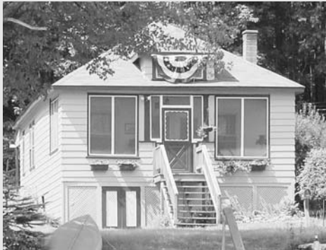
Figure 5.1 Our second cottage renovation
