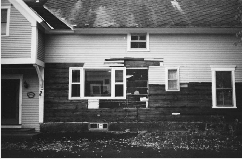
Figure 7.1 Back exterior during kitchen remodel
