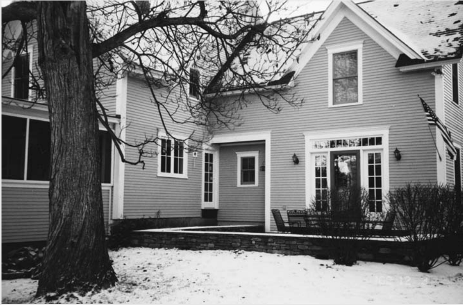
Figure 7.2 Side exterior after completed renovation
