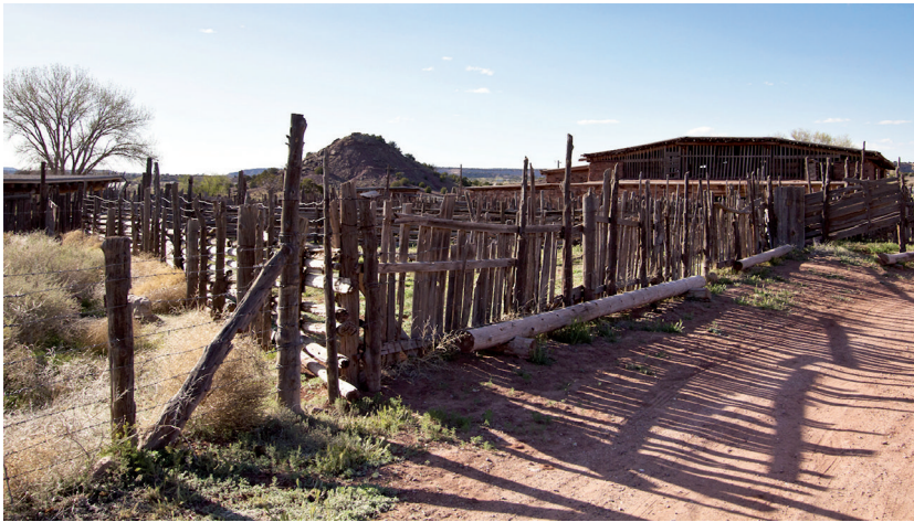
FIGURE 5.8 Outbuildings and fenced pasture at Hubbell Trading Post.
