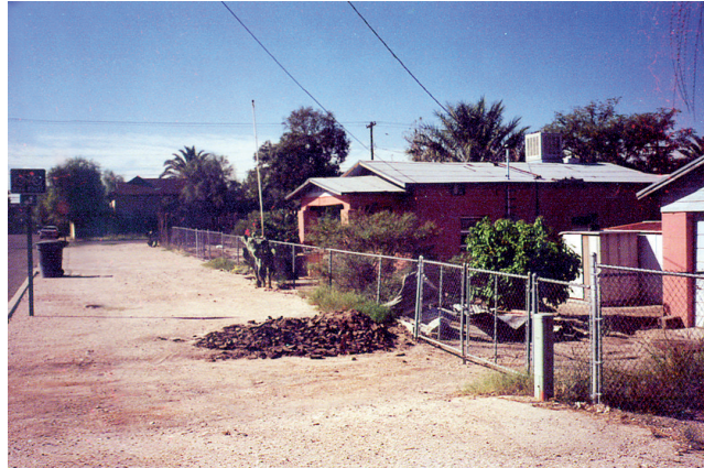
FIGURE 5.2A A street in the Dunbar/Spring neighborhood of Tucson, Arizona, in 1994, before swales were dug and food-bearing trees were planted.
