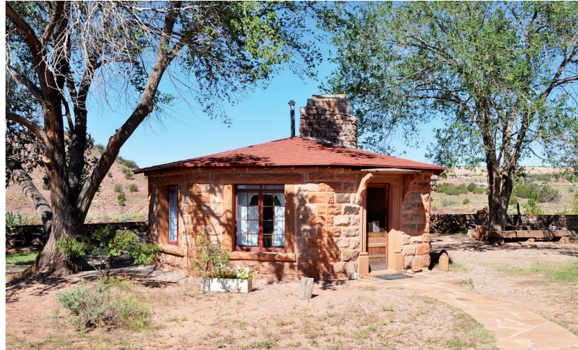
FIGURE 5.7 Stone hogans are traditional Navajo dwellings, often homes for extended families. This modified version (windows added) was originally used as a guest house.
