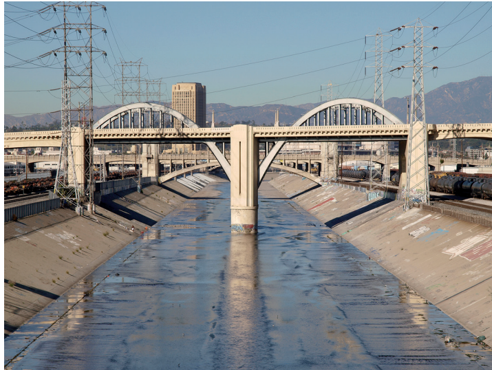
FIGURE 1.1 The highly engineered drainage system of the Los Angeles River exemplifies the almost total degradation of a natural riparian system.
