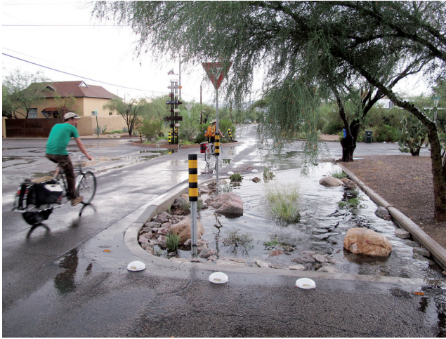
FIGURE 5.3 In the Dunbar/Spring neighborhood, a newly constructed water-harvesting chicane (basin) along a bicycle boulevard is filled with rainwater after a summer storm.
