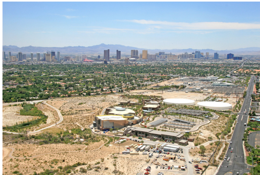
FIGURE 2.6 An aerial view of Springs Preserve in the construction phase, showing its location within the city in relation to the downtown strip.
