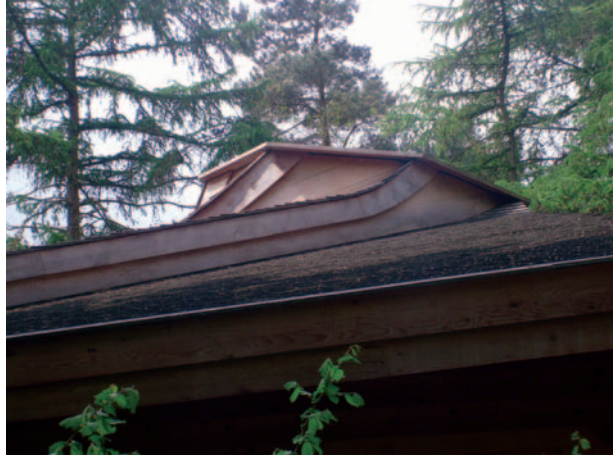
▲ 10.17 Chapel roof detail.
