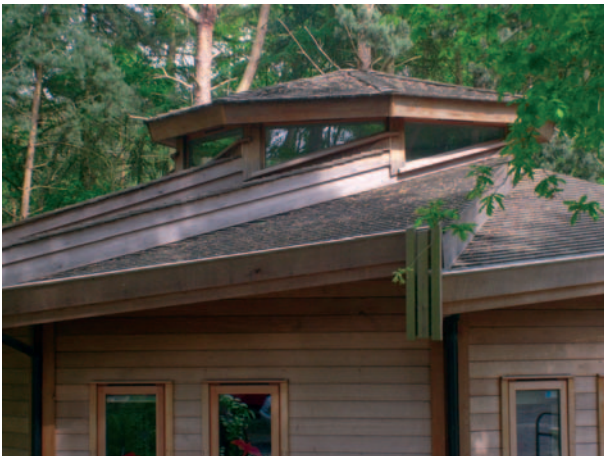
▲ 10.31 Office building – roof close-up.
