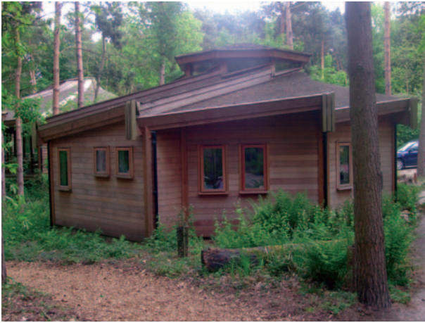
▲ 10.29 Office building – close-up.
