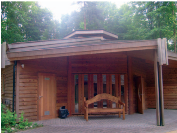
▲ 10.23 Gathering building – elevation facing the internal courtyard.
