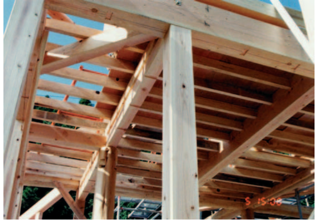
▲ 8.23 The New Farmhouse is a timber frame building. (Photo: Yoichi Kan.)
