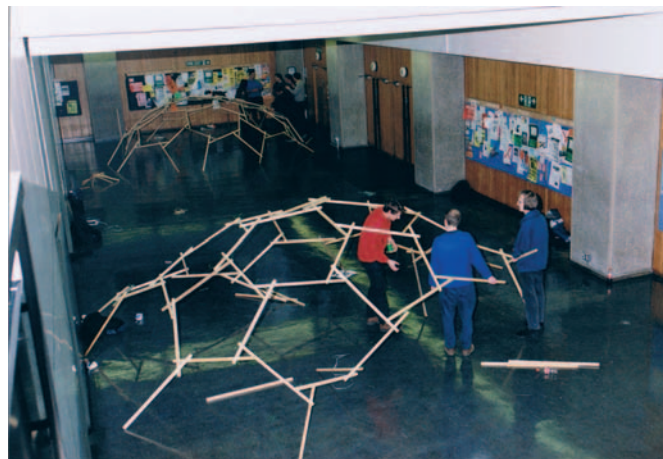
▲ 3.13 Constructing a multiple RF grid dome - 4.
