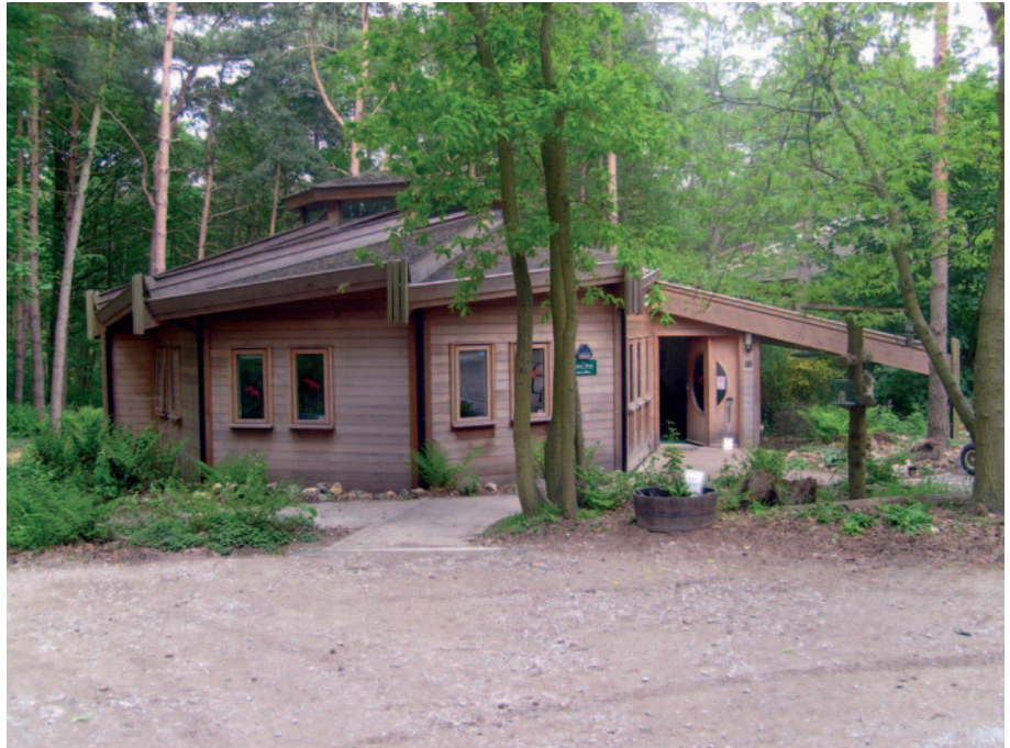
▲ 10.27 Office building – side elevation.
