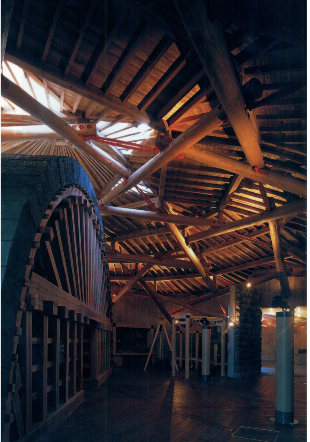
▲ 9.13 Interior view showing the permanent exhibit of a masonry bridge. (Photo: Keikaku-Inc.)
