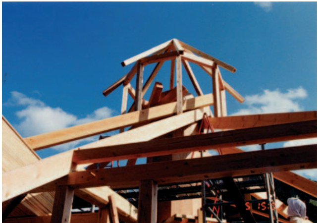
▲ 8.21 The RF beams form a full circle. (Photo: Yoichi Kan.)
