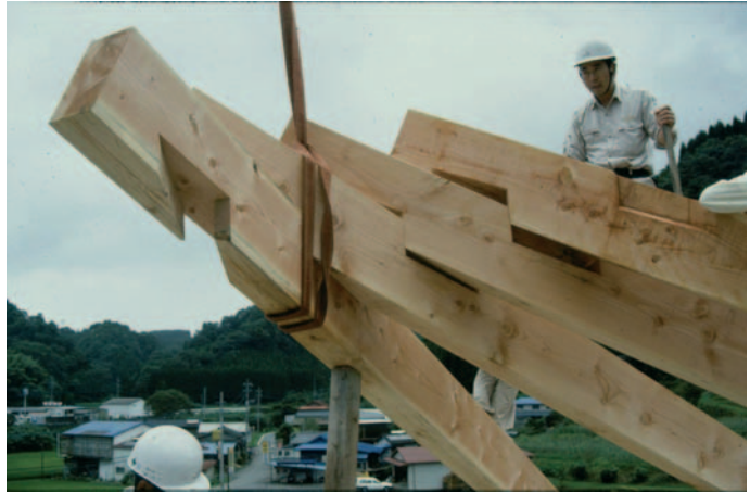
▲ 7.39 Assembling the pre-cut RF timber beams. (Photo: Kazuhiro Ishii.)
