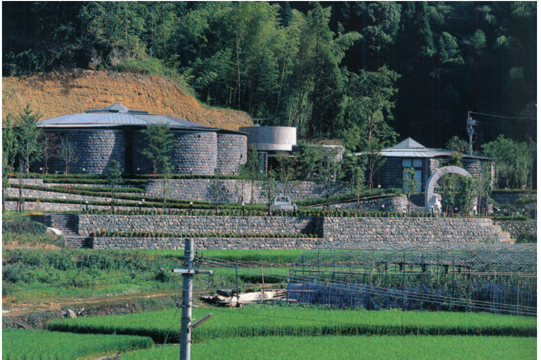
▲ 9.8 The Stonemason Museum in its surroundings. (Photo: Keikaku-Inc.)
