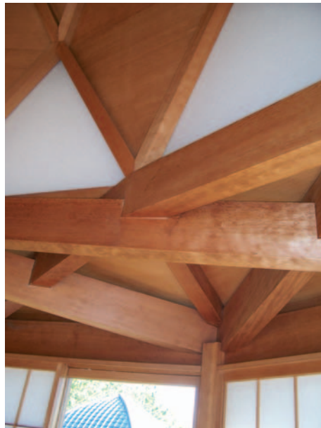
▲ 7.30 Complex notched timber connections.
