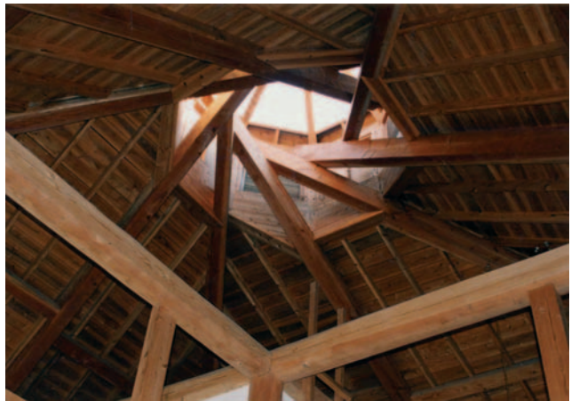
▲ 8.6 The RF roof structure is exposed internally. (Photo: Yoichi Kan.)
