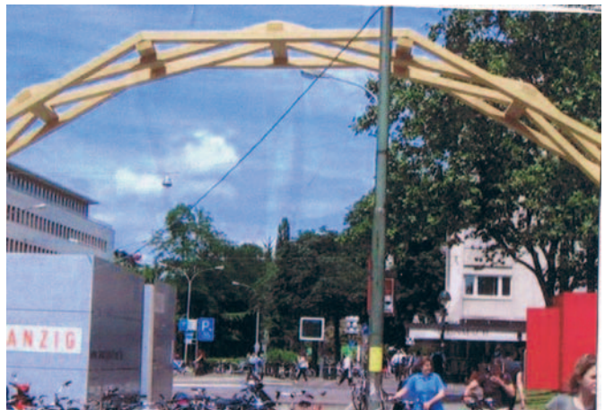
▲ 3.21 Student explorations – da Vinci-like bridge design.
