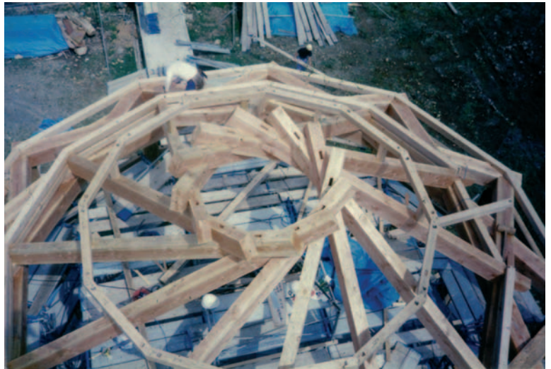
▲ 7.42 The structure of the RF roof is in place. (Photo: Kazuhiro Ishii.)
