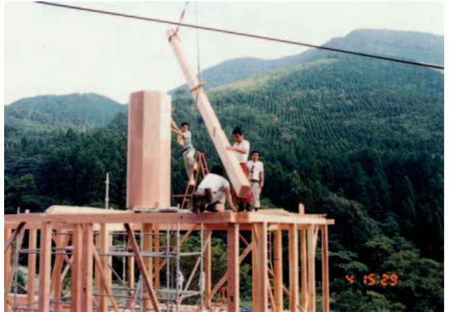
▲ 8.18 The RF beams are positioned on the temporary prop. (Photo: Yoichi Kan.)
