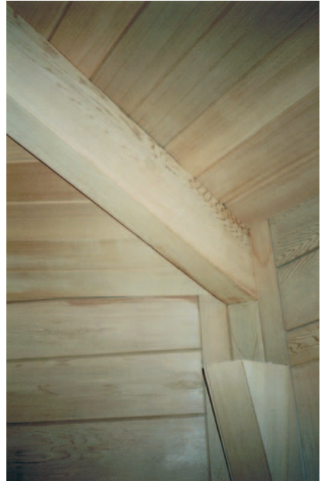
▲ 10.4 Gazebo – internal finishes.
