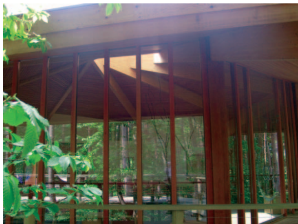
▲ 10.15 Chapel – the building blends into the woodlands.
