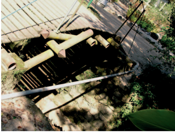
▲ 2.12 Pedestrian RF bridge. (Photo: Andy Tyas.)
