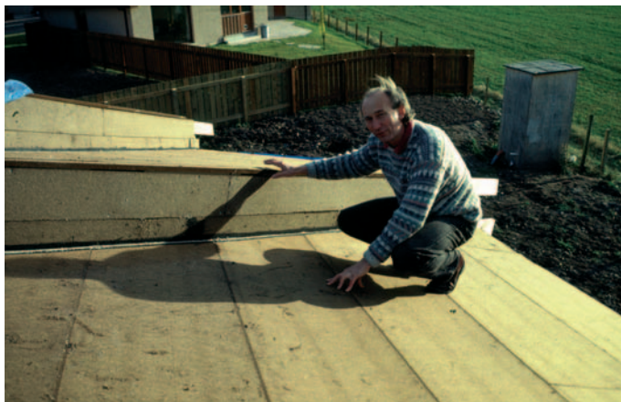
▲ 10.1 Graham Brown constructing one of his RF buildings.
