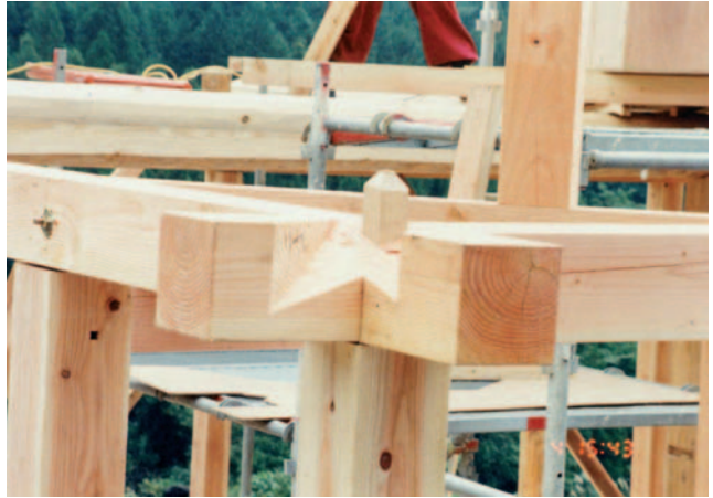
▲ 8.16 Traditional Japanese timber joints are used throughout the building. (Photo: Yoichi Kan.)
