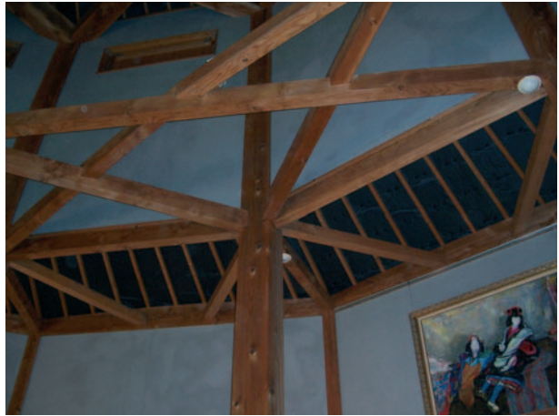
▲ 7.37 The RF-like ring beam reduces buckling.
