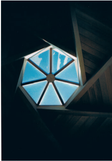
▲ 10.3 Gazebo – internal view.
