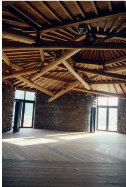
▲ 9.16 The intricate timber roof structure forms the space. (Photo: Keikaku-Inc.)
