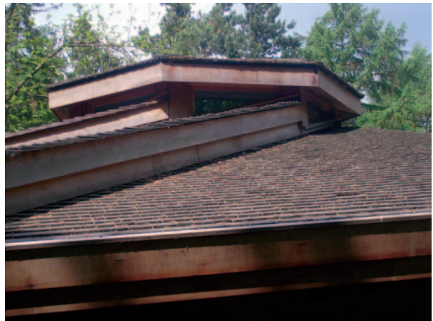
▲ 10.26 RF roof – close-up.
