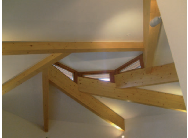
▲ 10.25 Internal view towards the roof light.
