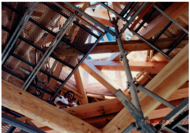
▲ 8.22 View through the roof light. (Photo: Yoichi Kan.)
