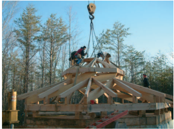
▲ 11.8 Fitting the roof light. (Photo: Fred Oesch.)
