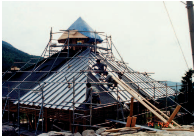
▲ 8.24 The roof is enclosed with metal sheet cladding. (Photo: Yoichi Kan.)
