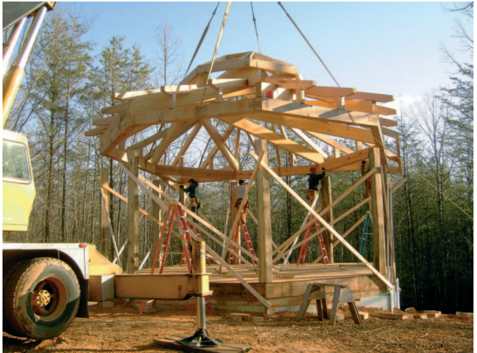
▲ 11.9 The finished skeleton. (Photo: Fred Oesch.)
