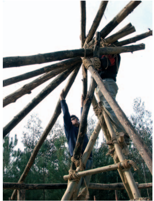
▲ 11.4 Constructing the roof. (Photo: Tony Wrench.)
