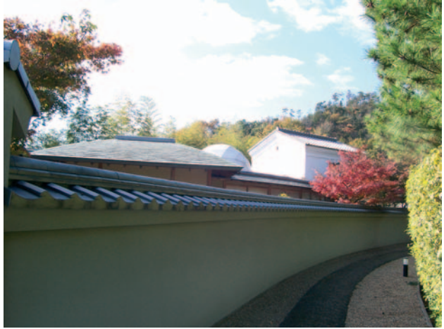
▲ 7.22 The sweeping wall marking the grounds of Sukiya Yu.
