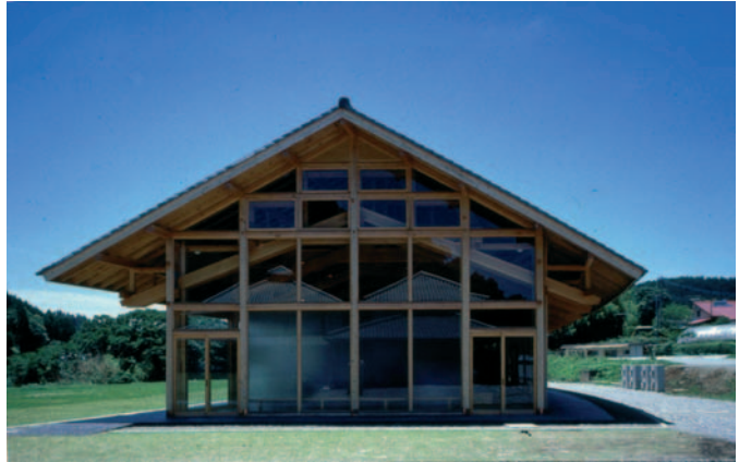
▲ 7.53 The shop and café building – elevation. (Photo: Kazuhiro Ishii.)
