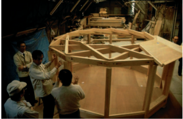
▲ 7.31 Constructing the physical model of the RF roof in 1:5 scale. (Photo: Kazuhiro Ishii.)
