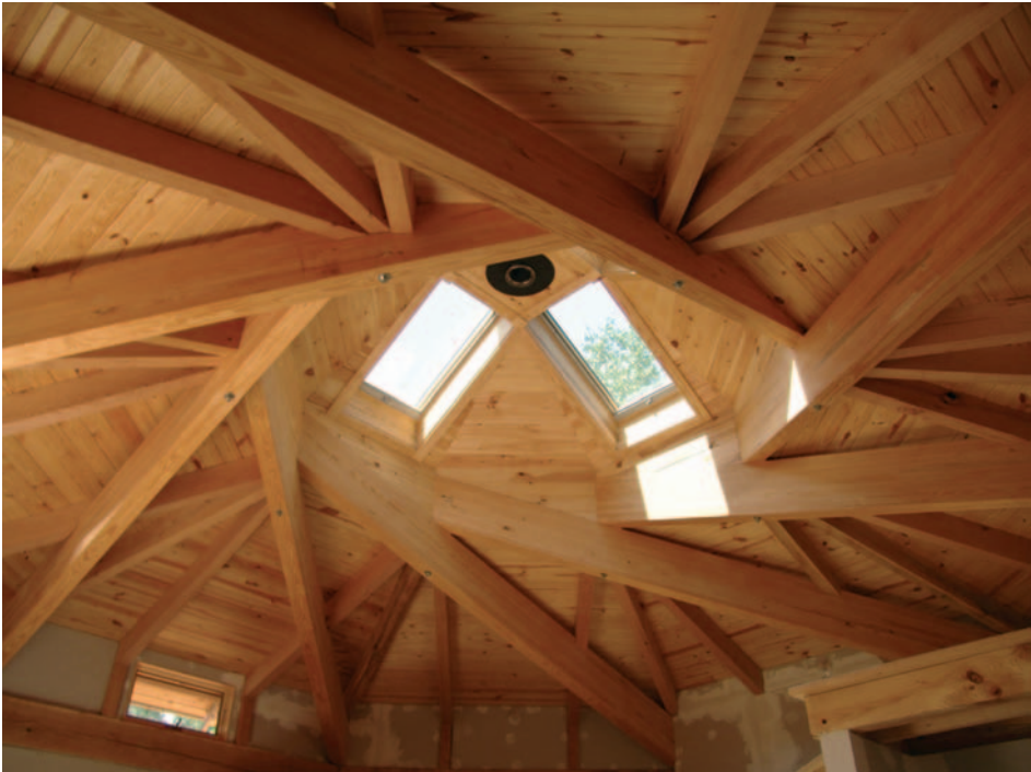
▲ 11.10 The RF roof – internal view. (Photo: Fred Oesch.)
