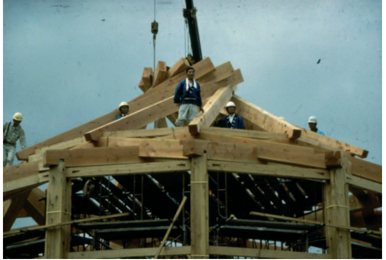
▲ 7.41 All RF timber beams are in place – elevation. (Photo: Kazuhiro Ishii.)
