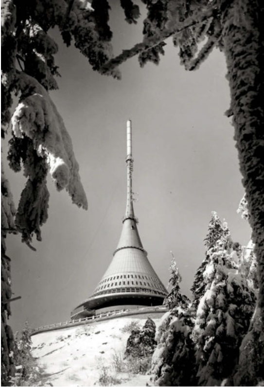
fig. 2 Karel Hubáček (Architect) and Zdeněk Patrman (Engineer): Antenna tower with hotel and cable car on Ještěd Mountain near Liberec.
