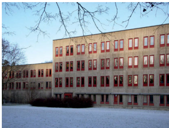
fig. 1 KBS's buildings for the National Telecommunication Board in Farsta outside of Stockholm, completed in 1969 and designed by Bengt Hidemark and Gösta Danilesson. Photo Holger Ellgaard, CC, 2012.
