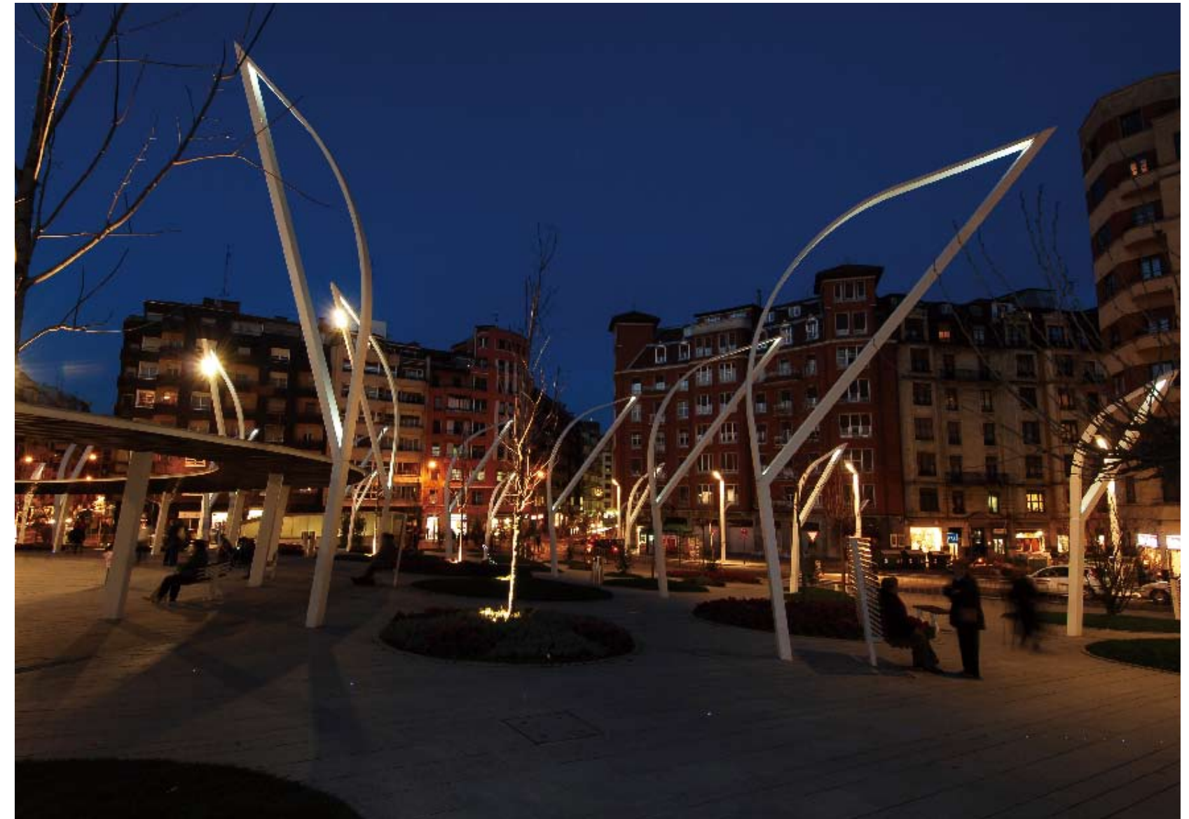
Upper left: Night view of the plaza Lower right: Sculptural light pole as a decorative streetscape
