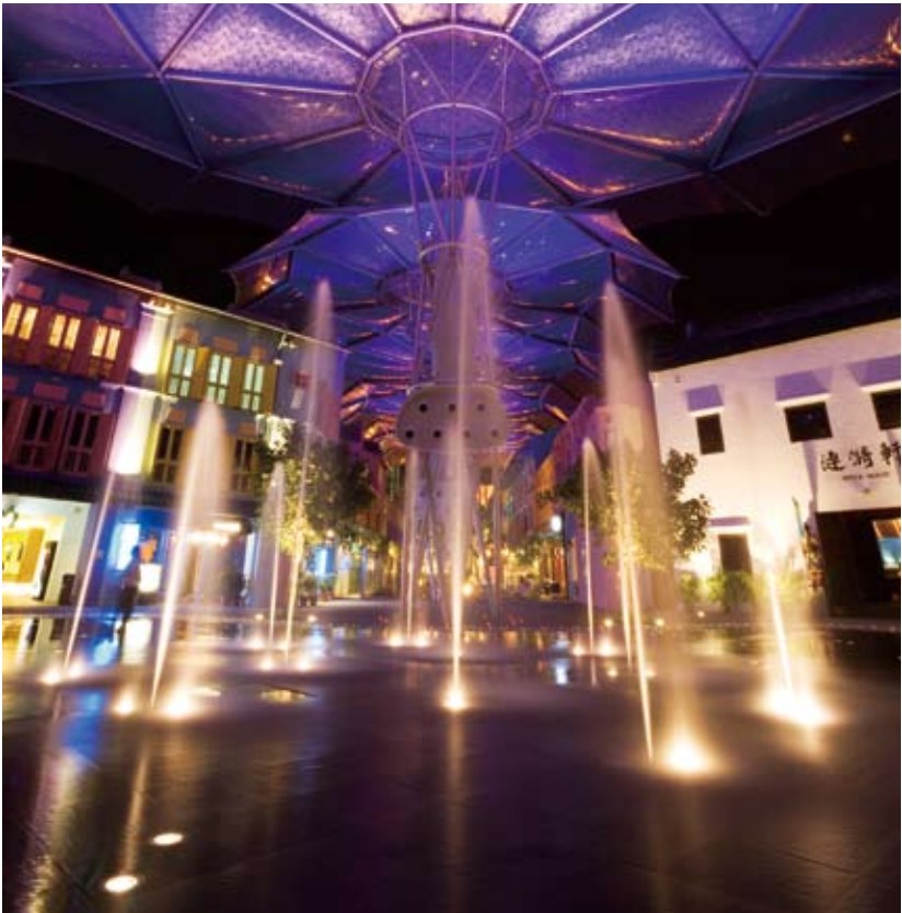
Left: Elegant canopies provide environmentally friendly shading and cooling, which protect visitors against the extremes of the Singaporean climate and maintain the temperature at 28 centigrade
