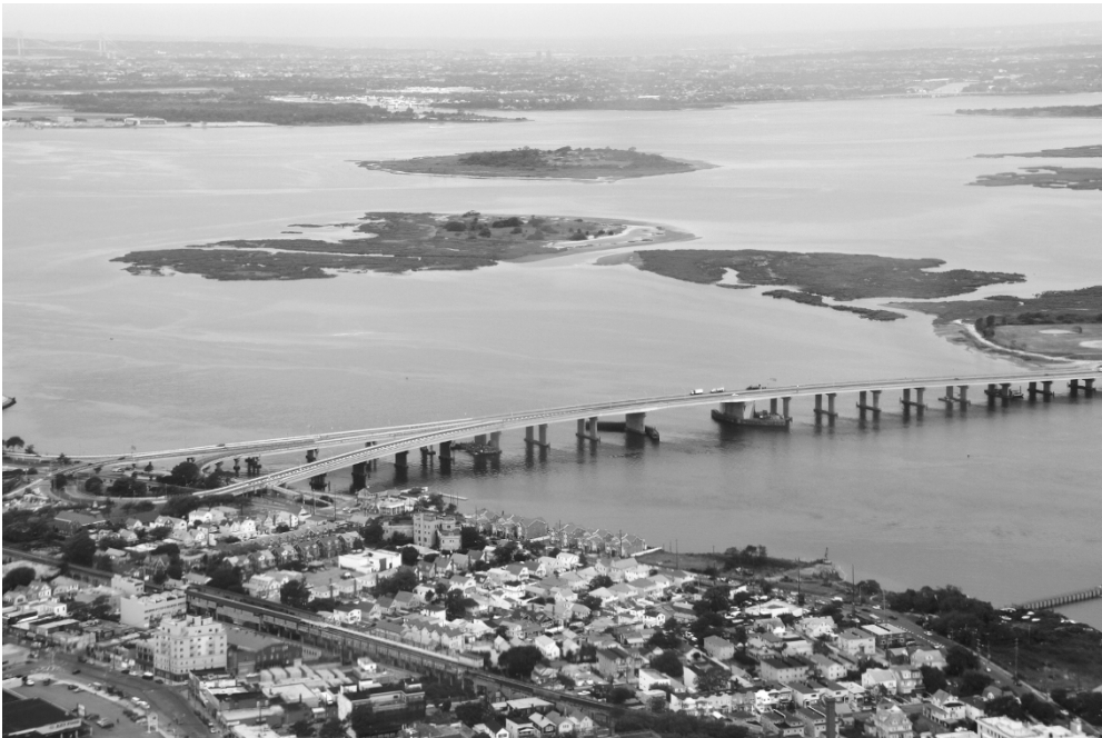
Figure 1-3. A view of Jamaica Bay. Jamaica Bay and its watershed form a coupled SES where there are strong interactions between land and water, as shown in this aerial photograph of the Cross-Bay Veterans Memorial Bridge, which connects Broad Channel with the Rockaway Peninsula, shown in the foreground. The photograph was taken by Erlend Bjørtvedt in July 2012, courtesy of Wikimedia Commons.
