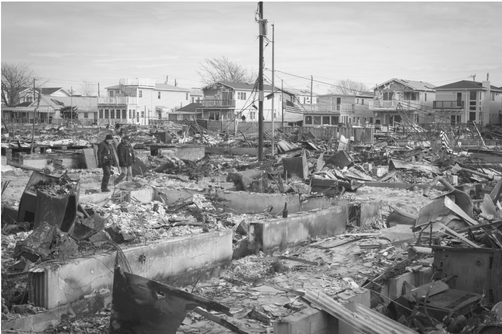
Figure 1-2. Fire and storm damage at Breezy Point, New York. The Breezy Point fire, ignited as a result of damage from Hurricane Sandy, destroyed 130 homes and damaged many more. Breezy Point is the westernmost community on the Rockaway Peninsula, a barrier island that separates Jamaica Bay from the Atlantic Ocean (see color plate VII). The photograph was taken by Chief Mass Communication Specialist Ryan J. Courtade of the U.S. Navy, and is courtesy of the U.S. Department of Homeland Security, Federal Emergency Management Agency.
