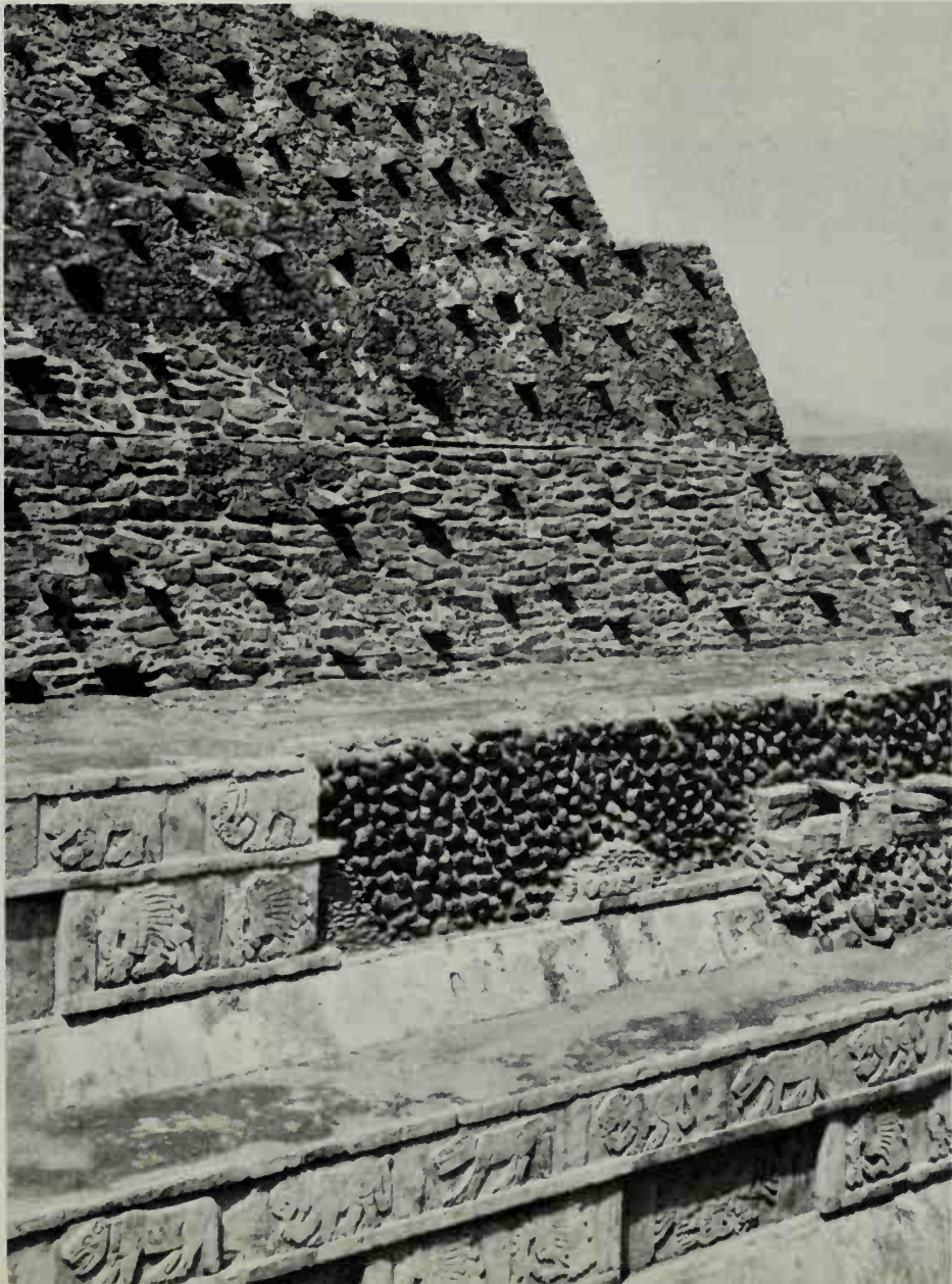
46. Pyramid of Tlahuizcalpantecuhtli, Tula. Detail of taluds and tableros.
