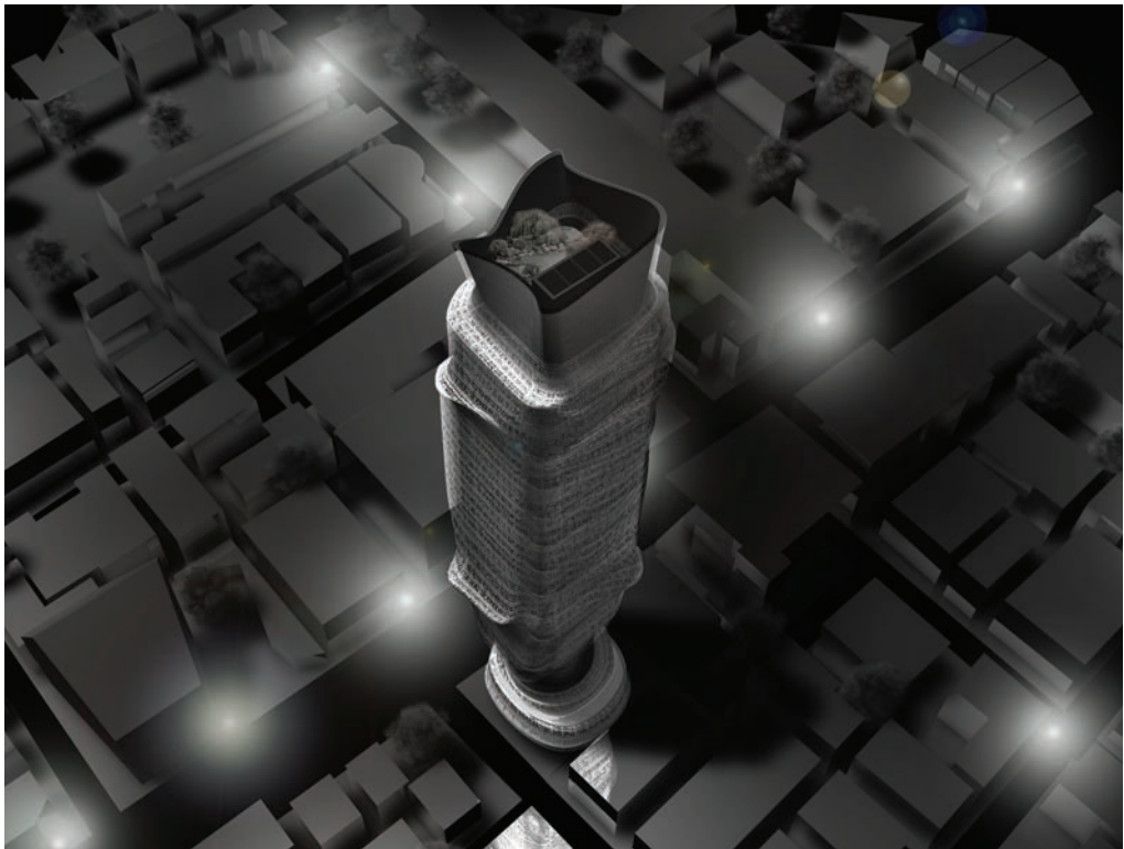
The outer skin of the double-wall façade structure would consist of carbon fiber sheets that are impregnated with carbon nanotube (CNT) prepreg. The CNT-resin mix would give these panels an extraordinary strength-to-weight ratio when compared to metals or other composites. (Courtesy Decker Yeadon LLC)
