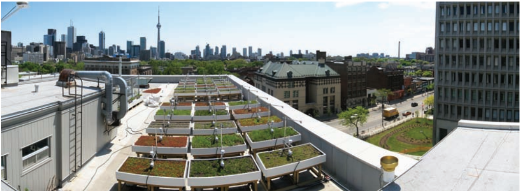
Green Roof Innovation Testing Laboratory (GRITLab) Panoramic view of green roof instrumentation at the John H. Daniels Faculty of Architecture, Landscape and Design—University of Toronto. (Courtesy Liat Margolis)
