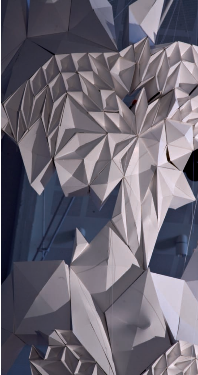
Porous Ascend utilizes a spatial structure based on geometry derived from patterns of aperiodic tiling and recursion. (Courtesy Jacob Rüber)
