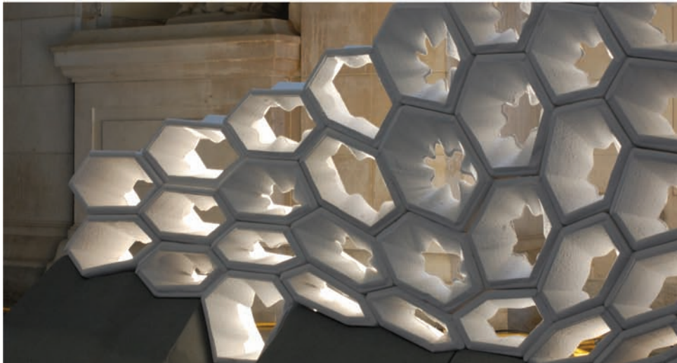
Pinch Wall is comprised of 145 plaster components, each unique and variable in size, in response to degree and angle of porosity. The components are organized as strata and rest upon a buttressing base; they utilize a “valley” method of stacking in which adjacent casts lock into position. (Courtesy Jeremy Ficca)
