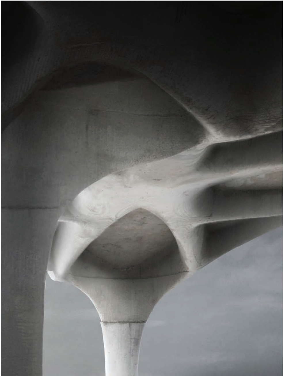
Optimized rib system, disclosing the trajectories of the forces to the observer. (Courtesy Per Dombernowsky & Asbjørn Søndergaard)
