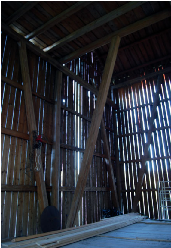
Typical Norwegian barn, 1950s The interior view of the barn shows the gaps between the planks, as well as the slenderness of the barn's structure.
