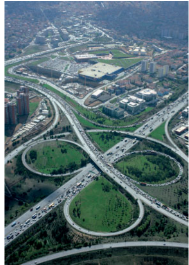
Above: Foreign Office Architects, Meydan Retail Complex and Multiplex, Istanbul, Turkey, 2007. The aerial photograph shows the Meydan complex as a continuation of the landscaped surface of the wider area.
