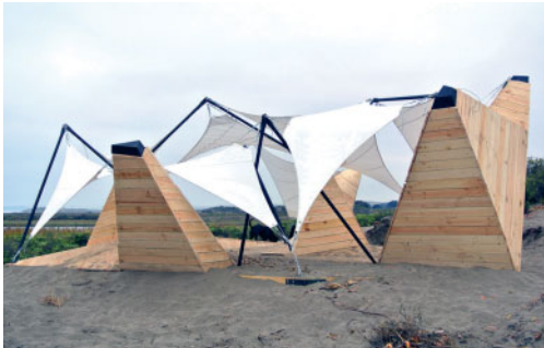
Las Piedras del Cielo – Membrane Shelter – Open City Ritoque, Scarcity and Creativity in Latitude 33 Master-Studio, Oslo School of Architecture and Design, Norway, 2012 The membrane shelter designed by masters students at the Oslo School of Architecture and Design for the Open City in Ritoque in Chile consists of a landform podium with embedded spaces and a roof of nine membranes. The structure will serve as a sheltered meeting, cooking and eating area for the Open City.
