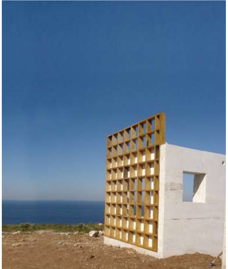
2008 mockup—with local, craftsman-built wood fenestration—in Akbuk, Turkey
