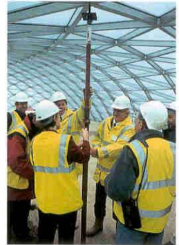
Above: With most of the glazing in place, Spencer de Grey, Suzanna Taverne and representatives from Buro Happold and MACE remove the last of 593 temporary roof supports, 13 April 2000.
