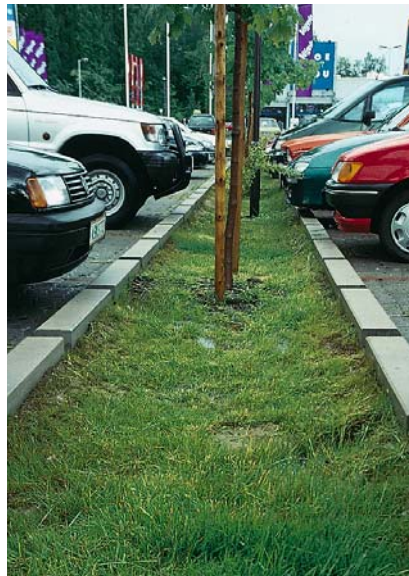
Grassed swales are placed next to the parking spaces, the trees planted there flourish even in the conditions prevailing in locations of this kind.
