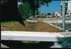
A footpath crossing a drainage ditch, here still under construction
