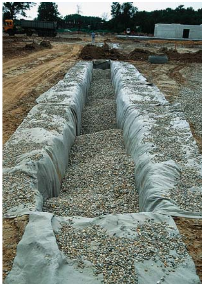
Constructing a swale system between parking spaces
