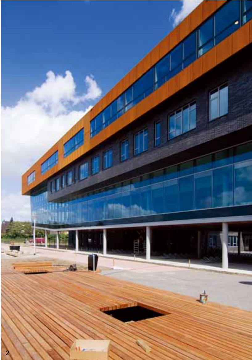
1. Overall view of water bank building 2, 3, 4. Contrasting colours and materials are also used on the exterior; dark brick façades are clad with corten steel
