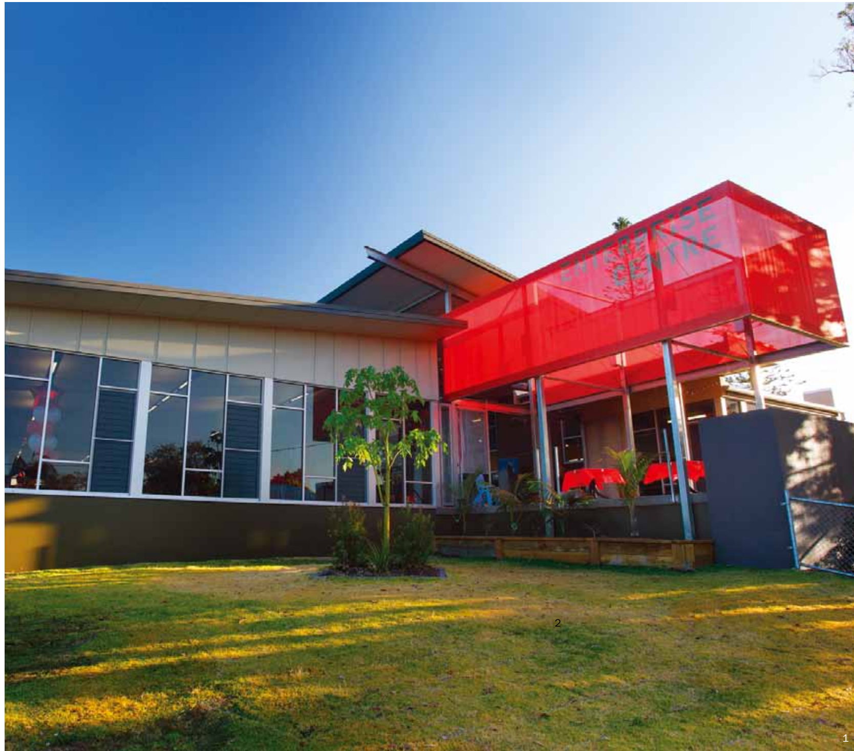
1. Side view of façade 2. Access to the entrance 3. Airconditioning services
