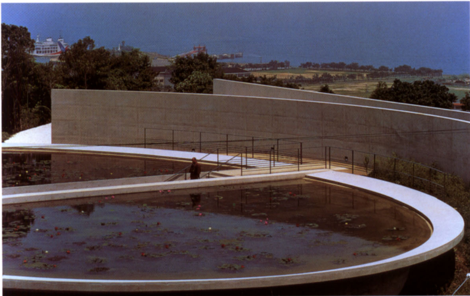
Tadao Ando Hompuku-ji Temple Awajishima, Japan, 1989–90 The entrance to this temple leads the visitor to the curving concrete wall seen to the left, before he discovers the artificial pond and the stairs, which lead down into the temple itself. There, a representation of Buddha sits, with its back to the setting sun.
