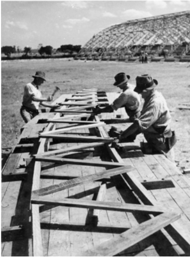
Figure 7. View of walls, abutment pads and arches. 2nd store in similar stage of construction. Rydalmere. Construction US Stores. February 1943. (Item 53.1/2.7, box 17, series B5281, National Archives of Australia.)
