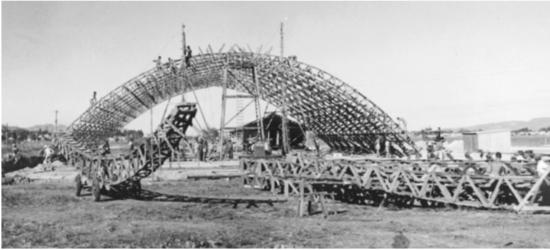
Figure 10. Showing igloo framework under construction. Townsville – Garbutt – RAAF Store. July 1943.
