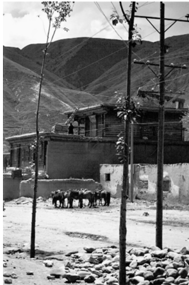
Figure 2. Tibetan street, Dengke, in north-west Sichuan, July 1999. Traditional 2–3 storey dwelling house with timber clad living areas within rammed earth walled enclosure. (Photograph by author.)
