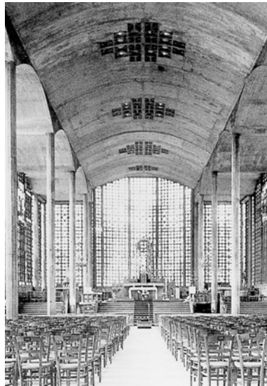
Figure 20. Nave, Notre Dame de Raincy, Auguste Perret, 1924–25
