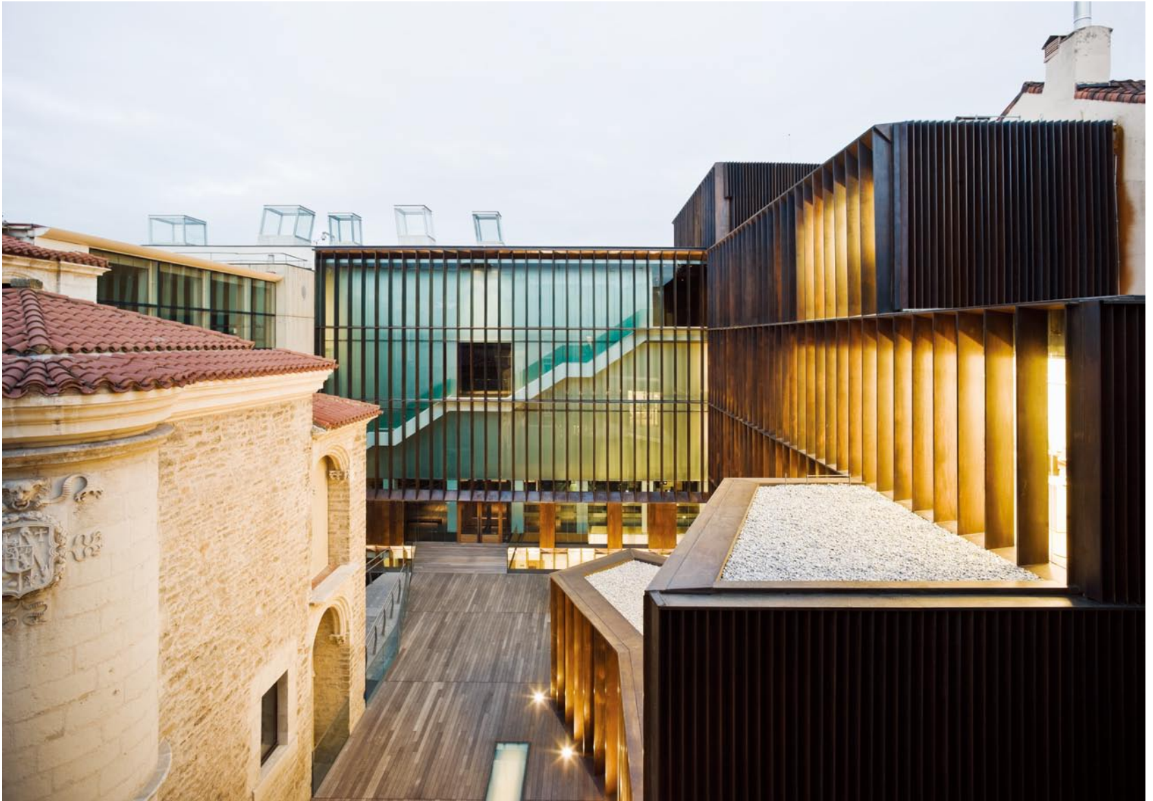
Left The museum seems like a compact jewel box concealing treasures. Upper right Cast bronze pieces configure the outer façades that define the access court. Lower right Courtyard view.
