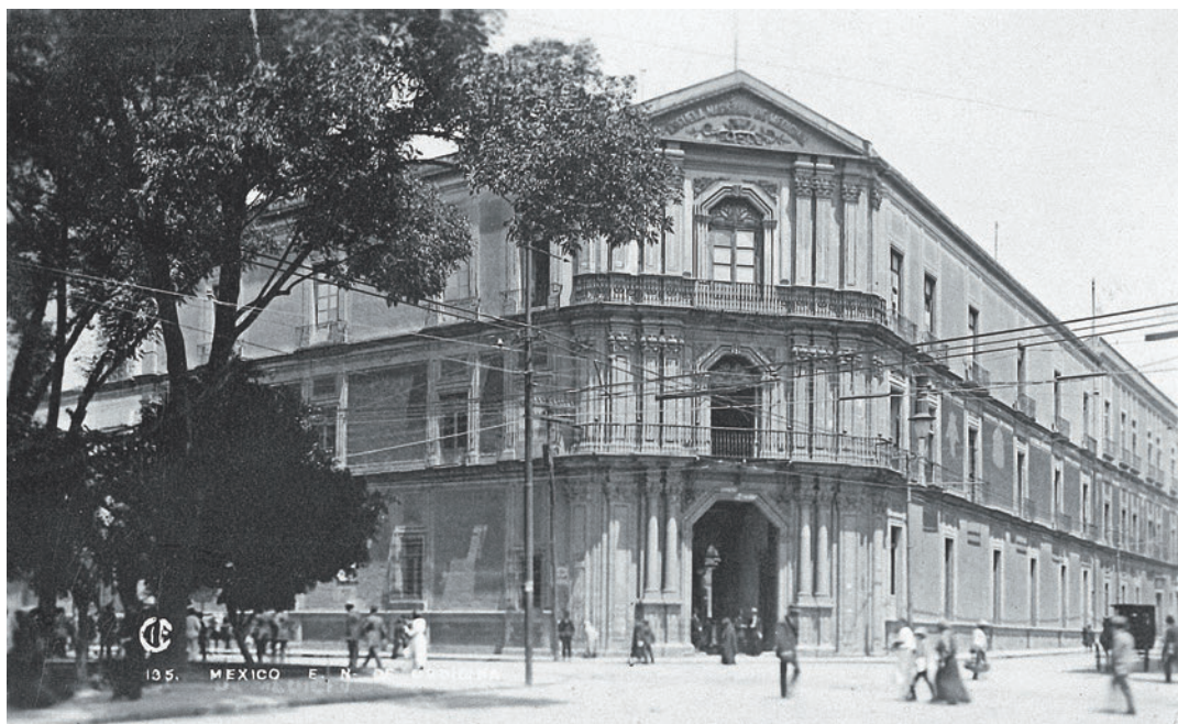
FIGURE 2.11. Pedro de Arrieta, Palace of the Inquisition (later, National School of Medicine), Mexico City, 1695.
