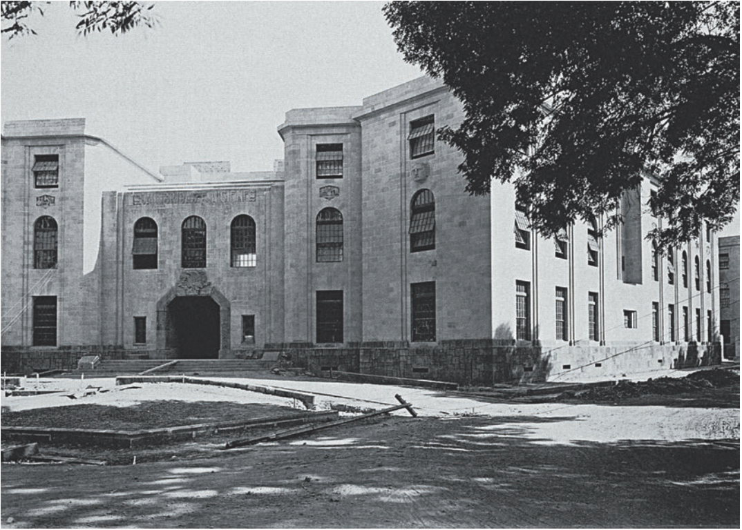
FIGURE 2.1. Carlos Obregón Santacilia, Ministry of Health, 1925–29. Photograph by Guillermo Kahlo.
