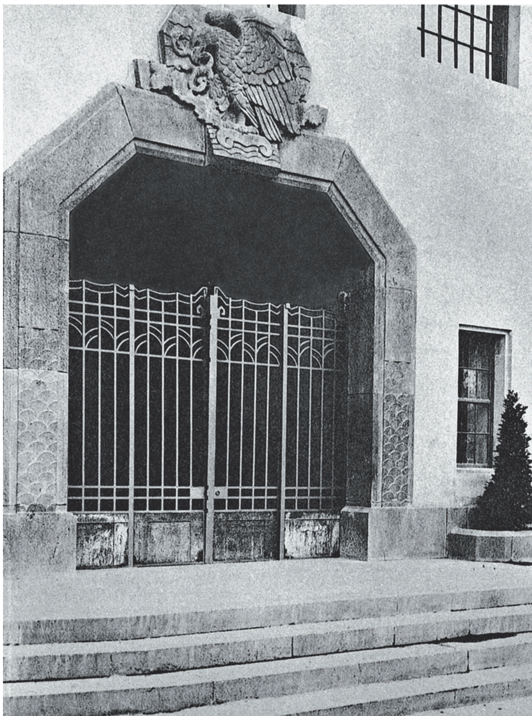
FIGURE 2.10. Obregón Santacilia, Ministry of Health, door. Photograph by Guillermo Kahlo.
