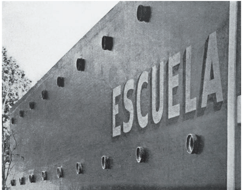
FIGURE 4.26. Melchor Ocampo School, in Escuelas primarias .
