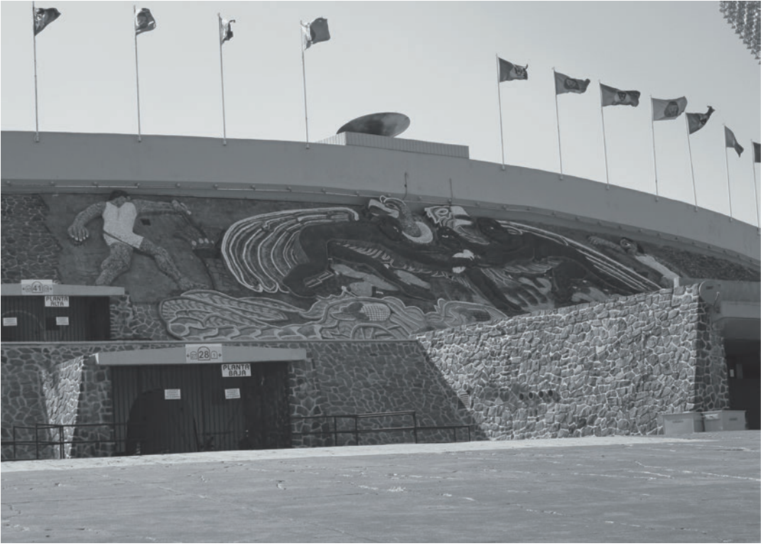
FIGURE 5.5. Augusto Pérez Palacios, Jorge Bravo, and Raúl Salinas, Olympic Stadium, with Diego Rivera's partially completed mosaic on the east facade.
