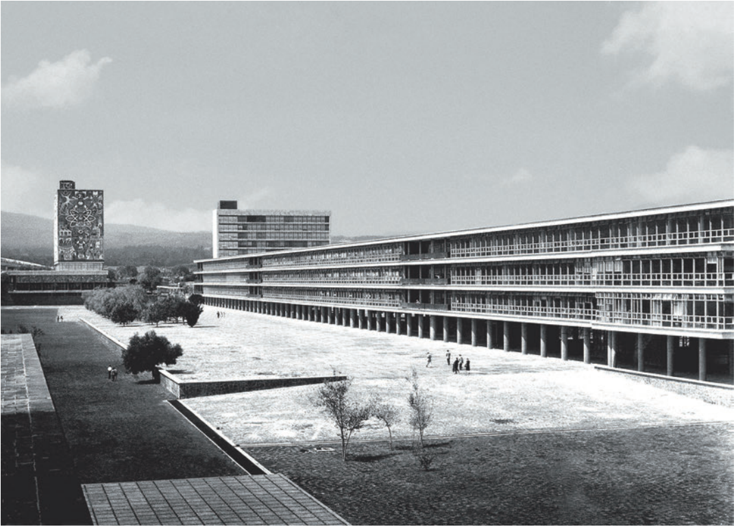
FIGURE 5.9. Faculty of Philosophy and Letters (Enrique de la Mora, Enrique Landa, and Manuel de la Colina) and Law buildings (Alonso Mariscal and Ernesto G. Gallardo) on the right. The Central Library can be seen in the distance.
