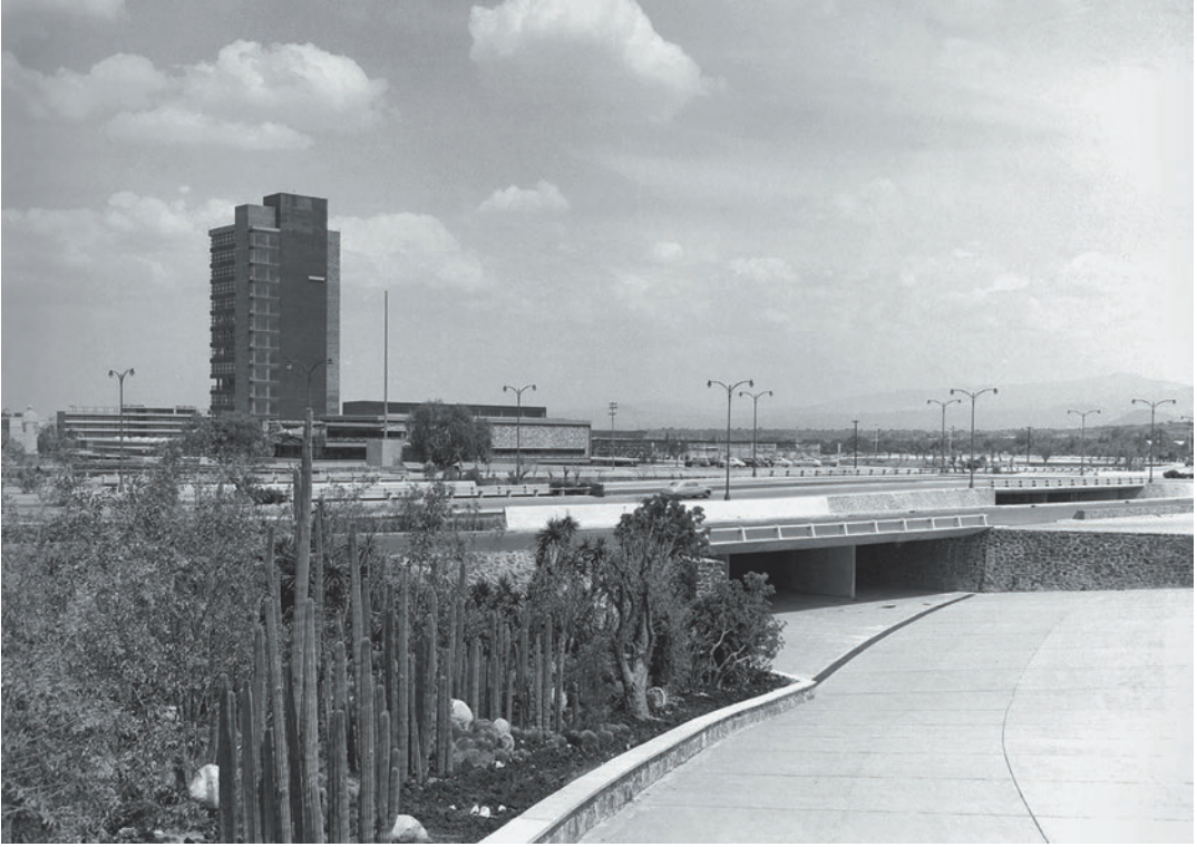
FIGURE 5.2. View of University City looking southeast from the Olympic Stadium, ca. 1952. Bridge and road design by Santiago Greenham and Samuel Ruiz García.
