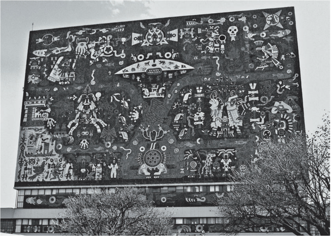
FIGURE 5.10. Central Library, north facade.
