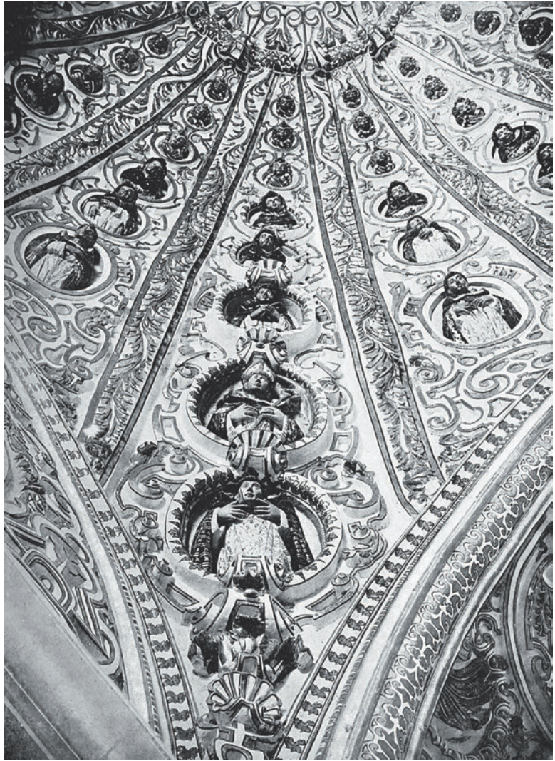
FIGURE 1.9. Cortés, Church of Santo Domingo, Oaxaca, vault above the choir, eighteenth century, from García, La arquitectura en Mexico: Iglesias .
