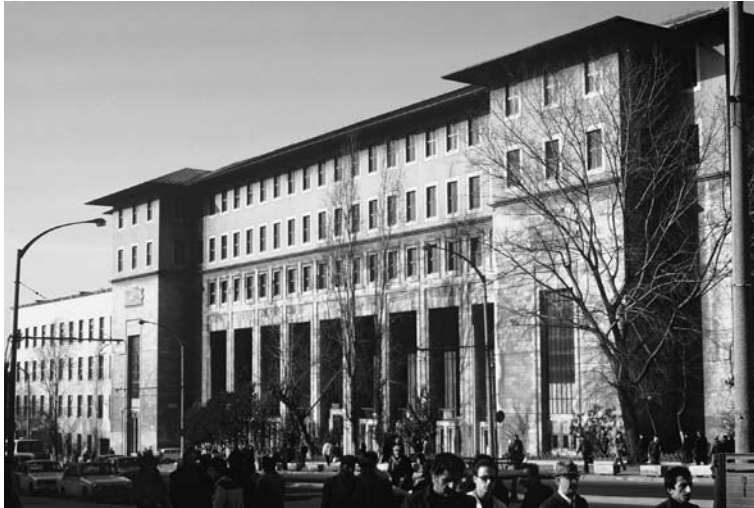
6.5 Sedad Eldem. Main façade of the Faculty of Sciences and Literature, Istanbul University, 1942.
