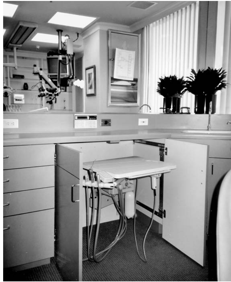
Figure 10-34. Custom casework in treatment room features retractable doors to conceal assistant's mobile cart. (Photo courtesy: Cheryl Sheets, D.D.S.; Photographer: Jain Malkin.)
