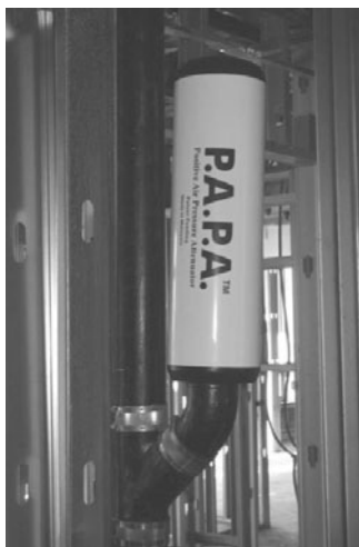
PHOTO 14.15 A positive air pressure attenuator (PAPA) is a product developed to protect buildings of 10 or more stories against the unwanted positive pressures (i.e., back pressure/positive transients) generated in the DWV system. PAPAs are installed at the base of the soil and waste stack and at various floor intervals, depending on the height of the building. (Used with permission of ABC)
