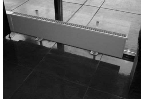
PHOTO 7.33 A close-up view of the front of a convective radiator. (Used with permission of ABC)
