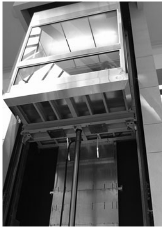
PHOTO 24.2 Hydraulic elevators use a fluid-driven hydraulic jack to lift the elevator car. Shown is the bottom side of a conventional (holed) hydraulic elevator. The elevator car is made of the cab, which carries the passengers and the platform, which consists of structural framework. The hydraulic plunger connects to the center beam of the car platform. Behind and alongside the cylinder (to left) is the traveling cable. Guide rails are evident on the left and right side of the hoistway walls. (Used with permission of ABC)
