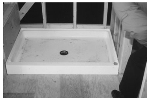
PHOTO 12.20 A roughed-in plastic shower pan. (Used with permission of ABC)
