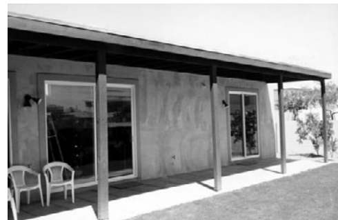
PHOTO 11.36 An overhang providing summer shade. (Courtesy of DOE/NREL)
