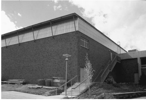
PHOTO 20.35 Exterior windows designed to introduce daylight in a gymnasium. (Used with permission of ABC)
