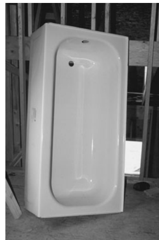
PHOTO 12.17 An enameled iron bathtub stored before installation. (Used with permission of ABC)
