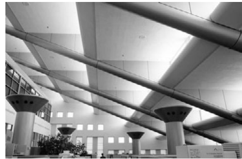
PHOTO 20.39 Stepped windows and light shelves throw natural light deep into the building. (Courtesy of NREL/DOE)
