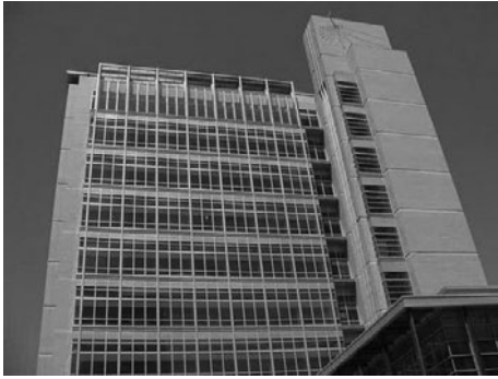
PHOTO 25.20 Building-integrated PV (BIPV) at the Alfred A. Arraj U.S. Federal Courthouse, Denver, Colorado. (Courtesy of DOE/NREL)
