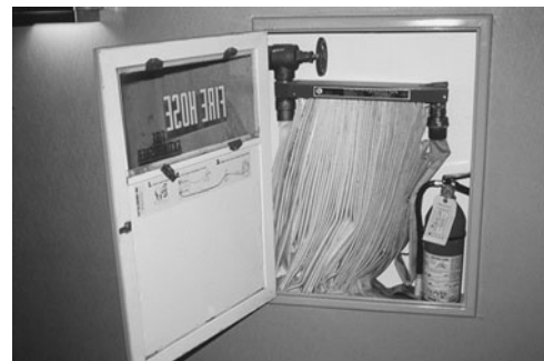
PHOTO 21.4 A typical fire hose outlet and release rack connected to a standpipe. (Used with permission of ABC)
