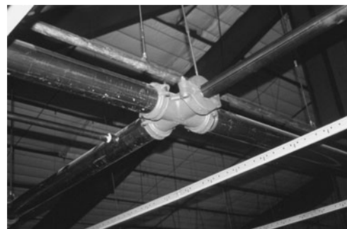
PHOTO 21.10 A Victaulic tee coupling. (Used with permission of ABC)
