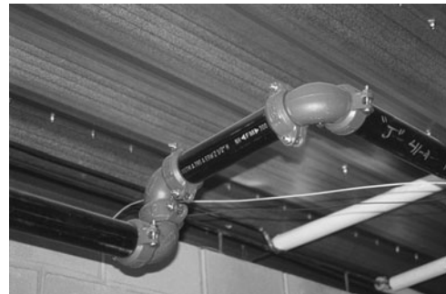
PHOTO 21.8 Victaulic elbows used to connect a cross main. (Used with permission of ABC)
