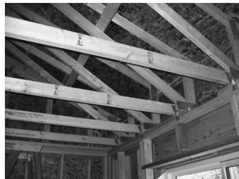
PHOTO 3.2 Lightweight construction typically consists of light timber frame. (Courtesy of DOE/NREL)
