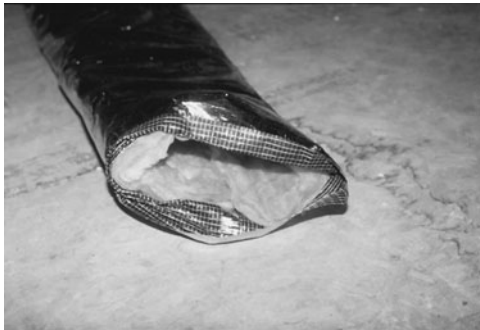
PHOTO 7.5 Lined flexible duct. (Used with permission of ABC)
