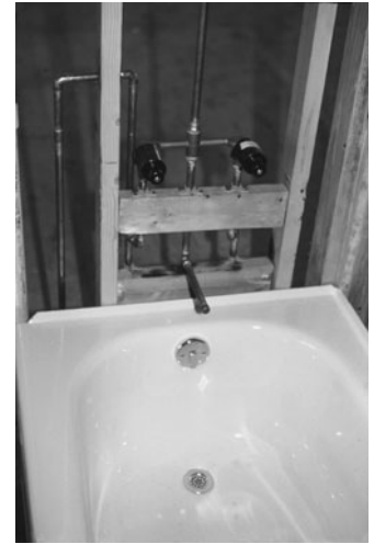
PHOTO 13.8 A front side view of branches connecting to a bathtub and showerhead. (Used with permission of ABC)
