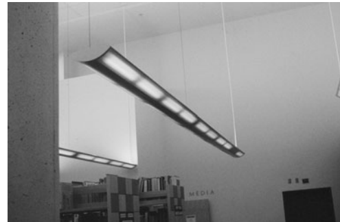
PHOTO 20.9 A linear fluorescent uplight used to provide ambient lighting in a library. (Used with permission of ABC)
