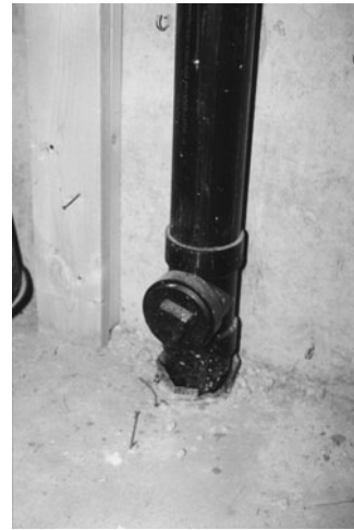
PHOTO 14.11 A close-up of a wall cleanout. (Used with permission of ABC)
