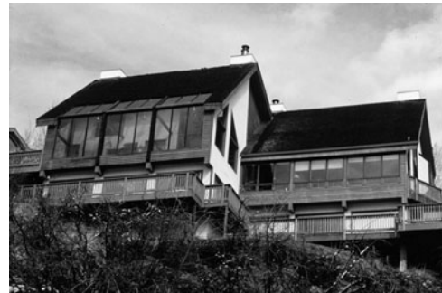
PHOTO 11.18 A passive solar residence with direct gain (right) and sunspace systems (left). Note that shades are used for control to prevent overheating and eliminate glare. (Used with permission from ABC)
