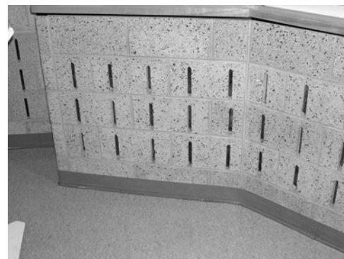
PHOTO 23.2 Slotted acoustical concrete masonry units dampen sound, thus improving the noise reduction attributes of an interior space. Acoustical units are often used in schools, industrial plants, churches, and other facilities to improve internal acoustics. (Used with permission of ABC)
