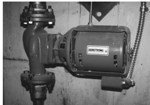
PHOTO 9.3 Pressure and temperature gauges on a hot water boiler. A small circulating pump used to circulate hot water.
