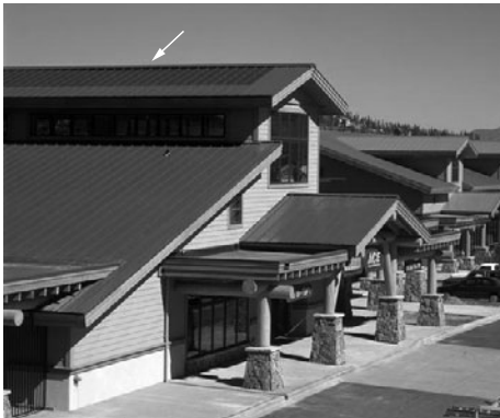
PHOTO 25.21 BIPV shingles serve to substitute for composition shingles. (Courtesy of DOE/NREL)
