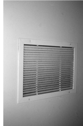
PHOTO 7.17 A wall register. (Used with permission of ABC)
