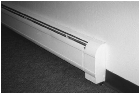
PHOTO 7.30 A finned tube, baseboard convector used for residential installations. (Used with permission of ABC)
