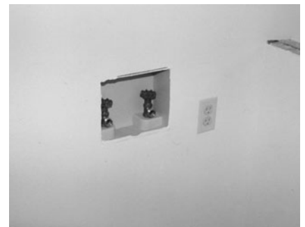
PHOTO 13.14 A finished laundry connection. (Used with permission of ABC)
