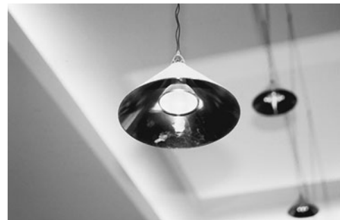
PHOTO 20.29 Halogen accent lighting used as task lighting over a conference table. (Used with permission of ABC)
