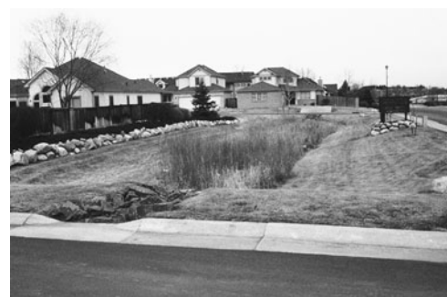
PHOTO 16.9 A detention pond designed to temporarily hold overflow storm water. (Used with permission of ABC)
