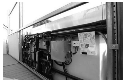
PHOTO 6.36 A small-scale ice storage system uses off-peak energy at night to chill ice used for cooling the house on hot days. (Courtesy of NREL/DOE)
