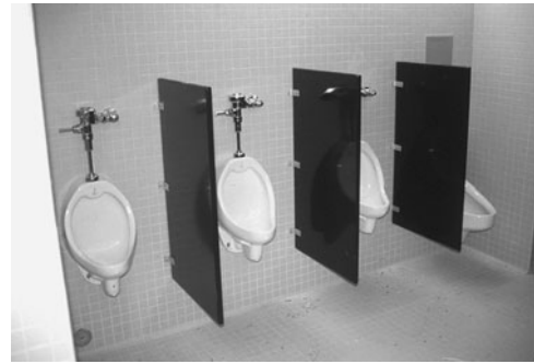
PHOTO 12.13 A group of urinals separated by partitions. (Used with permission of ABC)
