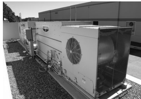
PHOTO 6.35 A commercial-scale indirect evaporative cooler. (Used with permission of ABC)
