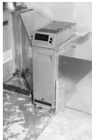
PHOTO 7.23 An in-duct electrostatic air cleaner. (Used with permission of ABC)
