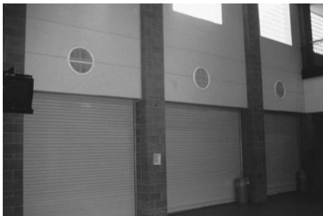
PHOTO 7.16 Round, high sidewall diffusers. (Used with permission of ABC)
