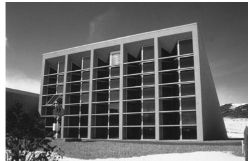
PHOTO 11.26 A direct gain and unvented thermal storage wall system at the National Renewable Energy Laboratory (NREL) Visitor Center, Golden, Colorado. (Used with permission from ABC)
