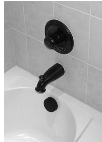
PHOTO 12.18 A tub faucet with tub/shower control. (Used with permission of ABC)
