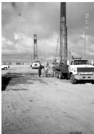
PHOTO 25.9 Drilling boreholes for a vertical ground closed-loop system. (Courtesy of DOE/NREL)
