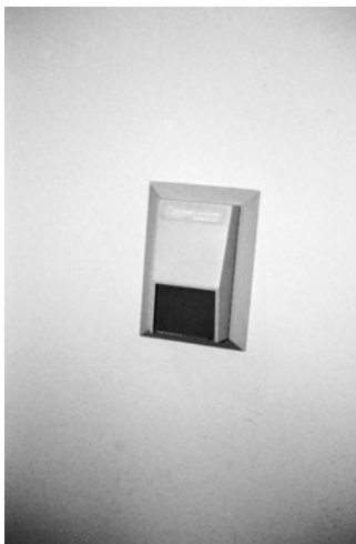
PHOTO 7.43 A nonprogrammable, thermostatic sensor. The unit is controlled by a remote energy management system. (Used with permission of ABC)
