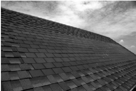
PHOTO 25.21 BIPV shingles serve to substitute for composition shingles. (Courtesy of DOE/NREL)
