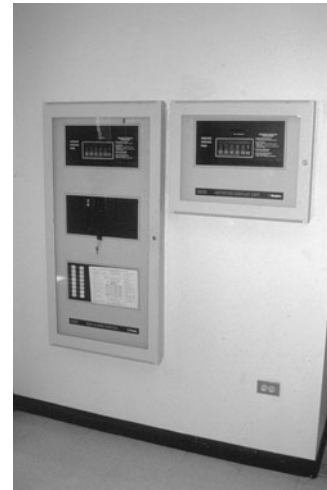
PHOTO 21.26 A fire command center. (Used with permission of ABC)
