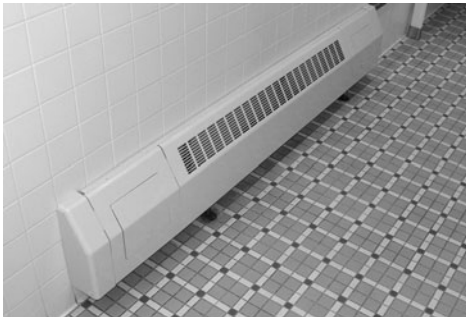
PHOTO 7.31 A finned tube, baseboard convector, typically used in commercial installations. (Used with permission of ABC)
