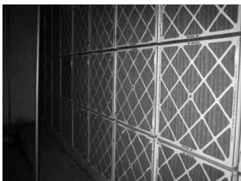
PHOTO 7.22 A set of flat-panel, mechanical air filters in an air-handling unit (AHU). (Courtesy of NREL/DOE)
