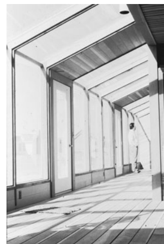
PHOTO 11.35 The interior of a sunspace integrated in a new home. Insufficient thermal mass and the upper glass will create overheating and drastic temperature swings (fluctuations). Shading of upper glass and venting will be necessary. (Used with permission from ABC)
