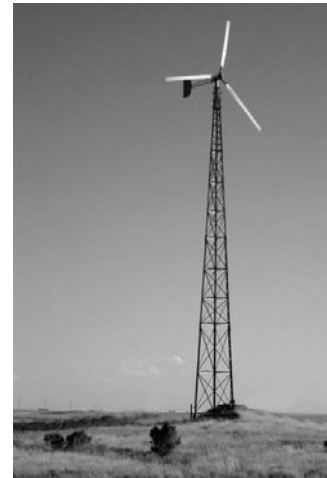
PHOTO 25.32 A 20-kW Jacobs wind turbine on a freestanding tower. (Courtesy of DOE/NREL)
