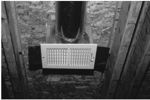
PHOTO 8.8 A ceiling register. (Used with permission of ABC)
