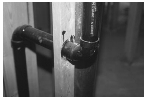
PHOTO 12.6 ABS pipe connected with a solvent welded connection. (Used with permission of ABC)
