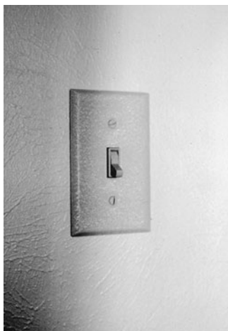
PHOTO 18.11 General duty wall-mounted switch. (Used with permission of ABC)
