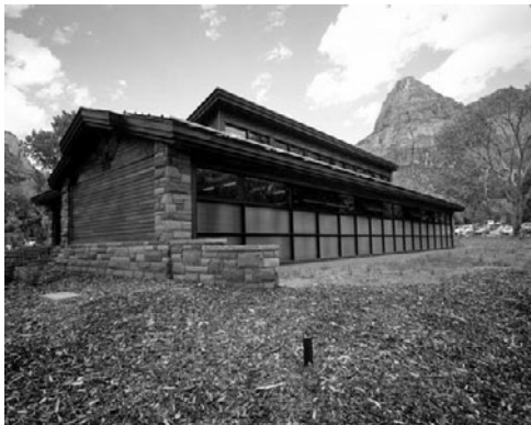
PHOTO 11.41 The trombe wall and clerestory windows of the Zion Visitor Center. (Courtesy of DOE/NREL)
