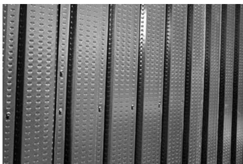
PHOTO 11.11 A close-up of the perforated transpired collector material. Outside air is drawn through the perforations and moves behind the metal material, which heats the air before it is drawn into an air-handling unit where it is further heated, if necessary. Lack of a need for glass on this system reduces collector costs. (Courtesy of DOE/NREL)
