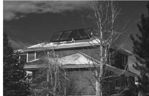
PHOTO 11.5 A liquid flat-plate collector system on a residence as part of an active solar heating and domestic water heating system. (Used with permission from ABC)
