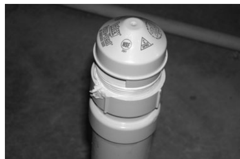
PHOTO 14.14 An air admittance valve (AAV) is a pressure-activated, one-way mechanical venting port used to eliminate the need for venting through roof penetrations. (Used with permission of ABC)
