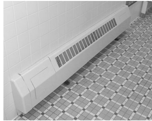
PHOTO 9.5 A baseboard convector typically used in commercial applications. (Used with permission of ABC)
