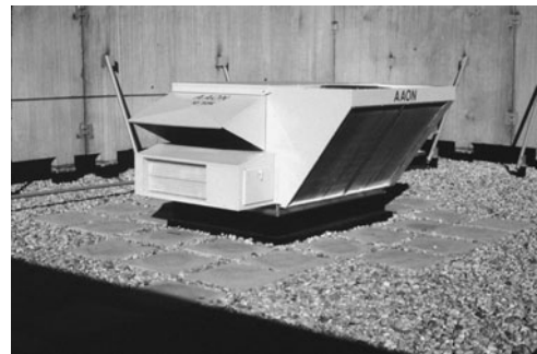
PHOTO 6.19 A 10-ton rooftop PTAC. (Used with permission of ABC)
