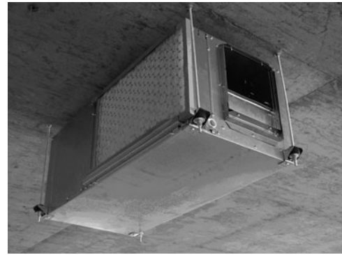
PHOTO 7.45 A water-source heat pump (under construction) for a water-loop heat pump (WLHP) system, which will heat and cool a high-rise condominium unit. (Courtesy of NREL/DOE)
