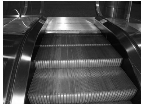
PHOTO 24.10 An upper landing of an escalator. Note how the stairs fold in at the top of the escalator.
