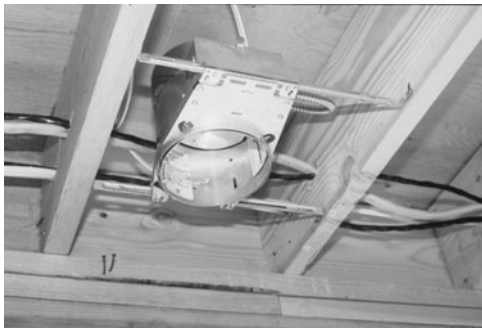
PHOTO 19.17 Roughed-in recessed light fixture. (Used with permission of ABC)
