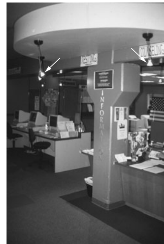
PHOTO 20.30 Decorative halogen accent lighting can add interest to a space but can also cause glare. These eye-level accent lights were intended to provide accent and task lighting, but they adversely affect visual comfort from glare at eye level. (Used with permission of ABC)
