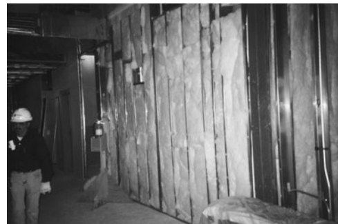
PHOTO 3.7 Blanket insulation installed between the cavities of wall studs or joists. (Used with permission of ABC)
