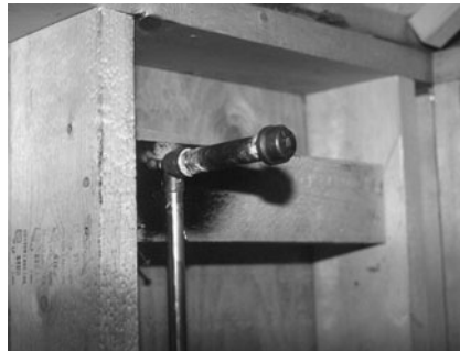
PHOTO 13.10 The rough-in connection for a showerhead. (Used with permission of ABC)
