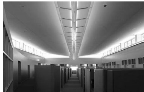
PHOTO 20.40 Side lights and a roof monitor in the center of the ceiling throws natural light evenly. (Courtesy of NREL/DOE)
