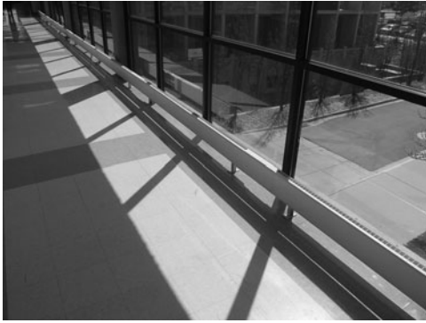
PHOTO 9.6 A convector-radiator. (Used with permission of ABC)
