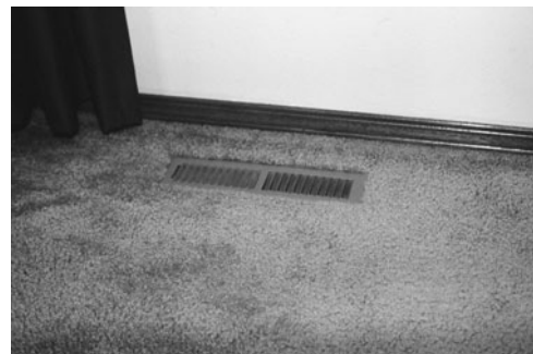
PHOTO 8.5 A floor register fits in the opening created for the register box fitting. Louvers and a damper of the register control airflow. (Used with permission of ABC)
