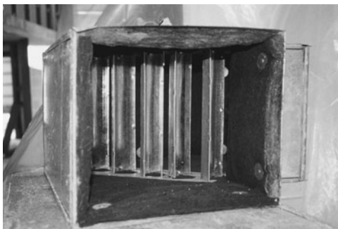
PHOTO 7.7 Turning vanes inside a lined rectangular bend. Turning vanes reduce pressure drop in a bend. (Used with permission of ABC)
