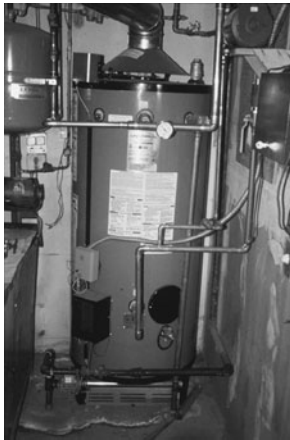
PHOTO 13.32 A commercial, gas-fired storage tank water heater. (Used with permission of ABC)
