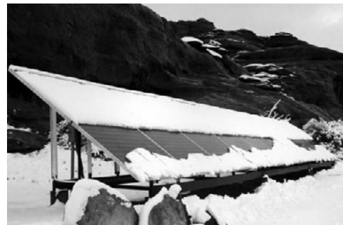
PHOTO 25.27 A PV array at the Needles general store and campground in Canyonlands National Park, Utah. Output varies with snow cover. (Courtesy of DOE/NREL)
