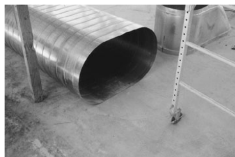
PHOTO 7.4 A section of unlined oval duct. (Used with permission of ABC)
