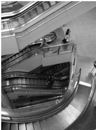
PHOTO 24.7 Various types of escalators.
