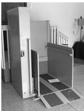
PHOTO 24.15 A wheelchair lift in a residential garage. (Used with permission of ABC)
