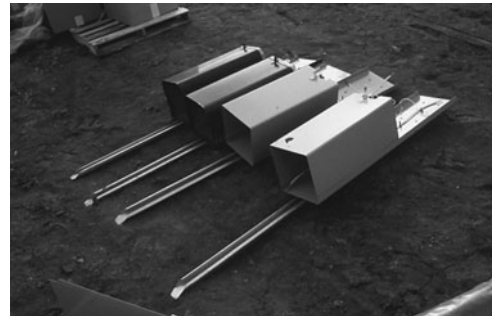
PHOTO 19.4 Power pedestals prepared for installation. (Used with permission of ABC)
