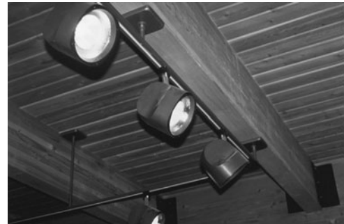
PHOTO 20.18 A track lighting installation. (Used with permission of ABC)
