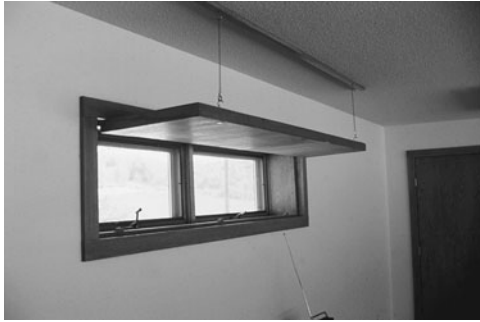
PHOTO 11.16 Insulating shutters on a passive solar system enhance the thermal insulating capability and reduce heat loss through the building envelope. (Used with permission from ABC)
