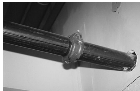
PHOTO 21.9 A Victaulic coupling is a quick method of joining sprinkler pipes. (Used with permission of ABC)
