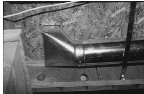
PHOTO 7.9 A register box fitting installed as part of a branch duct. This fitting introduces air through an opening in the subfloor to the floor above. (Used with permission of ABC)
