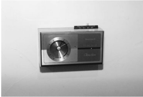
PHOTO 7.41 An electromechanical, clock-type thermostat. (Used with permission of ABC)
