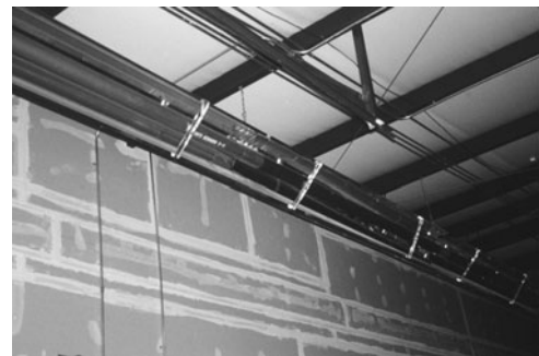
PHOTO 6.15 The heated tube and reflector of a gas-fired infrared heater are mounted at the ceiling-wall line. The heated tube emits radiant thermal energy to the space without directly heating the air. The reflector directs thermal radiation to the space, which improves efficiency of the unit. (Used with permission of ABC)
