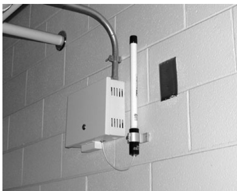
PHOTO 22.15 A wireless access point (station). (Used with permission of ABC)
