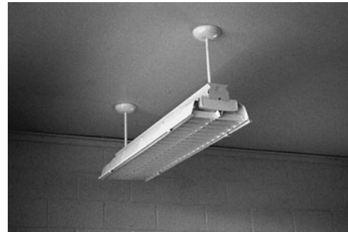
PHOTO 20.21 A linear fluorescent luminaire. Baffles create openings for emitting light from the fixture but cut down on glare. (Used with permission of ABC)
