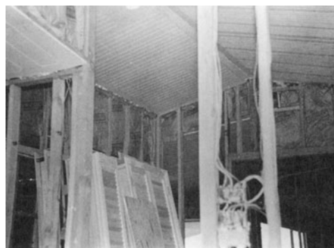
PHOTO 10.3 Electric heating panel for wet plaster ceilings.
