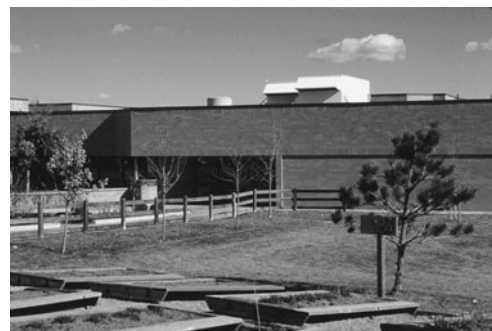
PHOTO 6.20 Rooftop units providing cooling and heating for an elementary school. (Used with permission of ABC)
