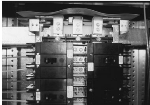
PHOTO 19.33 A close-up view of the three bus bars. (Used with permission of ABC)
