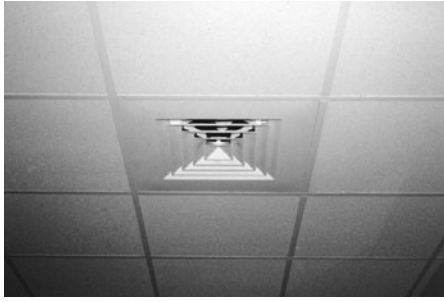
PHOTO 7.13 A ceiling diffuser placed in a suspended ceiling. (Used with permission of ABC)
