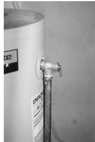
PHOTO 13.26 A temperature-pressure relief valve on a storage tank water heater. (Used with permission of ABC)
