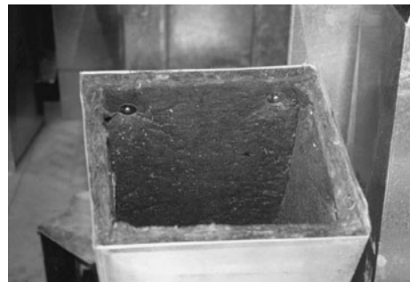
PHOTO 7.2 A section of lined rectangular duct. (Used with permission of ABC)
