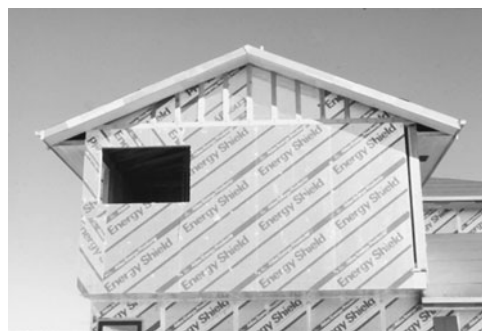
PHOTO 3.12 Foil-faced sheathing improves the thermal performance of insulation by reducing radiant heat transfer in the winter and summer. (Used with permission of ABC)
