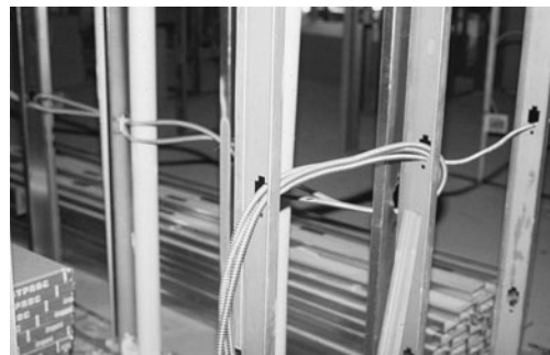
PHOTO 18.18 Armored (AC) in a steel-framed partition. (Used with permission of ABC)
