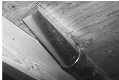
PHOTO 8.3 A fitting called a floor diffuser box or floor register box conveys air to a floor register. (Used with permission of ABC)
