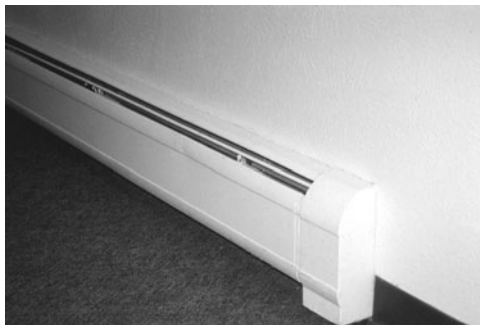
PHOTO 9.4 A baseboard convector typically used in residential installations. The position of the damper will control flow of air from natural convection and thus heat released by the unit. (Used with permission of ABC)
