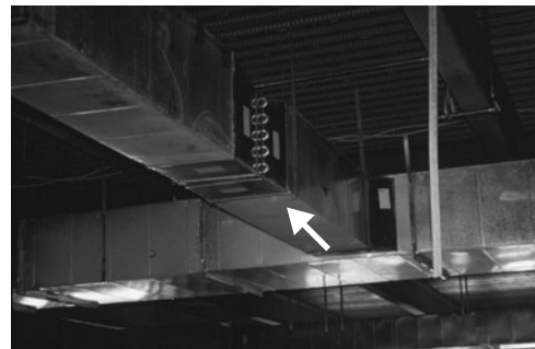
PHOTO 7.21 A reheat coil installed in a duct. (Used with permission of ABC)
