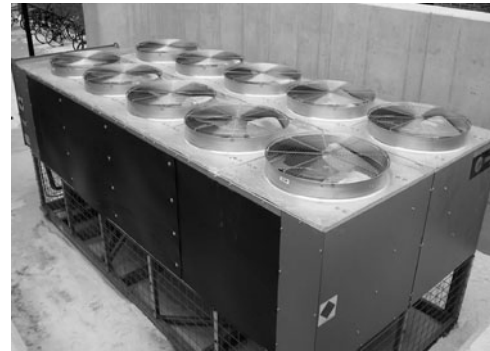
PHOTO 6.22 A packaged, air-cooled condensing unit. (Used with permission of ABC)
