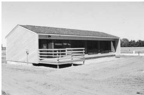
PHOTO 11.22 A simple passive solar residence incorporating direct-gain and unvented thermal storage wall systems. (Used with permission from ABC)
