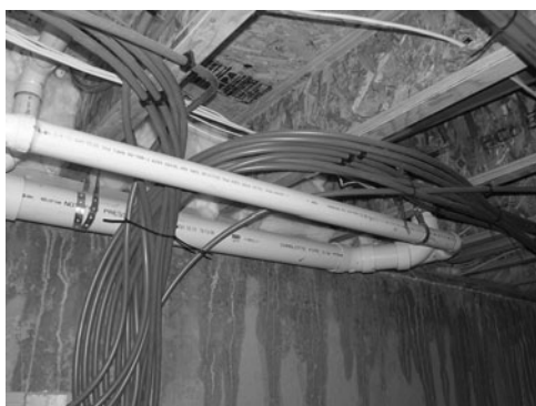
PHOTO 13.21 Water lines dedicated to each fixture run from the manifold to the individual fixture. Because of the flexibility of PEX pipe, fittings are not needed except at the start (manifold port) and end (fitting at fixture). (Used with permission of ABC)
