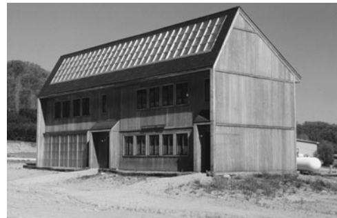
PHOTO 11.19 A passive solar residence with direct gain (small windows), thermal storage wall (large glazing on lower ground level) and attic sunspace systems (on roof). (Courtesy of DOE/NREL)
