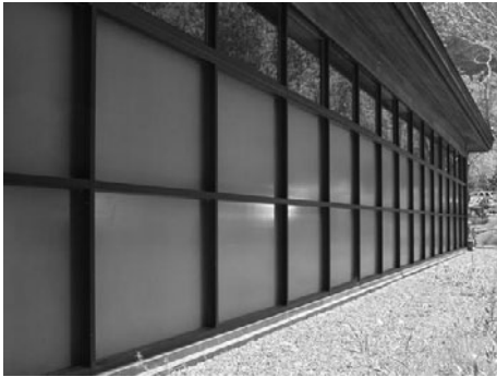
PHOTO 11.21 The trombe wall entails the lower obscured (but translucent) glass sections. It is exposed to direct sunlight (unshaded) during winter months and is shaded by the overhangs during the summer months. Heat from the sun is trapped between the translucent panes of glass and black selective coating on a masonry wall. The wall stores solar heat for later release into the building. (Courtesy of DOE/NREL)
