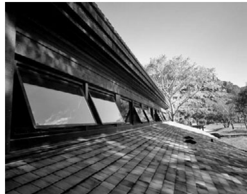
PHOTO 11.44 Clerestory windows at the Zion Visitor Center provide daylighting and ventilation. (Courtesy of DOE/NREL)
