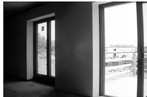
PHOTO 11.25 An interior view of the direct-gain glass and unvented thermal storage wall. (Used with permission from ABC)
