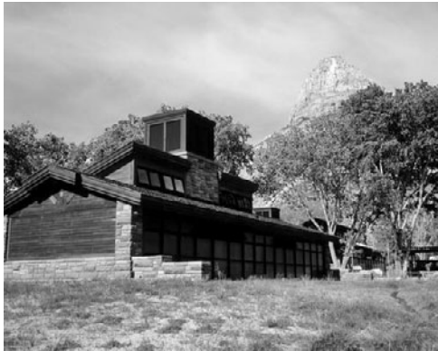
PHOTO 11.40 The trombe wall, clerestory windows, and passive downdraft evaporative cooling (PDEC) tower of the Zion Visitor Center. (Courtesy of DOE/NREL)
