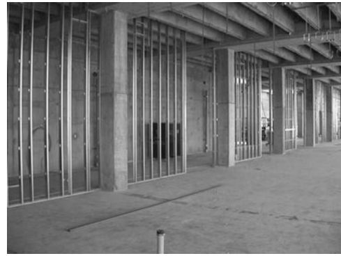
PHOTO 3.1 Cast-in-place (in situ) concrete is a heavyweight construction system. (Courtesy of DOE/NREL)
