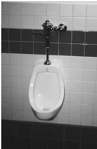
PHOTO 12.12 A wall-mounted, flush valve urinal. (Used with permission of ABC)
