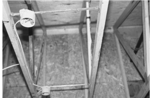
PHOTO 19.16 Roughed-in lighting box. (Used with permission of ABC)
