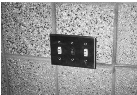
PHOTO 20.33 Ganged (multiple) key switched. Key switches are often used in lighting installations to provide better control of lighting (accidental or disruptive switch off). (Used with permission of ABC)
