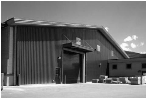
PHOTO 11.14 A transpired solar collector installed on the south wall of a home improvement center. (Courtesy of DOE/NREL)
