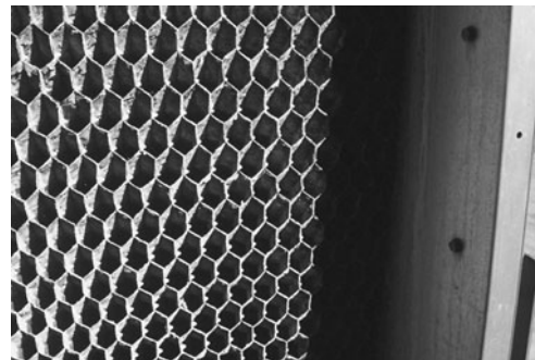
PHOTO 6.29 A close-up view of the fill in a cooling tower. (No water is flowing.) During cooling operations, water trickles down through the fill. The majority of heat removed from the water is by evaporation. (Used with permission of ABC)
