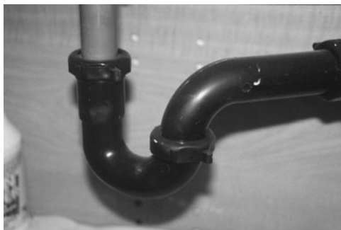
PHOTO 14.1 A P-trap. (Used with permission of ABC)
