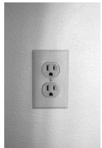
PHOTO 19.21 Covered convenience receptacle. (Used with permission of ABC)
