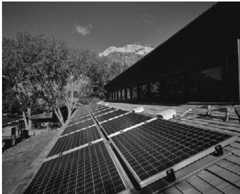
PHOTO 11.45 Rooftop photovoltaic (PV) solar collectors at the Zion Visitor Center provides electricity. PV technology is covered in Chapter 25. (Courtesy of DOE/NREL)
