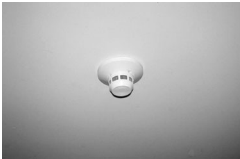
PHOTO 21.22 A smoke detector in a finished ceiling of a commercial building. (Used with permission of ABC)
