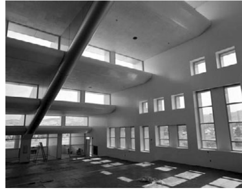
PHOTO 20.38 Stepped windows provide soft, natural lighting to the open office area below. (Courtesy of NREL/DOE)
