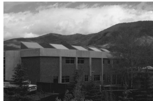
PHOTO 20.34 Skylights on a building roof. (Used with permission of ABC)
