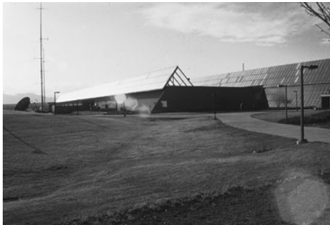
PHOTO 11.4 A commercial active solar installation with almost 4000 flat-plate collectors. (Used with permission from ABC)
