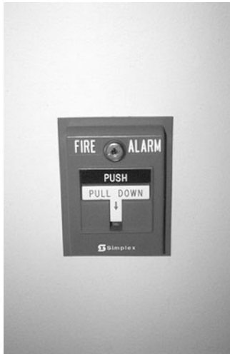
PHOTO 21.24 A manual pull station. (Used with permission of ABC)
