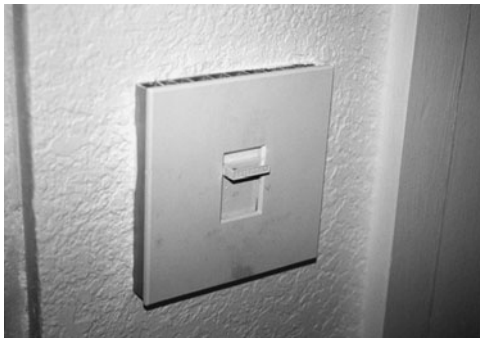
PHOTO 20.32 A wall-mounted dimmer switch used to control several banks of track lights. (Used with permission of ABC)
