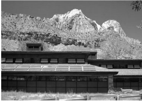
PHOTO 11.39 The south exposure of the Visitor Center at Zion National Park provides a well-suited location for trombe walls that provide most of the building's heat. In addition, a 7.2 kW photovoltaic array provides a significant portion of the electricity needed by the building and serves as an uninterrupted power supply for use during power outages. (Courtesy of DOE/NREL)
