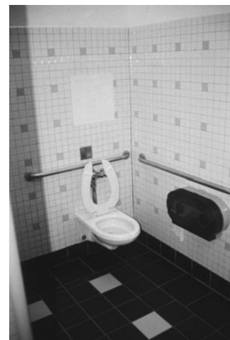
PHOTO 12.32 An accessible water closet with rear and side grab bars. (Used with permission of ABC)
