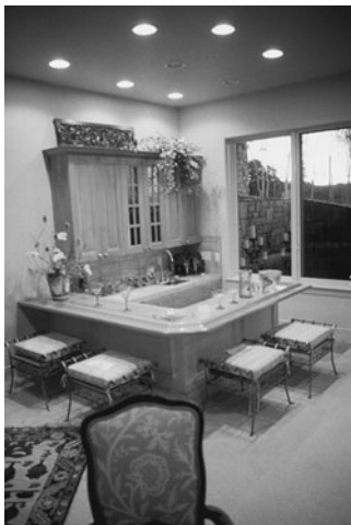
PHOTO 20.27 A bank of recessed luminaries provides ambient and task lighting in a kitchen area. (Used with permission of ABC)
