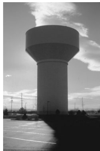
PHOTO 12.1 A private water storage tank. (Used with permission of ABC)
