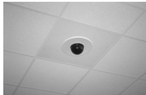
PHOTO 21.30 A remotely controlled closed circuit television (CCTV) video surveillance camera. (Used with permission of ABC)
