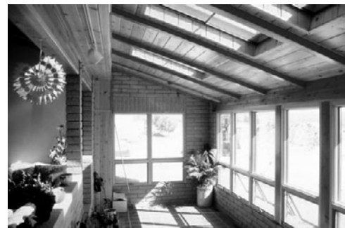
PHOTO 11.34 Thermal mass in this passive solar sunspace absorbs solar energy during the day without overheating the sunspace area receiving the direct sunlight. During the evening, thermal mass releases energy reducing the daily temperature swing (fluctuation) in the area. (Courtesy of DOE/NREL)
