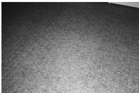
PHOTO 22.14 Raised floor system (closed). (Used with permission of ABC)
