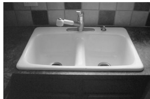
PHOTO 12.25 An enameled cast iron kitchen sink. (Used with permission of ABC)
