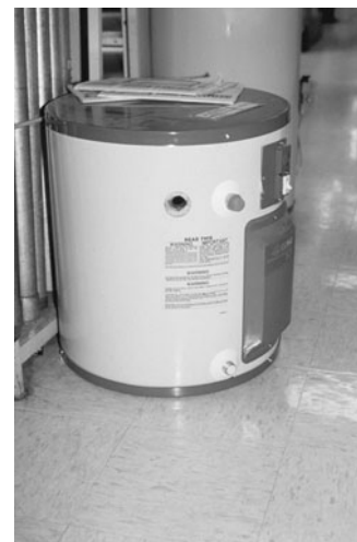
PHOTO 13.31 A short storage tank water heater. (Used with permission of ABC)
