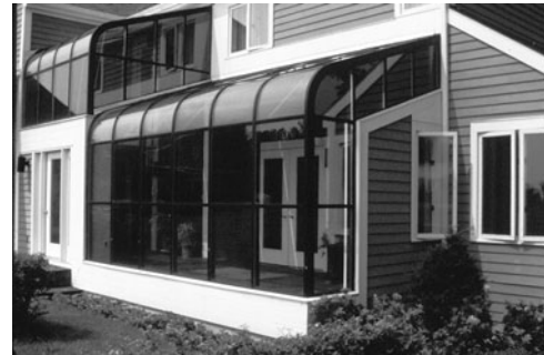
PHOTO 11.33 A commercially available attached sunspace. (Used with permission from ABC)
