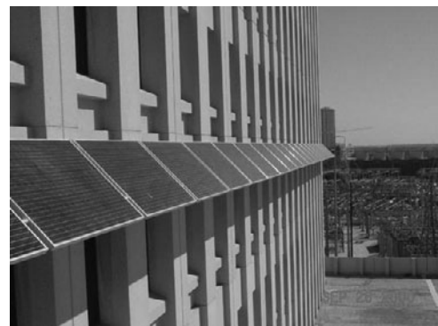
PHOTO 25.18 A 7-kW photovoltaic awning is situated above the eighth-floor windows of the 26-story University Center Tower on the Texas Medical Center campus in Houston, Texas. (Courtesy of DOE/NREL)
