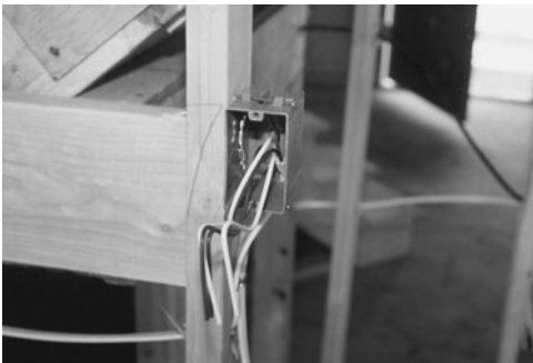
PHOTO 19.19 Roughed-in receptacle box. (Used with permission of ABC)
