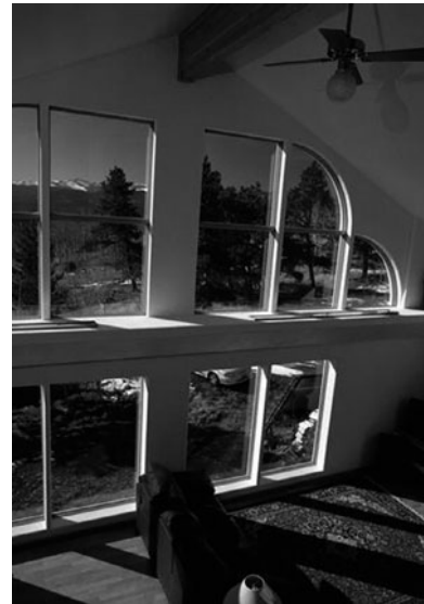
PHOTO 11.17 A direct-gain passive solar system. (Courtesy of DOE/NREL)
