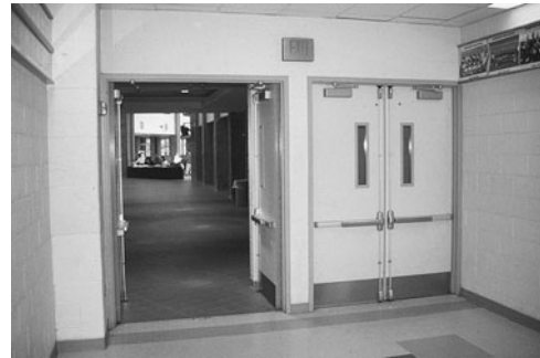
PHOTO 21.1 Fire separation doors are used to compartmentalize the building. (Used with permission of ABC)
