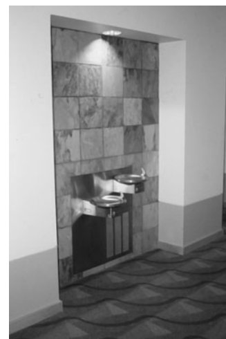
PHOTO 20.4 Local lighting used to highlight a task area. (Used with permission of ABC)
