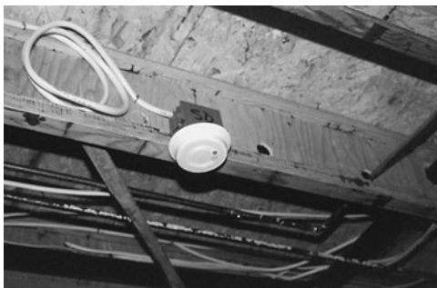
PHOTO 21.23 A hard-wired smoke alarm in an unfinished ceiling of a residence. (Used with permission of ABC)
