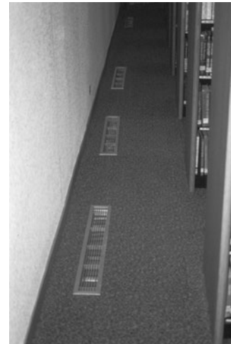
PHOTO 7.18 Floor registers located along an exterior wall. (Used with permission of ABC)
