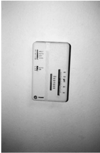
PHOTO 7.42 A programmable, electronic thermostat. (Used with permission of ABC)
