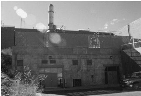
PHOTO 6.4 The main power plant facilities for an institutional building. (Used with permission of ABC)
