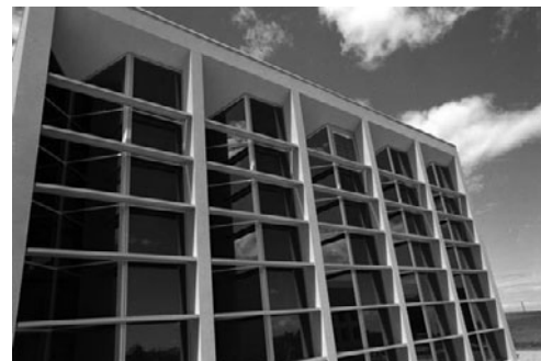
PHOTO 11.27 The articulated thermal storage wall at the NREL Visitor Center, Golden, Colorado. (Courtesy of DOE/NREL)
