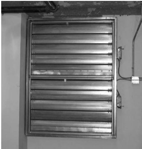
PHOTO 7.12 A parallel blade damper. (Used with permission of ABC)
