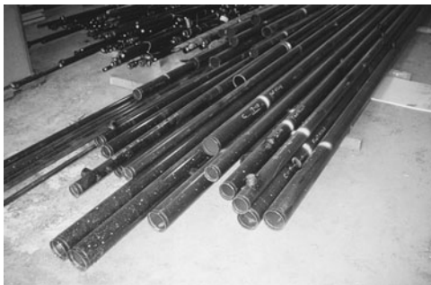
PHOTO 21.6 Sprinkler pipe precut, numbered, and ready for installation. (Used with permission of ABC)
