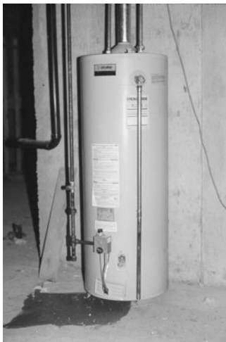
PHOTO 13.28 A residential storage tank water heater. (Used with permission of ABC)
