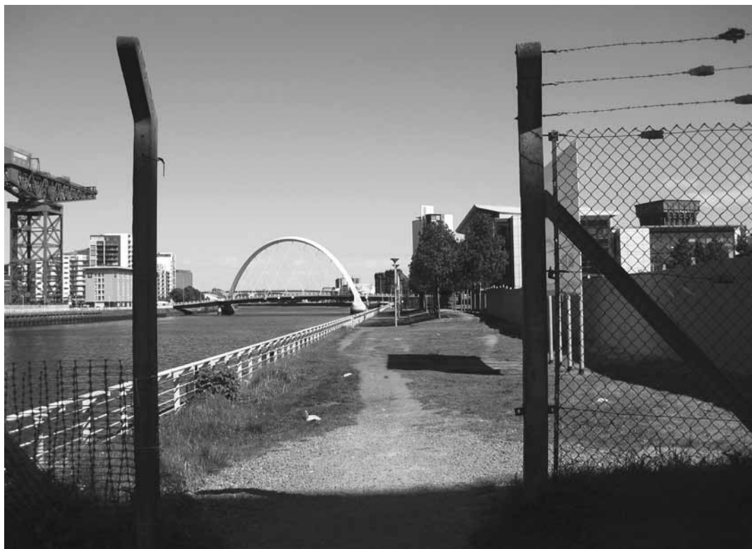
6.14 Accessibility of the Pacific Quay site. (b) The connection from the northern edge, on Bell's Bridge
