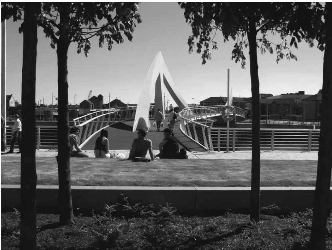
6.41 The new pedestrian and cycle bridge at Broomielaw
