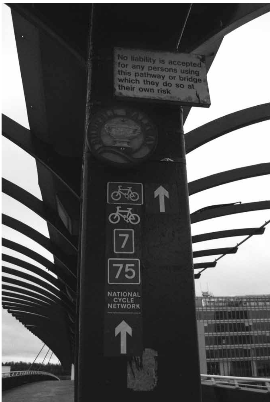
6.14 Accessibility of the Pacific Quay site. (a) The connection from the eastern edge
