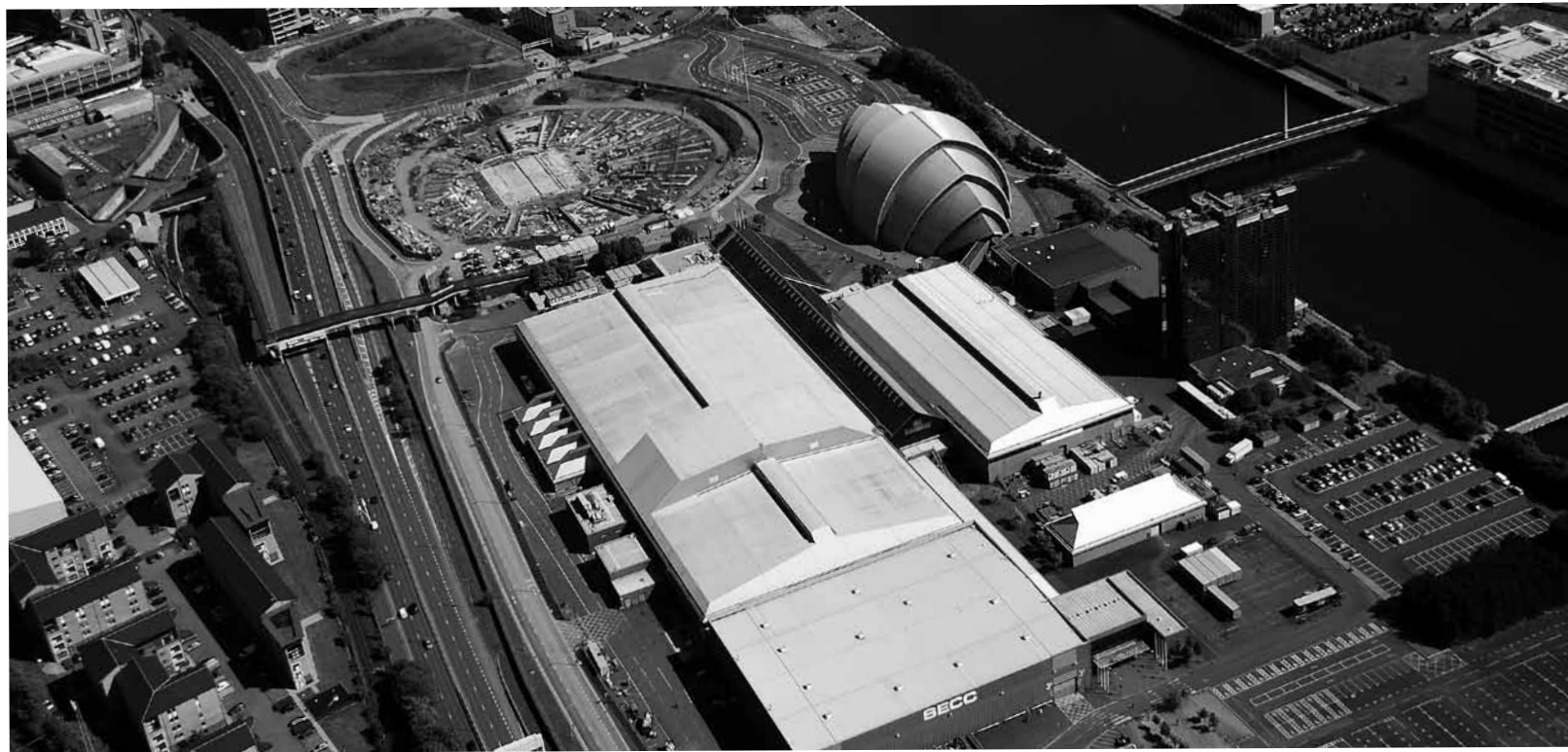
5.6 The Scottish Exhibition and Convention Centre (SECC) – the first large public amenity building on the post-industrial waterfront of the Clyde. Courtesy of Scottish Enterprise
