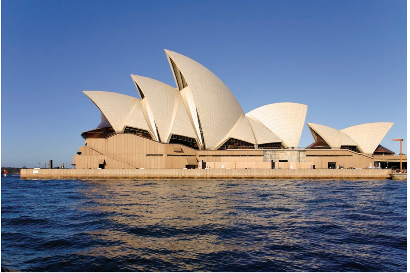
Plate 24. Shell and podium structure of the Sydney Opera complex. Photo by Matthew Field
