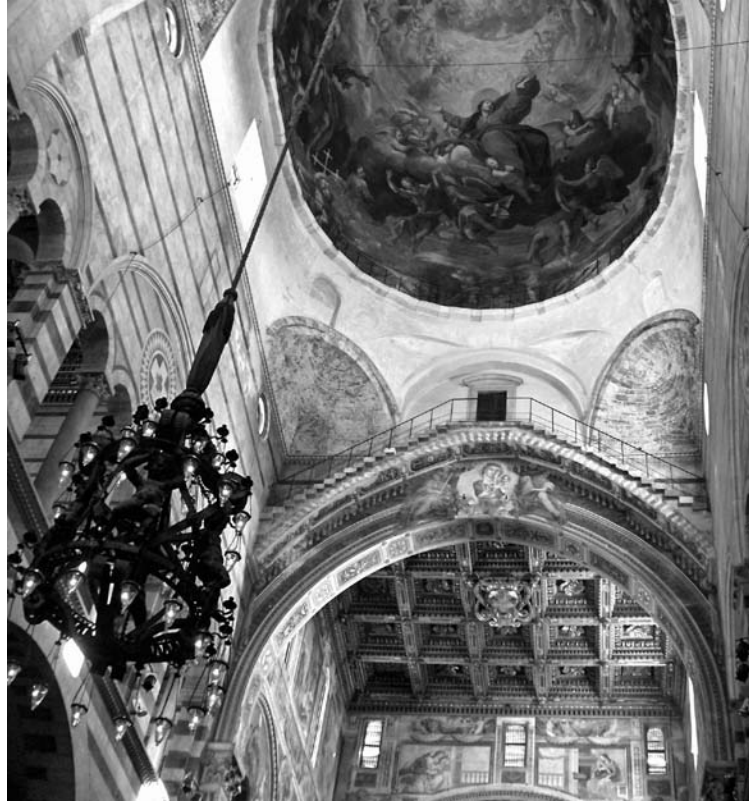
Figure 3.37. The arches and squinches that support the vault and dome of the Cathedral of Pisa. Photo by JoJan
