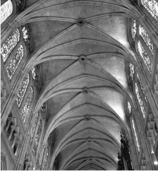
Figure 3.21. Ribbed vaults over several bays in the ceiling of a Gothic cathedral. Photo by Magali Ferare
