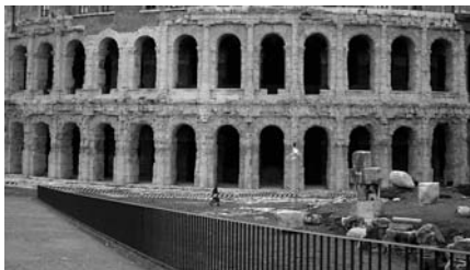
Figure 2.36. Remaining wall structure of the Theater of Marcellus, Rome. Photo by Joris van Rooden
