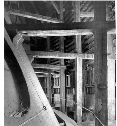
Figure 6.3. Inner timber structure resting on the brick cone in support of the outer dome. Conway Library, The Courtauld Institute of Art, London. Photo by A. F. Kersting
