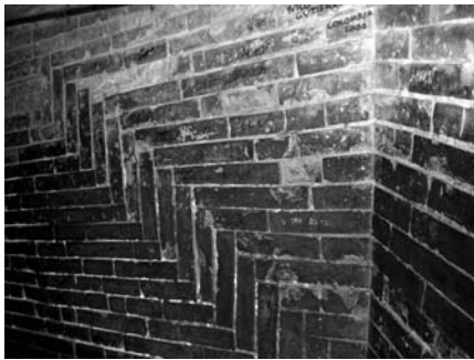
Figure 4.30. Herringbone brickwork pattern in the two shells. Photo by Philip Holtzman and Rose Holtzman
