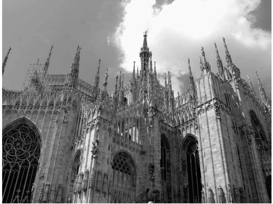
Figure 3.31. A view of the exterior, including the apse, transept, and the tower over the crossing of the Milan Cathedral. Photo by Fabio Alessandro Locati
