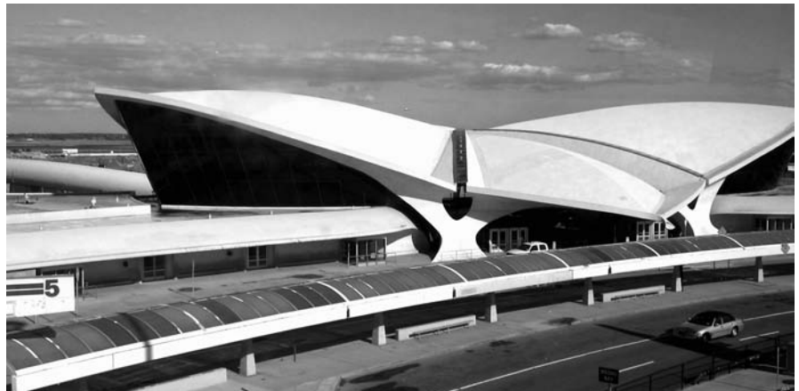
Figure 7.29. Saarinen's terminal at JFK showing three of the four vaults and two of the Y-shaped columns. Photo by Pheezy
