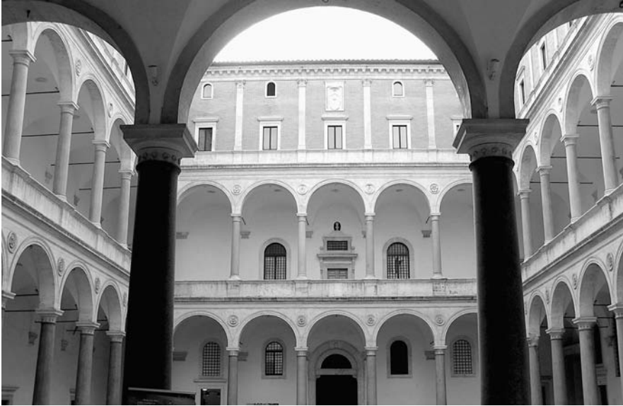
Figure 5.3. Courtyard of the Palazzo della Cancelleria, the Vatican Chancellery, 1489–1513, Rome. Architect unknown. Possibly by Francesco di Giorgio. Incorrectly attributed to Donato Bramante. Photo by Emmanuel Brunner
