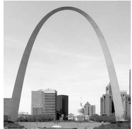
Figure 7.20. The Gateway Arch in St. Louis. Photo by Bev Sykes
