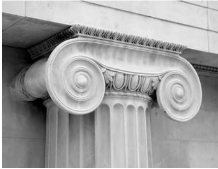
Figure 5.65. An Ionic column in the British Museum, London. Photo courtesy Wayne Boucher, © Cambridge 2000
