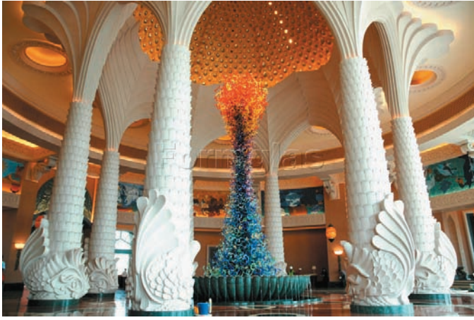
FIGURE 7.3 Over 57,000 pieces of QuarryCast, MetalCast, and Glassfiber Reinforced Gypsum (GRG), representing virtually every column, wall panel, moulding, and so on, are visible in these photographs. Photo courtesy of Formglas.
