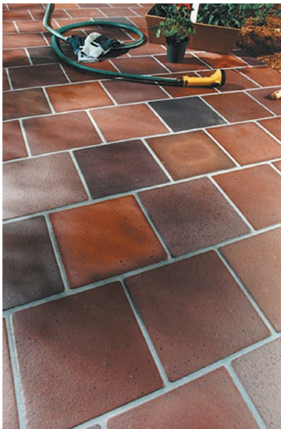
FIGURE 4.12 Notice how the contrasting grout of this quarry tile makes the pattern stand out, whereas if the grout had matched the color of the tile it would give a blended look. Photo courtesy of Seneca Tile.
