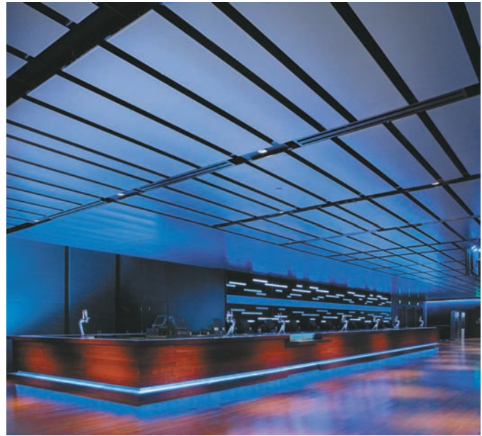
FIGURE 6.4 Gensler Architects of Santa Monica, California, used MetalWorks Custom Plank System for Club Nokia in Los Angeles. Photograph courtesy of Armstrong World Industries.
