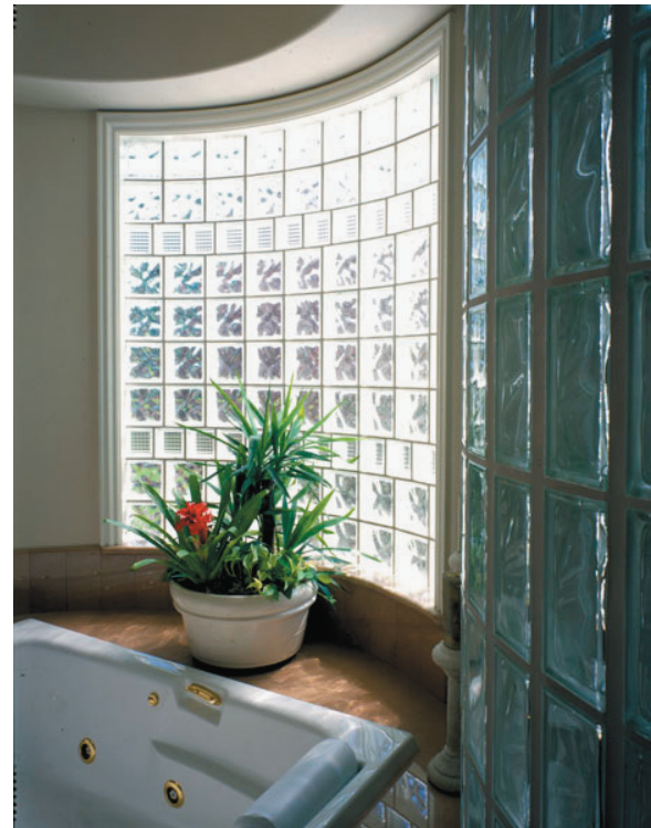
FIGURE 5.7 Private residence. Blocks used are Argus Parallel Flutes and Decora pattern. Photograph courtesy of Pittsburgh Corning Glass Block.
