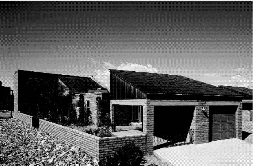
Civano - Solarbuilt Home, Tucson, AZ
