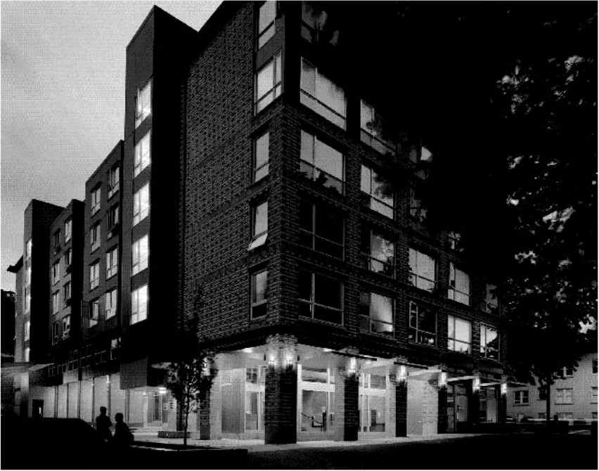
Epler Hall, Portland State University, Portland, Oregon, (Courtesy of Interface Engineering, Inc.)
