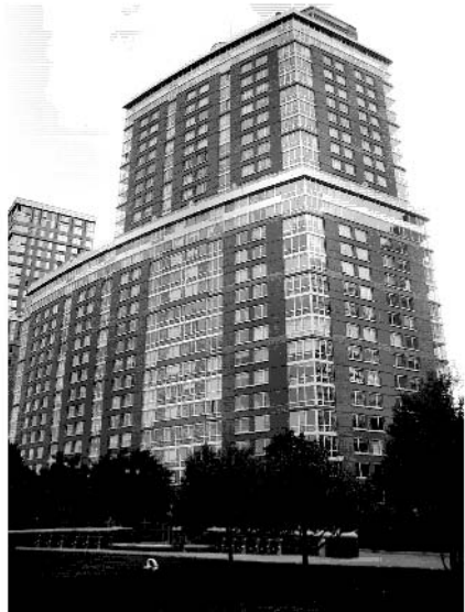
The Solaire, New York, NY (Photo courtesy of the author)
