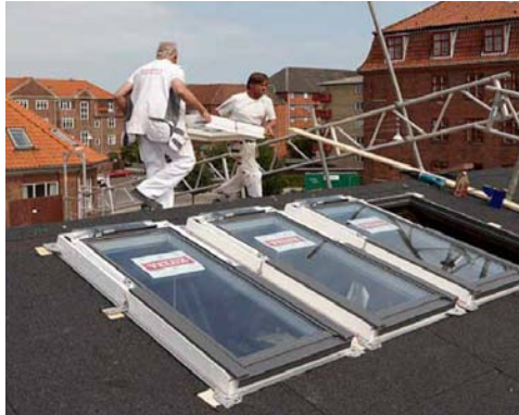
Figure 1: Roof windows installation in a school in Glasgow.
