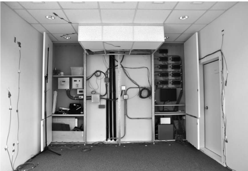
Figure 2: View of Facade Lab interior with remote sensor equipment.
