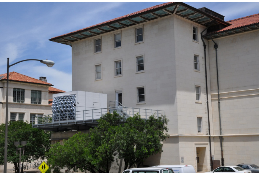
Figure 9: View of experimental prototype shading structure on Facade Lab.
