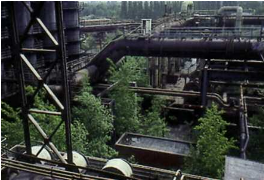
The Landscape Park at Duisburg in the Ruhr Valley, Germany, created around the industrial remains of the redundant steelworks. Regarded by many as one of the finest new memorial landscapes in Europe.
