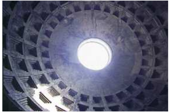
The Pantheon in Rome, built AD 118–25 and a model for many subsequent forms of commemorative architecture: the famous oculus at the apex of the dome lights the whole building.
