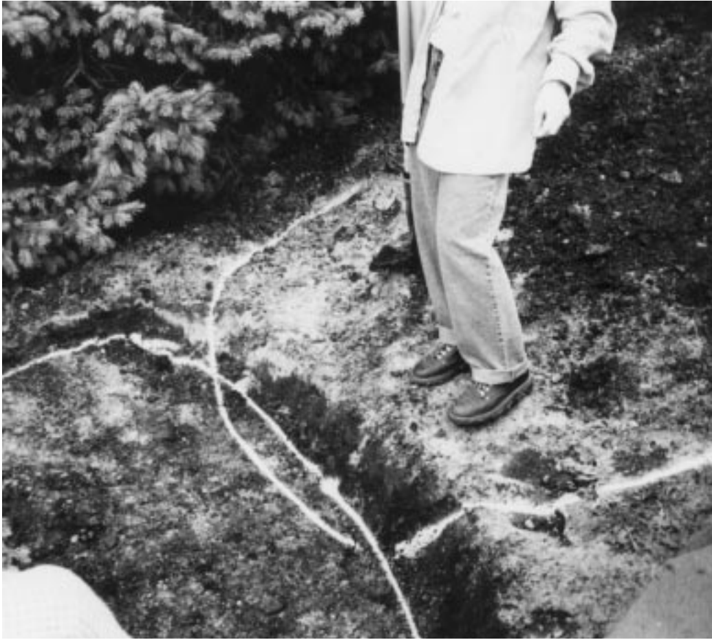
Figure 34–2 Layout of a multilevel water feature to be constructed with flexible pool liners. White lines indicate the approximate outside edge of each pool. Overlap area is where waterfall will be placed.
