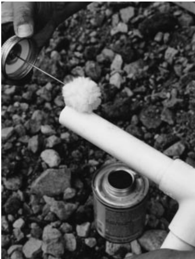
Figure 7-13 Cleaning PVC pipe with pipe-cleaning solution. Clean the outside of the pipe and the inside of the fitting. When dry, liberally apply glue in the same manner. Most cleaning and joining solutions provide a swab applicator in the can.
