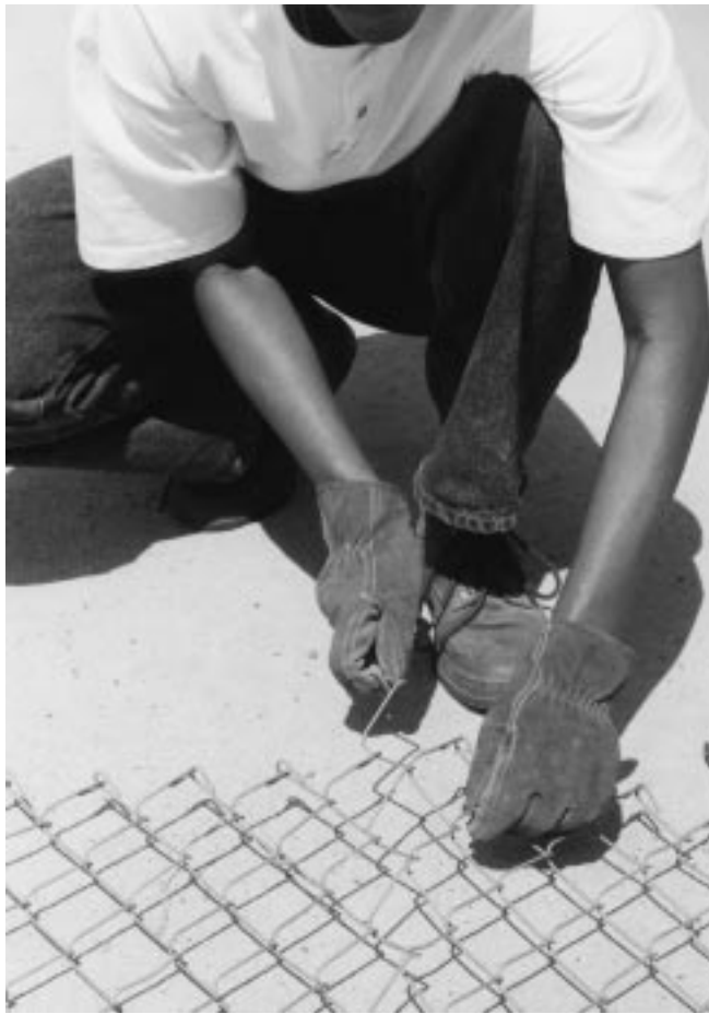
Figure 32–26 Separating links of chain link fencing.
