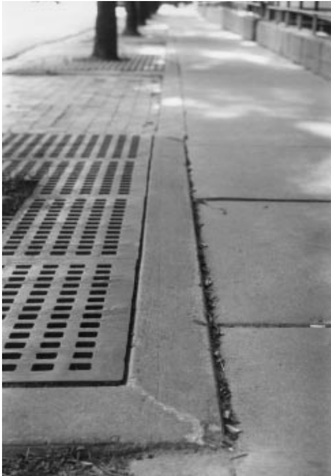
Figure 36-16 Curbing with tree grate in place. Frame for tree grate can be placed in walk or placed in separate curb as shown here.
