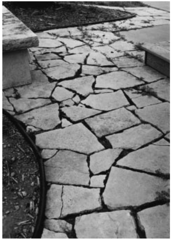
Figure 22-4 Dry-laid stone paving provides texture and natural feel.
