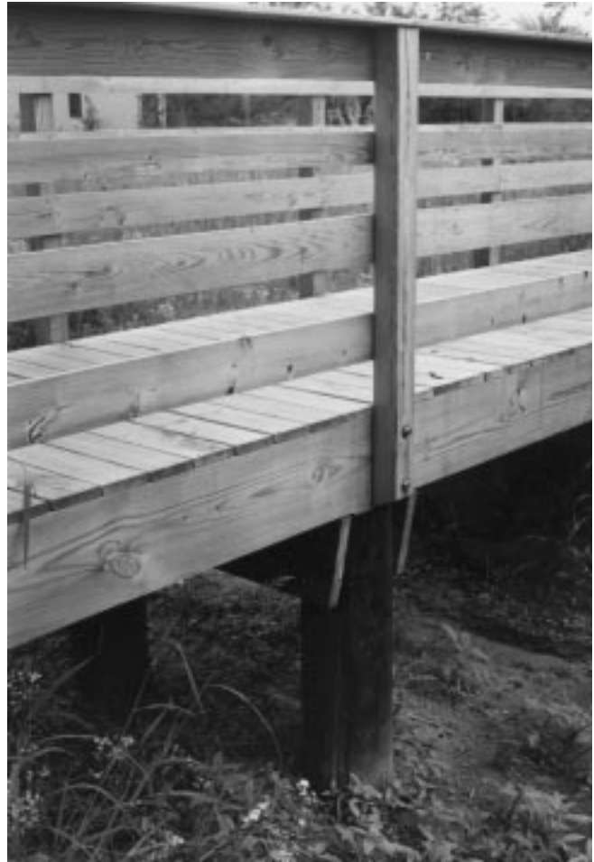
Figure 34–19 Use of posts installed as bridge piers.
