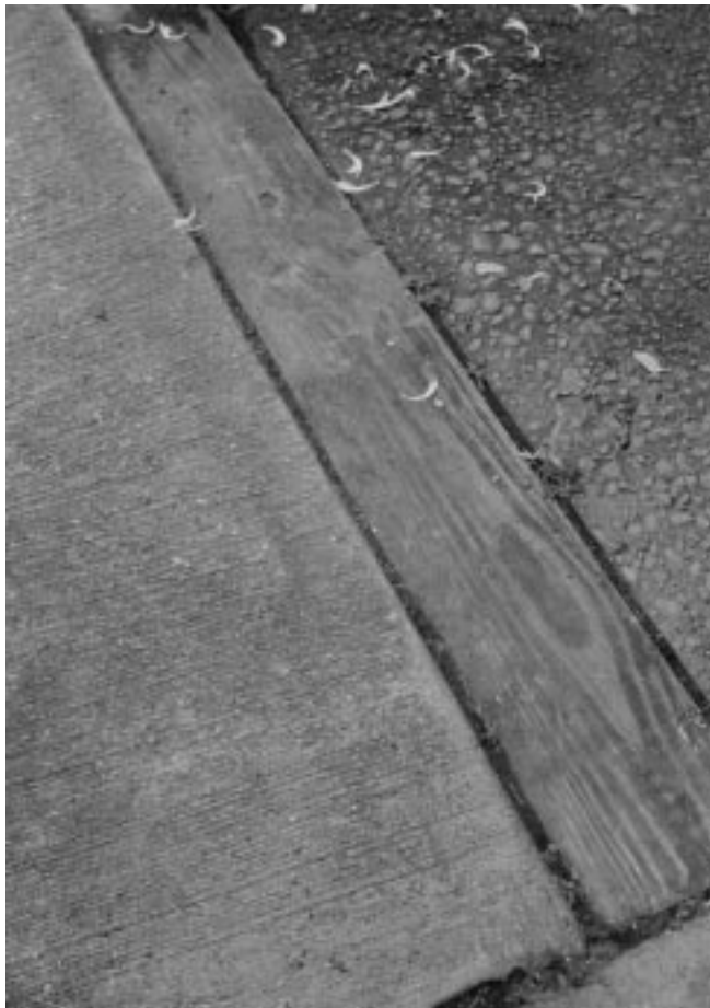
Figure 23–10 Wood header between paved slabs.
