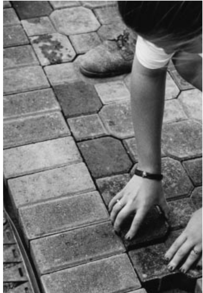
Figure 24–7 Setting cut pavers.
