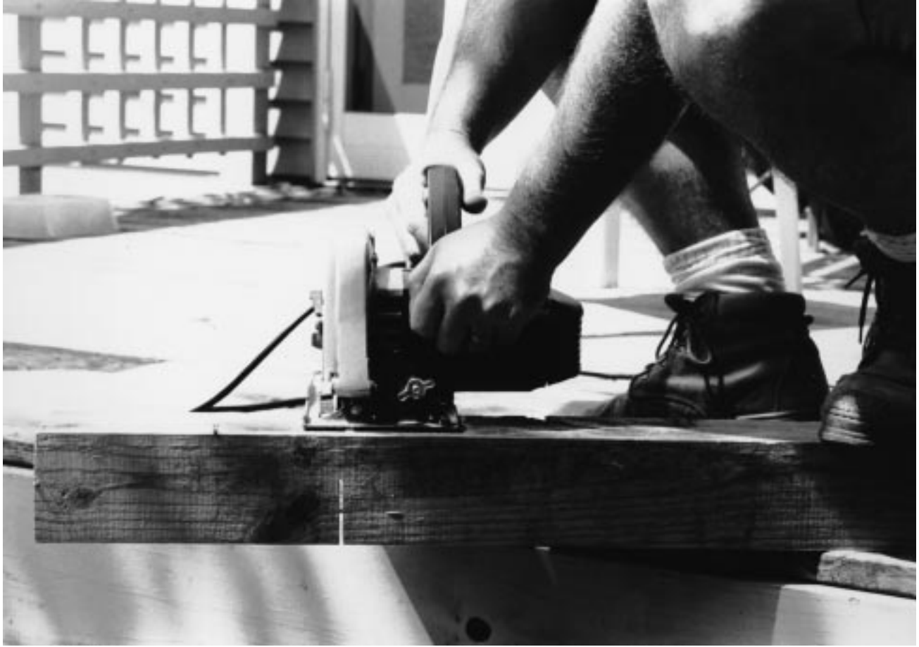
7-20 Proper cutting technique for a circular saw.
