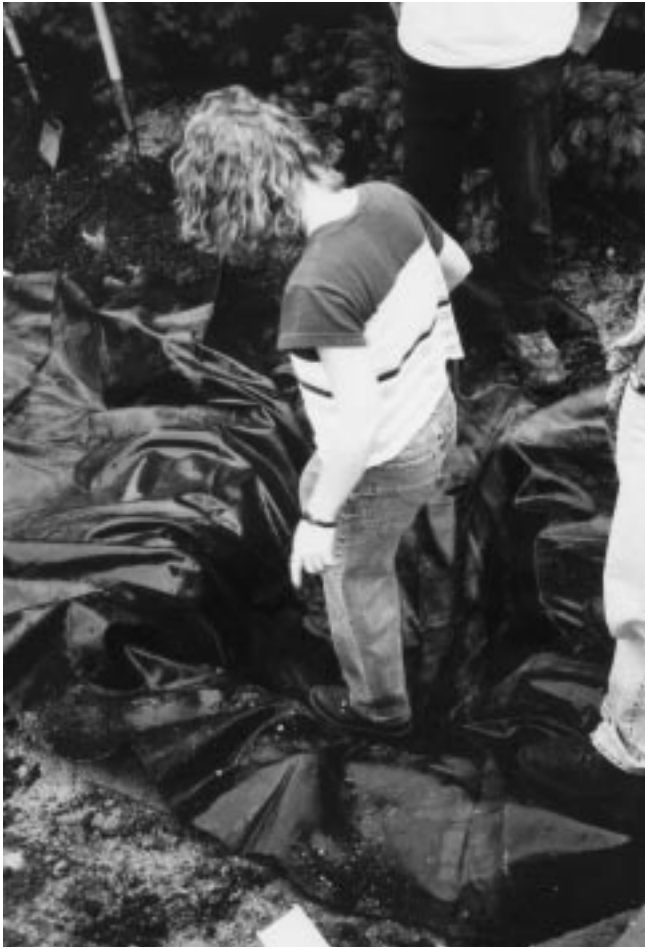
Figure 34-6 Installation of liner in flexible liner pool.
