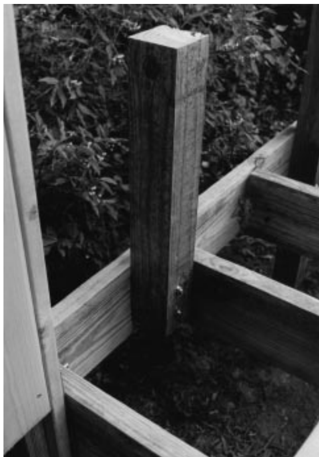
Figure 30–9 Support bolted to inside deck framing.
