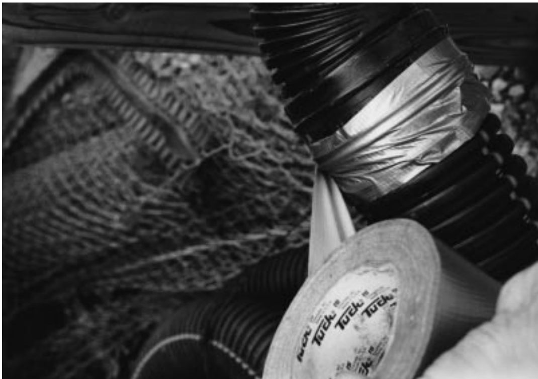
Figure 7-8 Securing corrugated plastic joints with duct tape.
