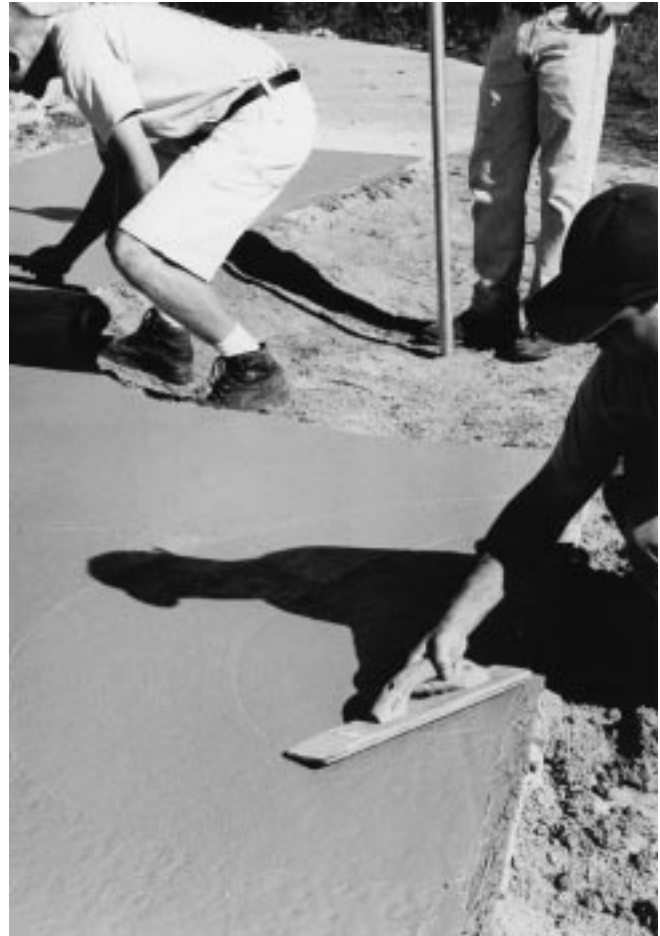
Figure 23–20 Floating a concrete slab from the edge.
