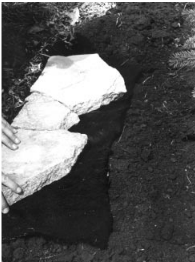
Figure 36–13 Edging with flagstone placed on weed barrier. Straight edge of flagstone is placed along turf edge with irregular edge facing planting bed. Place edging flush with turf and sloping up into planting bed.
