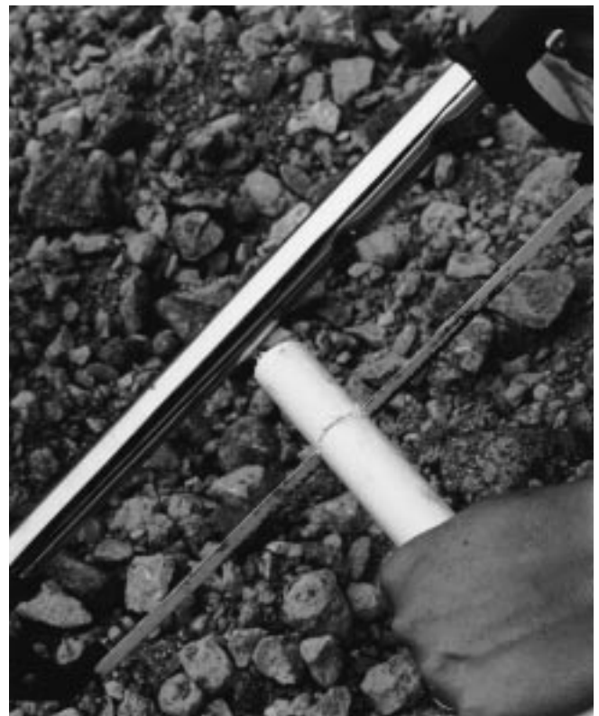
Figure 7-12 Cutting PVC pipe with a hacksaw.
