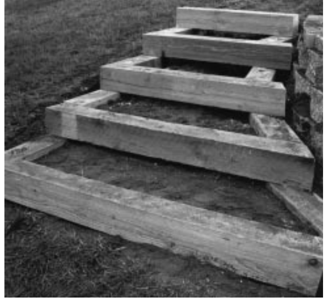
Figure 21-15 Subsequent steps of this freestanding stair installation rest on the sides of the lower stair. Treads will be filled with granular material.
