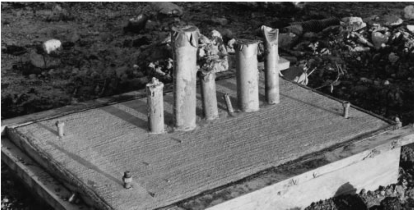
Figure 14–9 Poured concrete footing to which site electrical fixture will be bolted.
