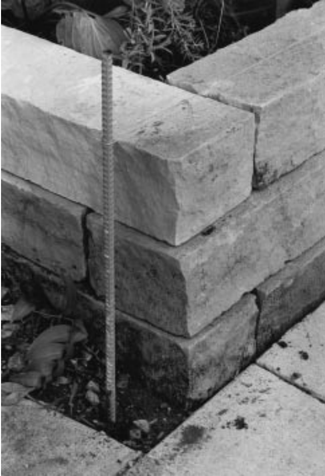
Figure 19–5 Dry-laid stone wall showing interlocking courses at corner.
