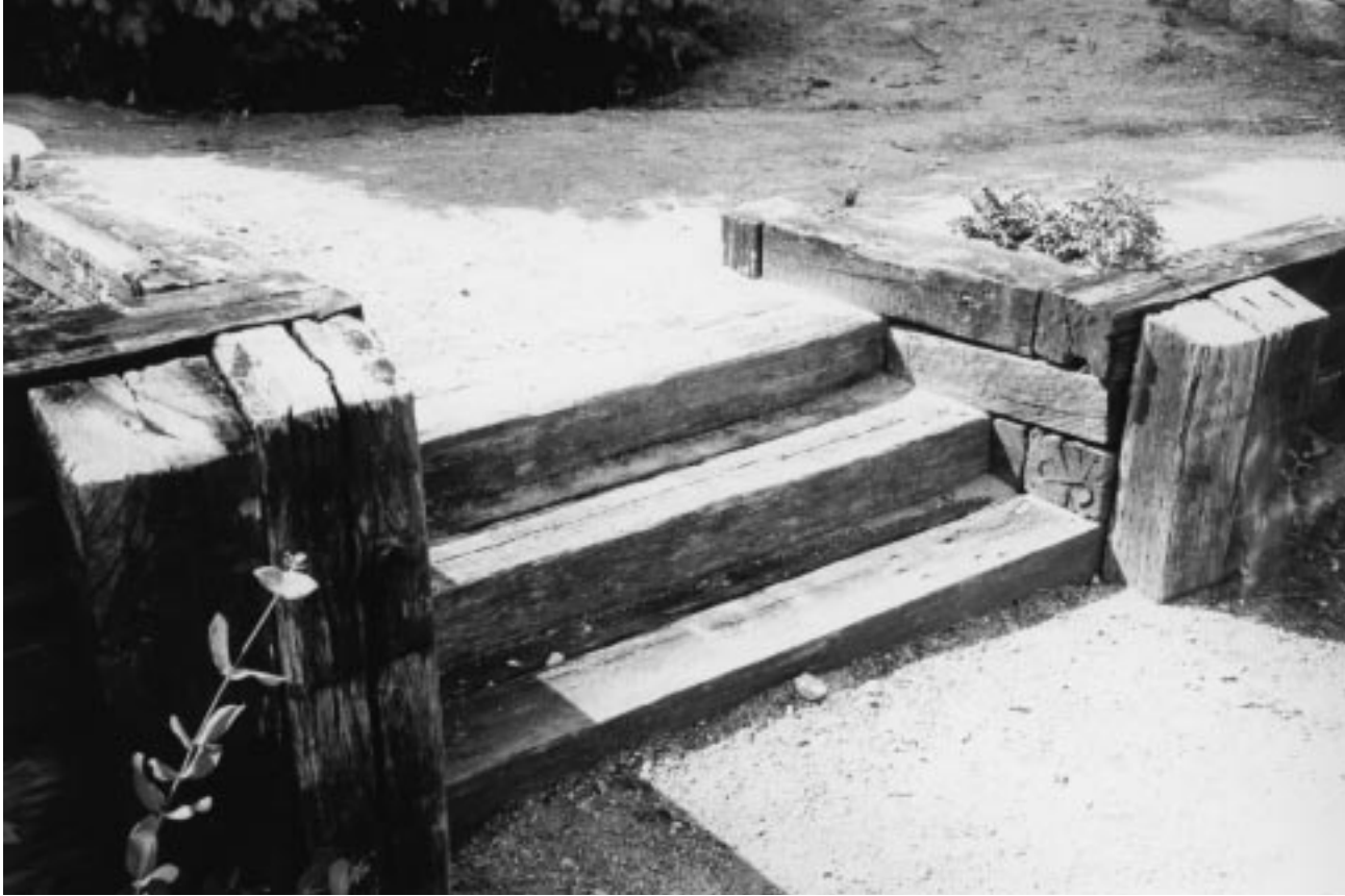
Figure 21-1 Stairs built as part of a wood tie retaining wall installation.
