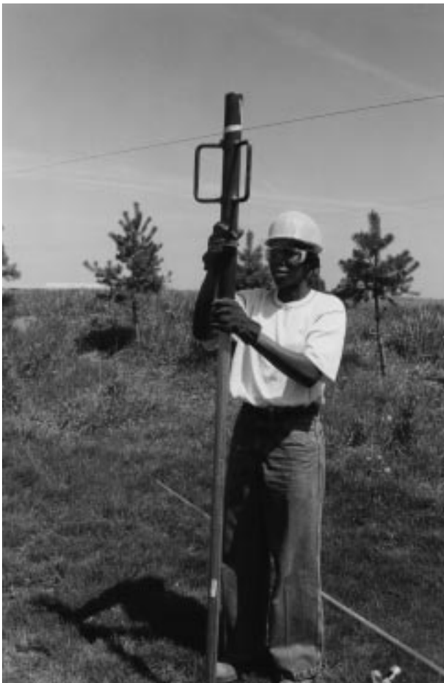
Figure 32–22 Chain link fencing line post driving.
