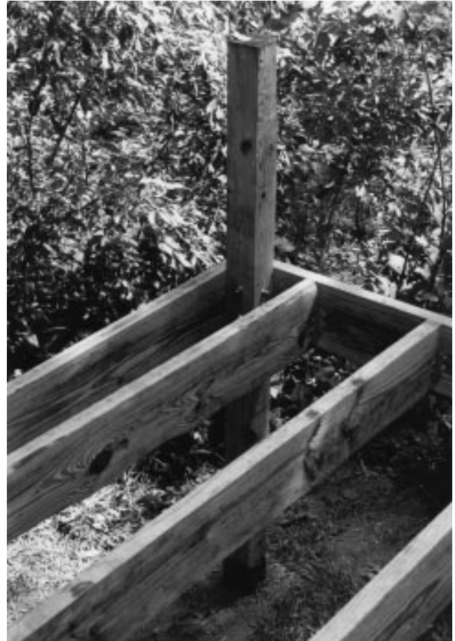
Figure 29–17 Post extensions through deck platform for seating supports.
