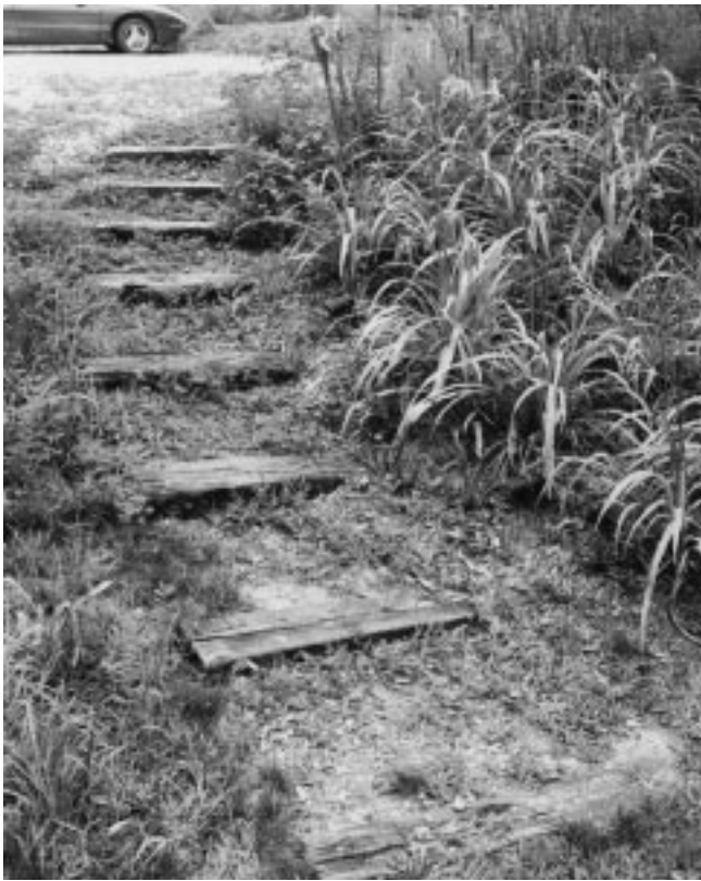
Figure 21-4 Freestanding stairs using railroad ties to create risers with a loose granular material used for the treads.
