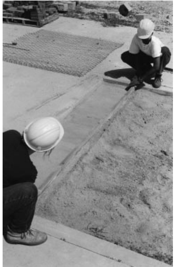
Figure 24-3 Screeding setting bed for unit pavers.
