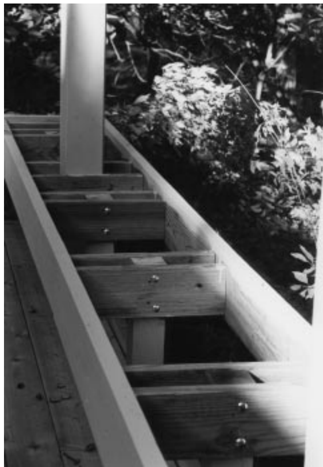
Figure 30-17 Box framing of seating.
