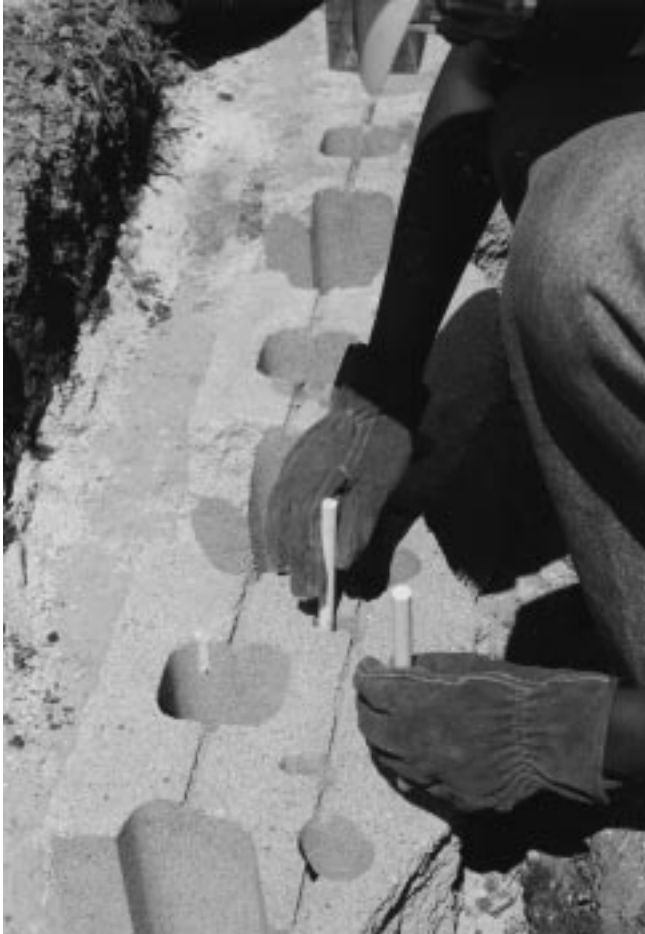
Figure 18-2 Fiberglass pin placement in precast segmental units.
