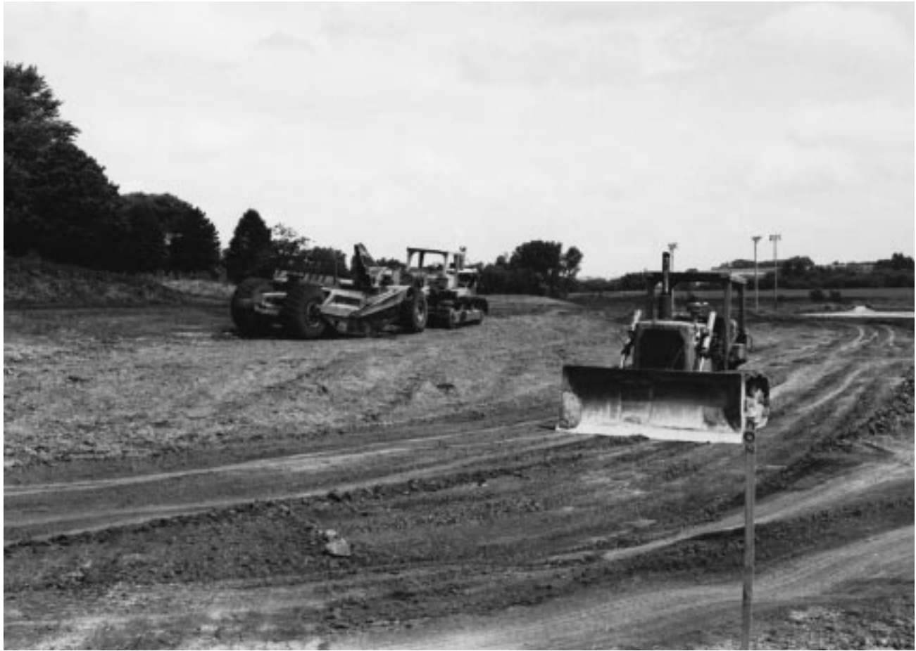
Figure 1-3 Rough grading an athletic field site.
