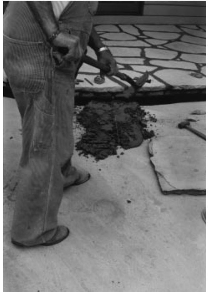
Figure 26-3 Mortar placement.
