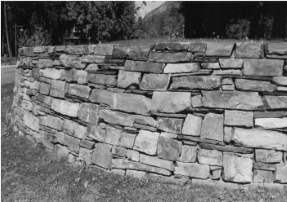
Figure 33-1 Rubble wall.
