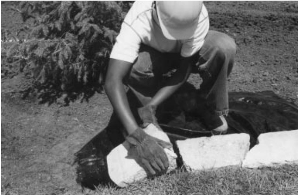
Figure 36–12 Edging with wall stone placed on weed barrier.
