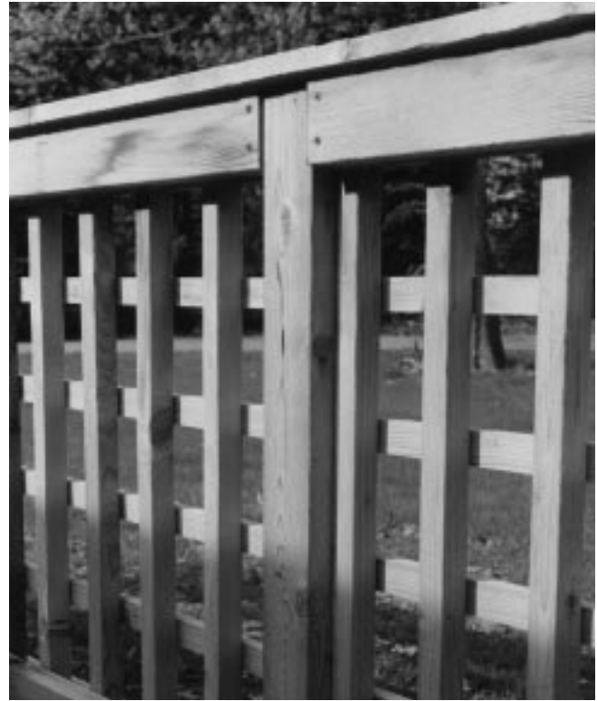
Figure 29–21 Trimming of deck railing.
