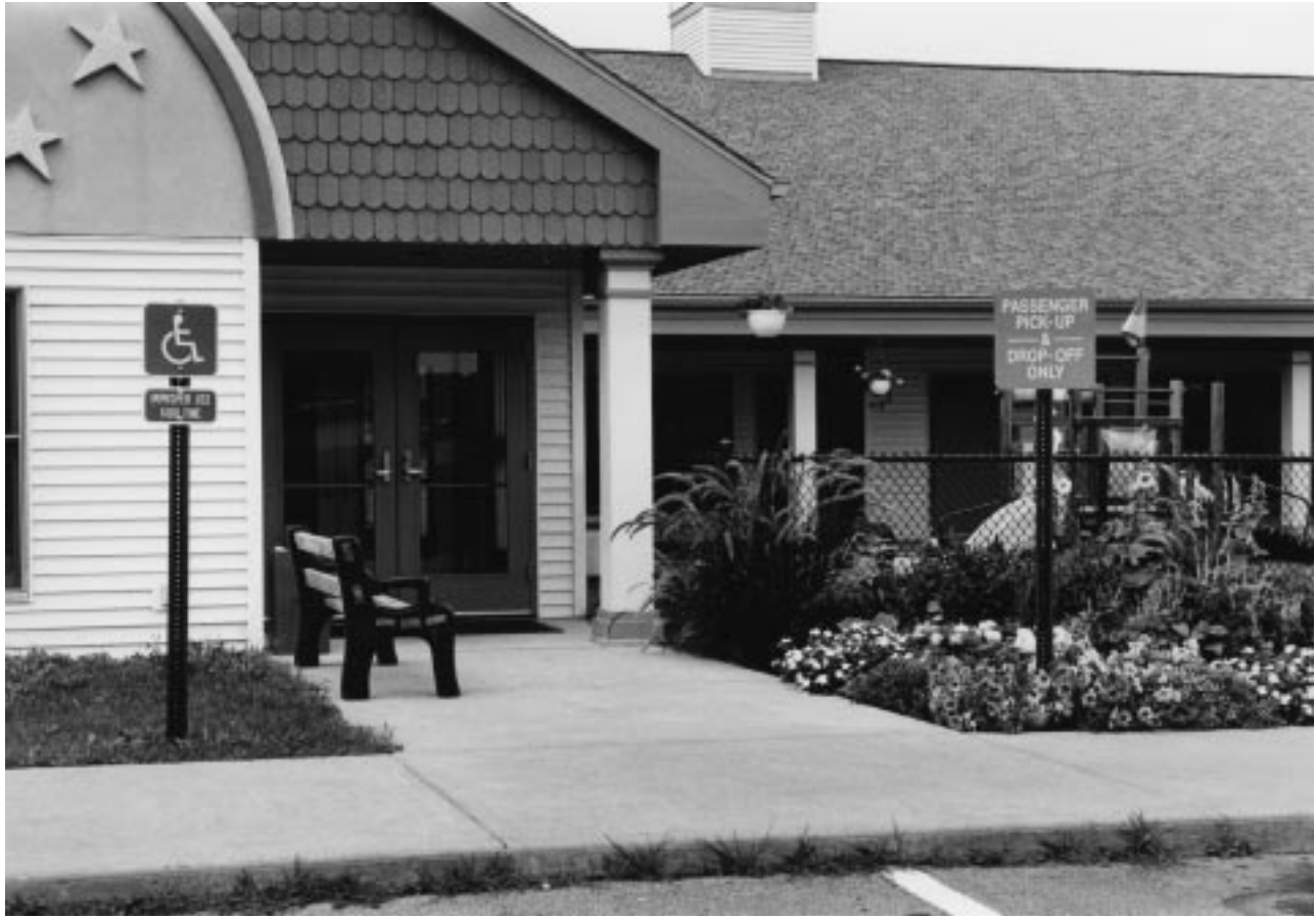
Figure 22-1 Concrete paving is used for this high-traffic entrance.
