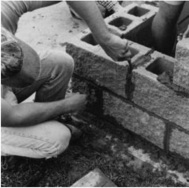
Figure 33–9 Striking joints on a masonry pier.
