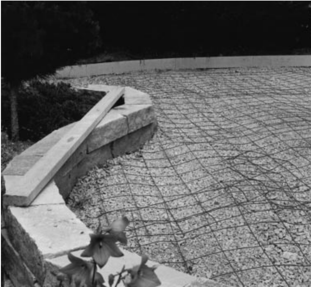
Figure 23–3 Welded wire mesh reinforcing cut and placed before pour.
