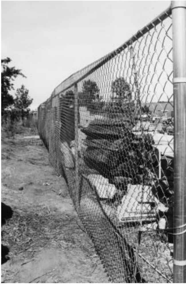
Figure 32-24 Chain link fencing fabric layout.
