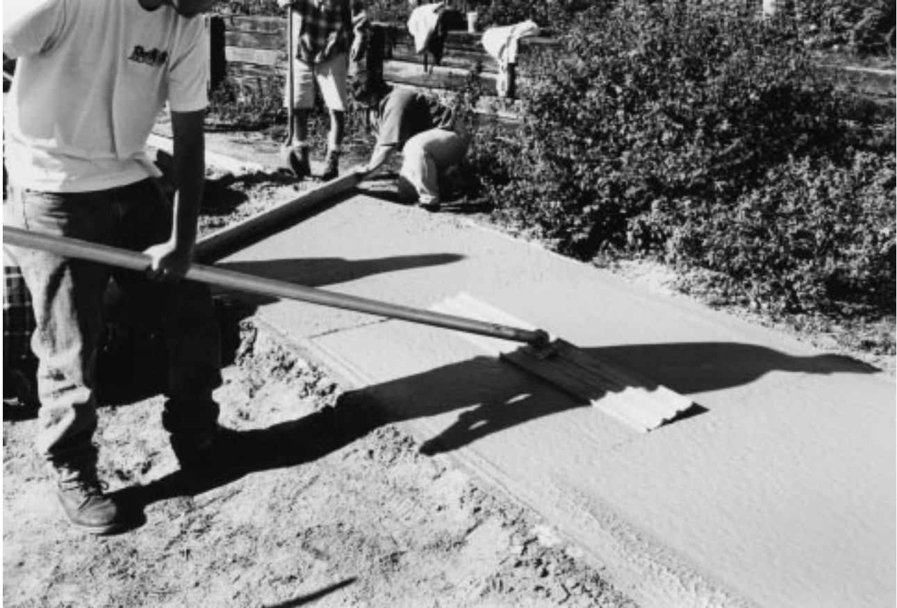
Figure 23–19 Bull floating a concrete slab.
