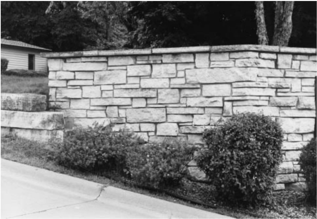
Figure 33-2 Stone masonry wall.
