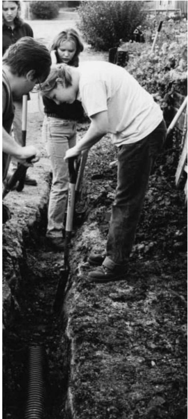
Figure 12–4 Trenching and placing plastic drain tile.
