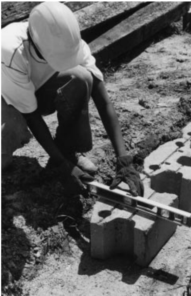
Figure 18-1 Leveling and placement of first units for precast segmental units.
