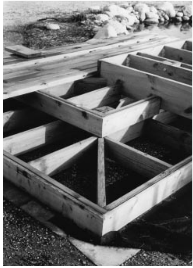
Figure 30-5 Framing for stairs with corners.
