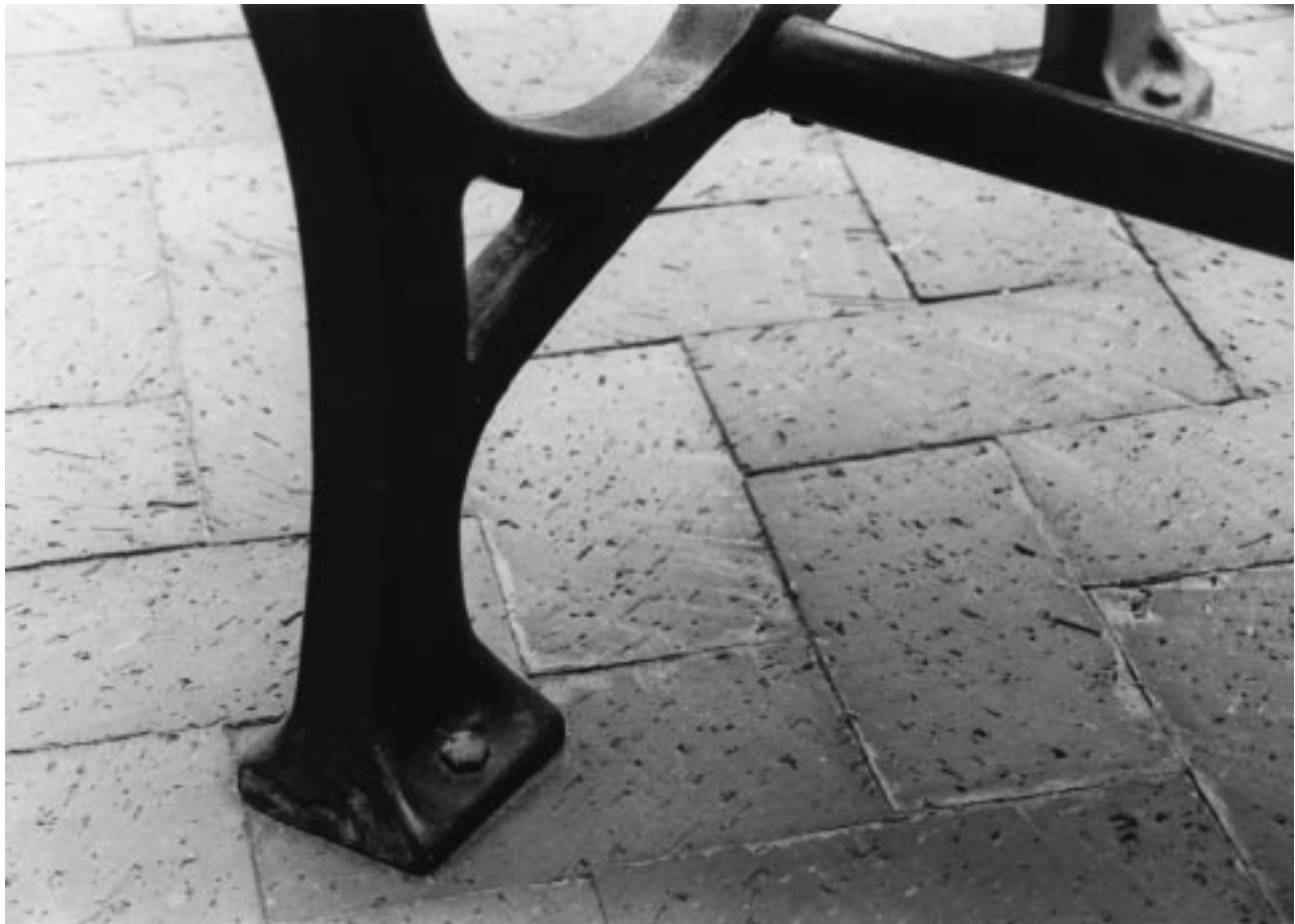
Figure 35–3 Anchoring of an amenity support post to paving using an anchor bolt placed through the paving. (Courtesy of Margaret Sauter)
