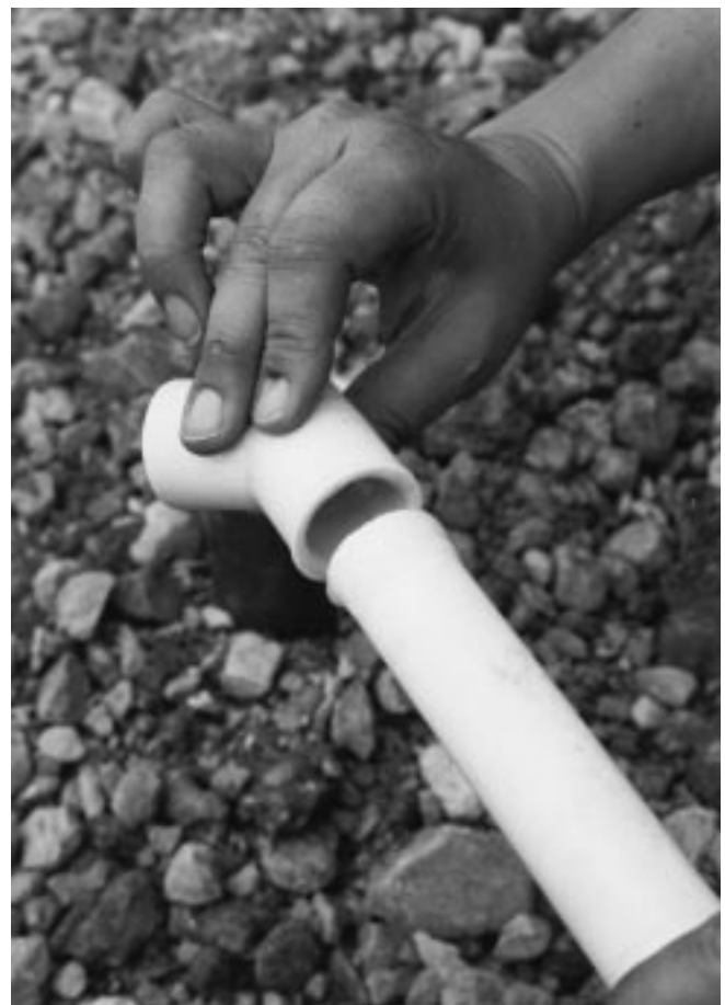
Figure 7-14 Joining PVC pipe after applying glue. Use a twisting motion to push pipe completely into fitting.
