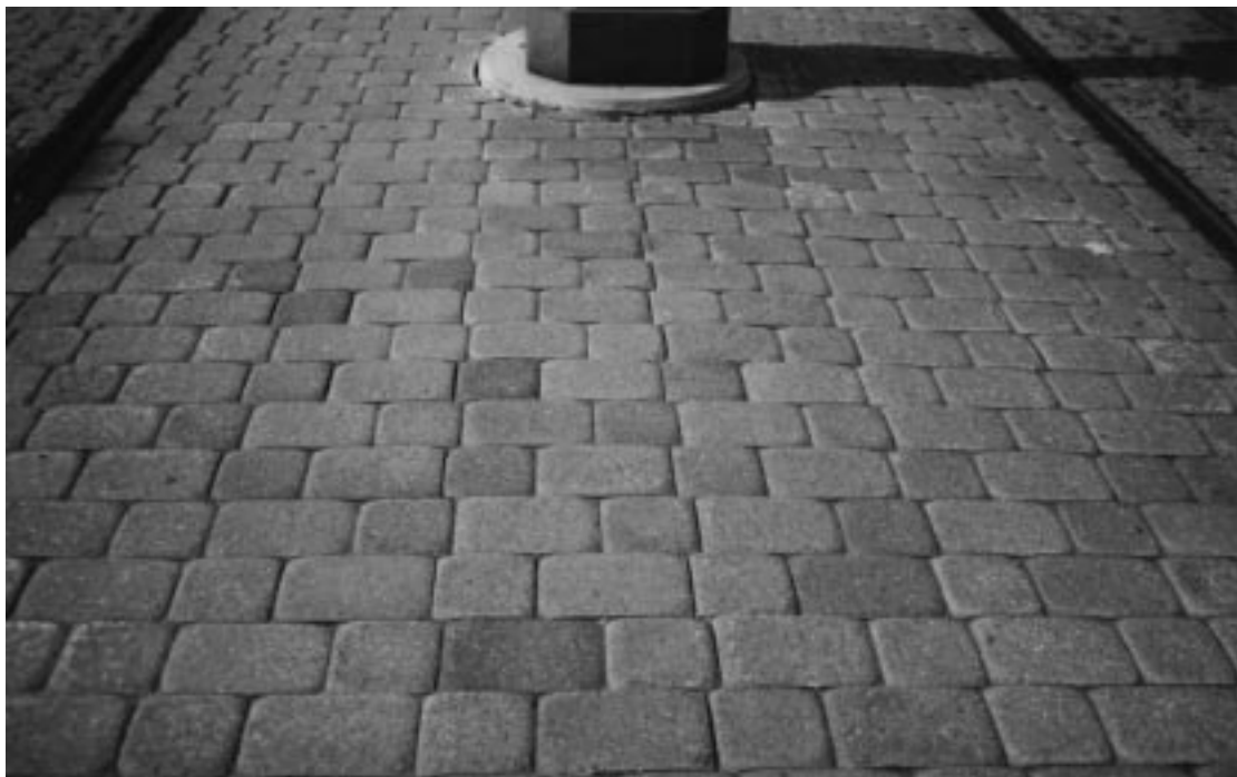
Figure 22-2 Interlocking concrete paving block is an excellent choice for both pedestrian and vehicular traffic.
