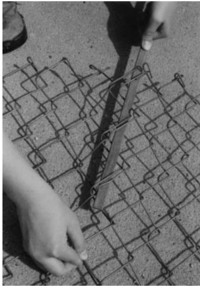
Figure 32–27 Installing stretcher bar to join sections of fabric.
