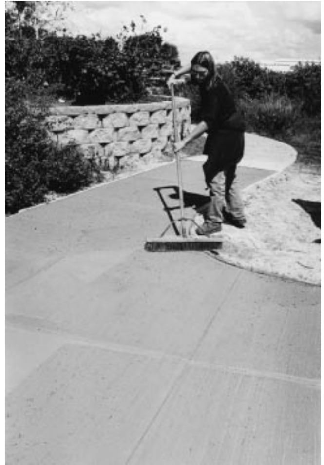
Figure 23–22 Broom finishing a concrete slab.
