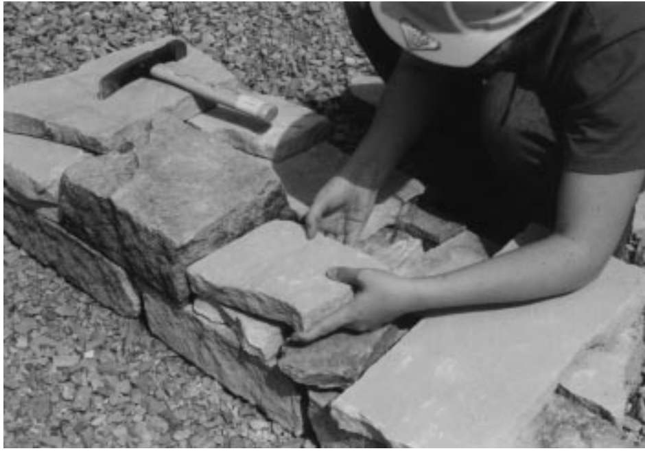
Figure 33–4 Rubble wall stone placement.
