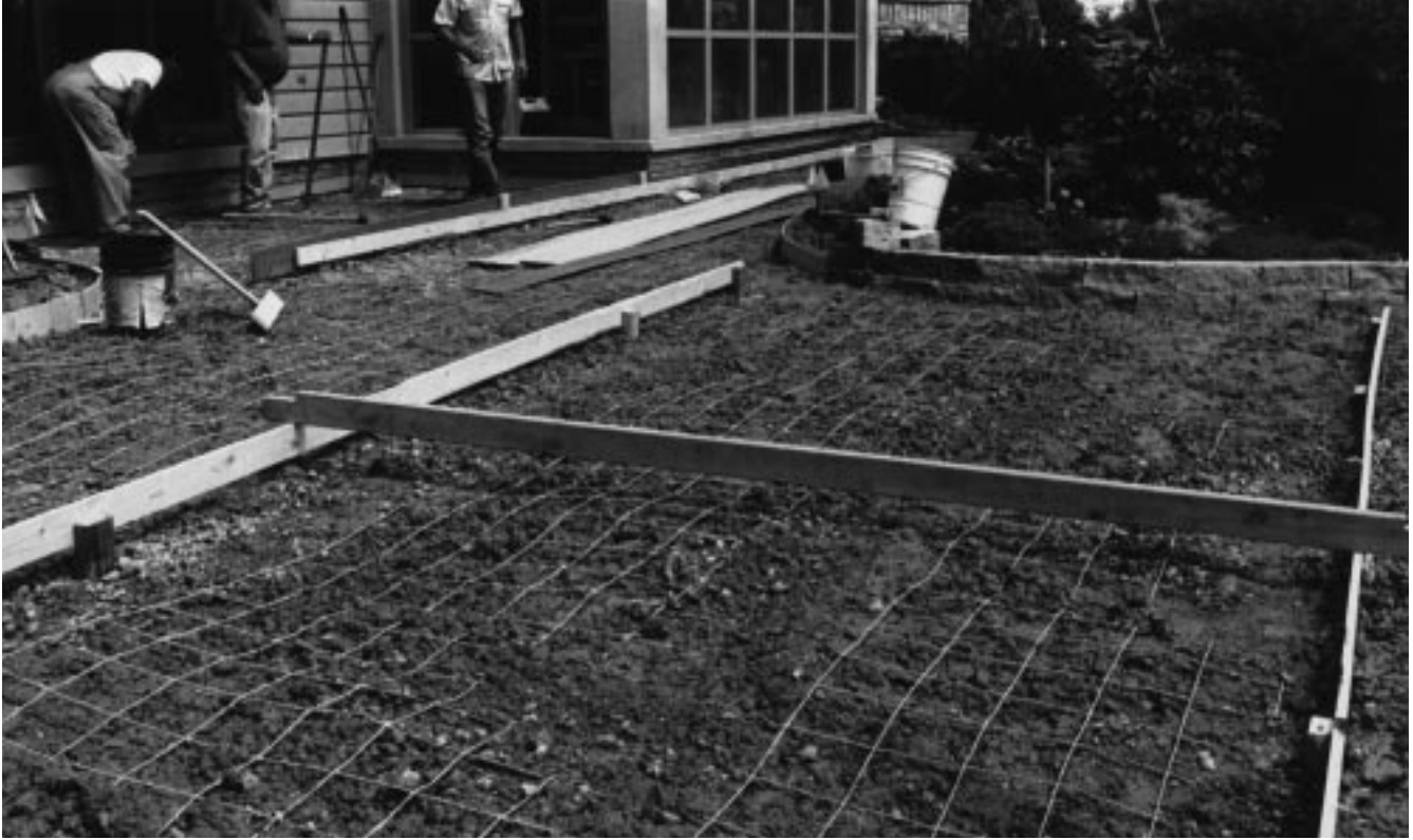
Figure 1-5 Preparing a site for landscape paving.
