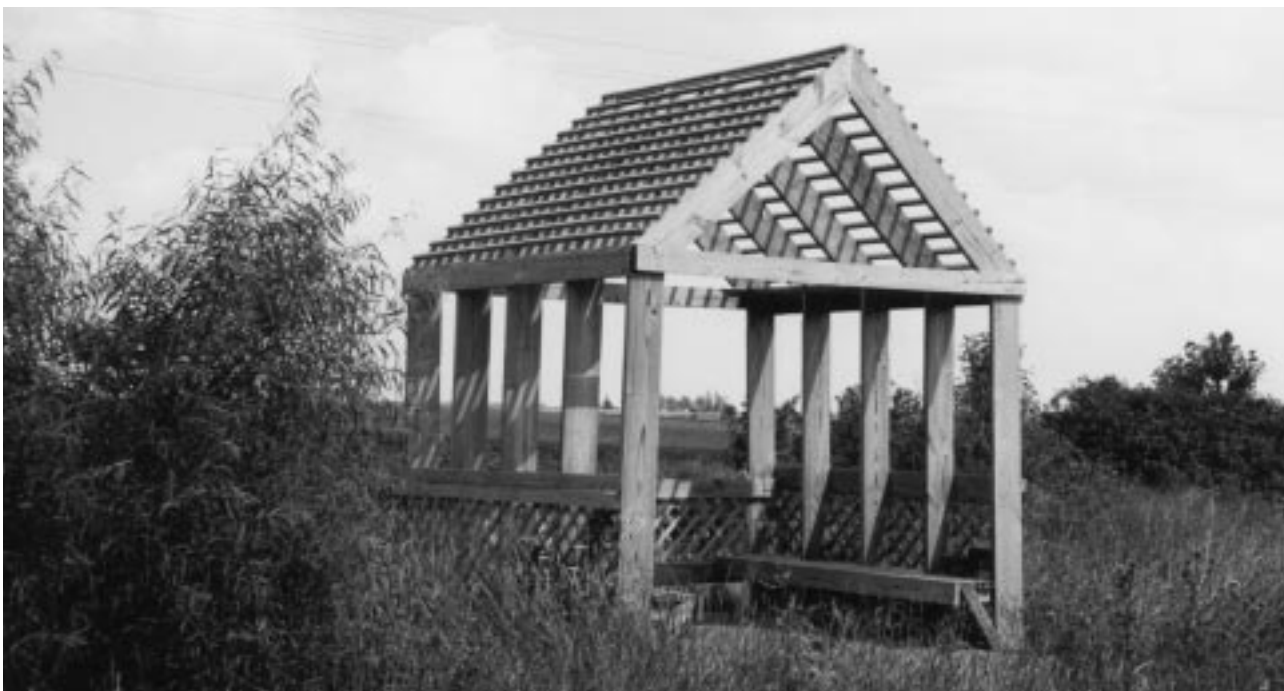
Figure 31-7 Gabled roof has a long peak and two sloped sections.
