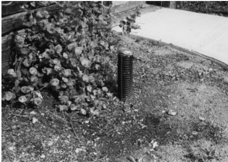
Figure 12-6 Tile riser before being trimmed for inlet installation.
