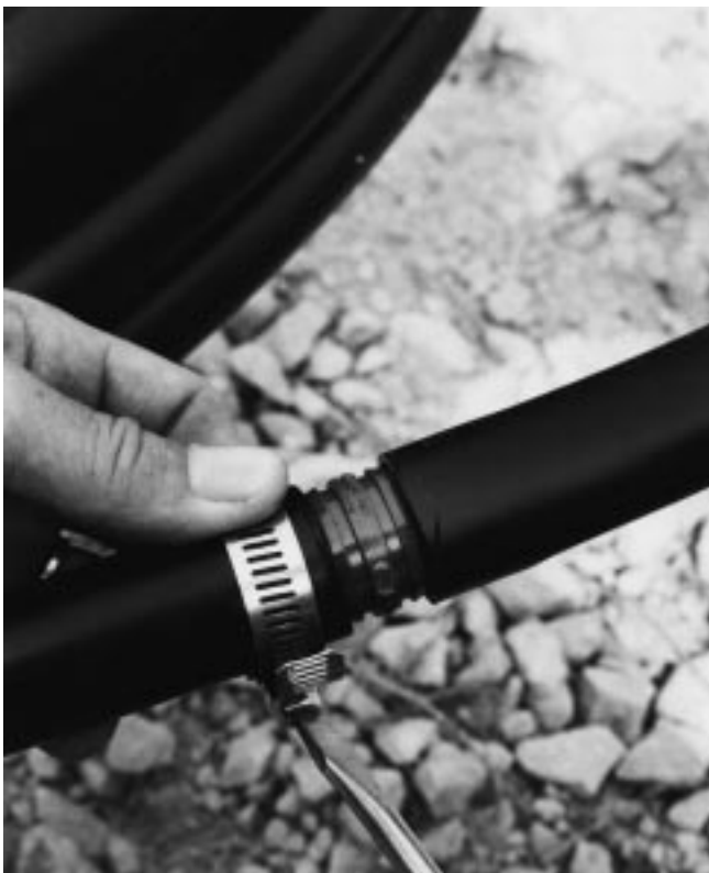
Figure 7-11 Clamping poly pipe around the fitting. Each pipe connected to a fitting should be clamped.
