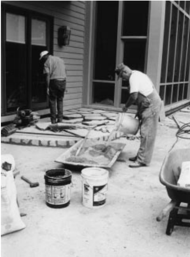
Figure 26-1 Preparing for placement of mortared limestone.
