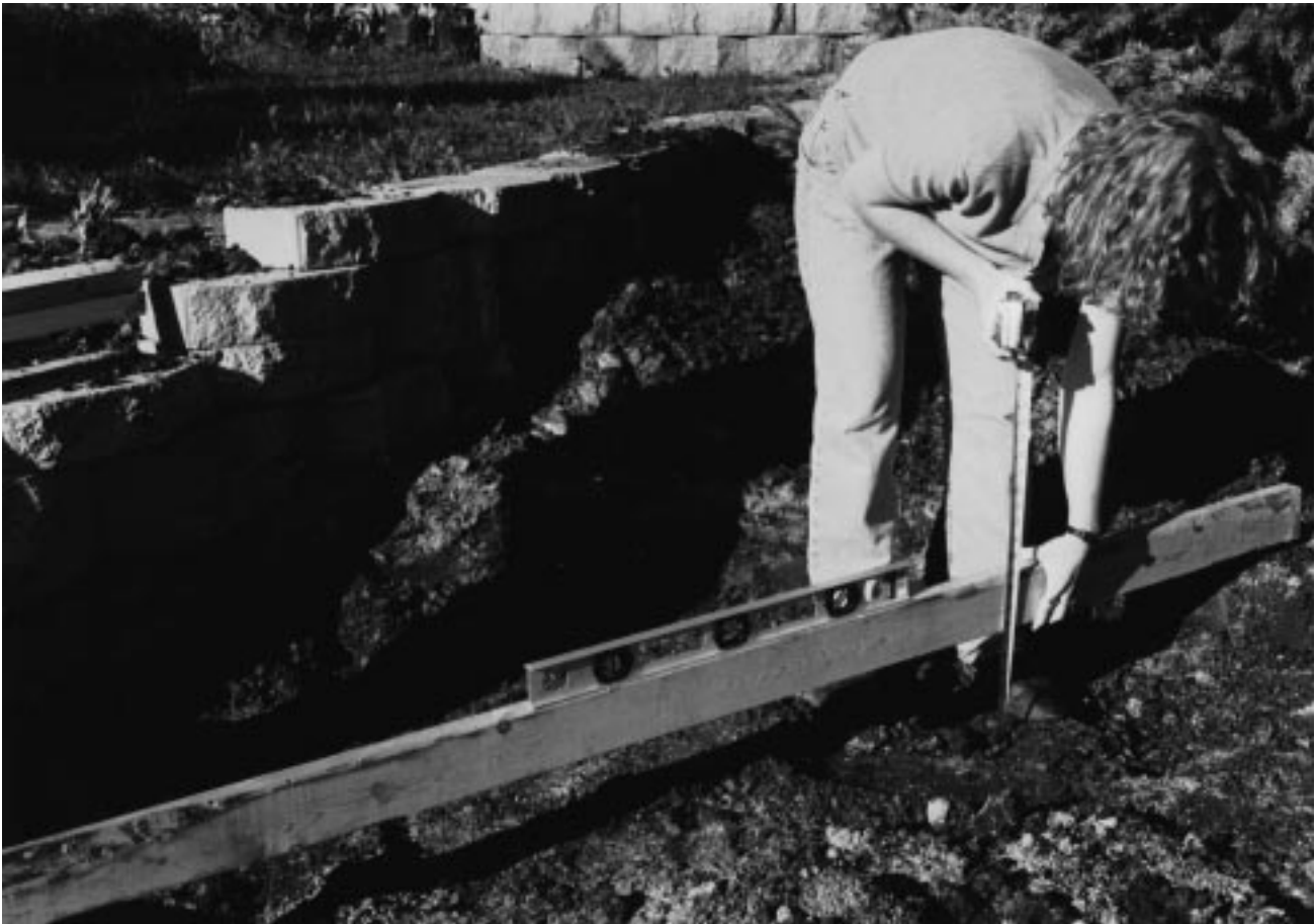
Figure 8-2 Determining slope by holding a board level and resting on the high point and measuring from the bottom of the board to the low point.
