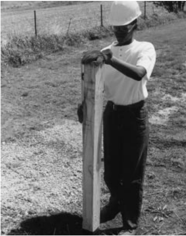
Figure 32-14 Rail/stringer fence post installation.
