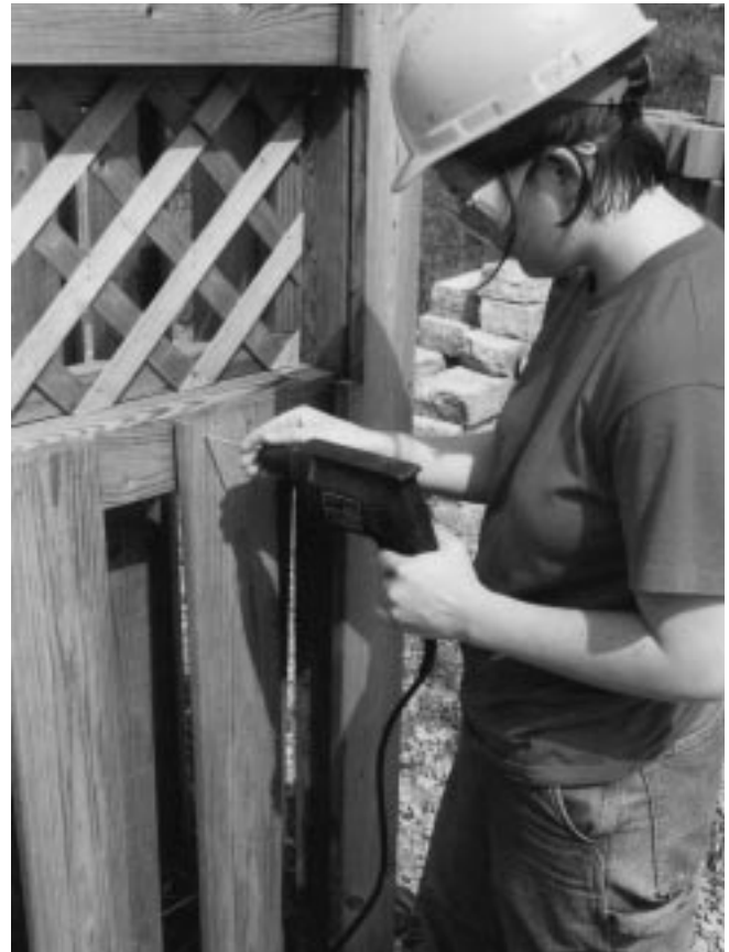
Figure 32–18 Fencing vertical surfacing attachment.
