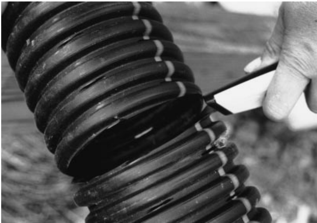
Figure 7-6 Cutting corrugated plastic drain pipe with carpet knife.
