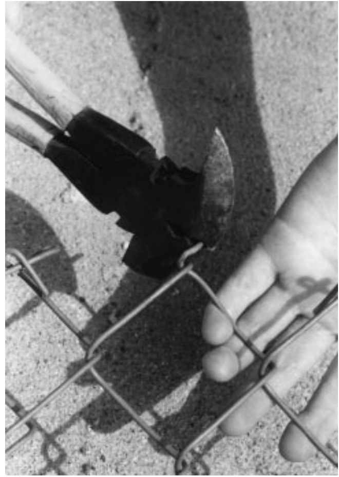
Figure 32-25 Disconnecting top link.
