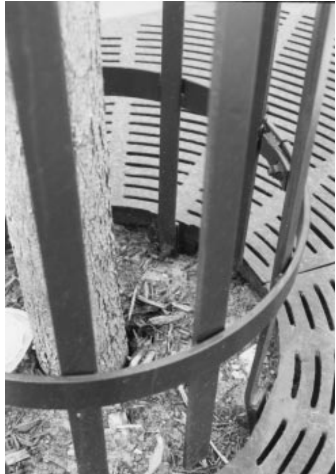
Figure 36-17 Tree grate sections are bolted together. Sections of guards are placed around the tree and bolted together, then bolted to the tree grate.
