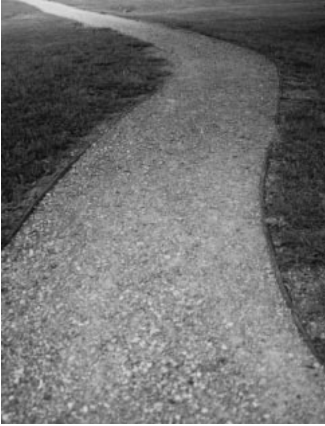
Figure 22–6 Granular paving provides functional walkways. (Courtesy of Margaret Sauter)
