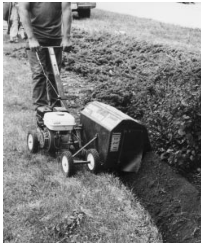
Figure 36-5 Excavation for edging using an edging machine.
