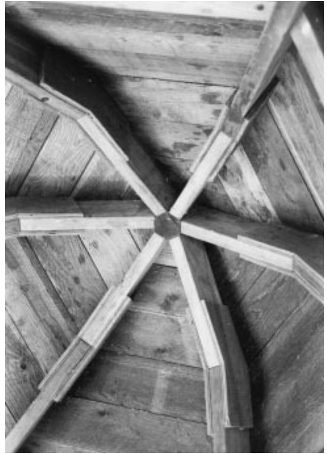
Figure 31-10 Closeup showing six rafters connected to hexagonal hub.
