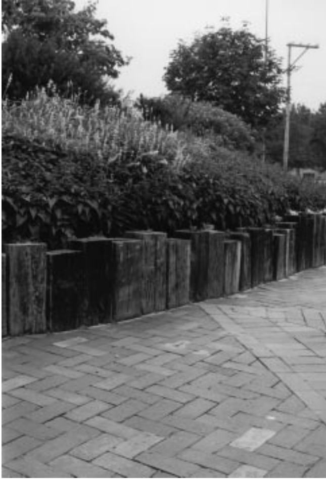
Figure 17-1 Tie retaining wall with all ties buried vertically. Elevations of tops are staggered for interest.
