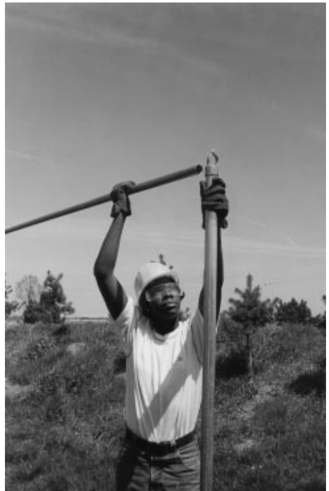
Figure 32–23 Chain link fencing top rail installation.
