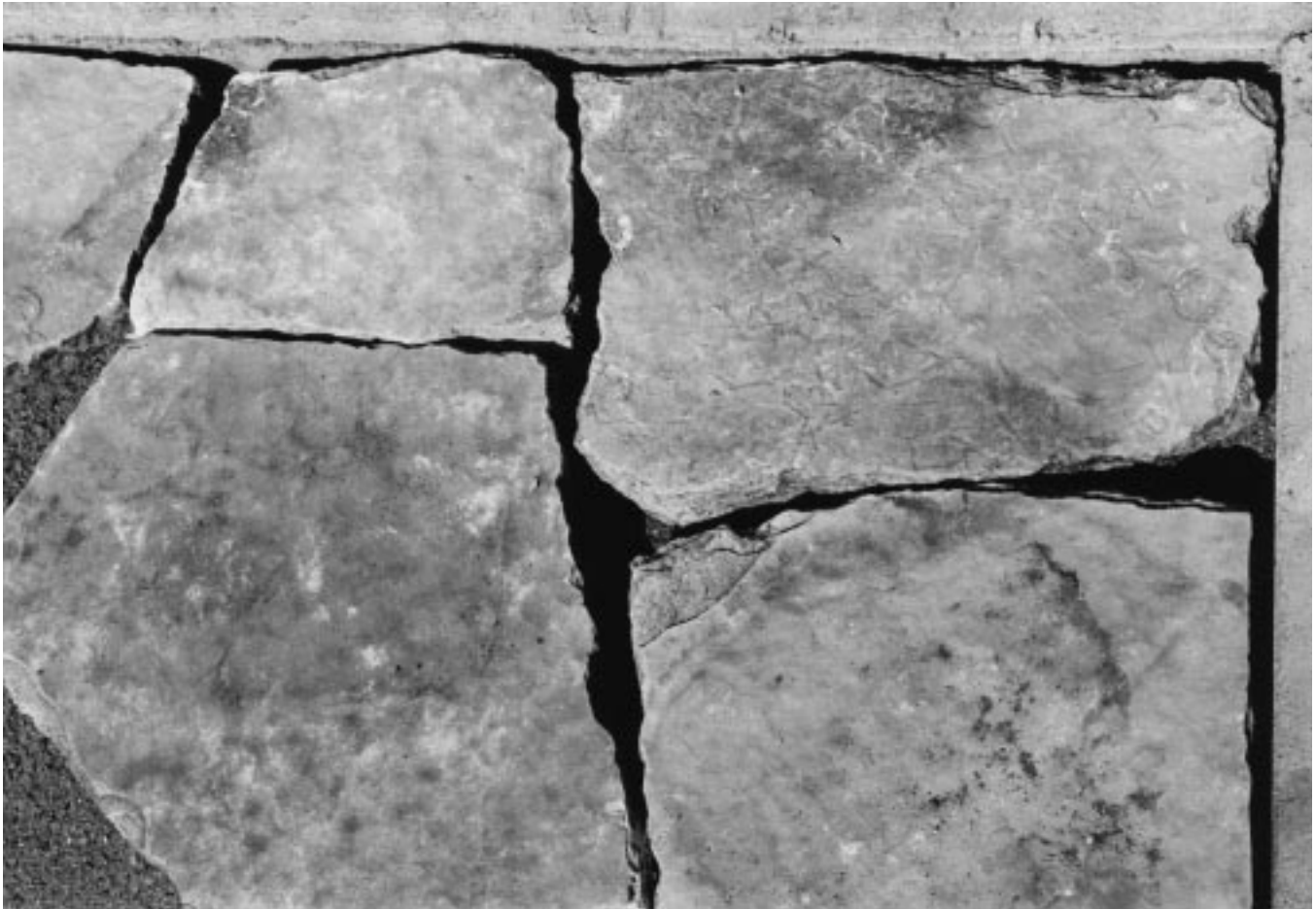
Figure 25-4 Placement of dry-laid stone in pattern.
