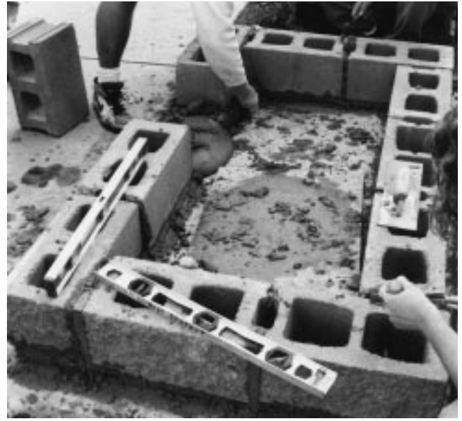
Figure 33–6 First course laying and leveling.
