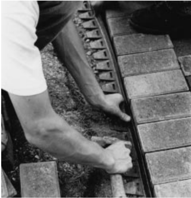
Figure 22–10 Installation of plastic edging after placement of pavers.
