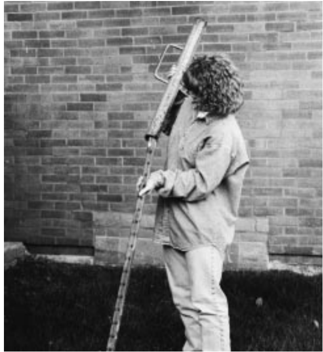
Figure 7–5 Preparing to drive a fence post by leaning the post at an angle and inserting post into driver. Return post and driver to plumb and being driving.
