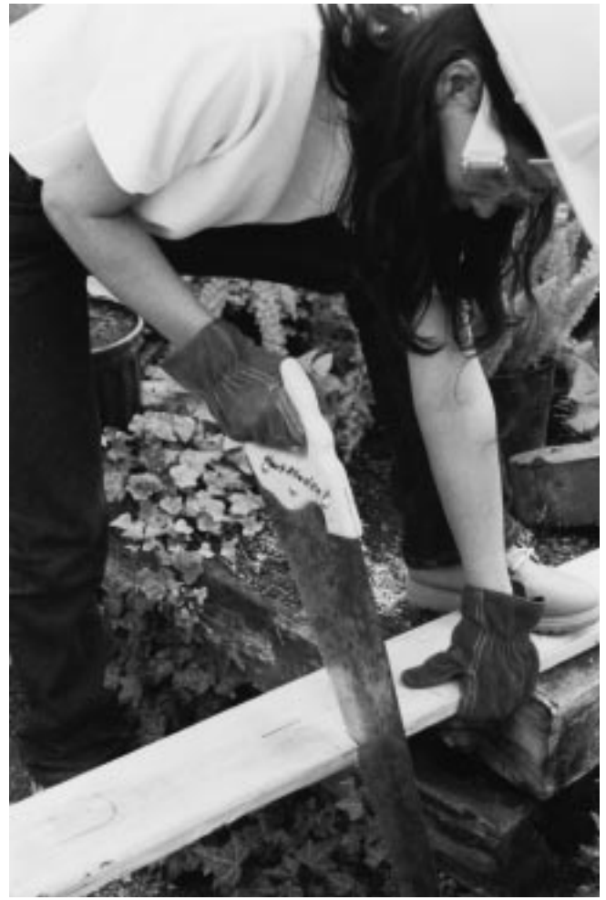
7-24 Proper hand-sawing technique.
