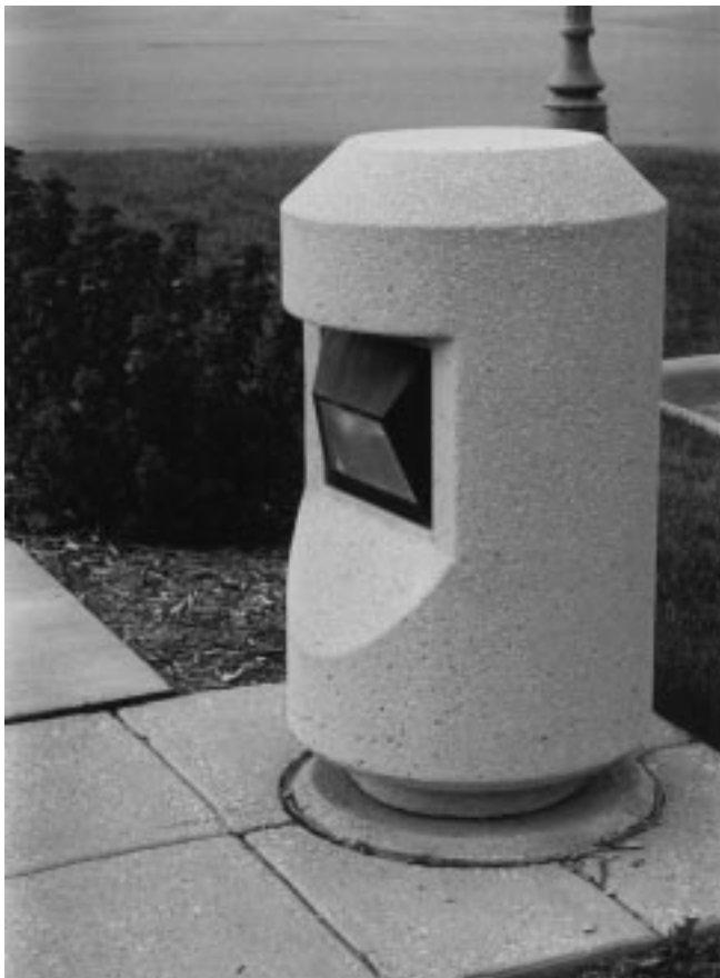
Figure 35–4 Anchoring of an amenity support on a footing poured separately from the concrete walkway.
