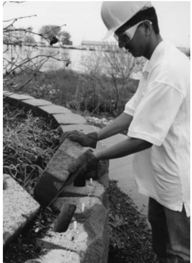
Figure 18–7 Cap installation for precast segmental unit walls.
