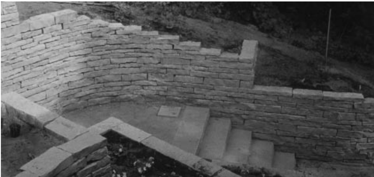
Figure 19–6 Rounded corners with dry-laid limestone walls. Shorter pieces are used to turn tighter corners. (Courtesy of Paul Dykstra, Iowa City Landscaping)
