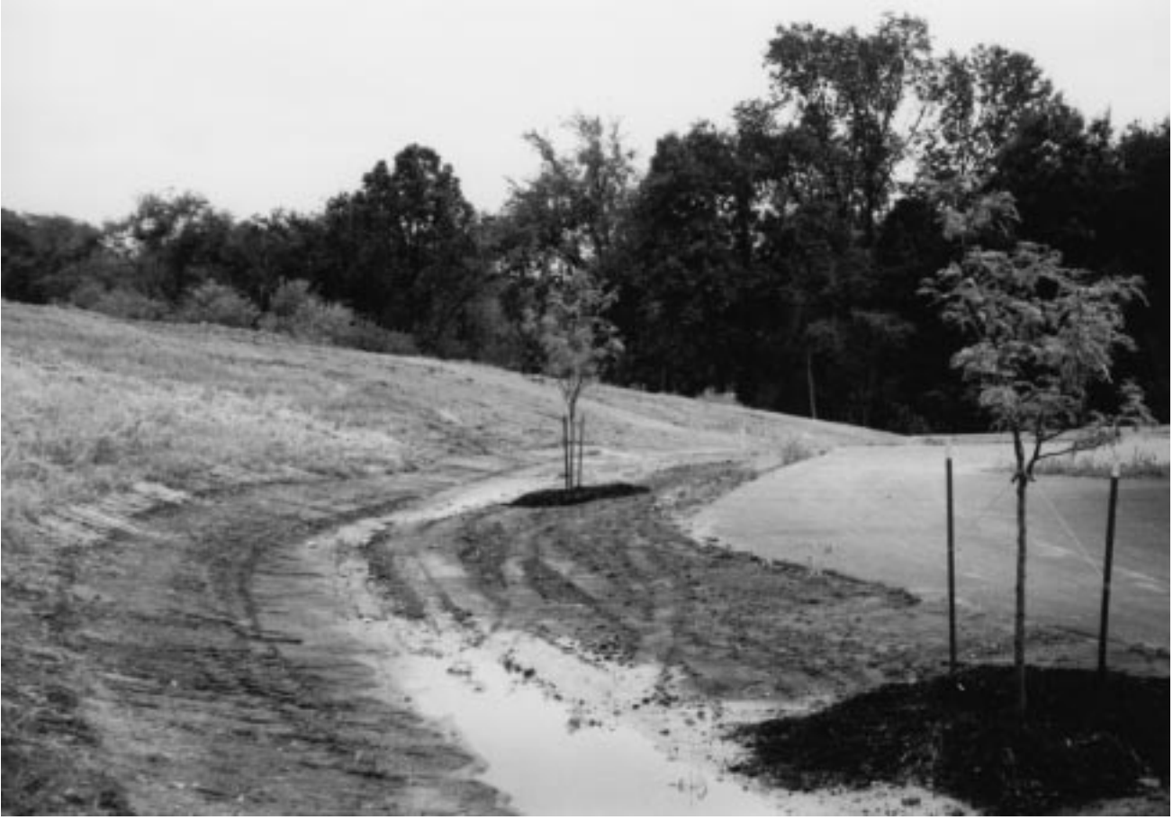
Figure 12-1 Drainage swale constructed to direct runoff away from improvements.
