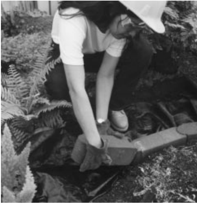
Figure 36-11 Placement of precast concrete edging. This edging may be placed in straight or curved alignments.
