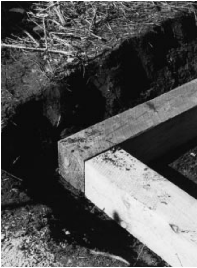
Figure 17-3 First course installation for stacked timber wall.
