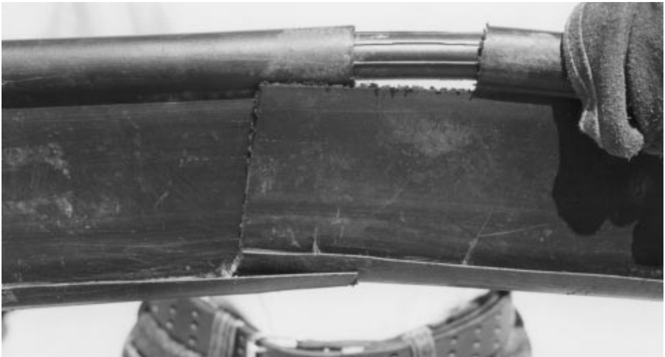
Figure 36-7 Joining pieces of plastic edging using tubing joiners supplied with edging kits. Notching the edge improves the connection.
