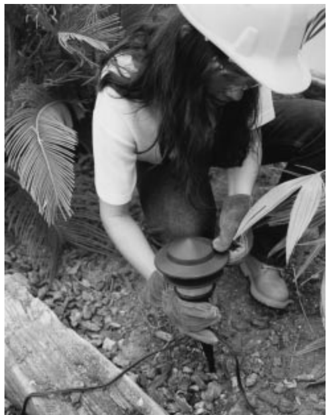
Figure 14-8 Gently pushing fixture into the ground.
