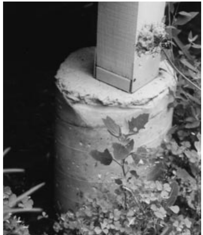
Figure 29-2 Galvanized post anchor placed in concrete footing.
