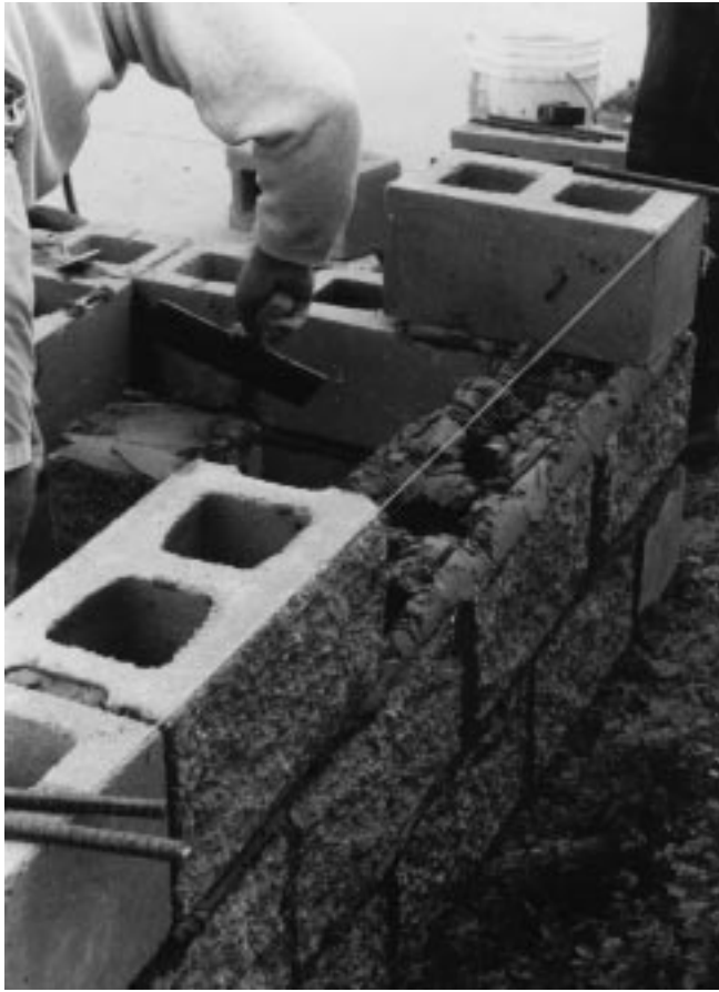
Figure 33-7 Masonry courses showing stringline used to keep blocks aligned.
