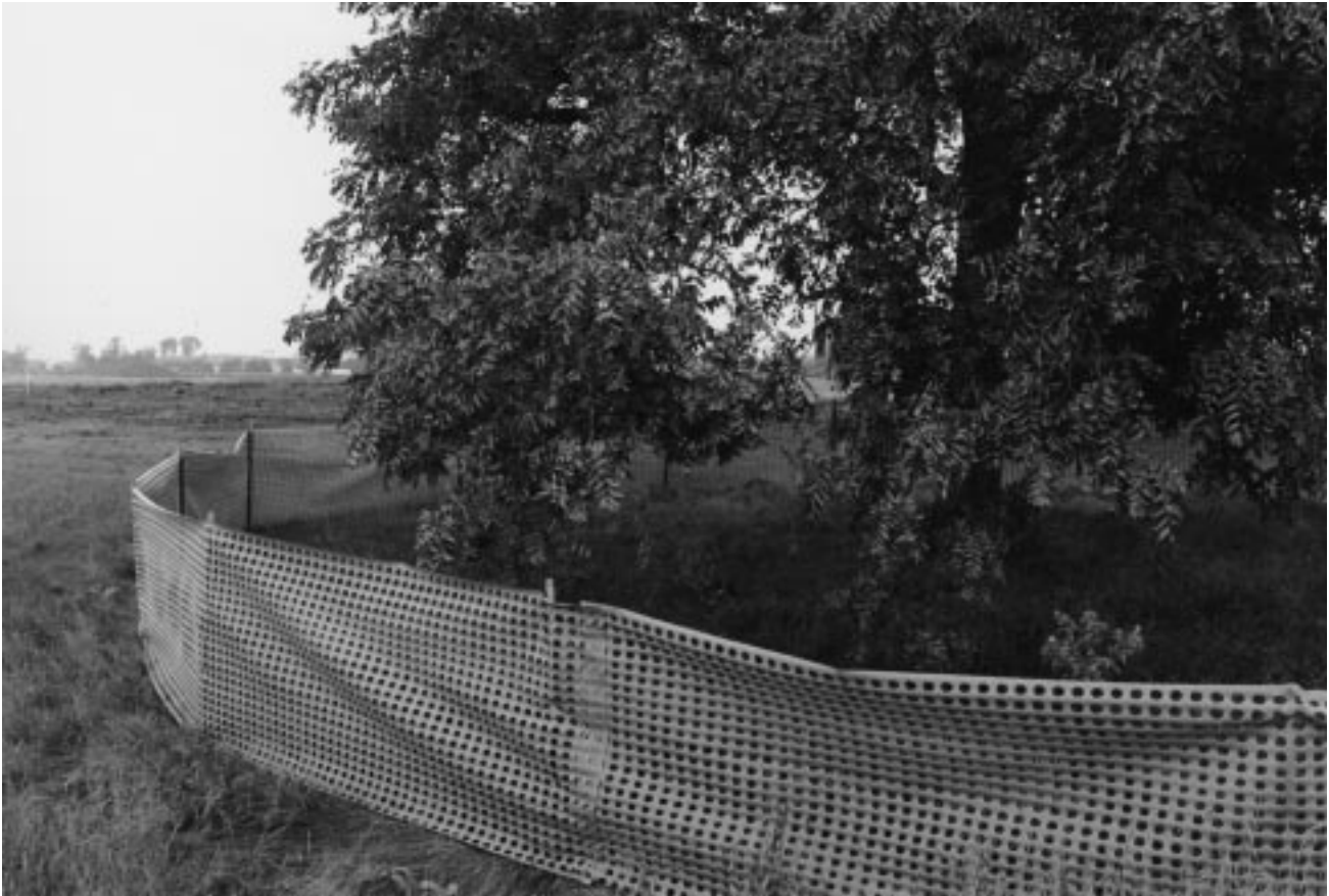
Figure 9–2 Fencing placed at drip line of a tree to protect the root zone.
