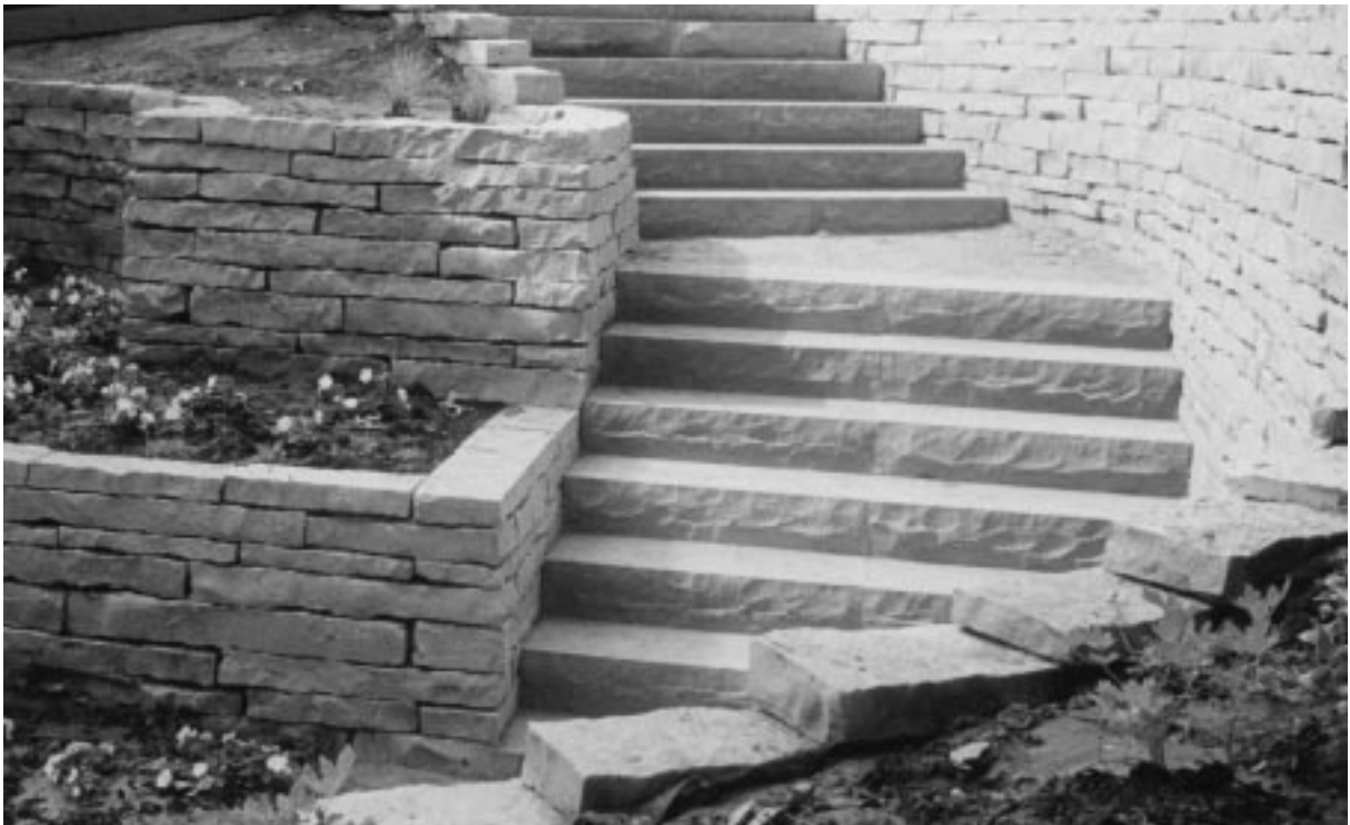
Figure 21–13 Completed butt stairs with precast stone steps. (Courtesy of Paul Dykstra, Iowa City Landscaping)
