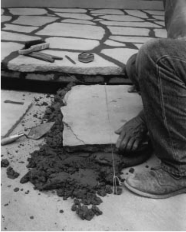
Figure 26-4 Placement of stone using stringline to maintain proper elevation.
