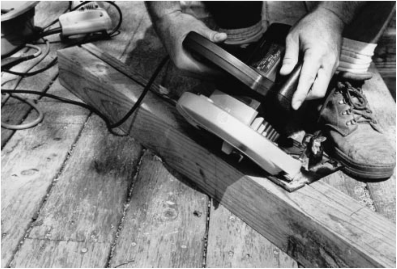
7-22 Bevel/rip cut along length of dimensioned lumber.
