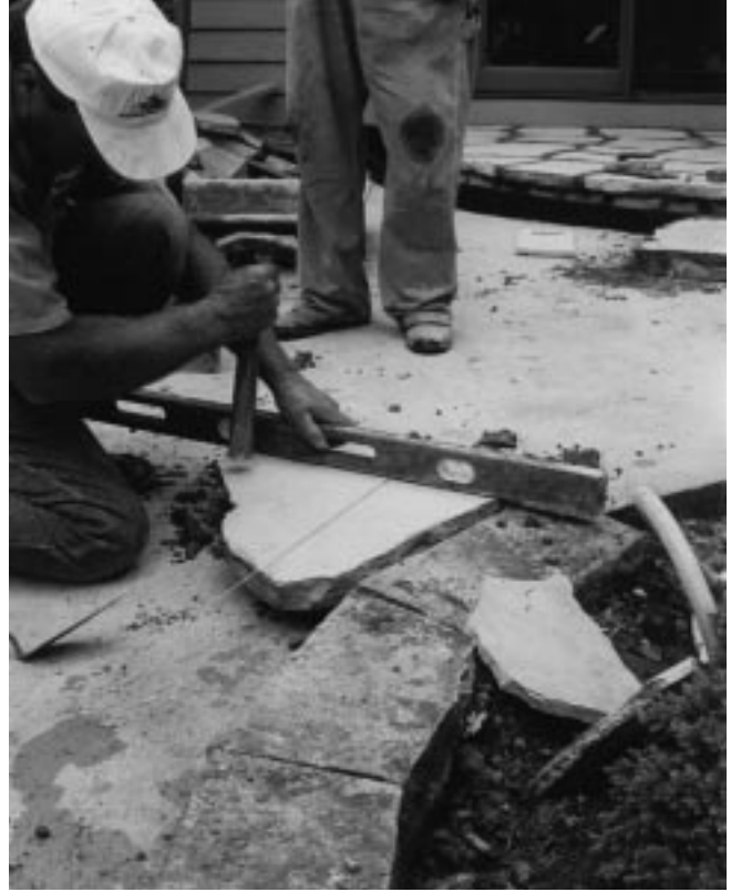
Figure 26-5 Leveling individual stones when placed.
