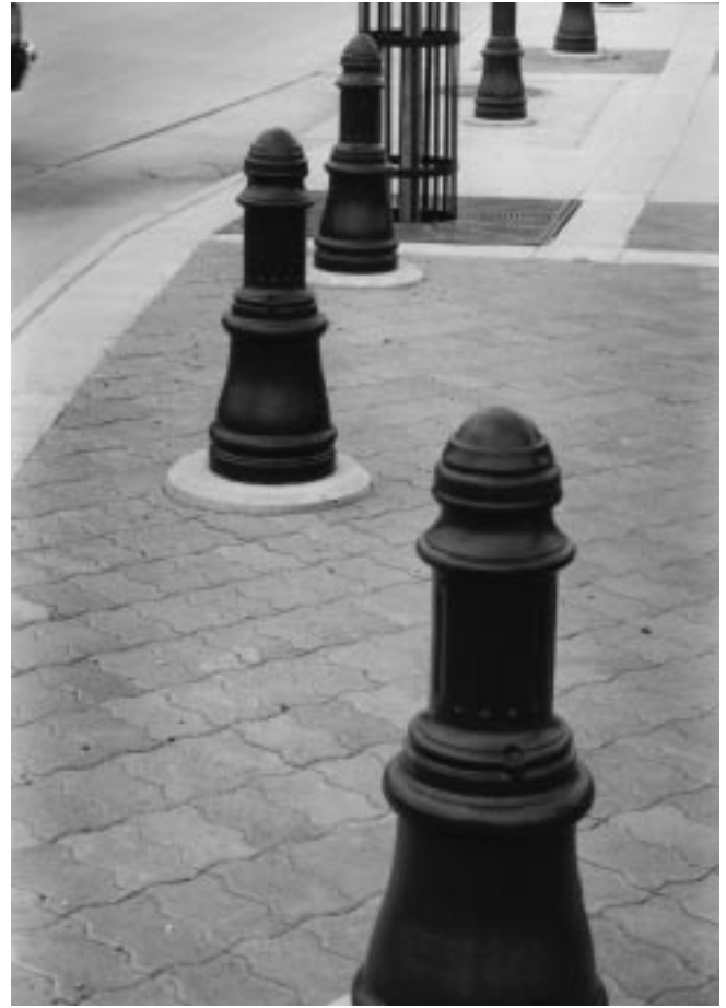
Figure 35-2 Bollards used to separate traffic from pedestrians.
