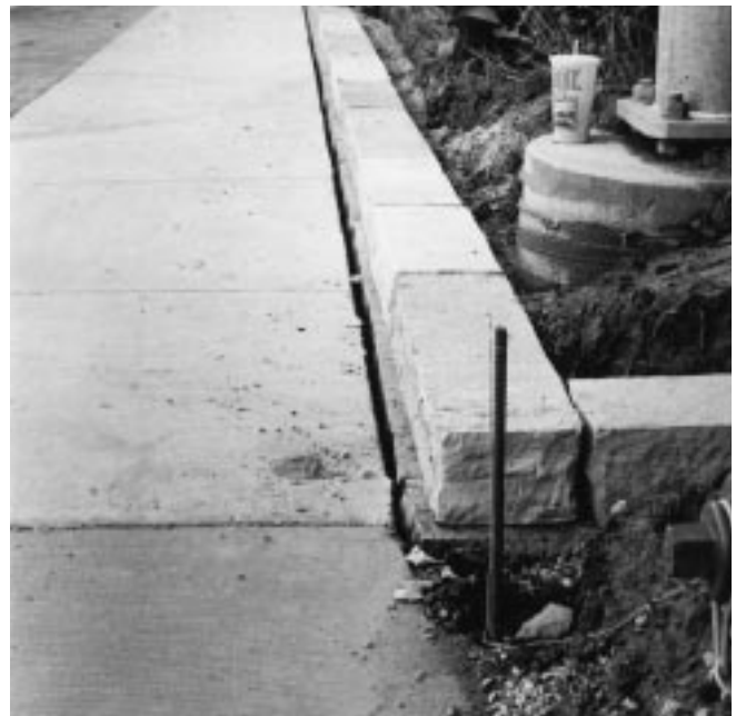
Figure 19-2 Stone wall first course installation.
