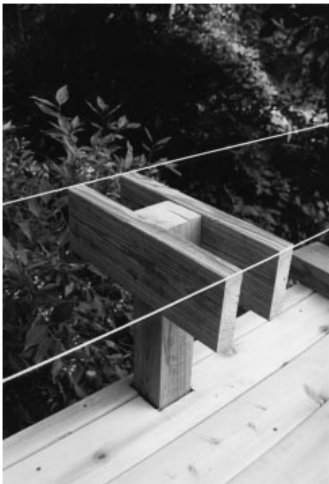
Figure 30-14 Seating framing with grab beams.
