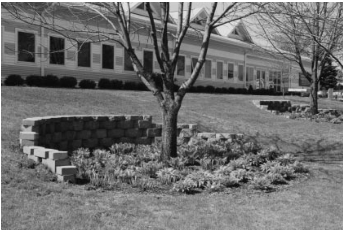
Figure 9-3 Tree wells installed to protect existing tree root zone from fill.
