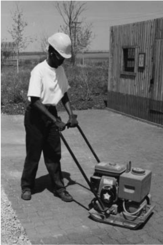
Figure 24–8 Seating pavers using plate compactor.
