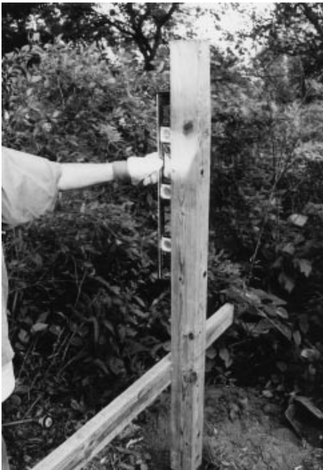
Figure 29–5 Setting and leveling posts for deck construction.
