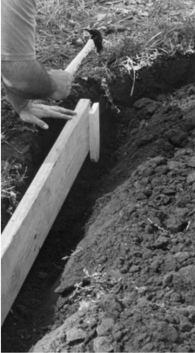
Figure 36–14 Staking for wood edging. Place end stakes and adjust for level. Joints should overlap a single stake.
