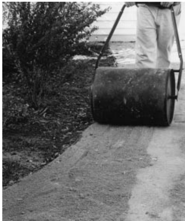
Figure 27-3 Leveling and finishing granular paving installation.
