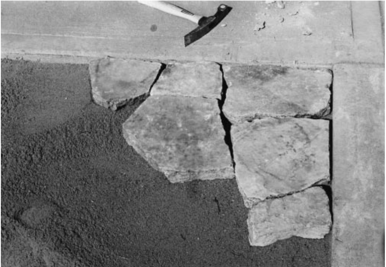
Figure 25-2 Proper placement of dry-laid stone. Note that surfaces are flush with surrounding stone and each stone makes contact with adjacent material.
