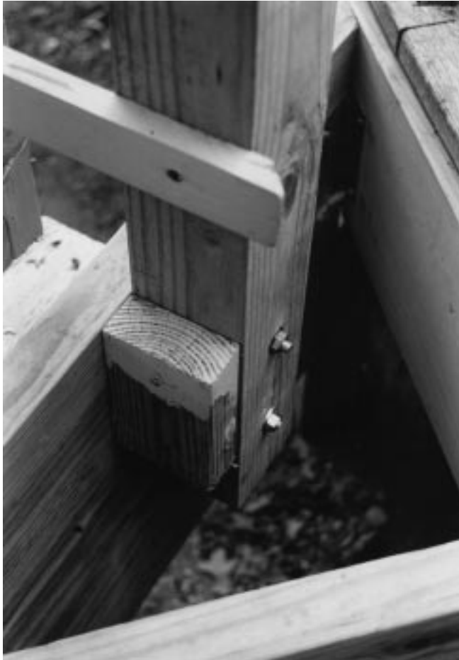
Figure 29–16 Cleat on which decking material will be fastened.
