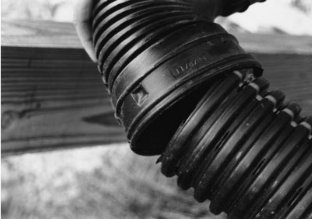
Figure 7-7 Joining corrugated plastic drain pipe to a premanufactured elbow fitting. Pipe “snaps” into fitting.
