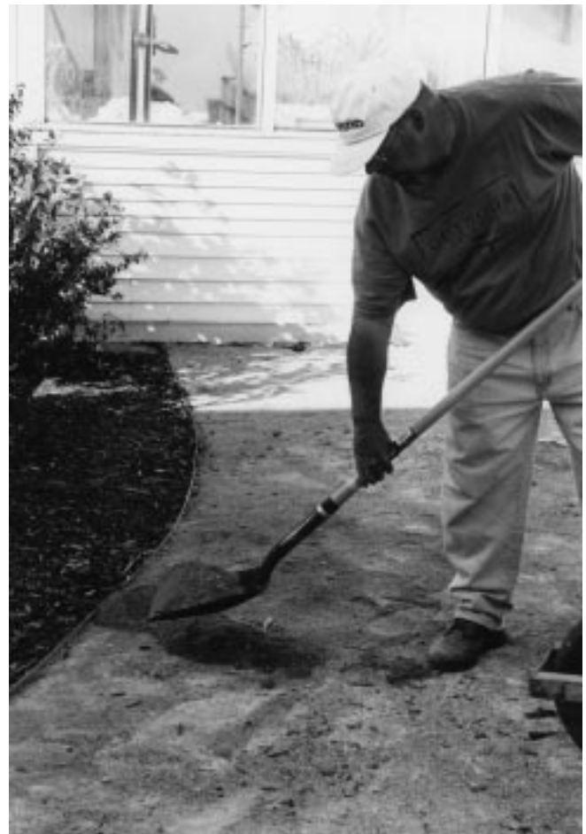
Figure 27–2 Placement of granular paving material.
