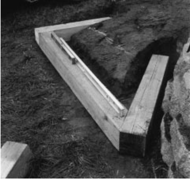
Figure 21-14 Building the base step of a freestanding wood timber installation.
