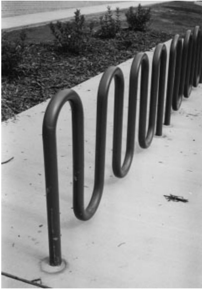
Figure 35-1 Bike rack anchored in a concrete slab.
