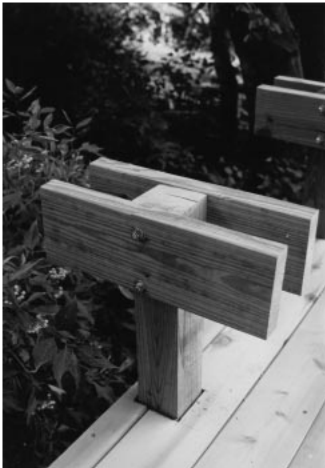
Figure 29-10 Grab beam connections used for seating framing.
