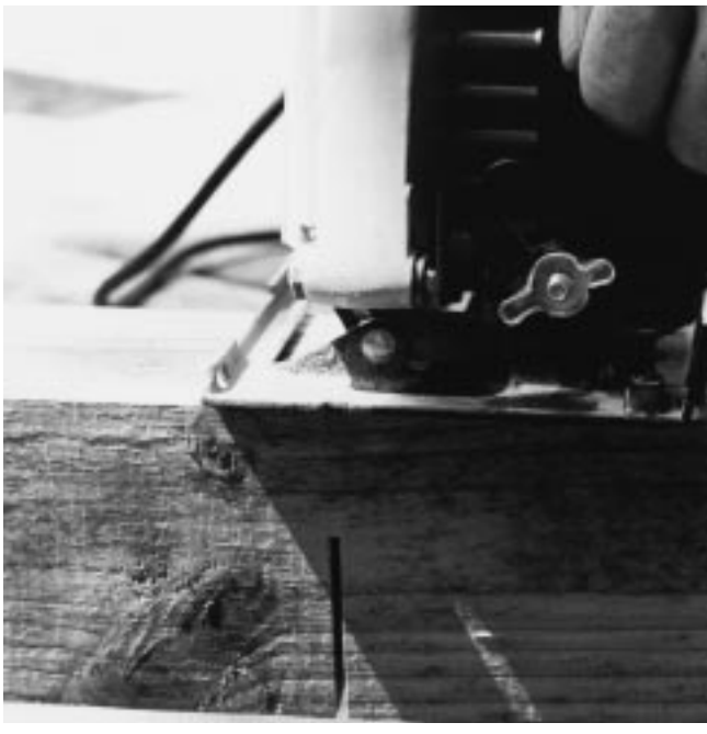
7-21 Cutting large-dimensioned lumber with two cuts.
