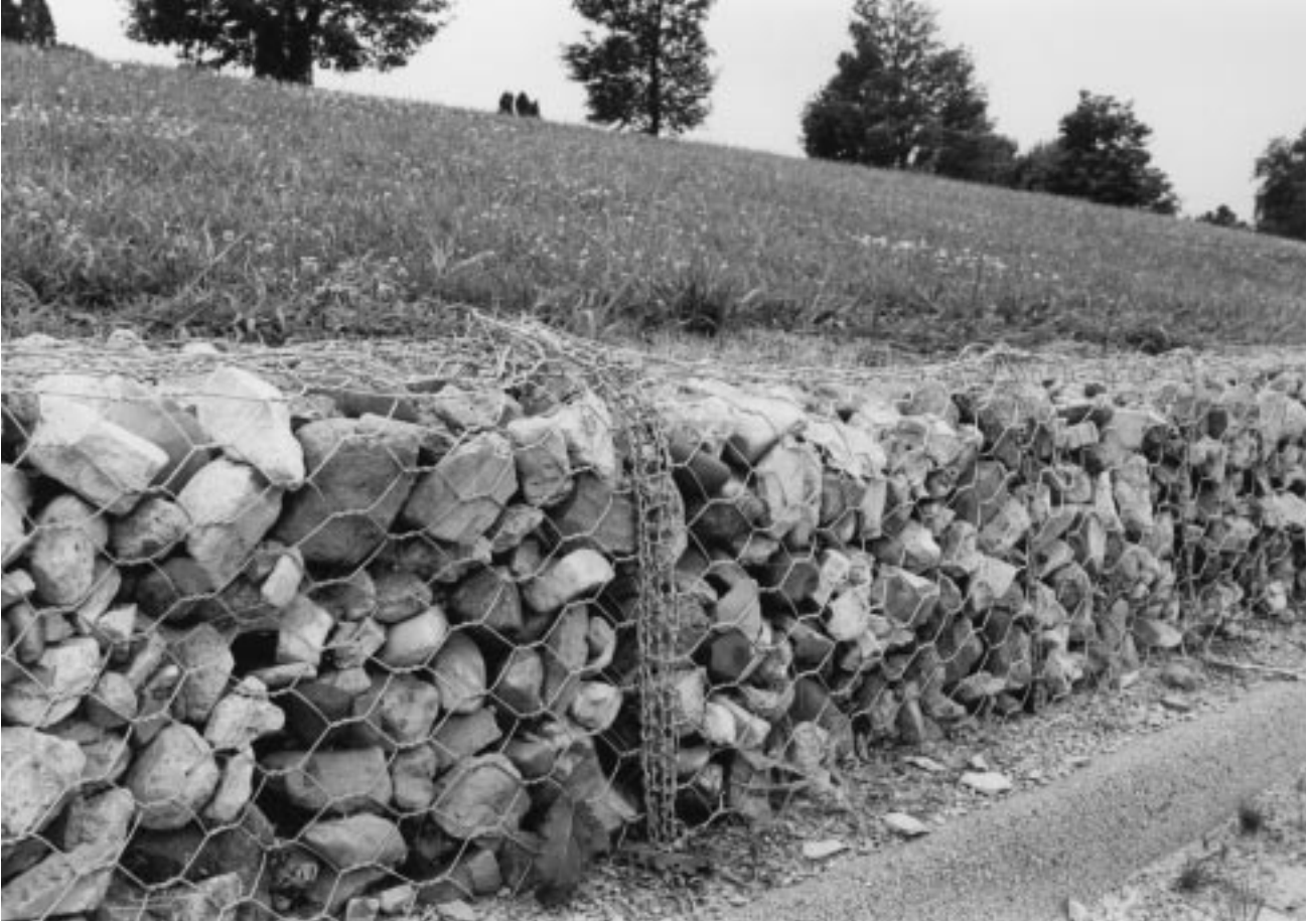
Figure 16-4 Gabion retaining wall one course high.
