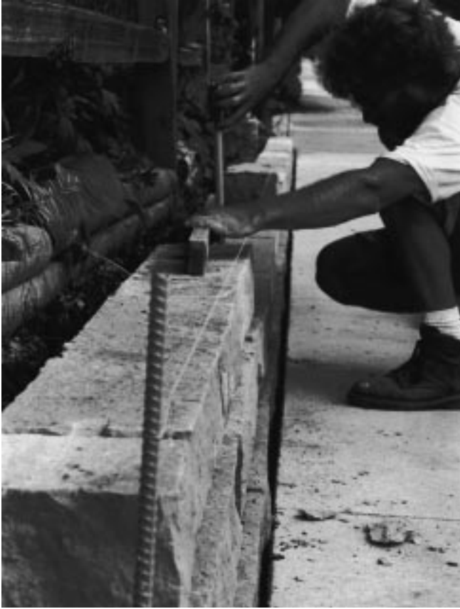
Figure 1–4 Building a dry-laid, limestone, landscaping retaining wall.
