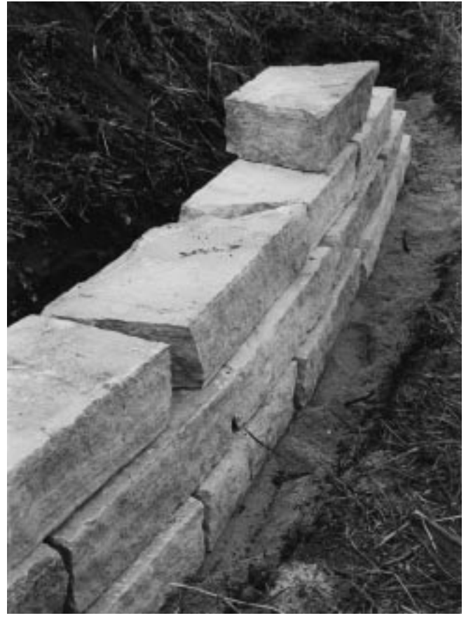
Figure 19-4 Placement of dry-laid stone wall material for a convex curve.
