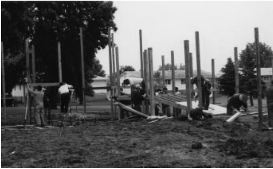
Figure 35-6 Layout of a custom-built play structure. (Courtesy of Janice Carter)
