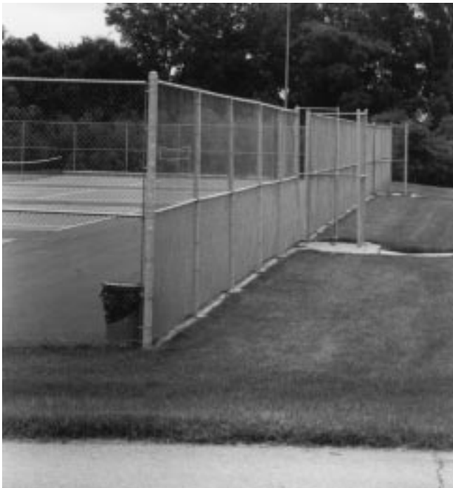
Figure 32–3 Chain link fencing.
