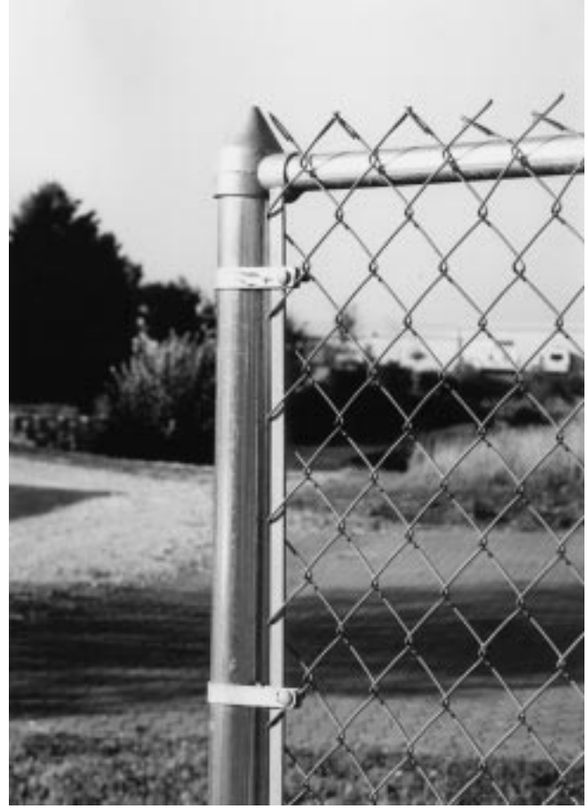
Figure 32-29 Chain link fencing hardware, showing top rail, post cap, stretcher bar, and connector clamps.
