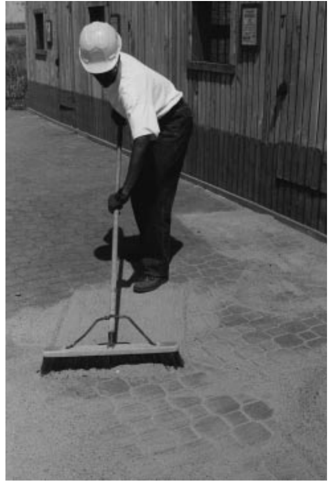
Figure 24–9 Sweeping dry sand into paver joints.
