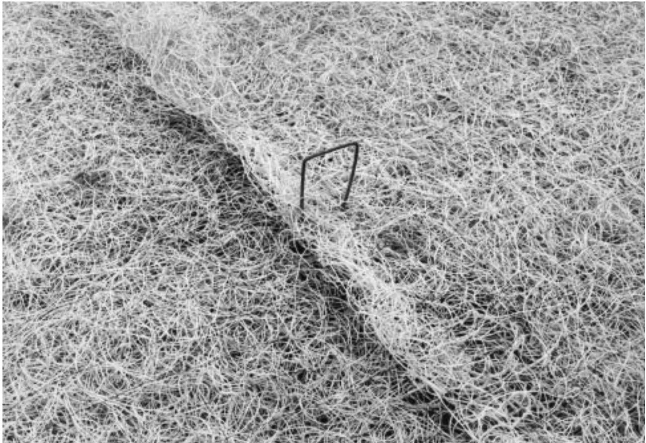
Figure 13–3 Anchoring erosion mat using metal staples.
