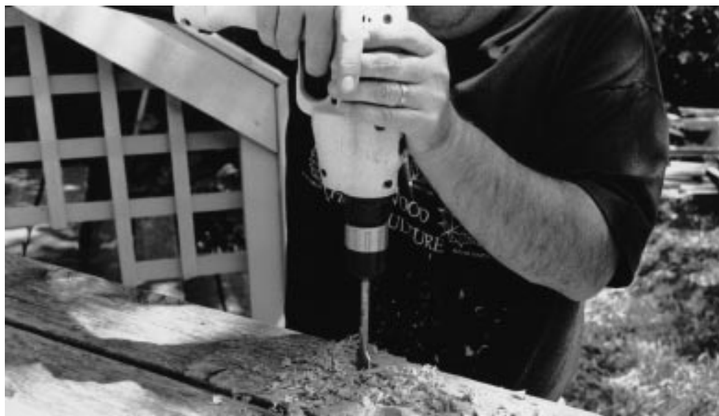
7-25 Drilling holes using a cordless drill.
