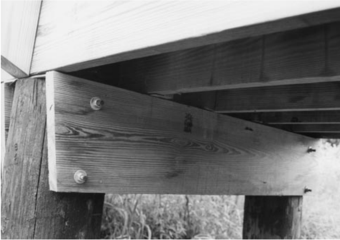
Figure 34–20 Deck framing for wood bridge.
