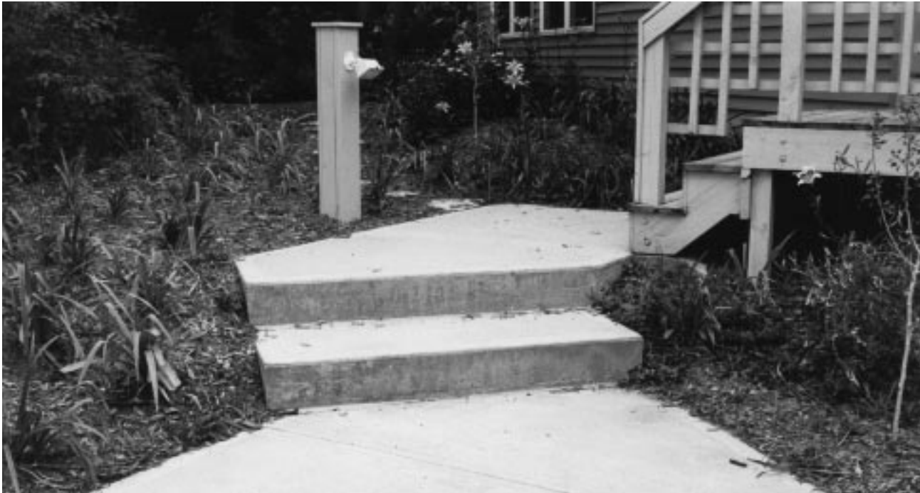
Figure 21–3 Freestanding concrete steps were formed and poured as part of this entry construction.
