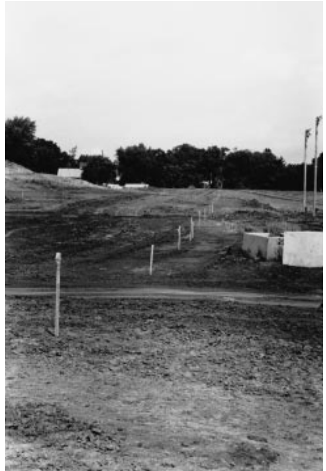
Figure 9-1 Baseline reference markings for project layout.
