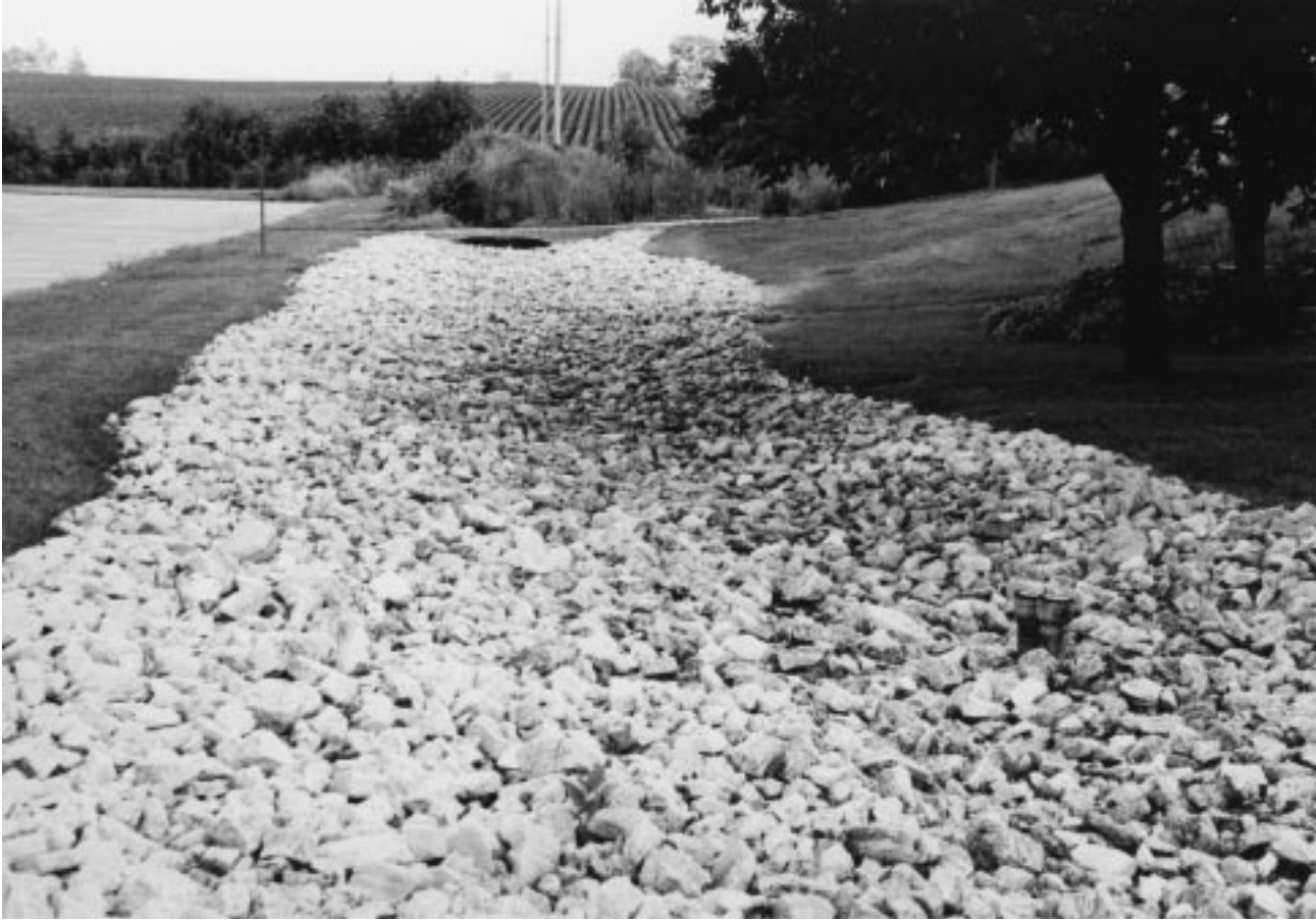
Figure 13–5 Swale protected with 4–8 inch rip-rap.
