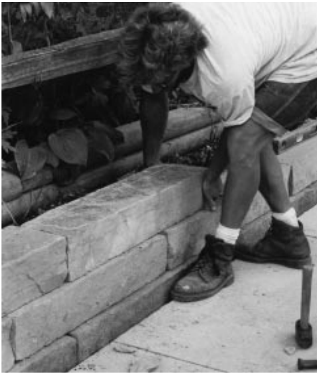
Figure 16-3 Dry-laid stone retaining wall.
