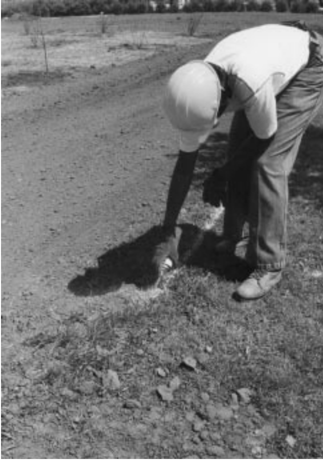
Figure 36-1 Layout of edging using marking paint.
