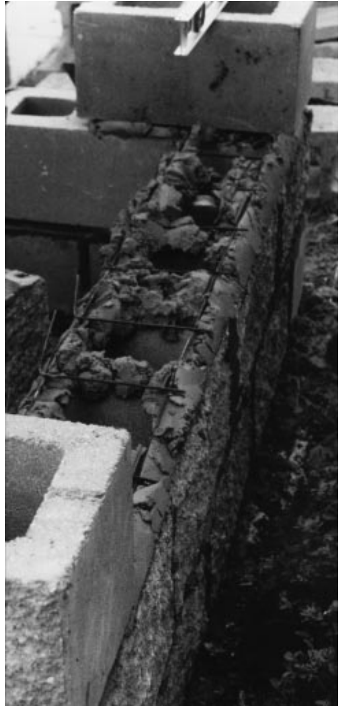
Figure 33-8 Horizontal steel reinforcement embedded in mortar.
