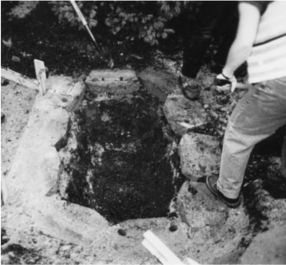
Figure 34–5 Flexible liner pool excavation.
