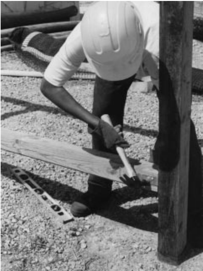
Figure 32–17 Fencing stringer attachment for vertical surfacing.
