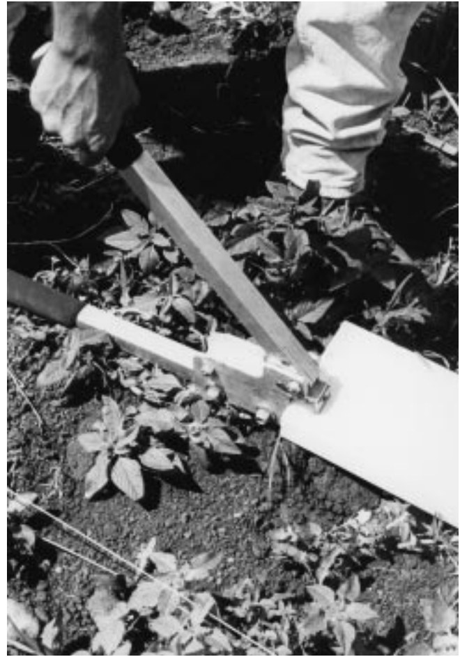
Figure 32-33 Crimping vinyl fence rail with crimping tool.
