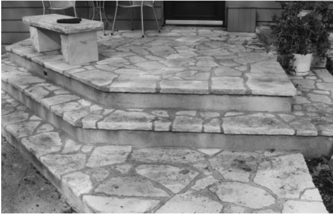
Figure 22–5 Mortared stone provides a rich, stable stone paving.
