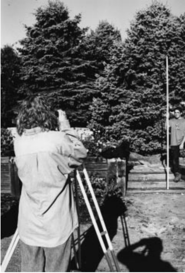
Figure 1–2 Using a surveyor’s transit to stake grades at a landscape project.
