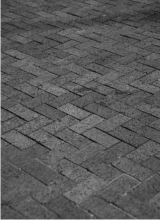
Figure 22-3 Brick paving provides rich colors and patterns.
