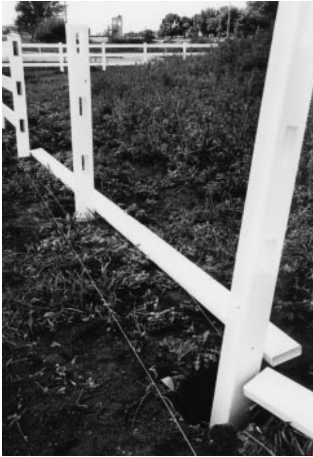
Figure 32-32 Vinyl fencing post installation.
