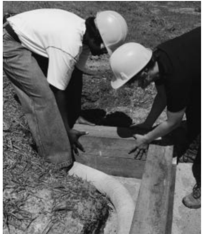
Figure 17-4 Placement of subsequent courses for timber wall.
