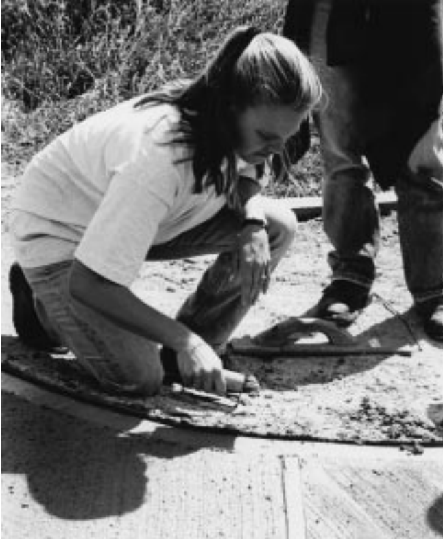
Figure 23–24 Edging a concrete slab.
