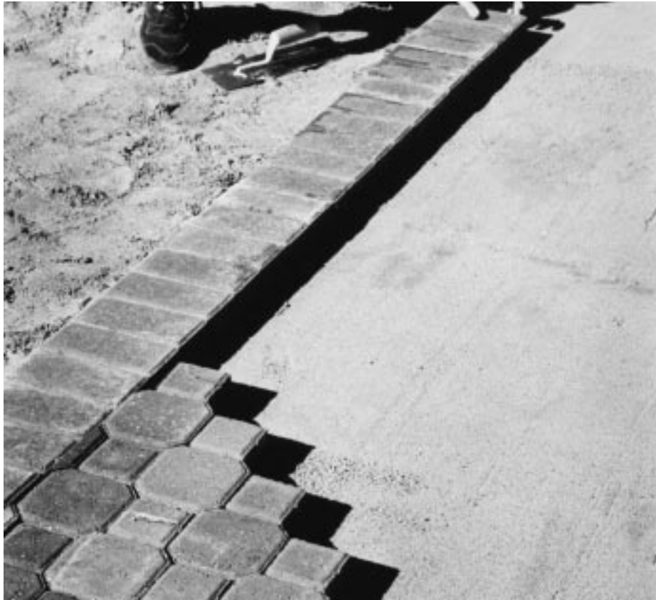
Figure 24-4 Soldier course at edge of pavement.
