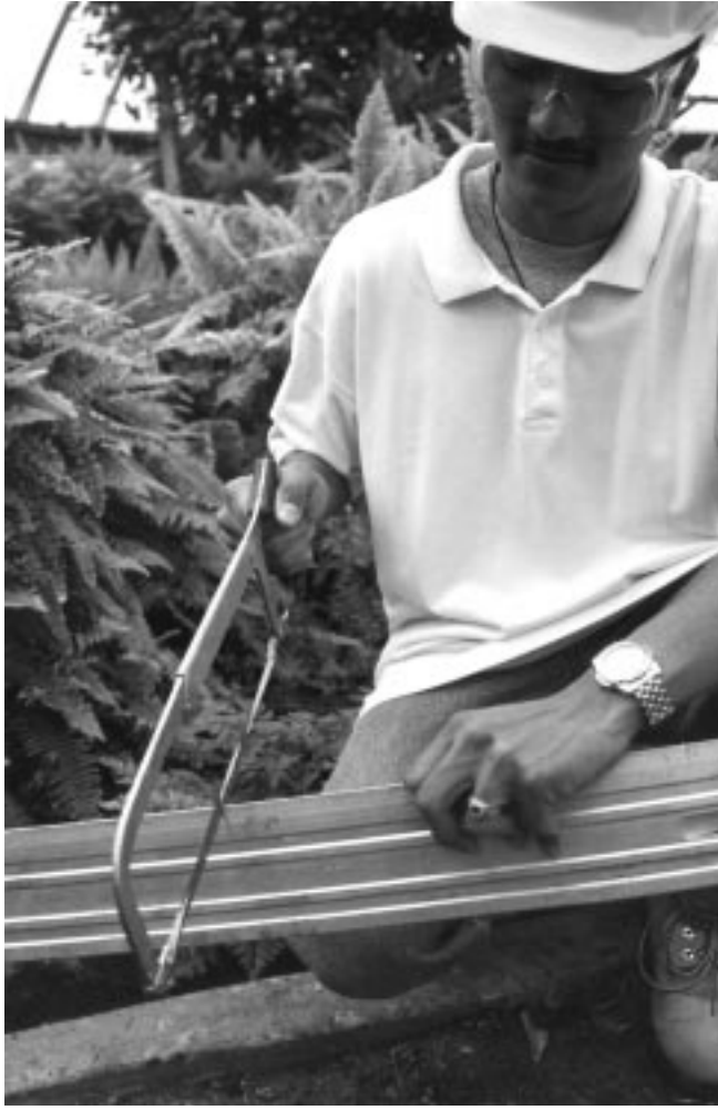
Figure 36–10 Cutting metal edging using a hacksaw.
