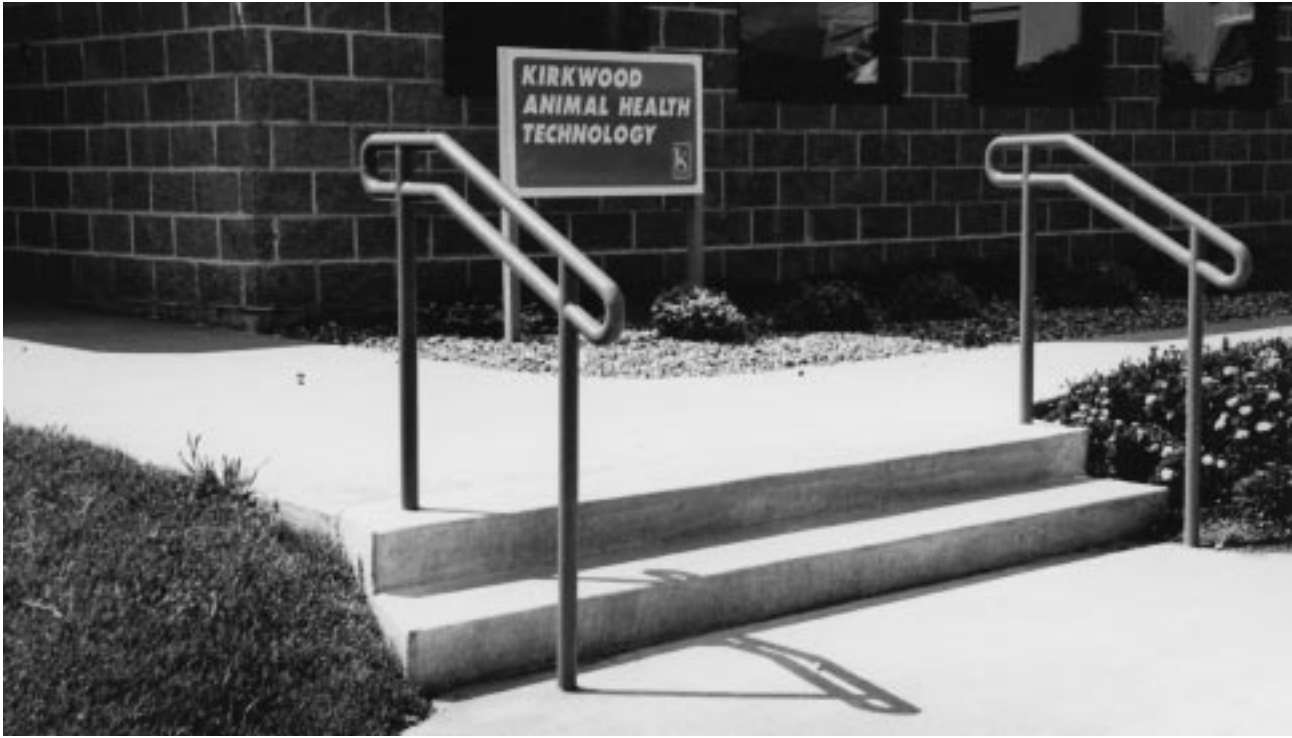
Figure 21-2 Freestanding concrete stairs.
