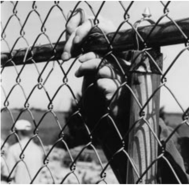
Figure 32-30 Connecting fabric to fence with ties.
