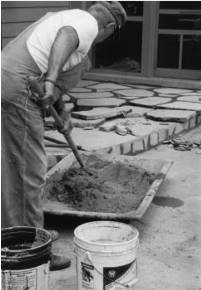
Figure 26-2 Mixing mortar with mortar hoe.
