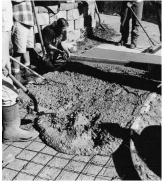
Figure 23–18 Placing and screeding concrete.
