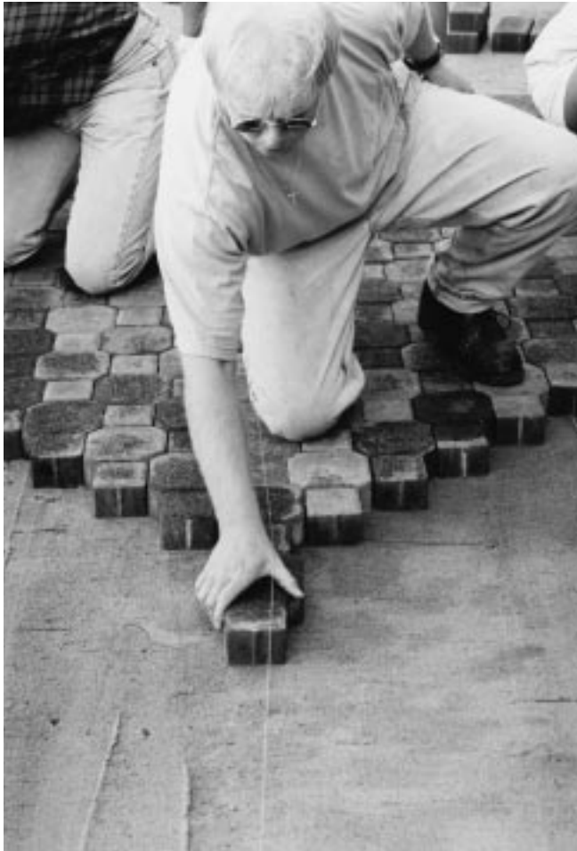
Figure 24–6 Beginning placement of interlocking concrete pavers.
