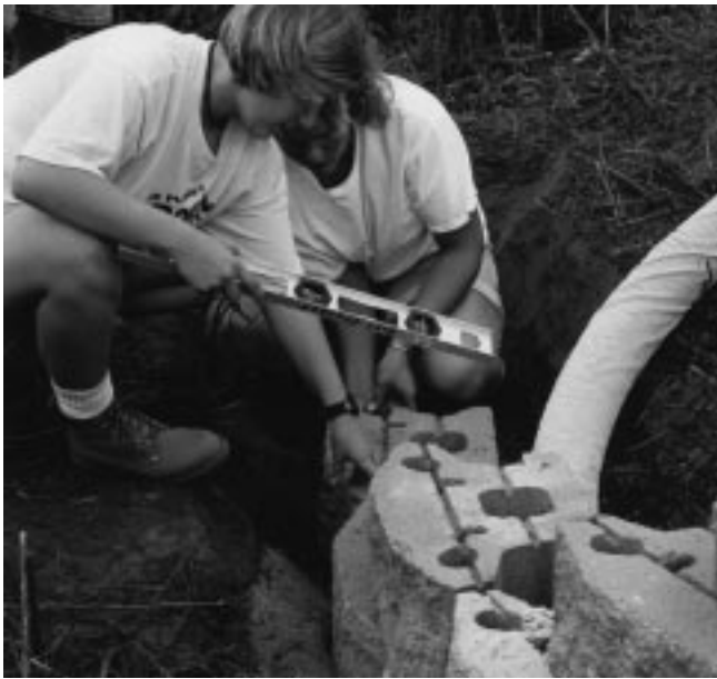
Figure 18-3 Unit placement for precast segmental units.
