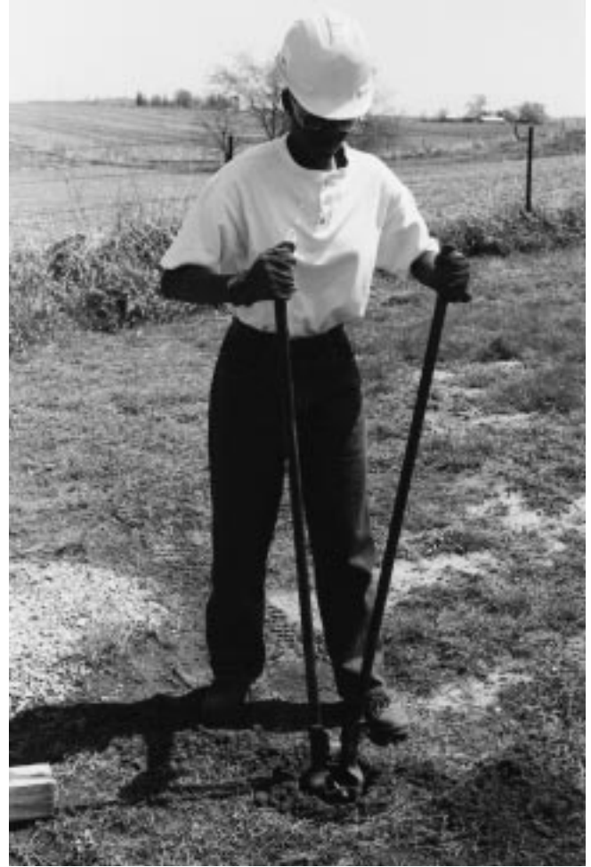
Figure 7-4 Operating clamshell type posthole excavator.
