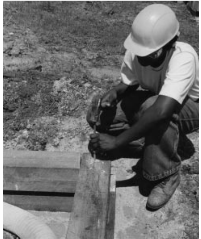
Figure 17-9 Driving spikes in timber with a 2 pound sledge.
