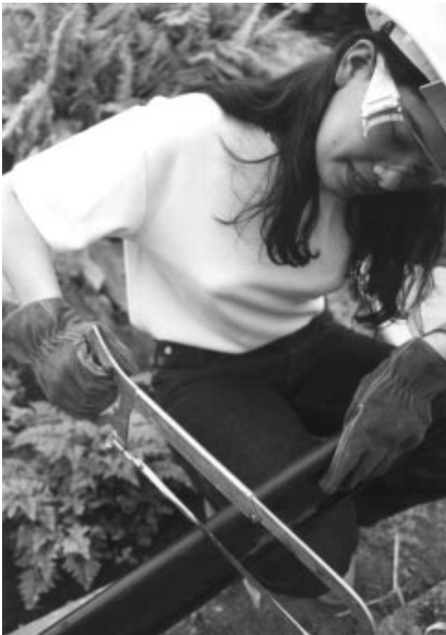
Figure 36–8 Cutting plastic edging using a hacksaw. Tin snips may also be used.
