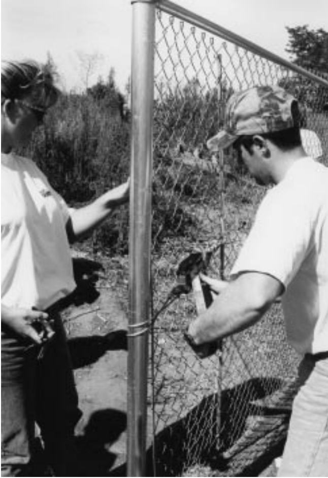
Figure 32-28 Stretching and connecting fabric for chain link fencing.
