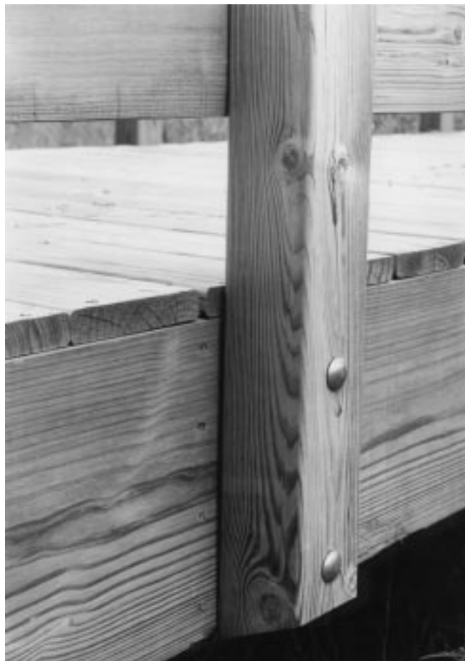
Figure 30–8 Railing support bolted to outside of deck framing.
