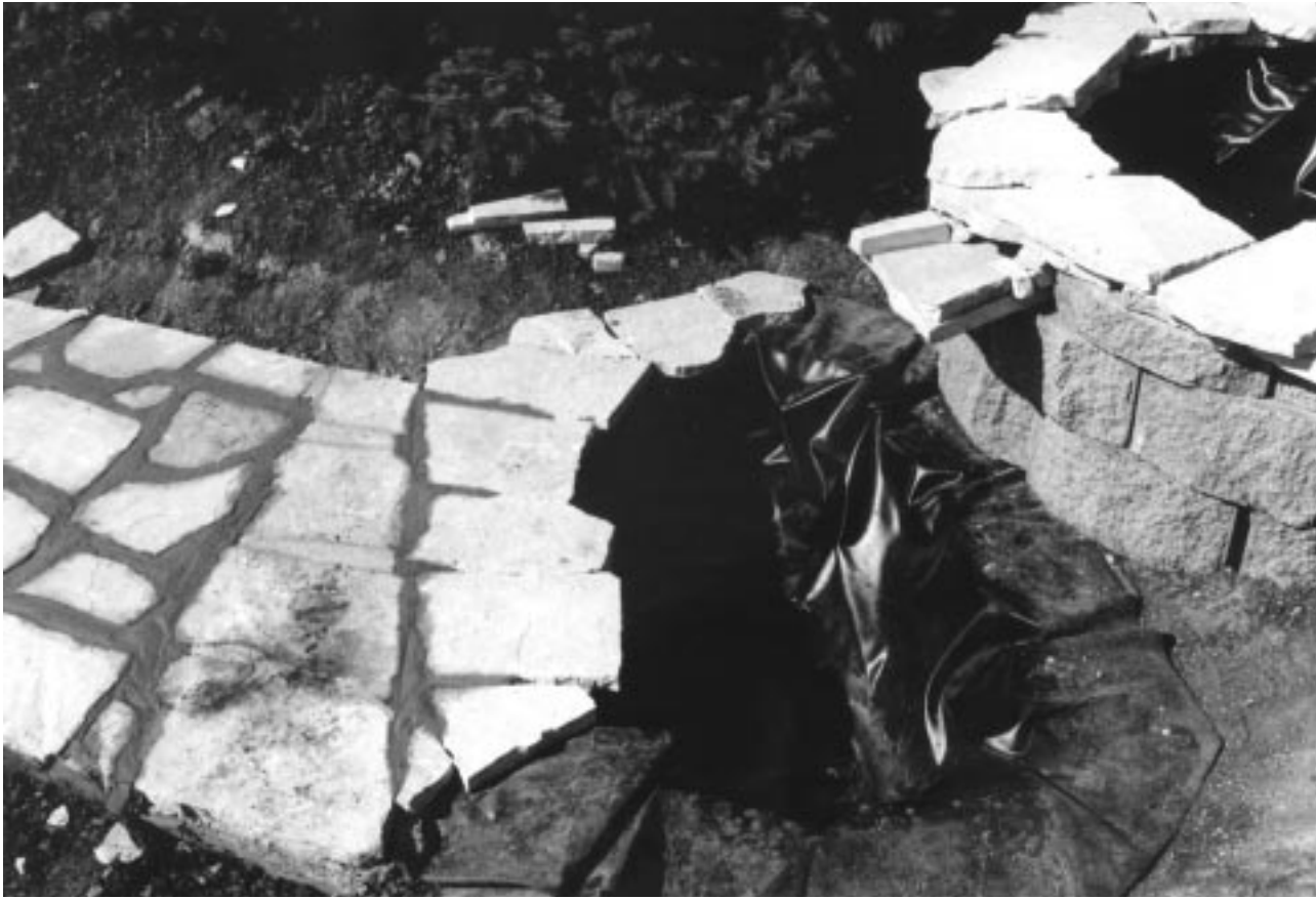
Figure 34–8 Edging a flexible liner pool.
