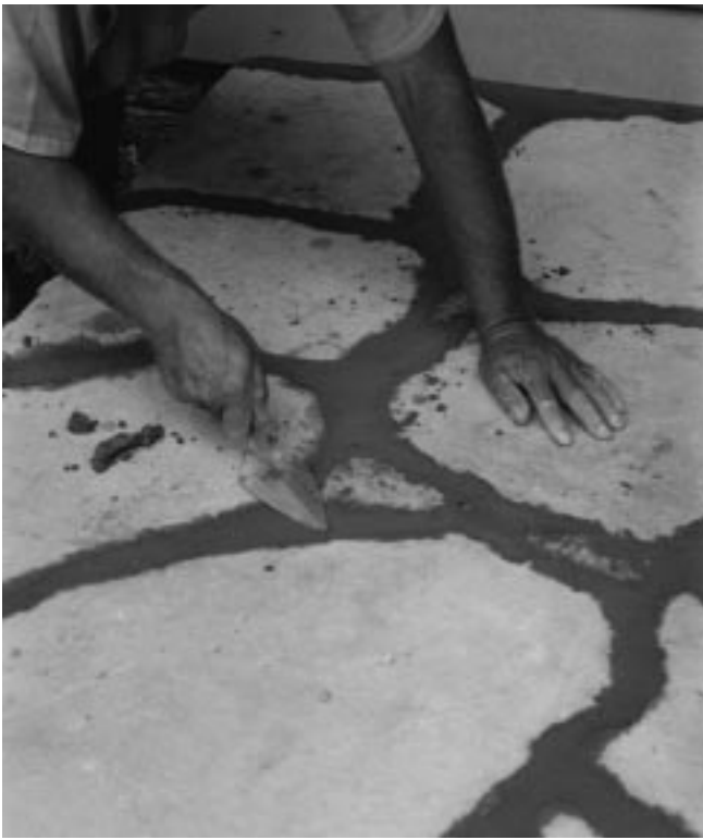
Figure 26-6 Finishing joints using mortar trowel.
