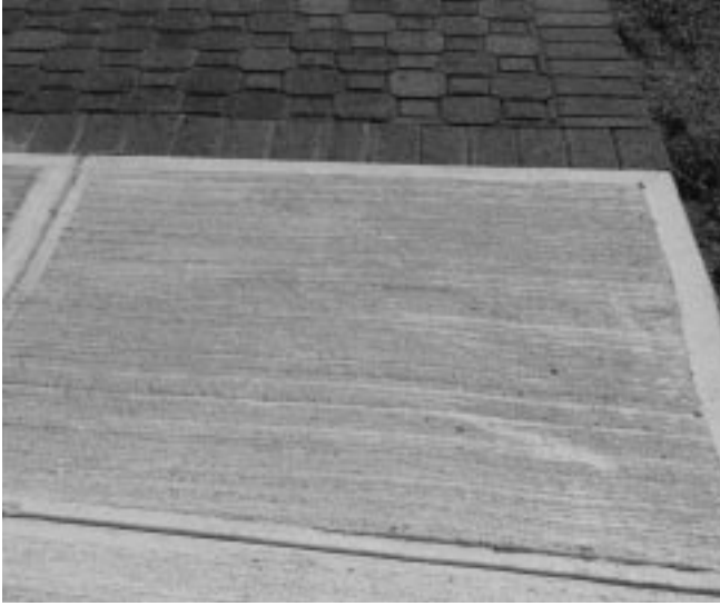
Figure 23-1 Broom finish for concrete walkway.
