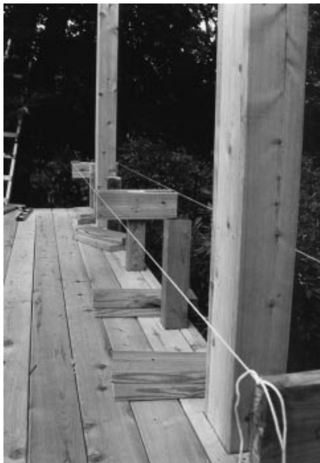
Figure 30-15 Layout and leveling of grab beams for seating supports. Stringlines are stretched from the end supports for the bench. Remaining supports are aligned with the stringlines.
