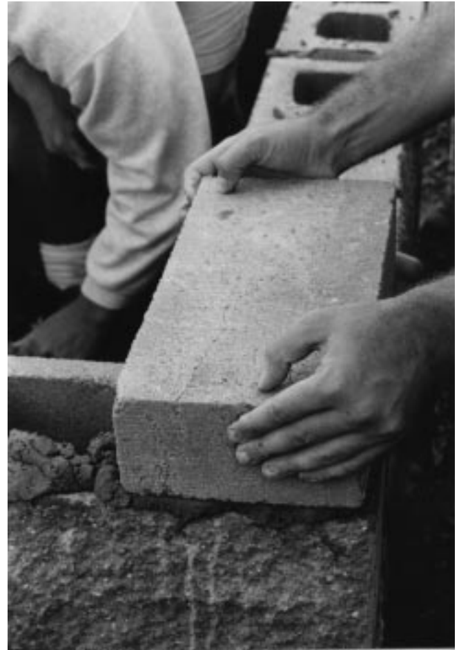
Figure 33–11 Capping a masonry pier.
