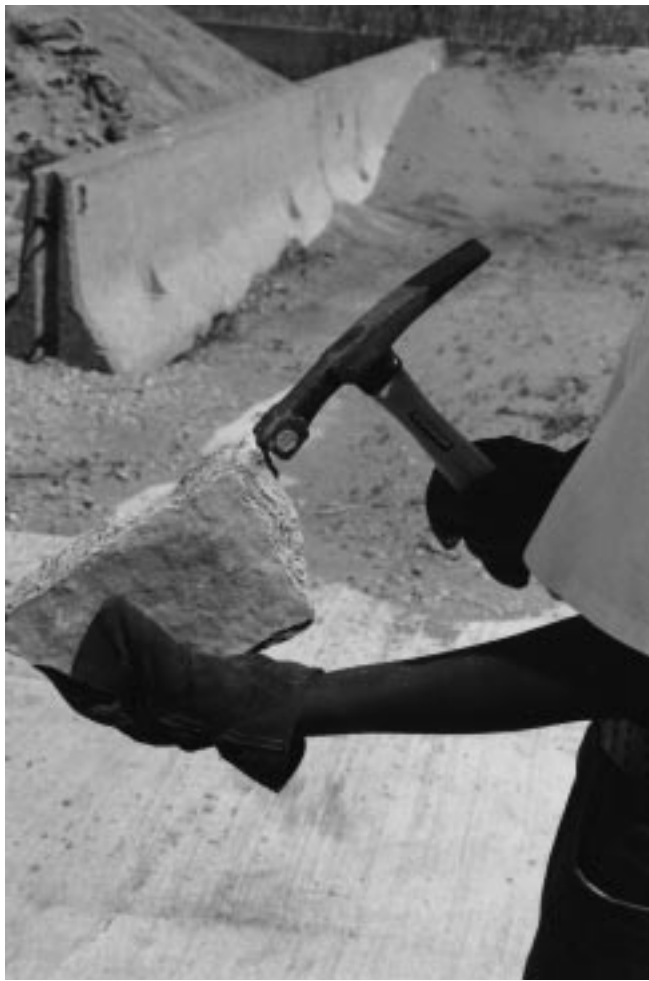
Figure 7-16 Shaping stone edge with a brick hammer.
