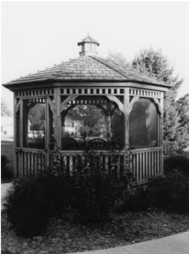
Figure 31-9 Hubbed roof has a high point with several sloped sections, or facets.
