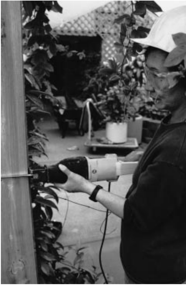
7-23 Cutting using a reciprocating saw.
