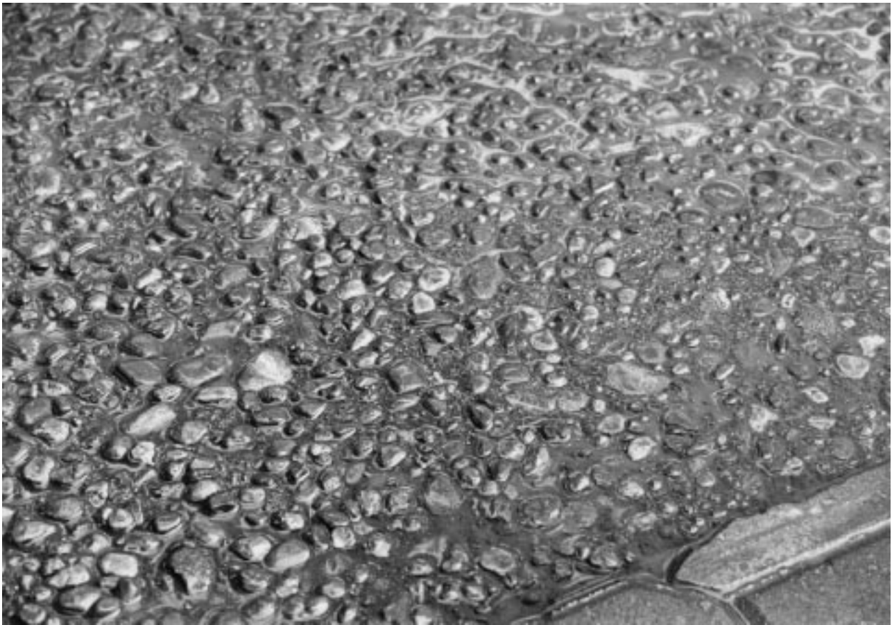
Figure 23-2 Exposed aggregate concrete finish.
