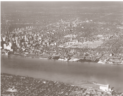
Figure 6.5 Gratiot Redevelopment (Lafayette Park), Detroit, site razed, aerial photograph, 1955.
