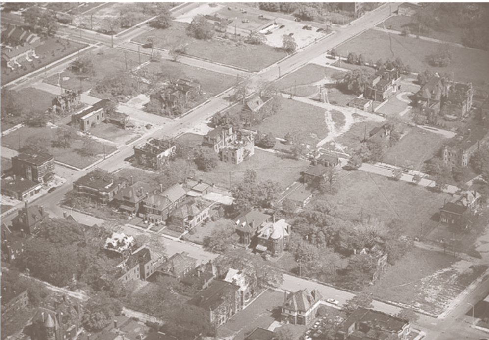
Figure 5.5 Alex MacLean, Brush Park, Detroit, aerial photograph, ca. 1990.
