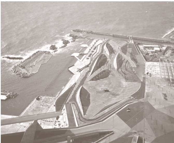
Figure 2.12 Alejandro Zaera-Polo and Farshid Moussavi/Foreign Office Architects, Barcelona Amphitheater, aerial view, 2004.
