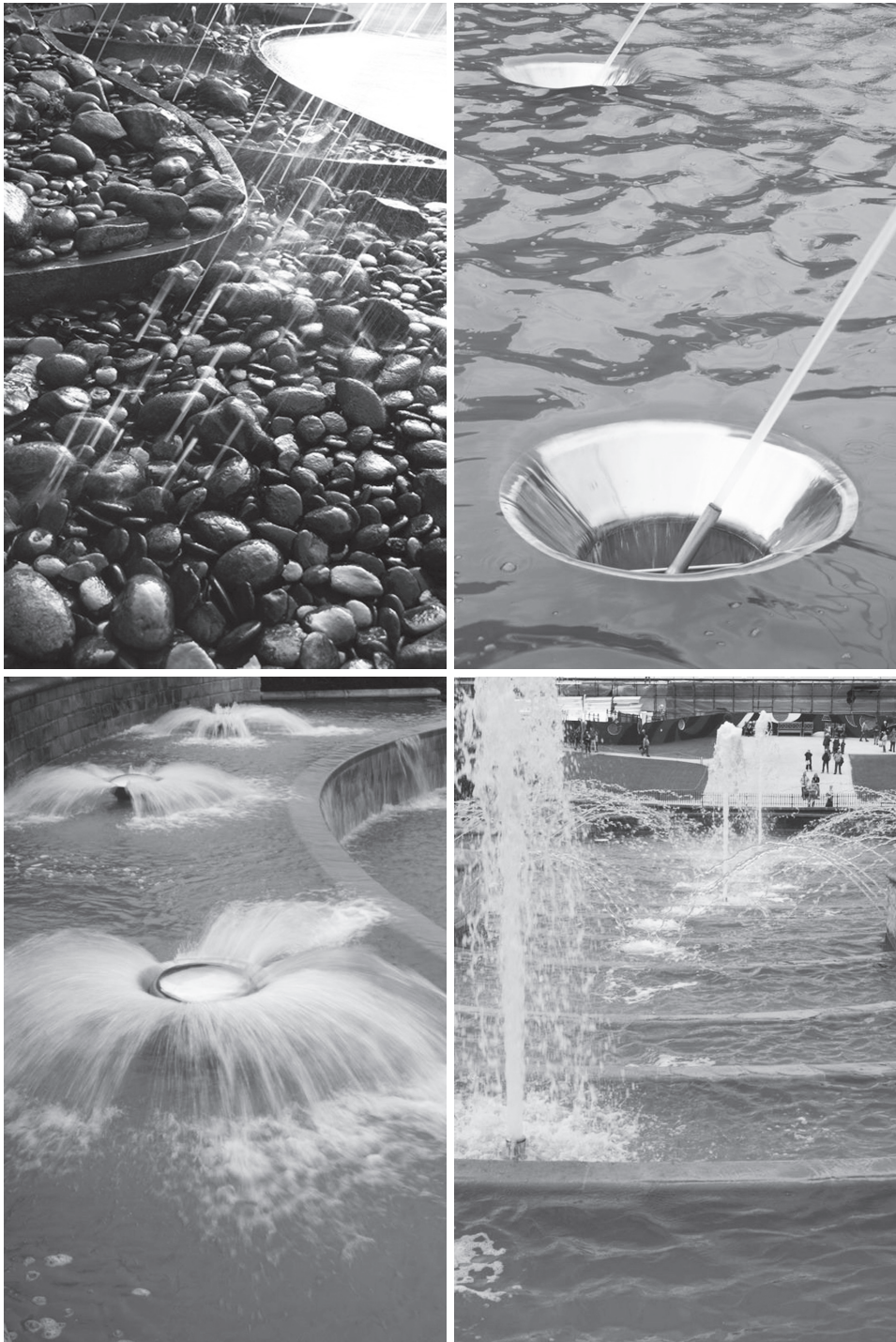
Figure 8.12 Effects of fountain nozzles making water go in different directions such as bore jets-water splashing film-like or knot-like
