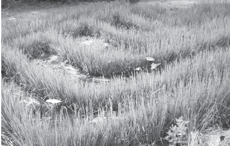
Figure 5.15 The planting of Vetiver grass to retain sediments and prevent erosion along the ditches
