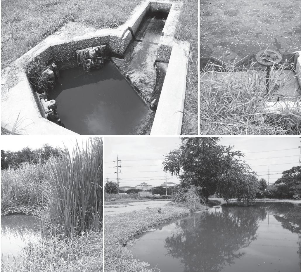
Figure 9.2 A facultative pond and a man-made pond in the Asian Institute of Technology, which covers a large area and is located on the main road. Later they were replaced by a treatment plant so that the area could be used for other purposes.
