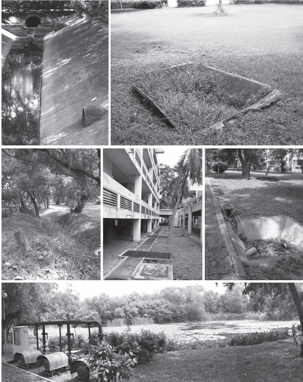
Figure 4.5 The storm drainage system at Asian Institute of Technology is separated from the sewer system. The drainage system is big enough to accommodate a large amount of water. The Figure shows different kinds of drainage system, catch basins and detention areas in the institute.
