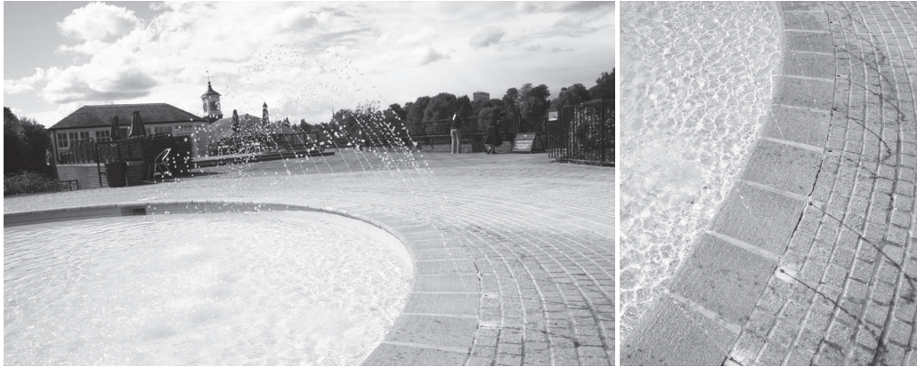
Figure 8.2 (above) A skimmer swimming pool whose water level is below the pool edges. This is the original system used in an old swimming pool called The Serpentine .
