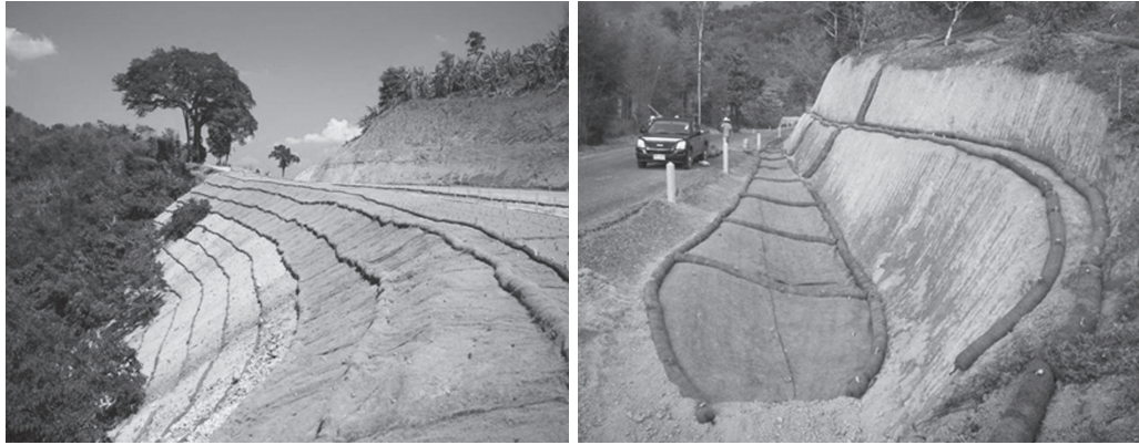
Source: Erosion Control Blanket (ECB) and Erosion Control Log (ECL), products manufactured by Grasgro
