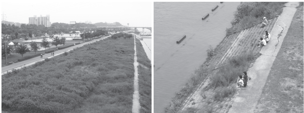
Figure 5.4 The waterfront set-back area (left) in the development of the river banks in Seoul and a multi-terrace (right) to create a green area for recreation during the dry season and a flood plain during the rainy season.
