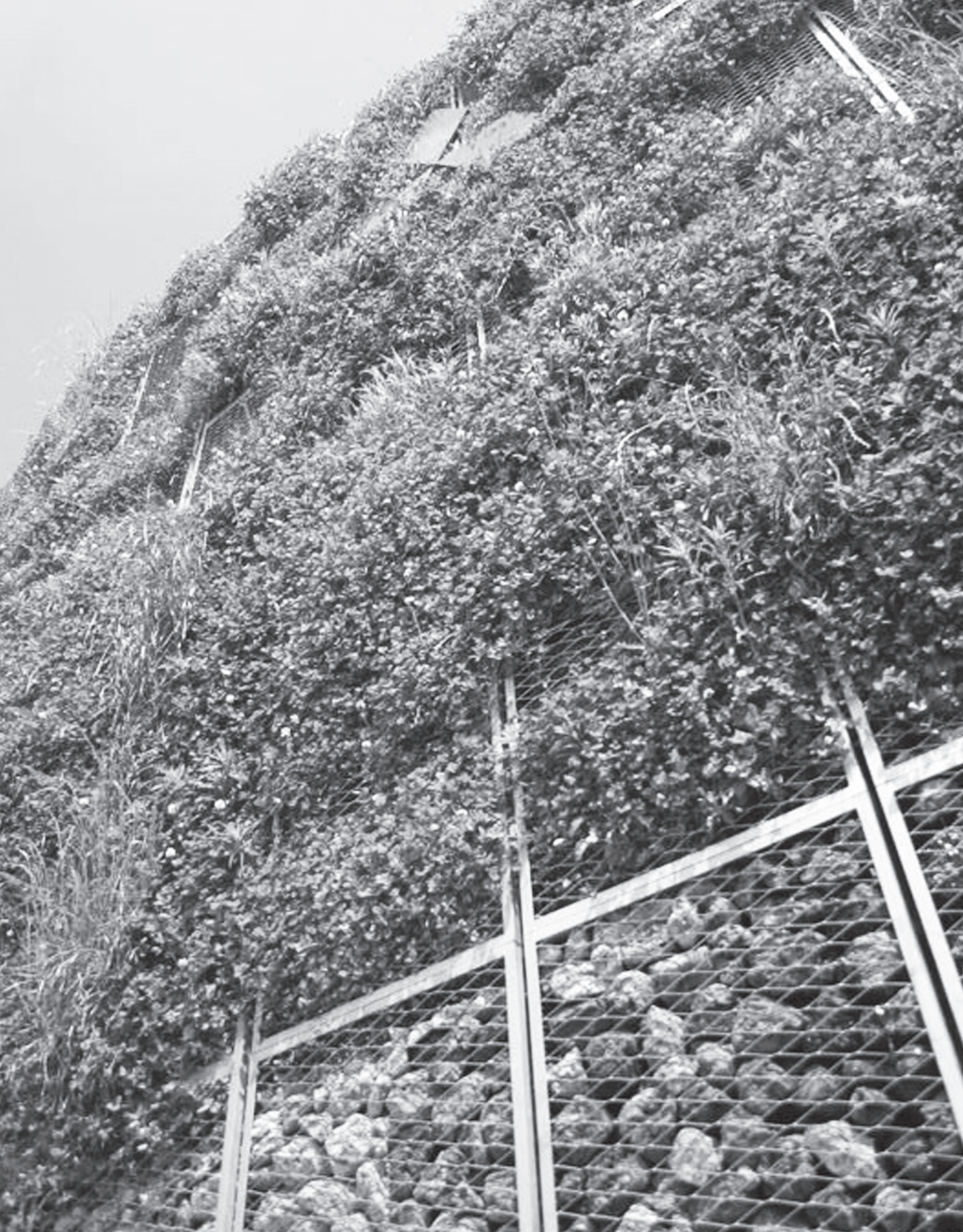
The vertical green area on the exterior wall of Mitsubishi Pavilion in the World Exposition in Aichi
