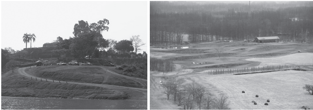
Figure 3.1, 3.2 Grading is carried out for vehicle purposes at Rajaprapa Dam (left) and for pleasant scenery in Tokachi Millennium Forest, Hokkaido (right)
