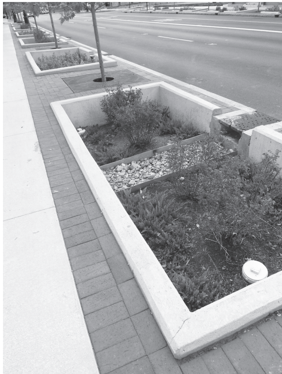
Figure 4.22 The drainage system in Columbus, Ohio, U.S.A. The system is environmentally friendly as seen from the sign “Dump no waste drains to river” because the water flow into the rivers. On both sides of the road, there are rain gardens to retain storm water.
