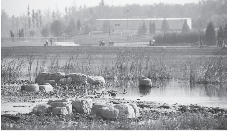
Figure 7.6 The treated wastewater is drained to the artificial ponds in the Beijing Olympics Park
