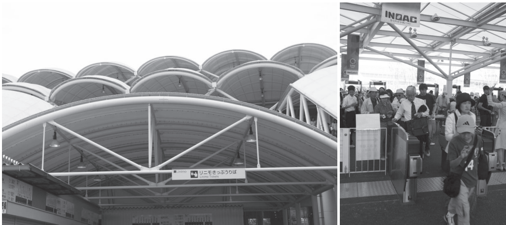
Figure 1.1 The arched entrance of the 2005 World Expo in Aichi, Japan. As the entrance was an open area, a roof was required but there had to be so few posts that they would not obstruct the flow of visitors. The architect used an arched roof made of iron trusses iron that could cover a large area but required few posts located at certain intervals.
