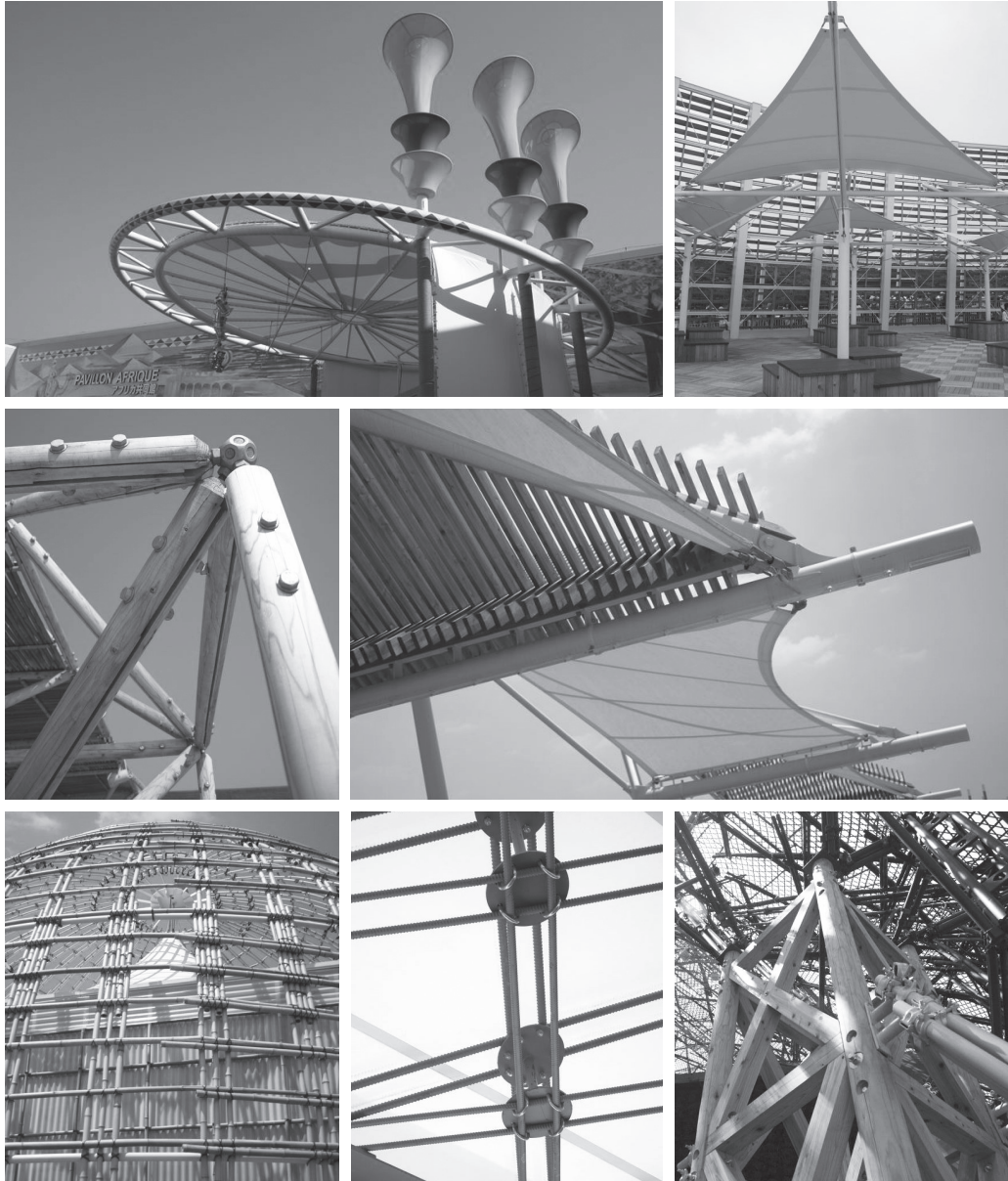
Figure 1.2 Summer pavilions with different kinds of roofs displayed in the 2005 World Expo in Aichi, Japan. These beautiful roofs were uniquely designed and built with modern techniques and materials. They were in line with the theme of the event – Natural Wisdom. The unique characteristics of these roofs were the design of joints and the binding of materials such as the stretching of canvas and the binding of circular-cut posts together with specially designed joints so that they could be adjusted into different shapes.
