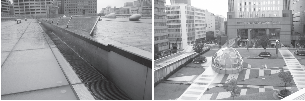
Figure 13.4 The roof garden that can harvest rain water in the Oasis 21 Project, Nagoya
