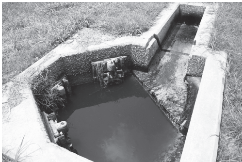
Figure 9.4 A man-made pond using combined systems to treat wastewater in the Asian Institute of Technology. Some plants are used to treat wastewater before the water is discharged.
