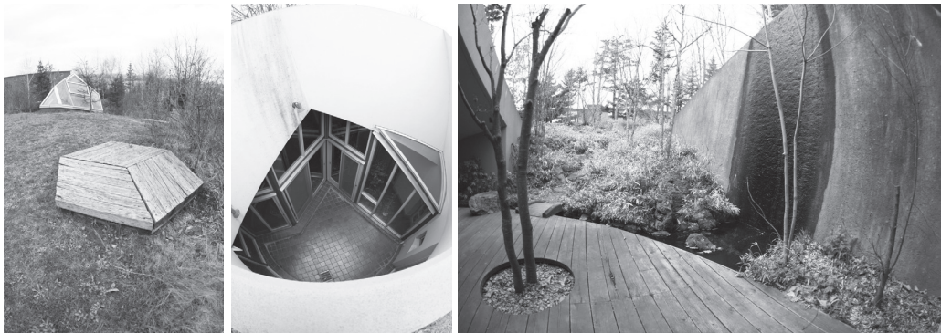
Figure 1.6 Takahachi Construction Headquarters (designed by Takano Landscape). Besides the green roof, the company is designed to be part of the surroundings by creating a friendly atmosphere and breaking away from a box-like office. The company also relies on natural light and cools itself with the variety of plants.
