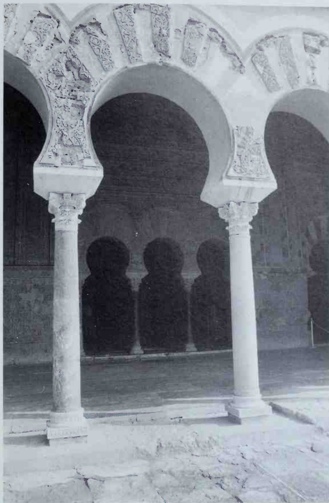
Madinat az-Zahra': heavily restored arcading in the former palace.
