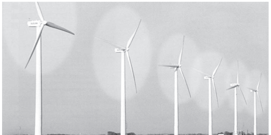
4.31. A large scale wind farm with 1 MW turbines.
