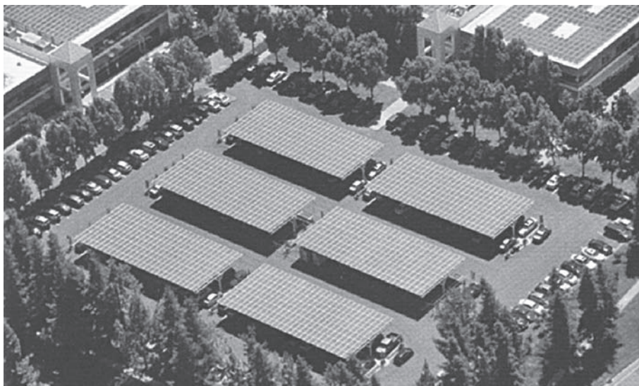
4.26. A 1.6MW PV system for Google's HQ in San Rafael, CA a roof over a parking area.
