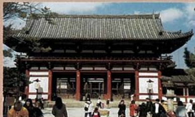
Rōmon: eight or twelve posts, two stories, one roof, e.g. Tōdaiji Temple, Nara City.
