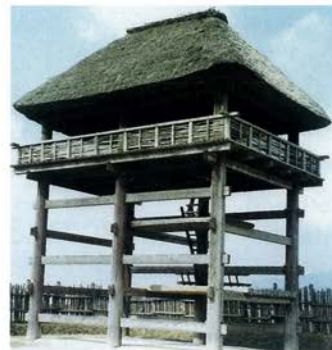
Lookout tower at Yoshinogari, reconstructed Yayoi village, Kyushu.
