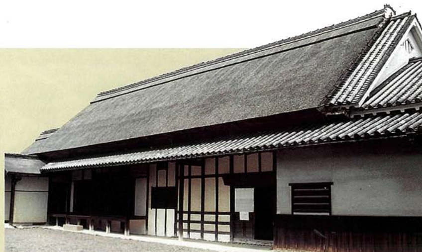
Yoshimura House, built in the Yamatomune style, with a thatched roof and tiled extensions.
