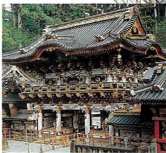
Yōmeimon at Tōshōgū is a two-story gate, 11.1 meters high and 4.4 meters deep, with a Chinese style curved roof. The building is decorated with 508 colorful carvings.
