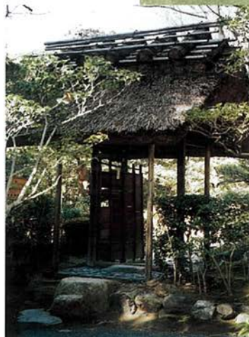
The Kayamon Gate is constructed of poles covered with a grass roof. On top of the roof is a bamboo and log frame designed to help hold the grass in place.
