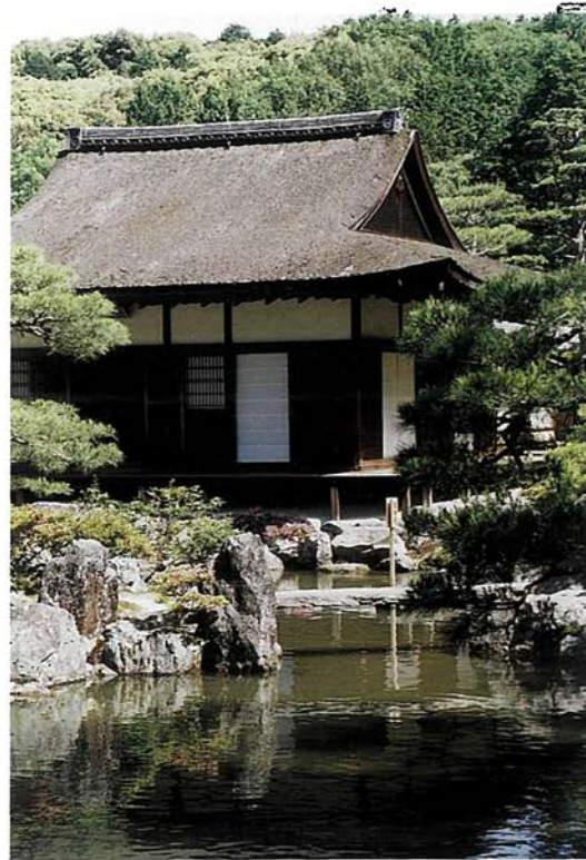
The Tōgudō at Ginkakuji is a single-story building with a hipped-and-gable roof covered with Japanese cypress bark. The Silver Pavilion and Tōgudō, much more restrained than the pavilion at Kinkakuji, have been designated as National Treasures.
