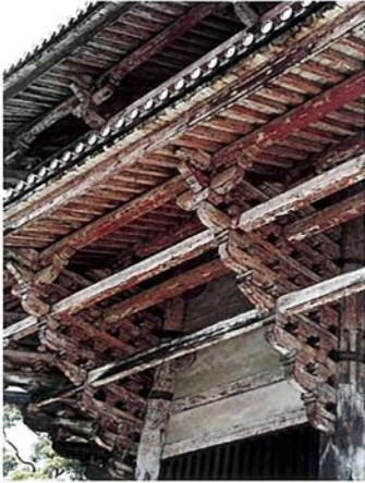
Detail of the Nandaimon Gate at Tōdaiji, showing the multi-tiered bracketing system.
