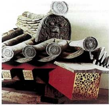
Model of an ornamental roof tile used on a corner of the roof of the second Daigokuden. The tile is called onigawara (tile with a "devil" face). The face shown here is a good devil, whose job was to frighten away bad devils that caused fire, lightning, wind, and other damage to buildings.
