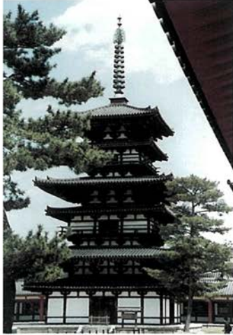
The East Pagoda of Yakushiji Temple, built in 730, is one of the few surviving buildings from the Nara Period. Intermediate covered eaves give the three-story building the appearance of having six floors.
