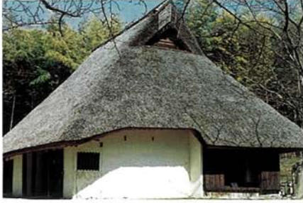
The former Yamashita residence from Fukui Prefecture is an Ō-uragata style farmhouse with thick pillars and beams to withstand the heavy snowfall in the area. The house has been moved to the Open-air Museum of Old Japanese Farmhouses in Osaka.
