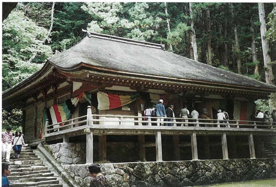
The Kondō (Main Hall) at Murōji, built in the early Heian Period, has a hipped shingled roof and is accommodated to the slope on which it is built by a stone terrace that supports the wooden veranda. The natural cypress forest can be seen in the background.
