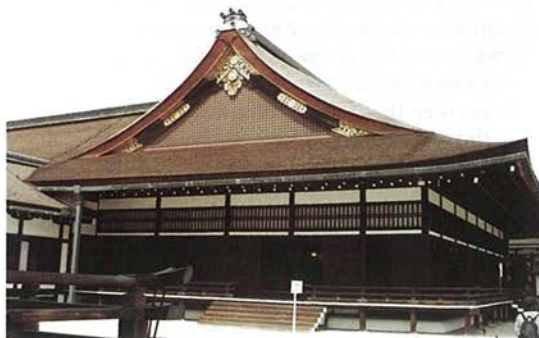
Ogakumonjo, a building in the Goshō Palace that was used for study, poetry reading parties, and other gatherings.
