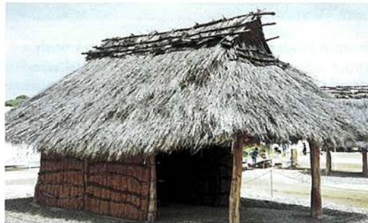
Above: A flat-land building ( heichi jūkyo ) in which poles were sloped to the top and thatched, serving as both walls and roof. The ground served as the floor.
