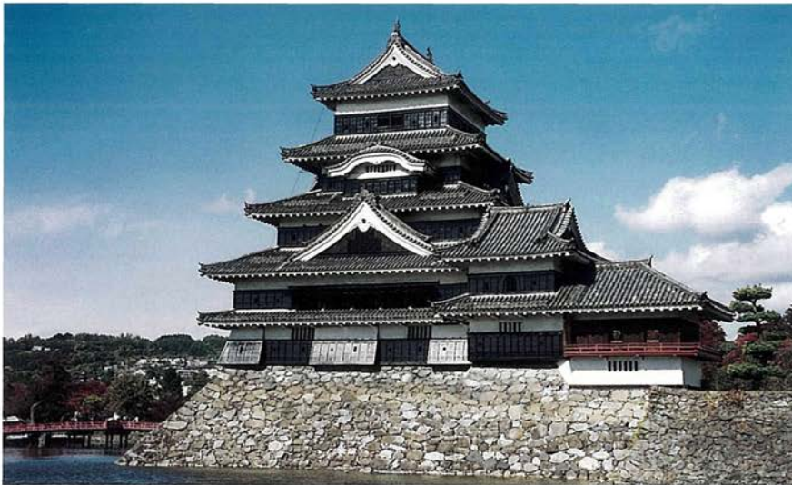
Matsumoto Castle in Nagano Prefecture, built in 1596, is one of the twelve remaining original castles in Japan.
