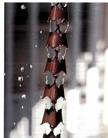
A traditional downspout consists of small linked metal cups. As a cup overflows, water is passed down the chain to the next cup, to form an interesting and dynamic pattern.
