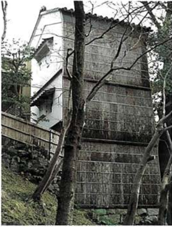
Three-story kura belonging to a traditional Japanese restaurant in Kyoto. The kura is covered on one side with bark to protect the plastered wall and to provide extra insulation. Three-story kura are rare today.
