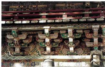
Detail from the Bell Tower, showing the elaborate bracketing system and colored decorations.
