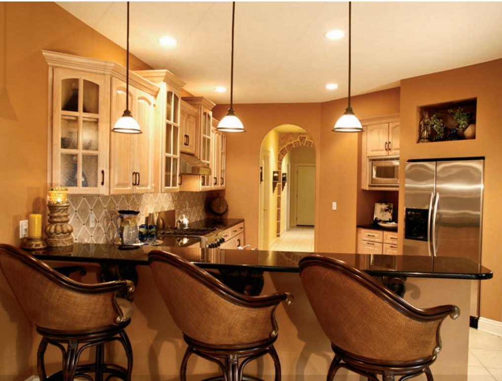
Figure 5.8 This kitchen uses direct downlighting, ambient eyeball spotlights, undercabinet task lighting, and three minipendants for lighting the informal dining bar. The lamps for these luminaires may be incandescent or fluorescent. Design by Shelya Huff-Hrenya, Hollywoodhomeware.com/© Marc Anthony Photography
