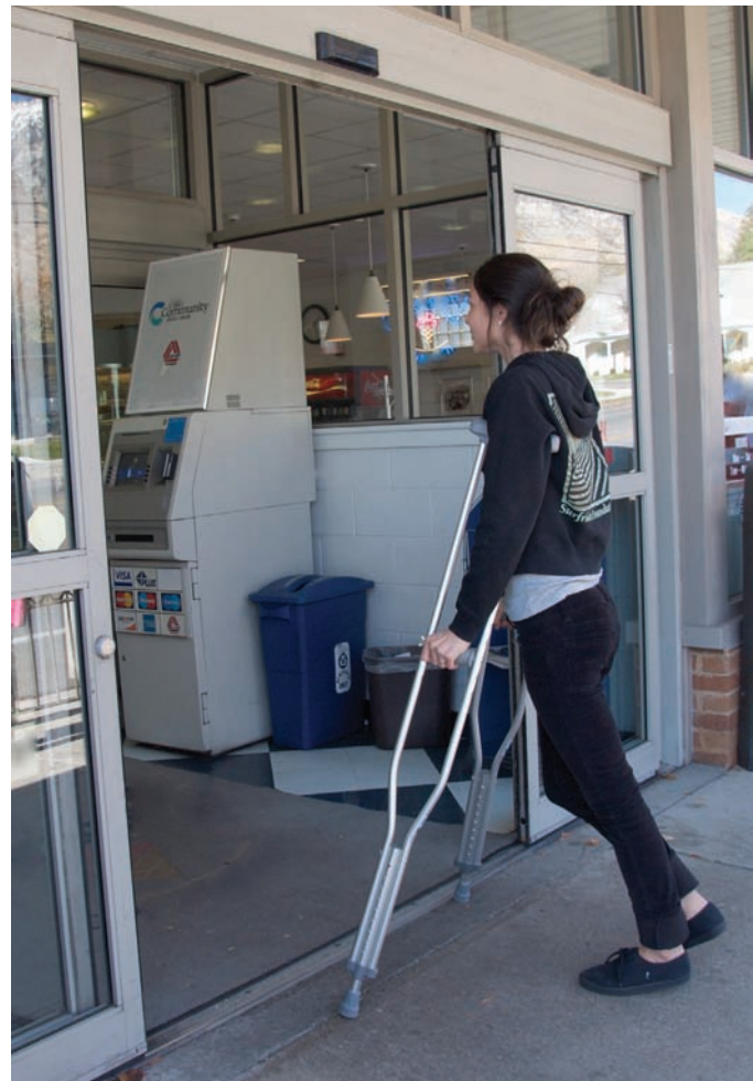
Figure 2.10 These sliding doors operate by overhead sensors that detect movement, opening for all users without calling attention to disability, qualifying them as universal design. Photo © Kathryn Taylor
