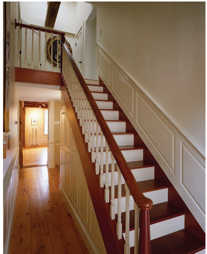
Figure 10.46 A straight-run, semi-housed stair also features traditional paneling on the walls. The contrast of white balusters and risers to the cherry-stained banister, newel post, wall stringer, and treads makes a high-contrast color scheme with a keen sense of rhythm by alternation. Design by Donham & Sweeney Architects/photo © Brian Vanden Brink
