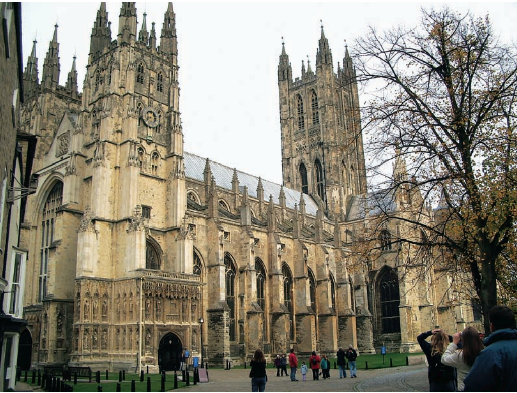
Figure 15.4 Canterbury Cathedral has an impressively scaled tower over its crossing, a typical feature of English Gothic churches. Photo © Kathryn Taylor
