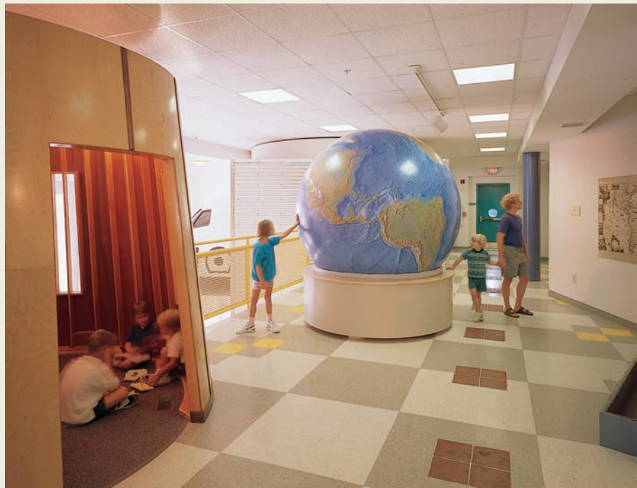
Figure 12.4 Resilient sheet flooring provides graphic design and relative warmth and quiet in the Portland, Maine, Children's Museum. Stephen Blatt Architects/photo © Brian Vanden Brink
