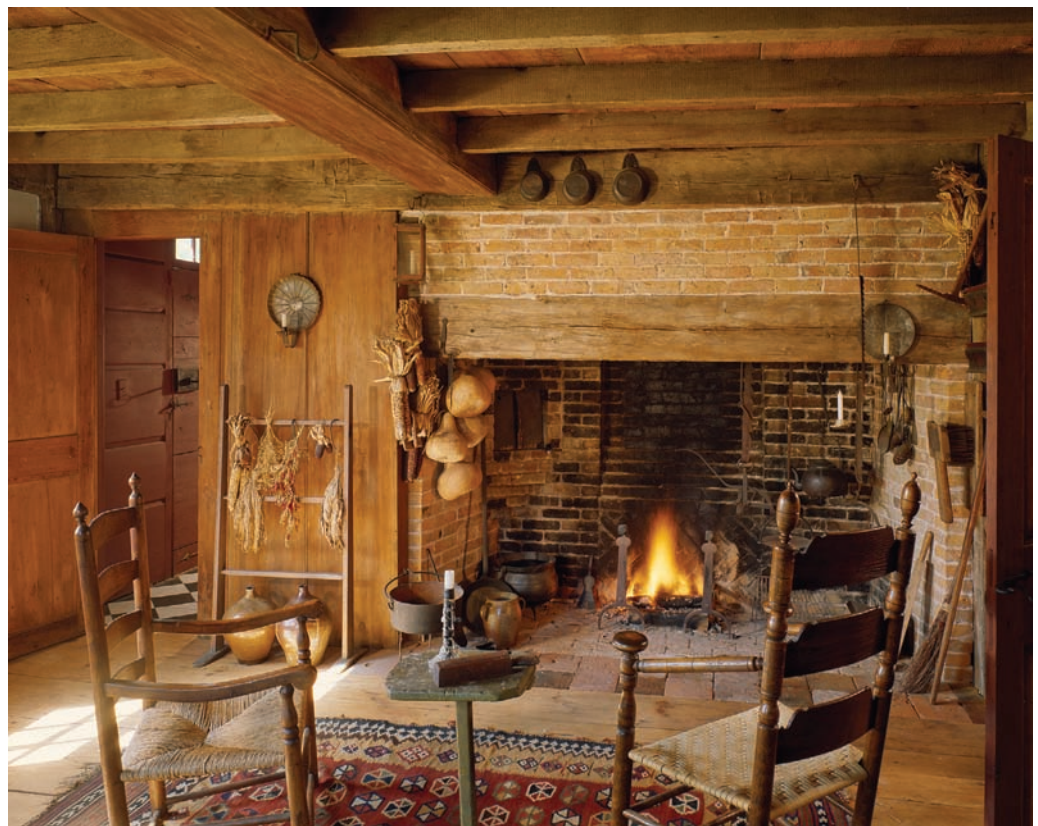
Figure 15.10 This English Medieval-style room incorporates many features common to seventeenth-century American houses, such as the summer beam, palisade wall, and a large timber mantelpiece. Photo © Brian Vanden Brink
