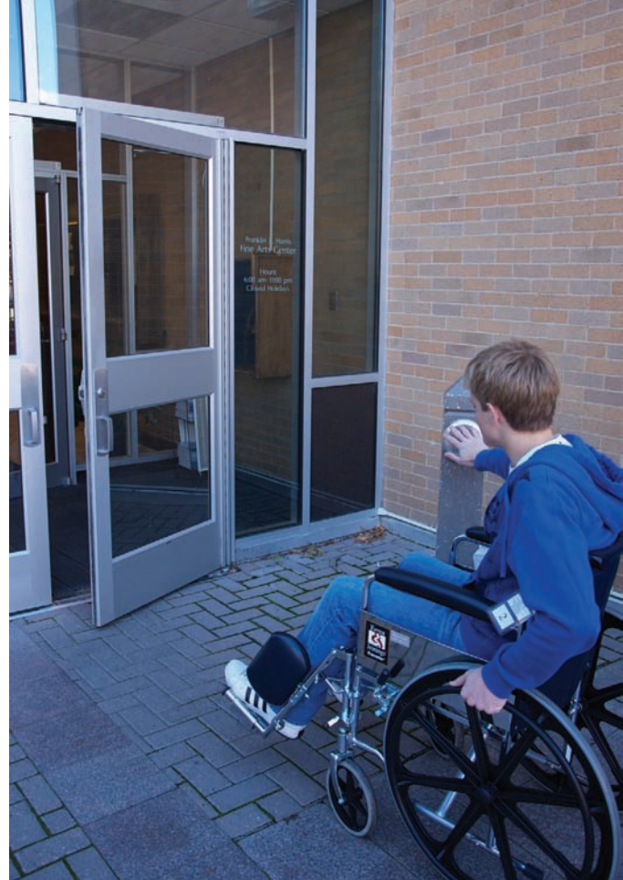
Figure 2.13 The Americans with Disabilities Act requires a level, barrier-free, and spacious entry and an easily accessed door-opening push-button device on at least one entrance of all public buildings. On push-command, the door opens slowly, giving the chairbound-disabled person time to maneuver and wheel through the entrance. These buttons are sensitive and should be treated with care and respect by pushing gently and firmly, not “hitting” the button. Also, when a person pushes the button and then impatiently forces the door by pushing on it, the unit can break. This scenario is often the result of an ambulant person who desires the convenience of the automatic door yet misunderstands the need for the device to work slowly for the safety of all and so that ambulant-disabled persons are not rushed in accessing the building. Photo © Kathryn Taylor
