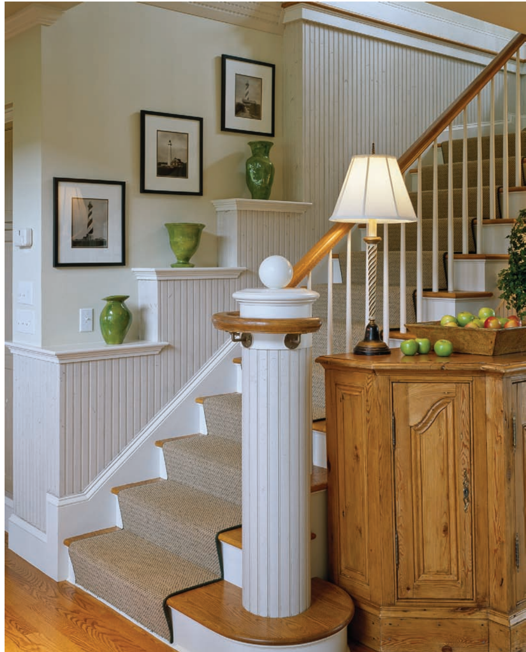
Figure 10.5 Beadboard is used creatively in this straight-run, semihoused stairwell. Design by Hutker Architects/photo © Brian Vanden Brink
