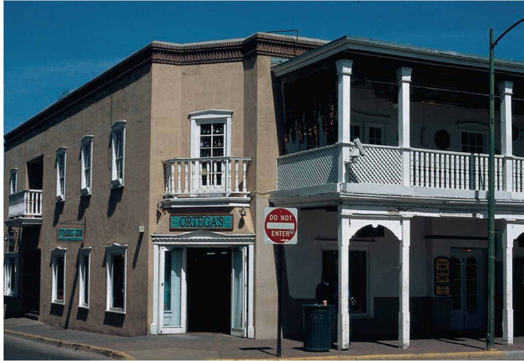
Figure 15.22 This building in Santa Fe, New Mexico, is an example of the Territorial style. Note the boxed columns and the brick pretil as well as the lack of vigas. Photo © David A. Taylor
