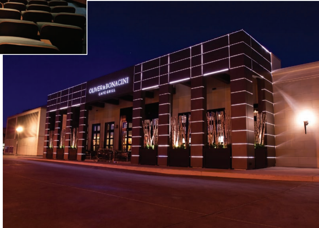
Figure 5.25 LED lighting was planned as an attractive design element in the reveals of aluminum panels of this new facade of the Oliver & Bonacini Café Grill. Design by Anacleto Design Associates/photo courtesy of Eventscape, Inc. www.eventscape.net
