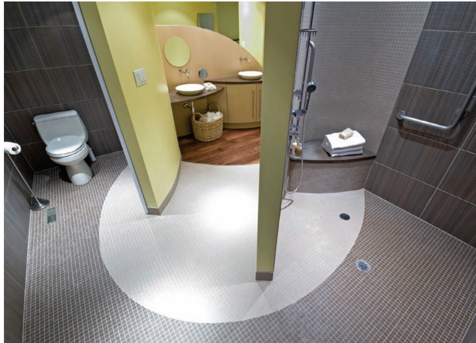
Figure 2.20 This handsome universal design bathroom is planned for users who are both ambulant and wheelchair bound. Features include a roll-under sink and accessibility to the toilet, with a sliding door for privacy. The open, roll-in shower area has a seat/bench and handheld “Swedish” shower and grab bars. Tile surfaces are impervious to water and barrier free. Design by Anthony Binns, CKD, CBD; Binns Kitchen + Bath Design/Photography: Tim McClean/NKBA Design Competition
