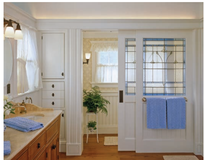
Figure 10.16 Beautiful art glass is inset into these traditional paneled doors. The sliding door pockets behind the front door, allowing access to the toilet area. The art glass brings natural light from the outside wall into the grooming area. Design by Hutker Architects/photo © Brian Vanden Brink
