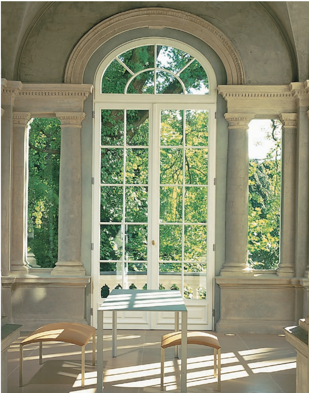
Figure 10.21 A “Palladian” arrangement of French doors, an elliptical fanlight transom, and a pair of fixed-glass windows are framed with Italian Renaissance columns, entablature, and raised podium. Photo © Paul Warchol
