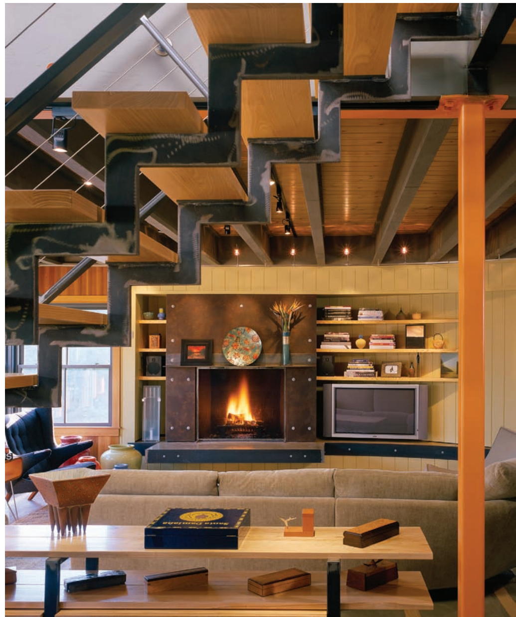
Figure 10.58 These ceiling beams are stained charcoal black, giving a greater appearance of strength and matching the black metal of the Modern open-riser stairs and fireplace surround. Design by Hutker Architects/photo © Brian Vanden Brink
