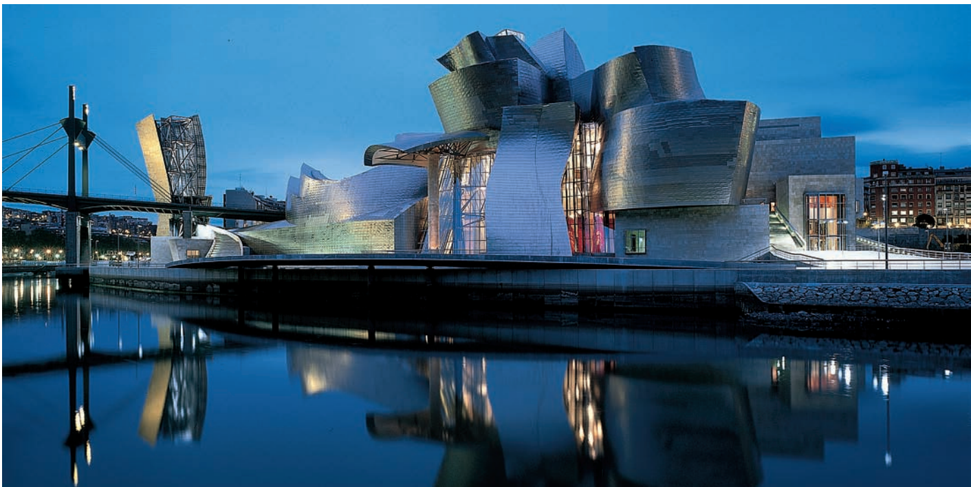
Figure 15.37 Frank Gehry's Guggenheim Museum in Bilbao, Spain, with its distinctive sculptural shapes and its brilliant titanium skin, is an internationally recognized example of Deconstructive design. The Solomon R. Guggenheim Foundation, NY/photo: David Heald
