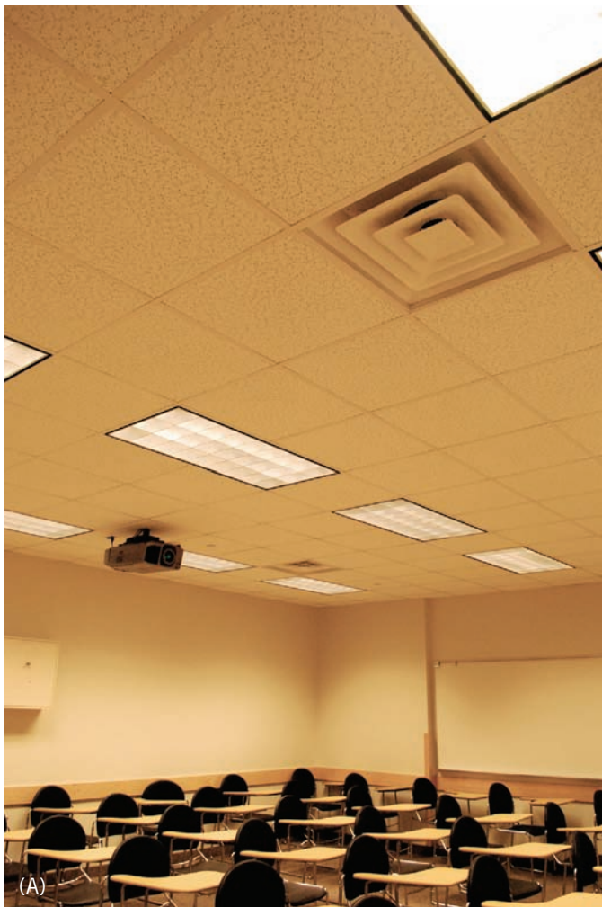
Figure 7.30 (A) The plenum is the area above the ceiling; here a suspended ceiling of acoustical tiles provides access to any of the systems in the plenum, including the lighting, heating/ventilation/air-conditioning (HVAC), the projection system, or the fire alert/sprinkling system. (B) Egress lighting must be visible both when the lighting works and when there is a temporary electrical outage or emergency, in which case the LED lights continue to operate to lead users to outdoor safety. Photo © Kathryn Taylor
