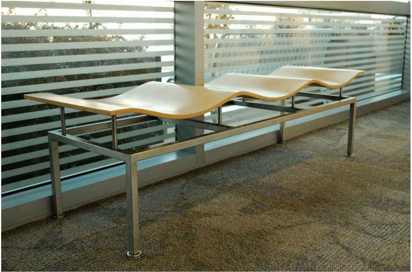
Figure 12.23 Modular carpet tiles in random abstract patterns allow for simple replacement of worn areas without the expense and waste of replacing carpet in large spaces, such as this heavy-traffic contract hallway. Photo © Kathryn Taylor
