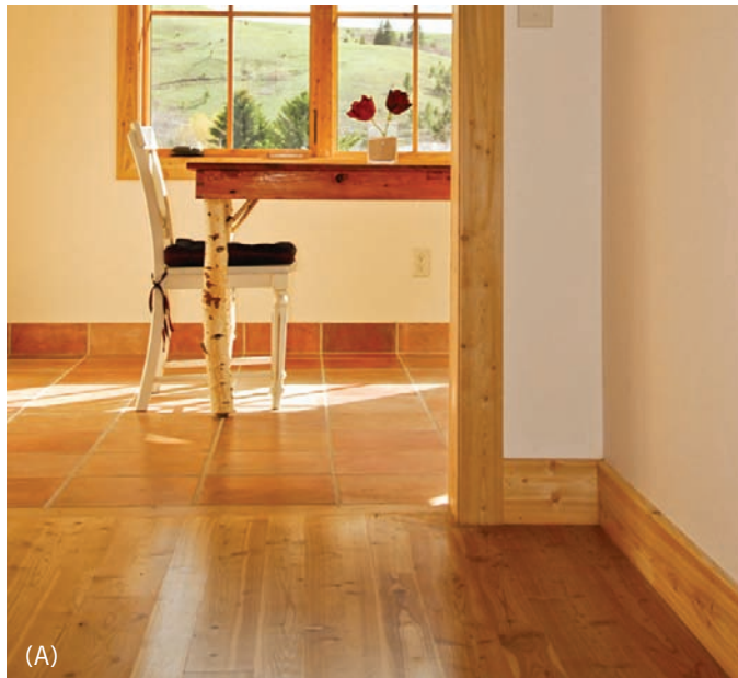
Figure 2.1 (A) This sustainable-source wood floor is harvested from forest restoration projects and only as small-diameter trees that allow old-growth forest conditions to return, restoring the forest to its original healthy integrity with greatly reduced danger of high-intensity fire. These smaller trees have a dense grain and hard fiber, perfect for beautiful durable flooring and trim. (B) Broadloom carpeting and cushions can be sustainable in a number of ways. High-quality, dense tufted carpets in neutral, variegated two-tone effects have a longer physical and aesthetic life span and are less likely to show soiling and wear from traffic. During production, green manufacturing methods use less water, less energy, or renewable energy from bio-based fuel. The carpet may pass the Carpet and Rug Institute (CRI) Green Label Plus, enhancing the contribution toward LEED-certified buildings. Carpets may contain postconsumer reused content, such as polyethelene (PET—recycled plastic bottles) fiber. Carpet can also be collected at recovery and recycling centers, which diverts waste from landfills. Carpet may be made completely or in part from polylactic acid (corn syrup) renewable fibers, such as DuPont’s Bio-PDO™, a key ingredient in Sorona® fiber used in Mohawk Industries SmartStrand™ carpet. And new carpets may be engineered to release far less greenhouse gas emissions, resulting in better indoor air quality (IAQ). (A) Photo courtesy of Lupine Design, Clawson Windows and North Slope Sustainable Wood, (B) Photo courtesy of Mohawk Industries
