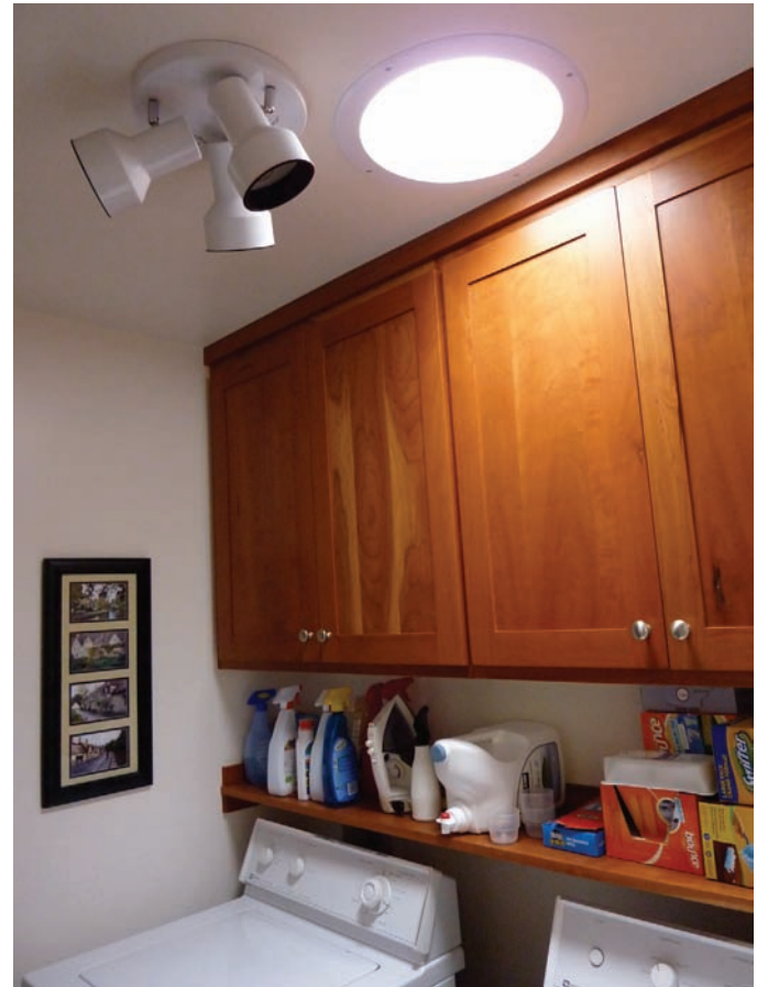
Figure 5.23 A Velux Sun Tunnel™ skylight delivers harnessed natural sunlight into this laundry room, thereby eliminating the need for artificial lighting until nighttime, when this flush-mounted ceiling luminaire is switched on. An option is to install a light kit with a socket for a lightbulb just above the Sun Tunnel diffuser, to provide nighttime artificial light from the same fixture. Photo © David A. Taylor
