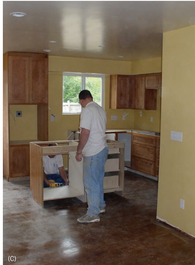
Figure 1.17 Interior designers work closely with trades professionals or subcontractors such as (A) painters; (B) electricians, who install rough wiring for lighting and technology systems and finish electrical—the installation of switches and outlets, luminaires, media, and electronic devices; and (C) cabinet-makers, who measure, construct, and install built-in cabinetry for kitchen, bath, dining room, office, or other residential and contract locations where custom built-ins enhance the design and function of the space. (A and C) © David A. Taylor, (B) © Judy K. Brody
