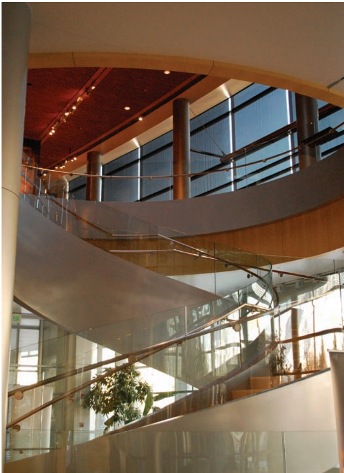
Figure 11.23 In the upper level of this modern structural building, automated roll-down solar shades protect a gallery display and seating areas from the potential harm of UV light and discomfort of excessive glare or heat gain. Photo © Kathryn Taylor
