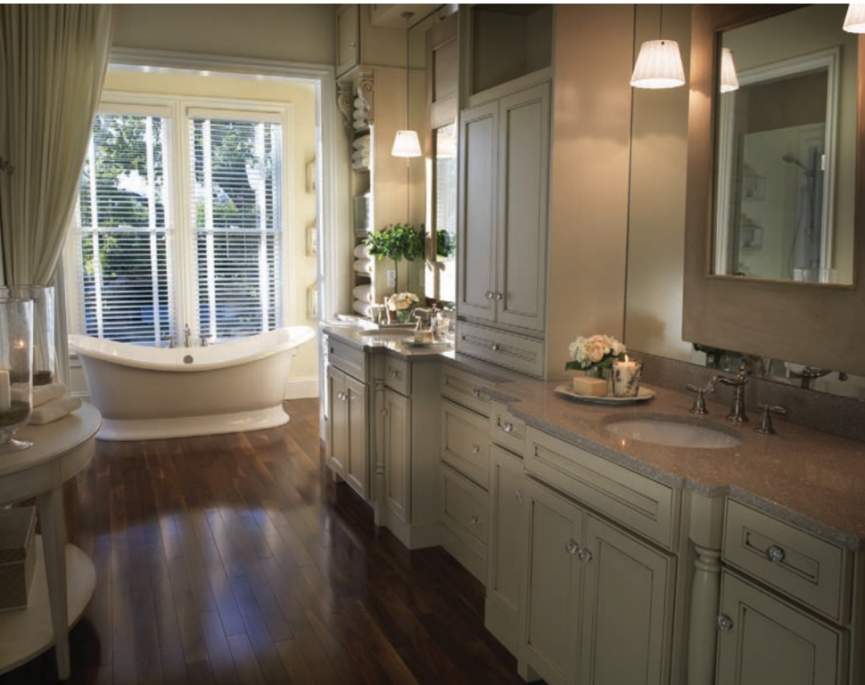
Figure 7.21 Finish plumbing is seen in this HGTV Dream House Master Bathroom as the free-standing bathtub and dual undercounter vanity sinks and dual control faucets. Photo HGTV
