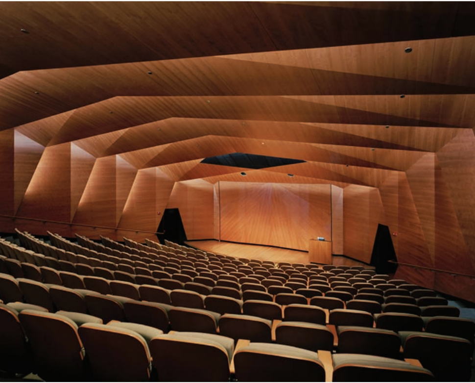
Figure 5.24 Cold-cathode fluorescent lighting is recessed into angled walls, creating a dynamic geometric architectural/lighting pattern in the Merck BRC Auditorium, Boston. Photo courtesy of NCC-National Cathode Corporation
