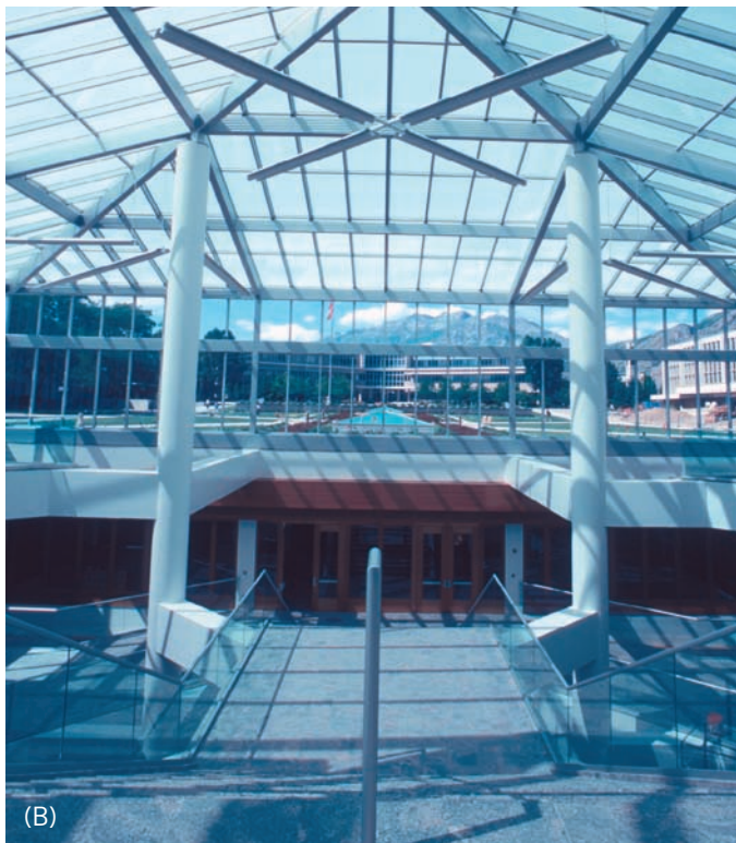
Figure 7.29 (A) The new addition to the old library, seen in the background at Brigham Young University, is underground. Three stories down, the new entry is in the glass enclosure at the back of the photo. A wall of windows and ground-level skylights bring natural light for studying into the first underground level. (B) Here the new main entrance is within a metal space framed enclosure, also called “curtain wall construction” where the curtain is glass. This enclosure feels much like a greenhouse space, counterbalancing the destination, which is the new library addition underground. (C) Students gather around a lit window well wall. (D) Inside the underground first story, these students study with the pleasant qualities of natural light from the window seen in photo (A). All courtesy of Brigham Young University
