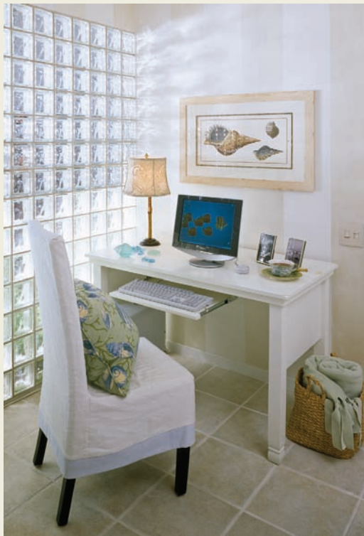
Figure 11.4 Glass block provides pleasant diffused daylight and privacy for a computer work area. Photo © Brian Vanden Brink
