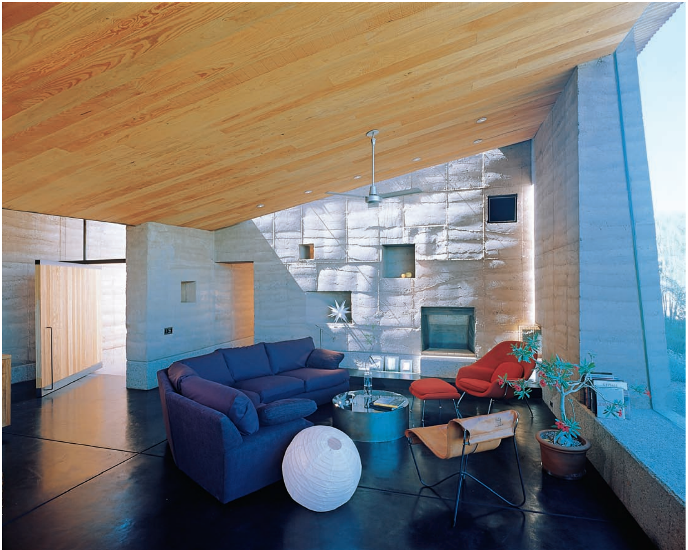
Figure 2.6 This contemporary Arizona home is constructed of rammed earth and makes use of a ceiling fan and natural light to minimize energy consumption. Palmer residence, Rick Joy Architect, Tucson/photo © Timothy Hursley/The Arkansas Office, Inc.
