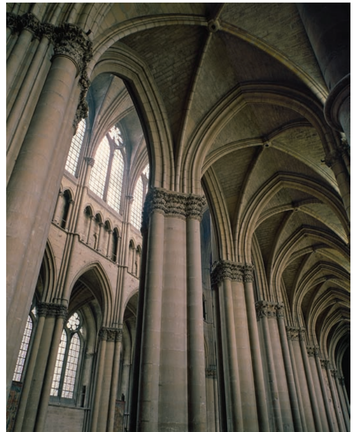
Figure 15.5 This view, from the aisle through the nave, provides a clear view of the arcade, the triforium, and the clerestory on the opposite wall of this Gothic church. Photo © Brian Vanden Brink
