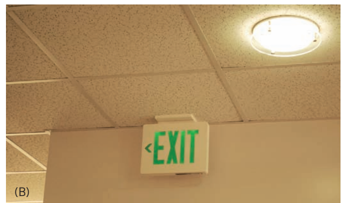
Figure 7.30 (A) The plenum is the area above the ceiling; here a suspended ceiling of acoustical tiles provides access to any of the systems in the plenum, including the lighting, heating/ventilation/air-conditioning (HVAC), the projection system, or the fire alert/sprinkling system. (B) Egress lighting must be visible both when the lighting works and when there is a temporary electrical outage or emergency, in which case the LED lights continue to operate to lead users to outdoor safety. Photo © Kathryn Taylor
