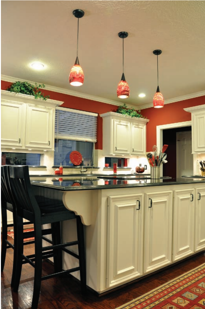
Figure 5.21 Beautiful red hand-blown glass minipendant diffusers accentuate the pools of light on the island bar of this Texas home. Recessed downlights and undercabinet light for evening illumination are balanced with windows over the sink and under the upper cabinets for daytime kitchen work. Photo © Kathryn Taylor
