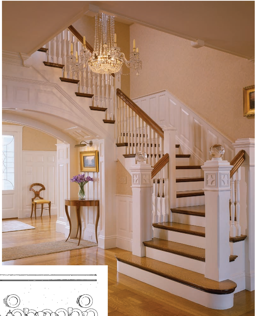
Figure 10.3 Traditional paneling is seen in the background at a wainscot level, as full wall panels behind the entry table, and around the stairs as a dado. Design by Seimasko + Verbridge/photo © Brian Vanden Brink
