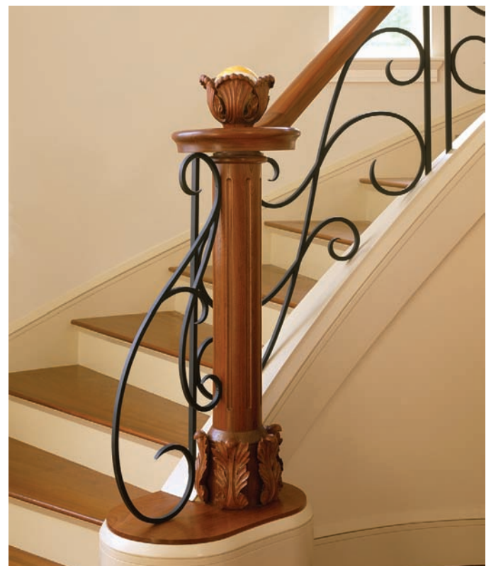
Figure 3.16 Flowing lines as balusters are the dominant element in this curved staircase balustrade. Design by Knickerbocker Group/ photo © Brian Vanden Brink
