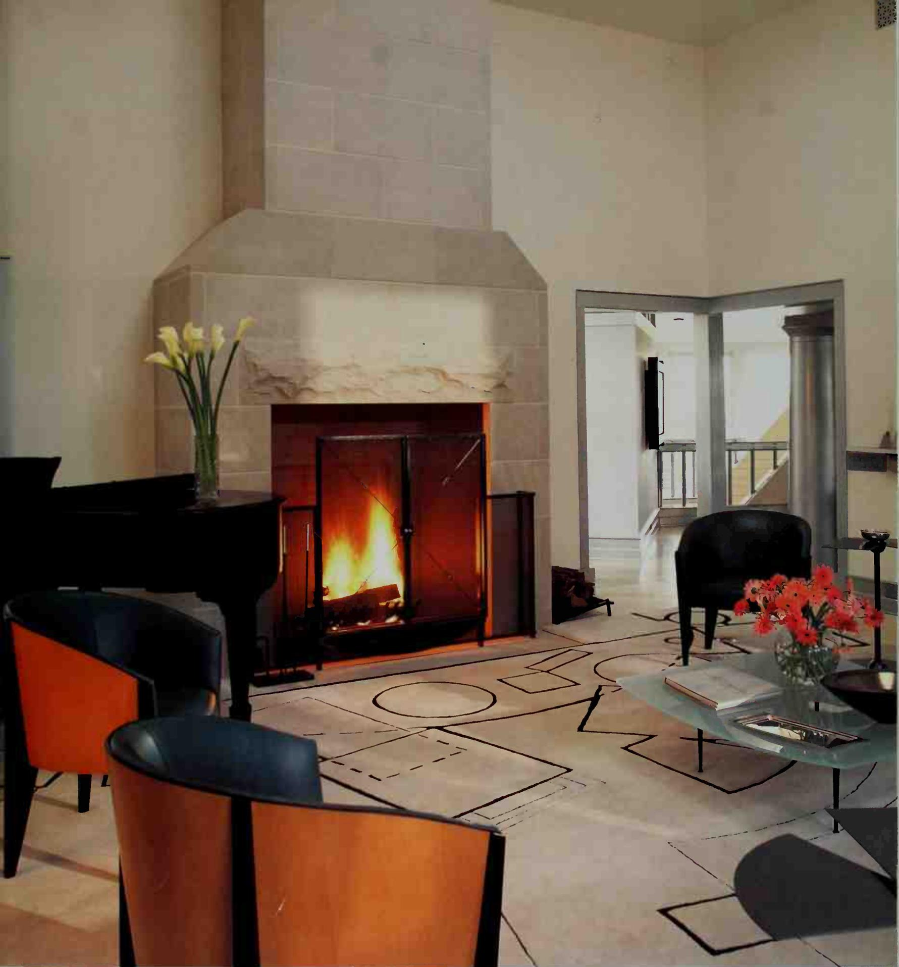
*The fireplace, based on a Count Rumford design, is made of limestone to match the exterior*
