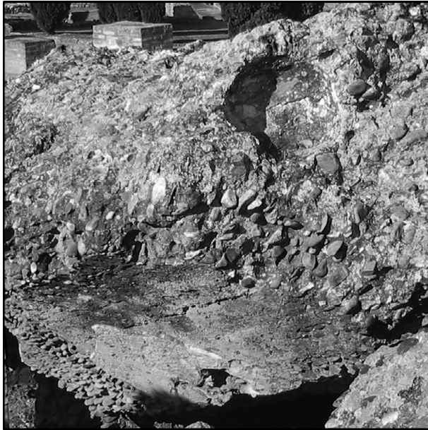
16. Casa de la Esedra at Italica, Spain (second century CE). Note the formwork imprints along the intrados and the use of smooth river stones set randomly in the mortar. The circular indentation at the top right is the impression of a Dressel 20 amphora, which was one of a number that were embedded in the vault (Lancaster 2005a: 70–71).
