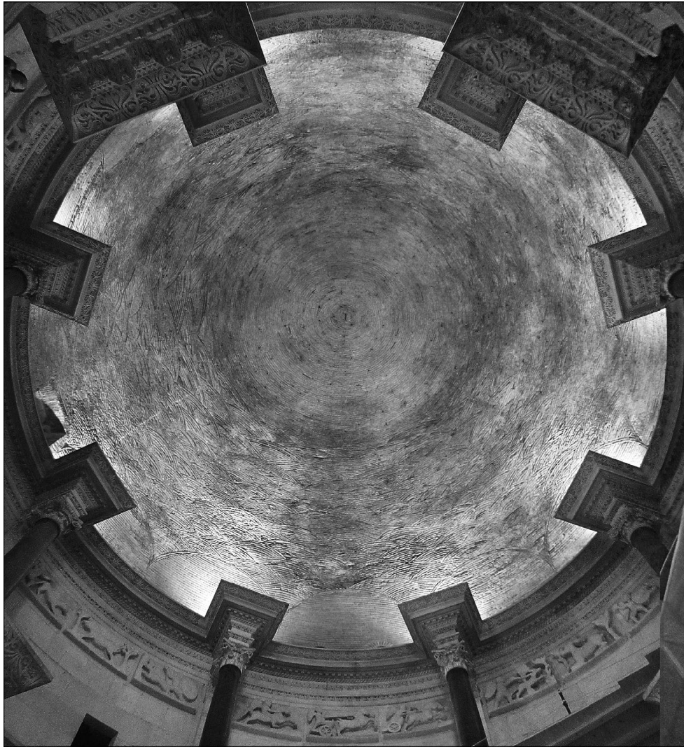
63. Mausoleum of Diocletian at Split, Croatia (c. 305 CE). The dome from below showing the fan construction and the spatial effect of the projecting cornice (photo: Goran Nikšić).
