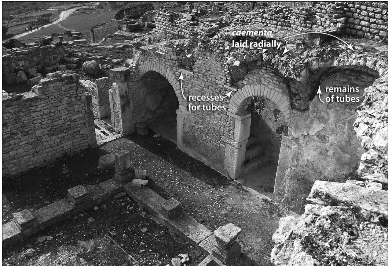
77. House of Dionysus and Ulysses at Dougga (ancient Thugga), Tunisia (second half of third century CE). Photo of remains of cross-vaulted portico built on shell of vaulting tubes. (Color image: WebFig. 25).
