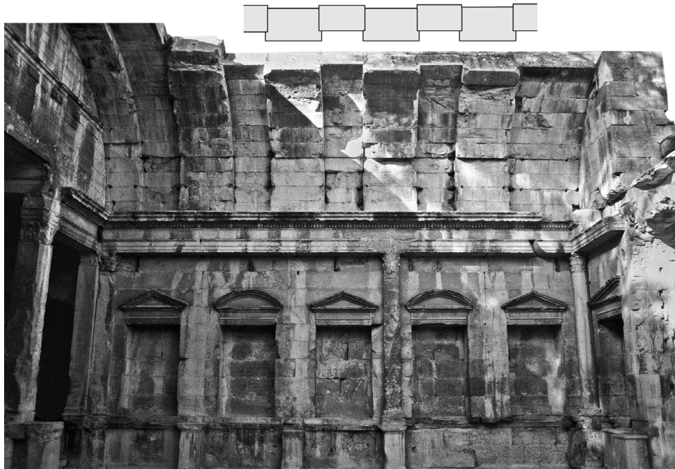
107. “Temple of Diana” at Nîmes, France. Barrel-vaulted roof built of stone armchair voussoirs supporting stone slabs in between. Above: diagram of block configuration in vault.
