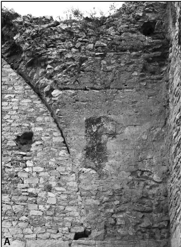
15. Examples of small irregular caementa laid radially. A: Entry vestibule in Baths of Julia Memmia at Bulla Regia, Tunisia (c. 230 CE) (see plan in Fig. 79). B: Bath at Antiochia in Pisidia, Turkey.
