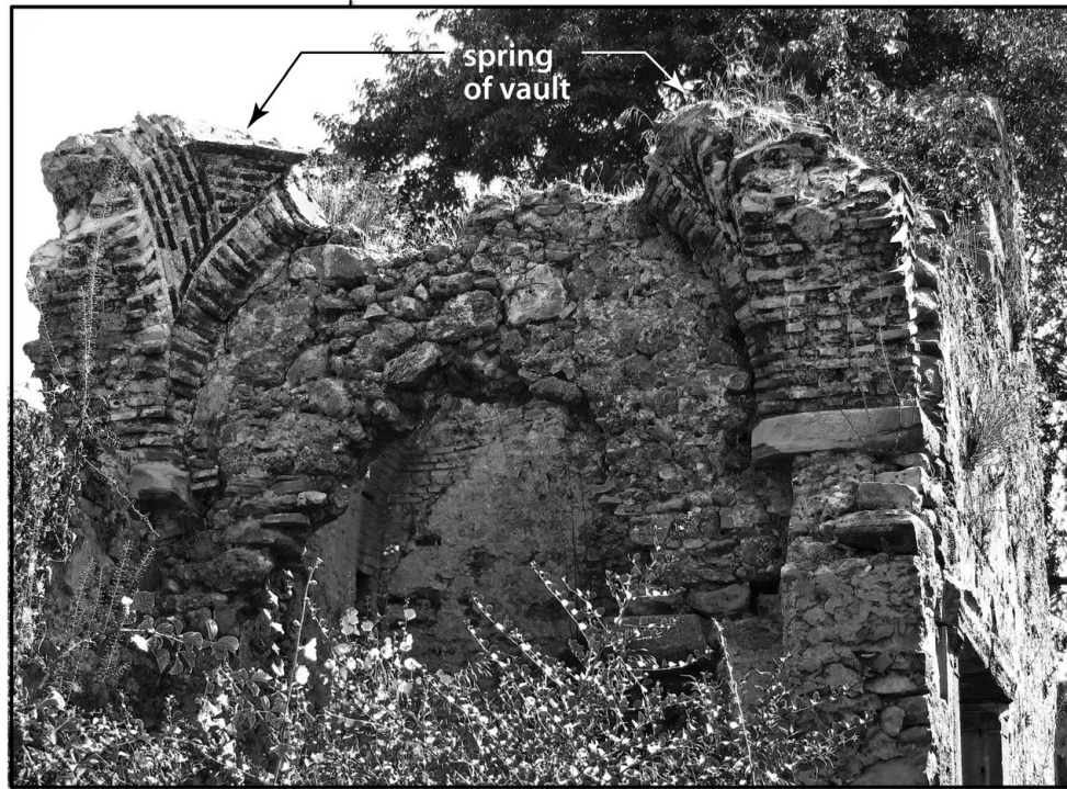
52. Plan of West Mausoleum at Side, Turkey, with a photo of remains of one of the sail vaults that once covered the north portico (plan based on reconstruction in Mansel 1963: Abb. 146).
