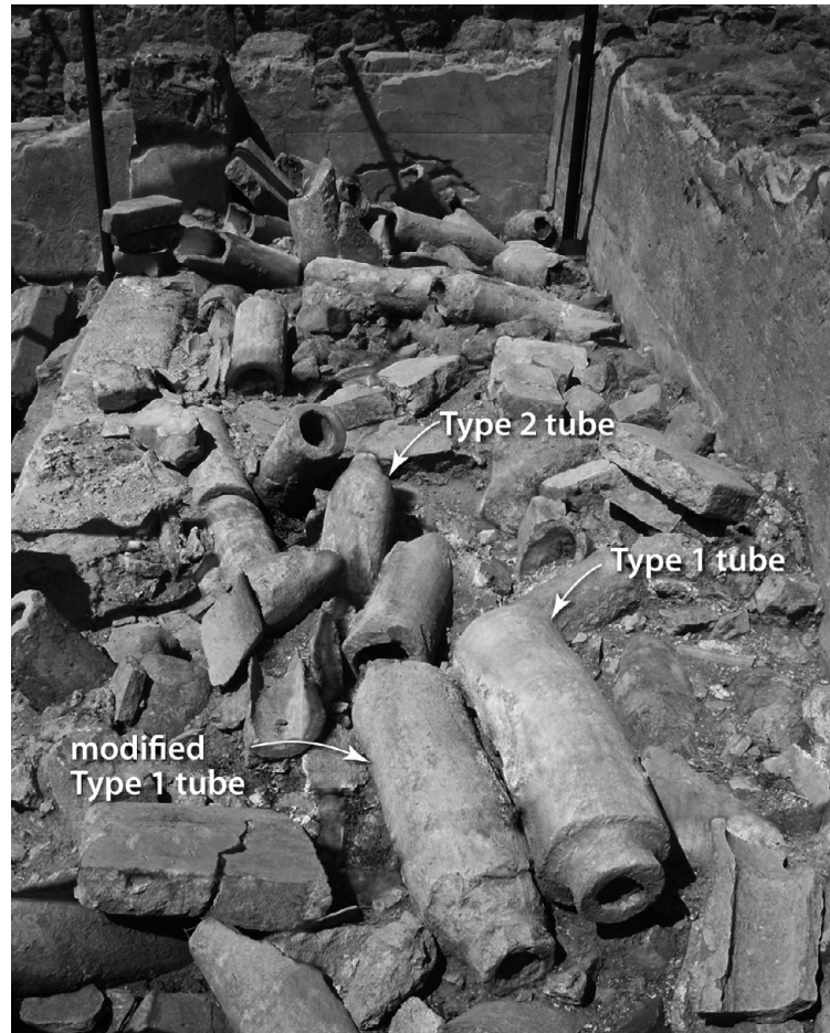
67. North Baths at Morgantina (mid-third century BCE). View of fallen vaulting tubes in the immersion bath of the caldarium showing a water pipe (Type 1) tube in the foreground with another next to it with the nozzle chiseled off to approximate a bullet-shaped tube (Type 2). In the background, a Type 2 bullet-shaped tube is visible (photo: Sandra Lucore).
