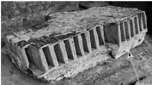
B extrados with small box-tiles in mortar
