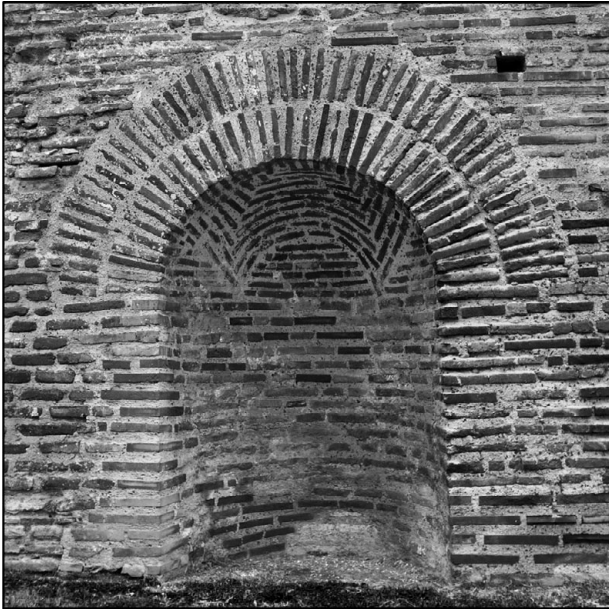
57. Rotunda of Galerius at Thessaloniki (early fourth century CE). Exterior niche with pitched brick along intrados.
