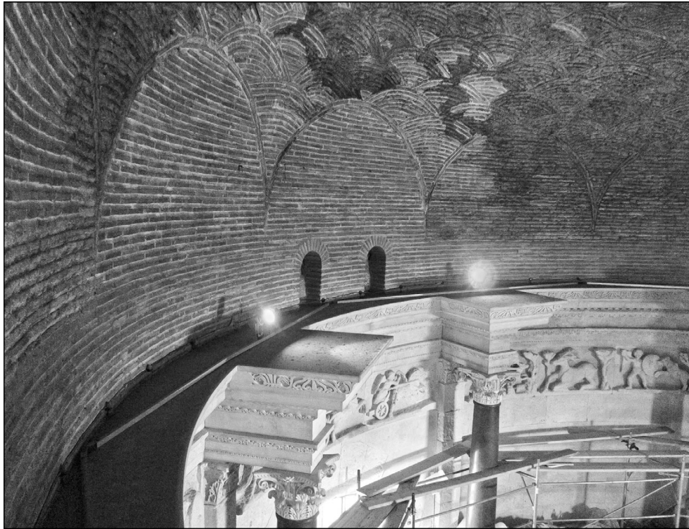
61. Mausoleum of Diocletian at Split, Croatia (c. 305 CE). View of the fan construction of the dome and the two (beam?) holes above the cornice.
