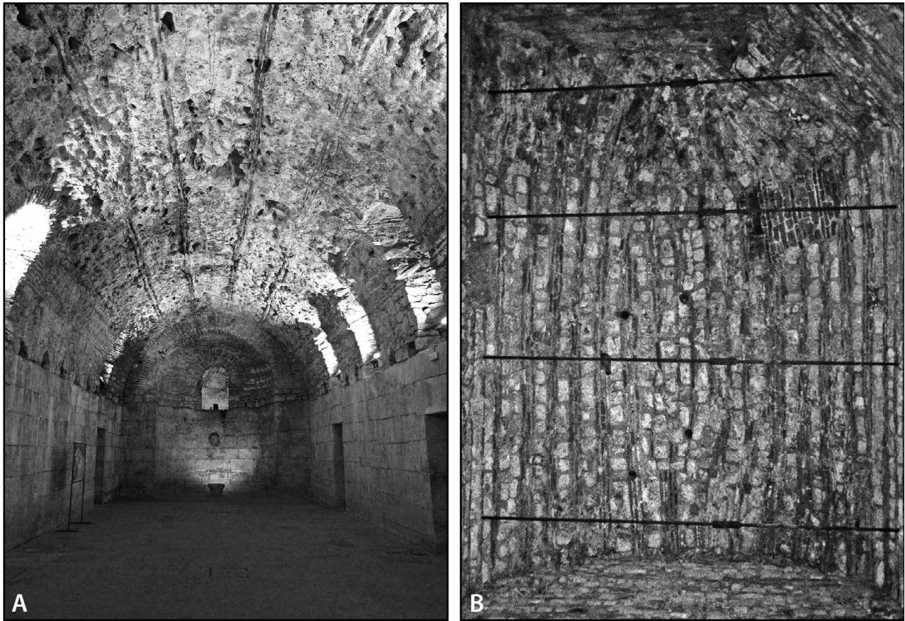
13. Examples of radially laid caementa combined with courses of radially laid brick. A: Substructures of the Palace of Diocletian at Split, Croatia (early fourth century CE). B: Praefurnium for caldarium of the Imperial Thermae at Trier, Germany (early fourth century CE). Note vertical tubes in vault for ventilation. The iron tie bars are modern. (Color image: WebFig. 6).
