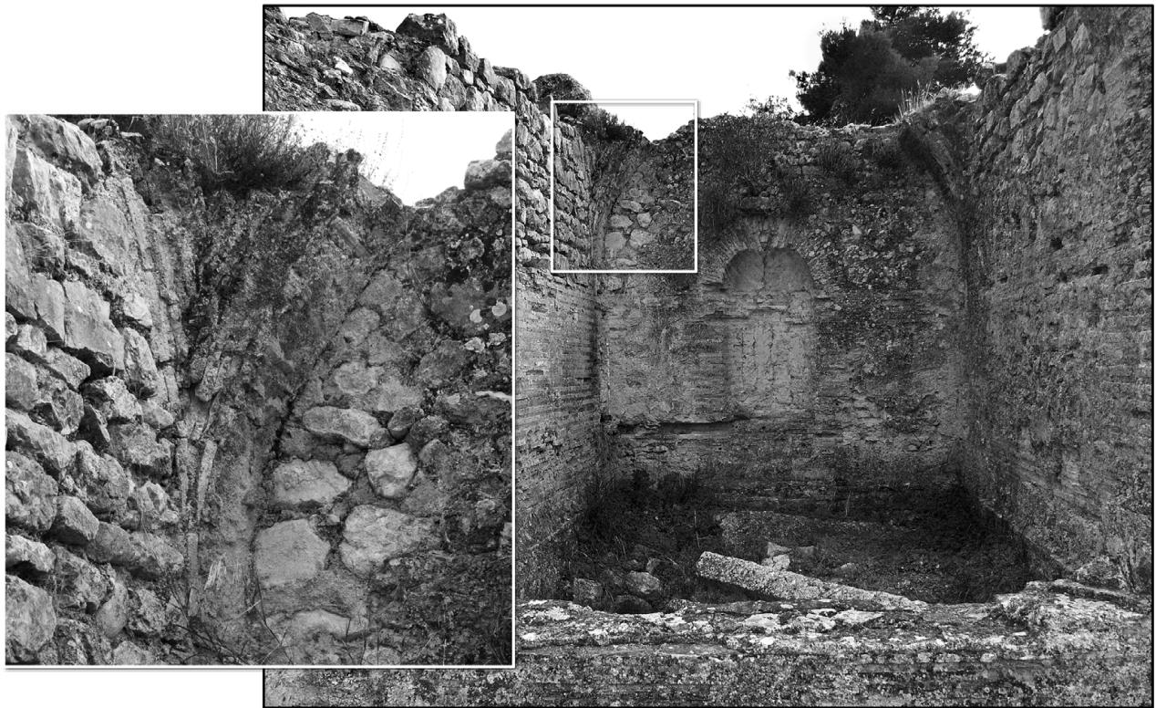
56. Northeast Baths in Sanctuary of Asclepius at Epidaurus, Greece (mid-second century CE). Pool of frigidarium covered by sail vault with remains of pendentive in inset. Note also the pitched brick construction of the semidome of the niche in the back wall. (Color image: WebFig. 21).
