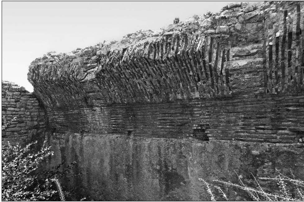
19. Remains of cistern vault at Rhodiapolis, Turkey. The section above the impost is laid radially with the holes for the centering beams still visible. In the upper parts the bricks are set vertically with occasional ribs of radial brick. Note that the radial brick ribs do not align with the centering holes.
