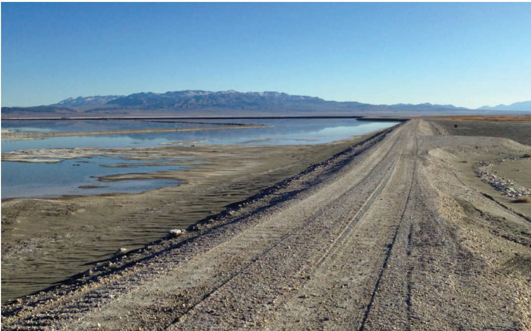
Figure 2.1 View of the Owens Lake Dust Control Project shallow flooding pond and berm road.
