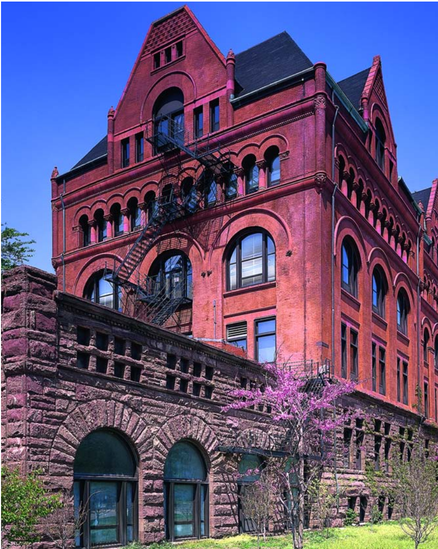
Original IIT Boiler Plant
