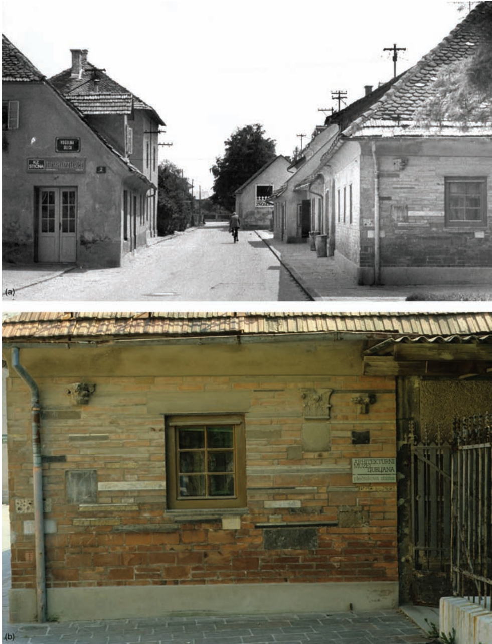
Figure 2.4 (a) Plečnik's house: street view. (b) Plečnik's house: walling detail.
