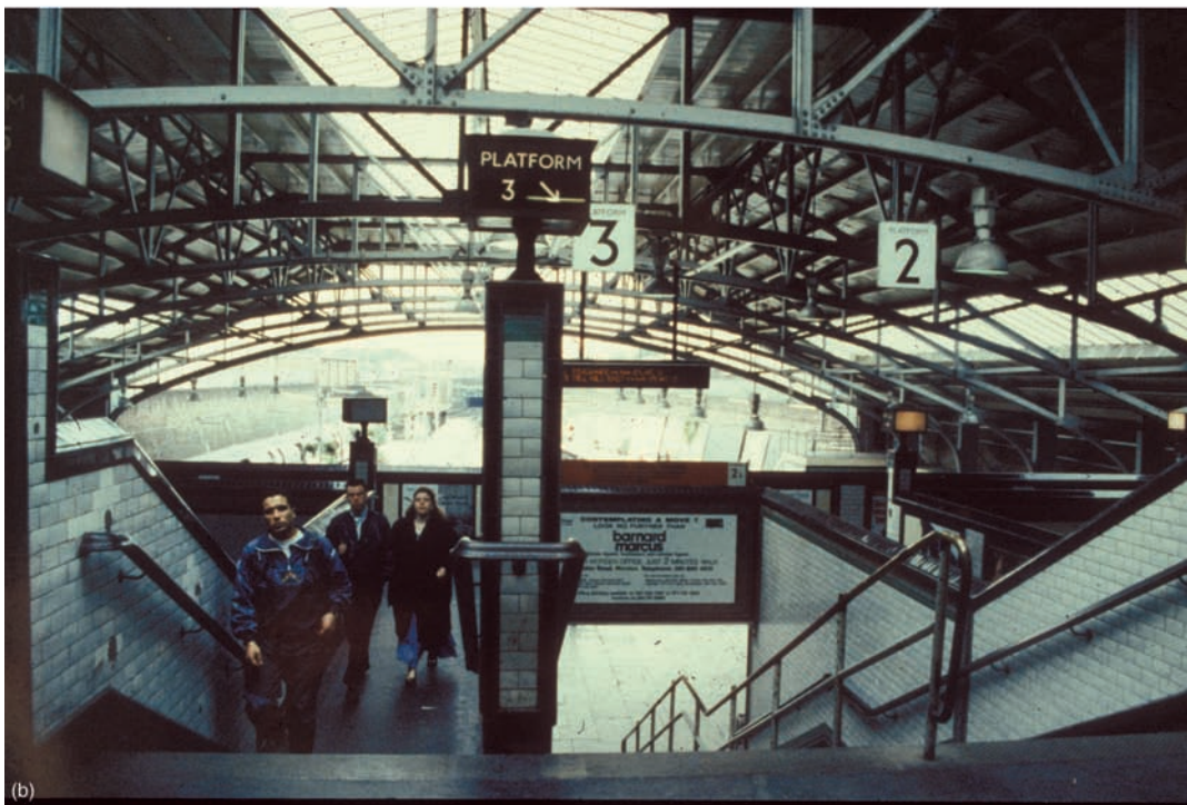
Figure 4.8 (a) The Morden booking hall. (b) Platform access at Morden.
