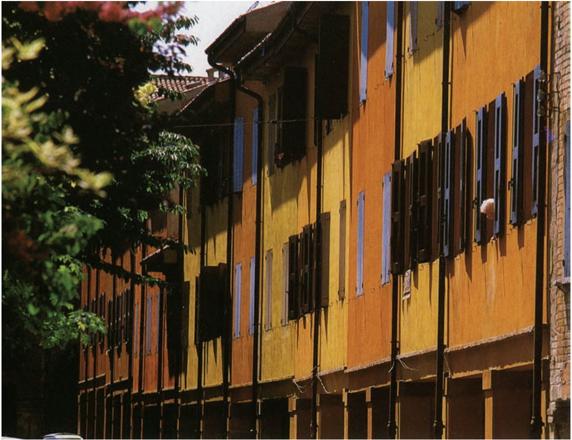
Figure 5.17 Restored houses in Via San Leonardo , near the University District.
