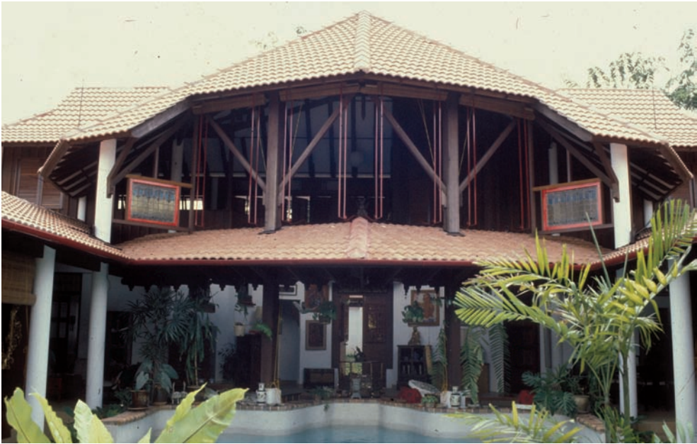
Figure 7.10 Precima House, the courtyard view.
