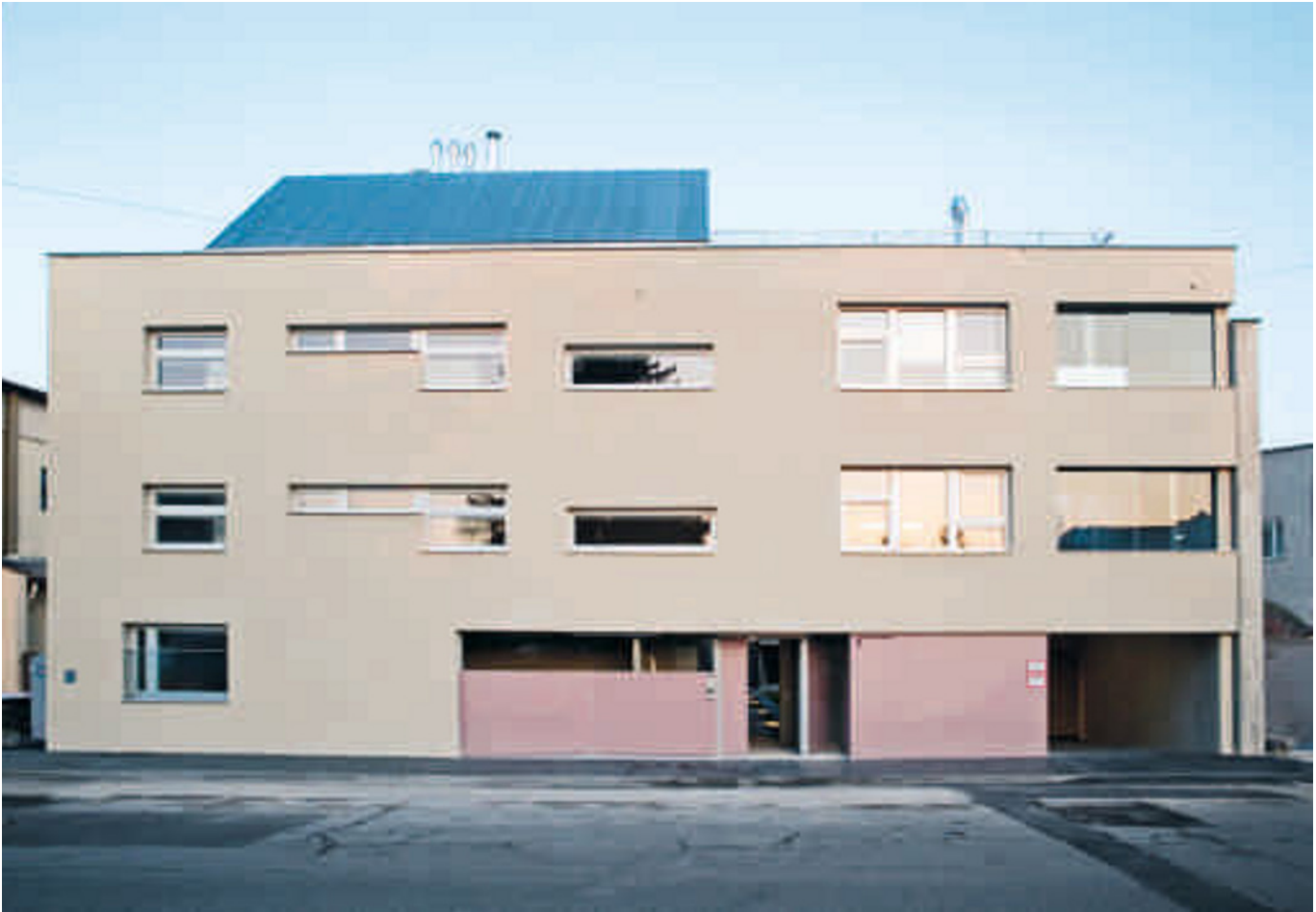
Residential Building Welingerasse Vienna, Austria, 2008
