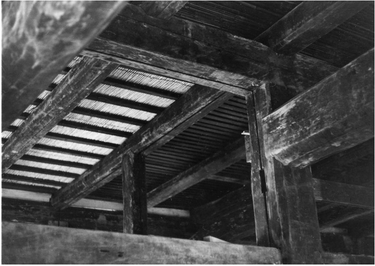
The central pillar and its massive beam-branches under the ceiling
