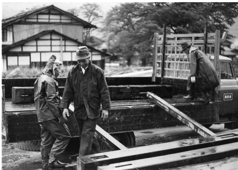
Disassembled and about to be trucked from Shirotori to Kamakura
