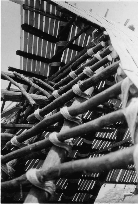
Innocent of nails, sturdy ropes secure the roof on its east side.
