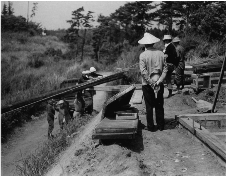
(top) A forty-five-foot beam, the first of many, rides on a two-ton truck to the site, Yochan at the wheel.
