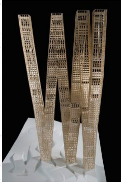
Typical tower configuration is inverted by reducing the footprint and maximizing the area of the upper levels.
