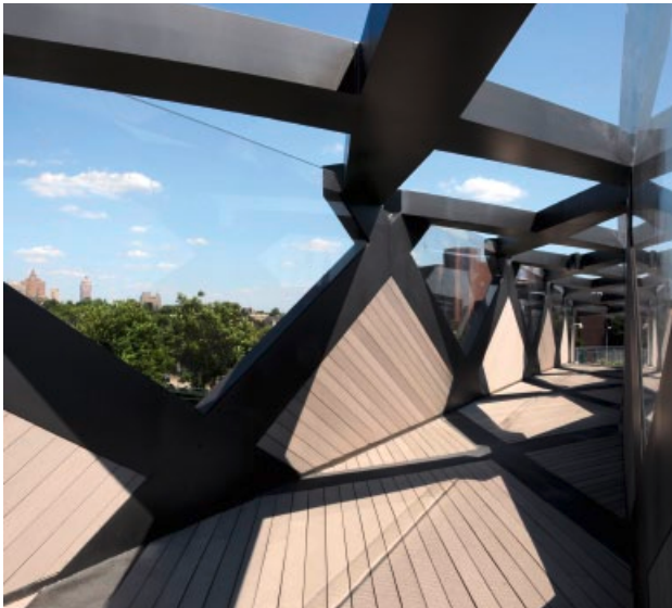
Figure 2. Arup AGU, Weave Bridge, University of Philadelphia, Pennsylvania, 2009 Interior view of the Weave Bridge with its interlacing steel structure and timber and glazed infill panels.
