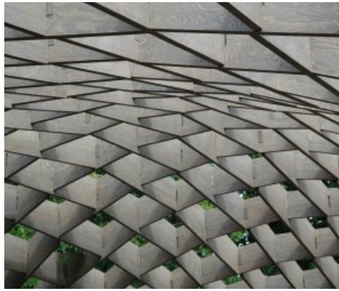
Figure 4. Alvaro Siza and Eduardo Souto de Moura with Arup AGU (Cecil Balmond, Daniel Bosia, Charles Walker and Lip Chiong), Serpentine Gallery Pavilion, Kensington Gardens, London, 2005 Interior of the 2005 pavilion with its reciprocal 'woven' pattern of flat timber beams.
