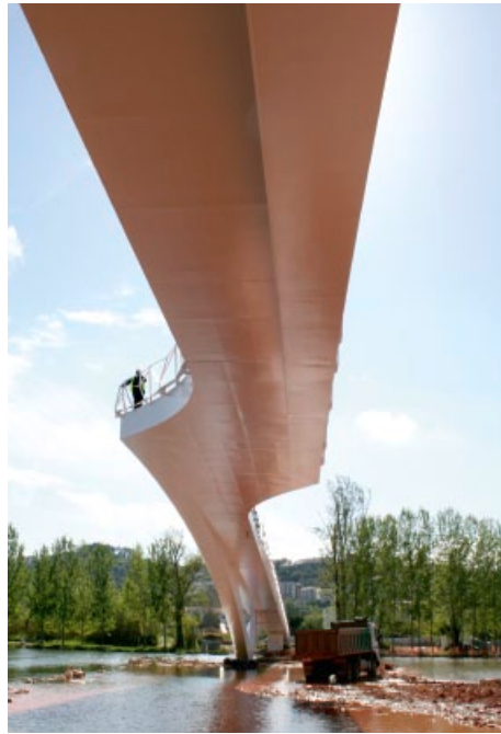
Figure 10. Arup AGU, Pedro and Inês Bridge, Coimbra, Portugal, 2007 View of the central 'floating' square with the folded balustrade pattern.
