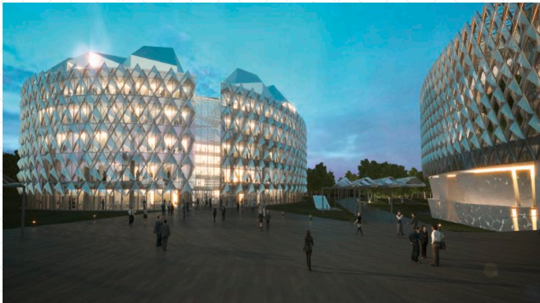
Foster + Partners, City of Justice, Madrid, 2007 The facades of both court buildings bear shading devices optimised to balance solar performance with views to the exterior.
