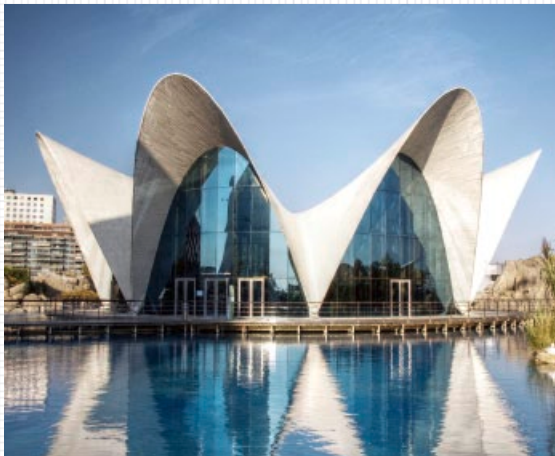
Figure 13. Félix Candela, L'Oceanogràfic, Valencia, Spain, 1998 A rich mixture of constructional logic, extraordinary structural performance and a compelling aesthetic that seems to work at any scale.
