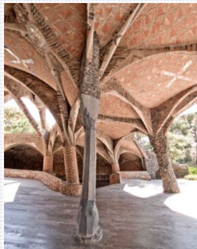
Figure 7. Antoni Gaudí, Colònia Güell Chapel porch undercroft, Santa Coloma de Cervelló, Catalonia, Spain, construction 1906–1912/14 In terms of doubly ruled surfaces, this building, at the middle stage of Gaudí's career, was his launching point. He uses singly ruled surfaces such as helicoids and hyperbolic paraboloids for both structural wall elements and decorative elements that assert the muscularity of the rib vaulting supporting the main staircase landing above and so forming the crypt's porch.
