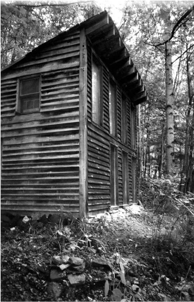
Fig. 20.1. The Long Branch pond cabin is naturally cooled, saving energy and money.
