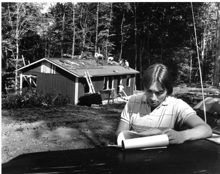
Fig. 21.1. A community center under construction near Clairfield, Tennessee
