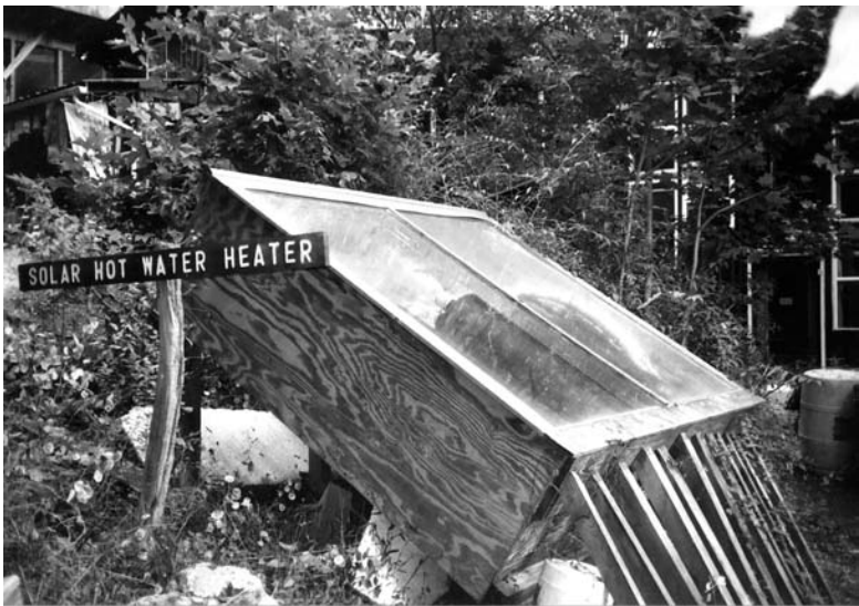
Fig. 5.1. Long Branch's solar hot water heater is of the breadbox type.
