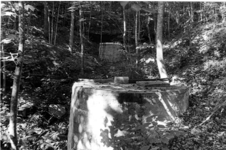
Fig. 29.2. ASPI cistern and sediment tank
