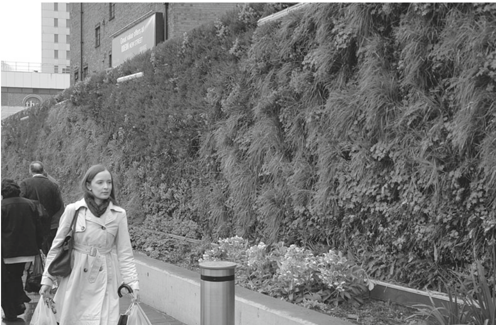
Figure 8.2. A green wall at the New Street (Rail) Station, Birmingham, UK. Credit: Photo by Tim Beatley.
