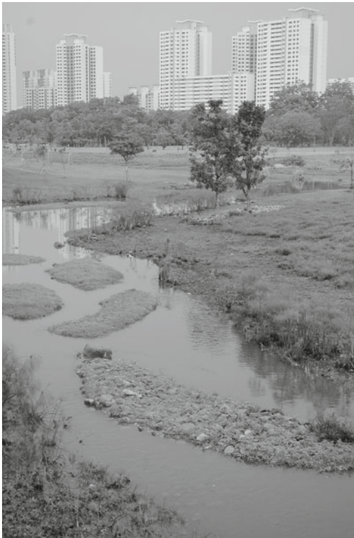
Figure 5.5. A former concrete drainage channel has been converted to a meandering Kallang River at Bishan-Ang Mo Kio Park. Credit: Photo by Tim Beatley.
