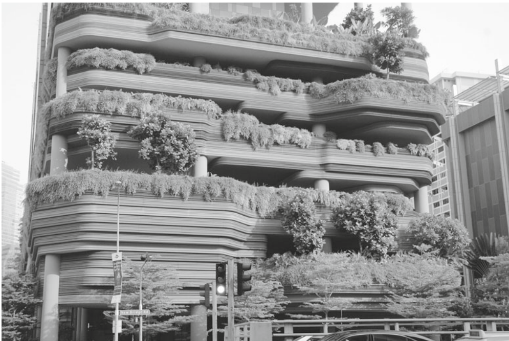
Figure 5.3. A View from the street of the PARKROYAL at Pickering Hotel in Singapore. This building incorporates more than 200 percent of the site in the form of vertical greening. The green features have done much to make this an attractive hotel to stay at, and the hotel has been able to double the projected room rate almost from the date the hotel opened. Credit: Photo by Tim Beatley.
