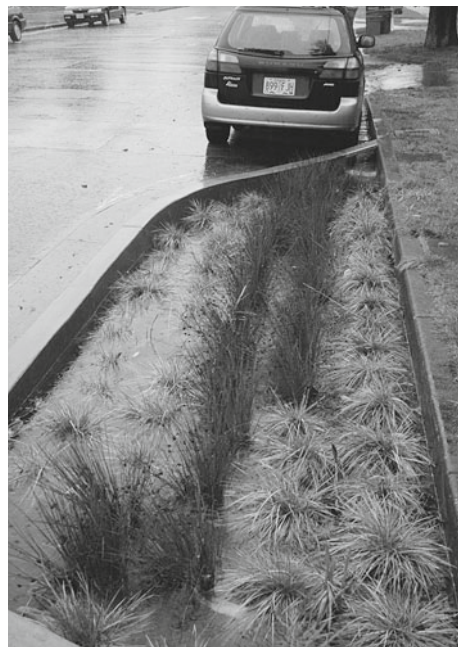
Figure 9.1. One of the more than 1400 green streets in Portland, Oregon. These bioswales collect stormwater and also provide an important measure of nature in this compact, walkable city. Credit: Photo by Tim Beatley.
