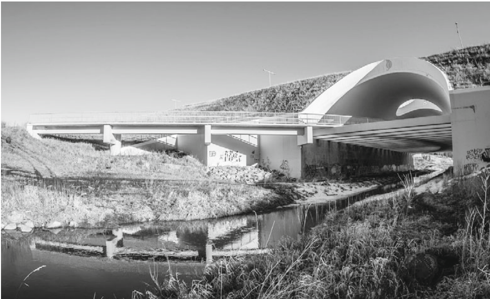
One of the growing number of wildlife passages in Edmonton, Alberta, Canada. Photo Credit: City of Edmonton.
