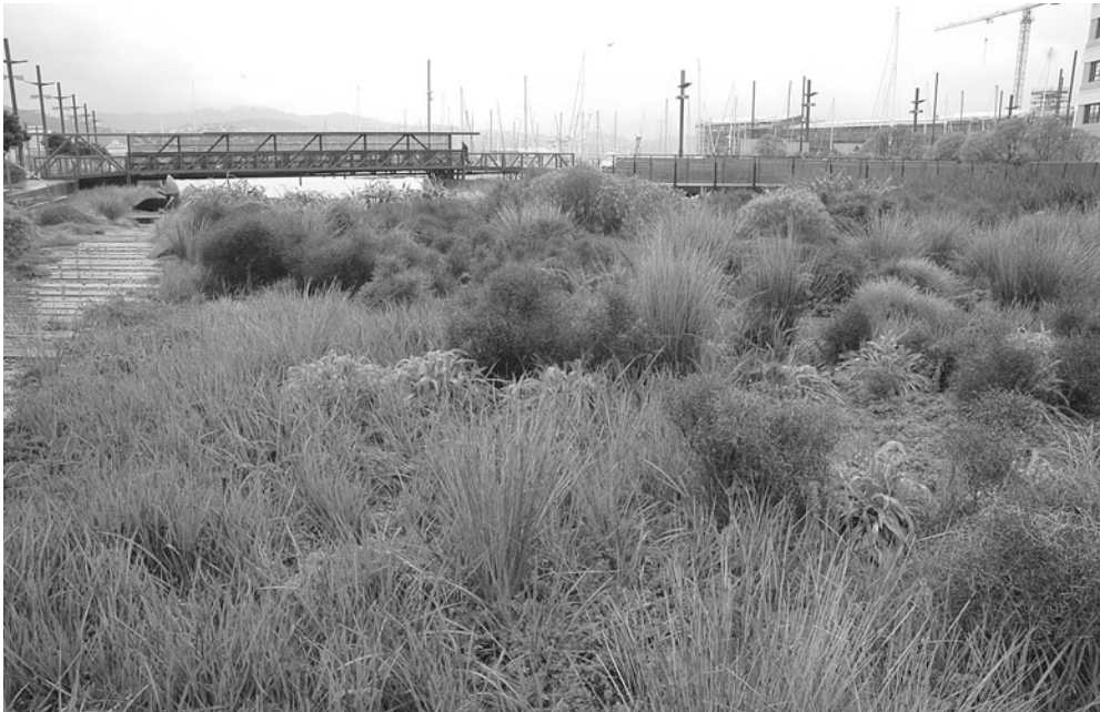
Figure 7.2. The Waitangi Wetlands Park, Wellington, New Zealand, is 6 hectares (15 acres) of sloped terraces adjacent to the city’s harbor. Planted with native plants, the wetlands collect and treat stormwater runoff and provide new water-adjacent public spaces. Credit: Photo by Tim Beatley.
